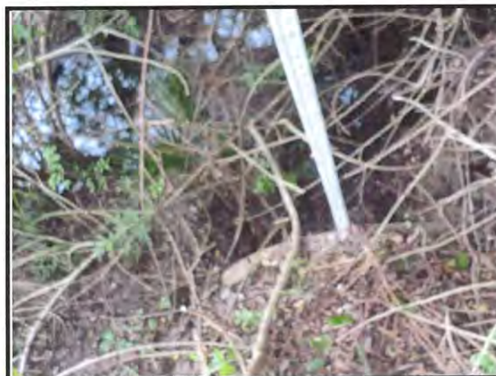
Existing East End of Cross Drain at MP 223.01
