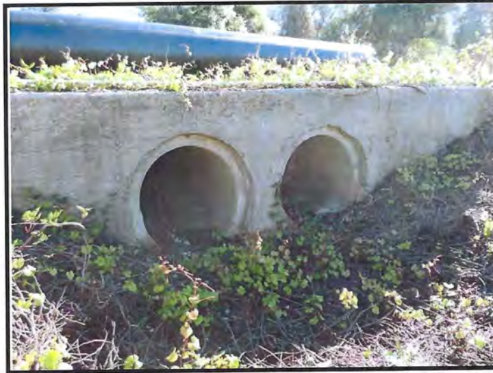
Looking at West (Upstream) Endwall and Double 42" Culverts at MP 191.17
