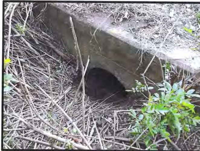
Existing Headwall East Side of Cross Drain at MP 183.22
