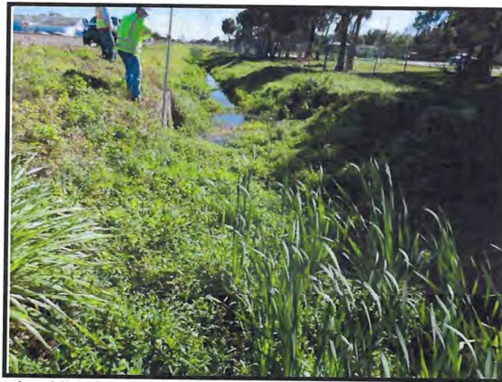
Looking South at West Headwall of 3 – 24" RCP Pipes
