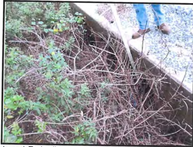
West (Upstream) Endwall and Five 30" by 33" RCP Culverts at MP 179.50
