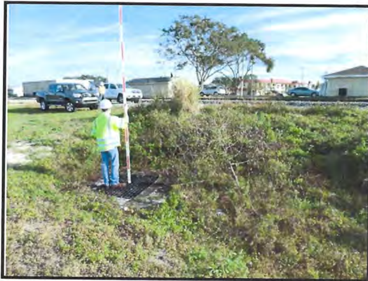
Looking East Across the Catch Basin West of the FEC ROW (The 54" Steel Culvert Installed by FDOT Connects this Catch Basin with the One Shown Above on the Eastern ROW)
