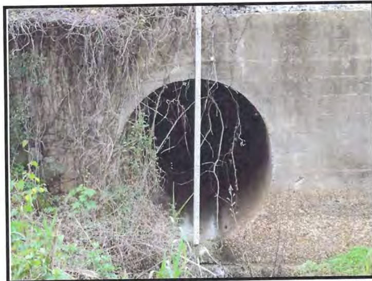
Looking at East Headwall of Southernmost 66" x 60" RCP.
