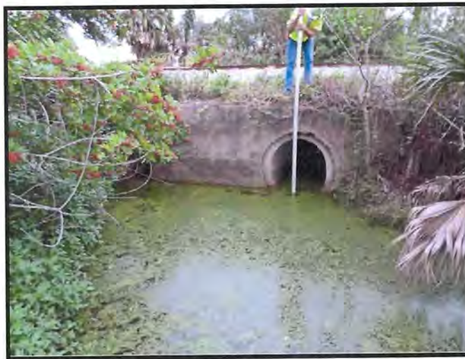
West (Upstream) Endwall and Double 36" RCP Culverts at MP 187.69
