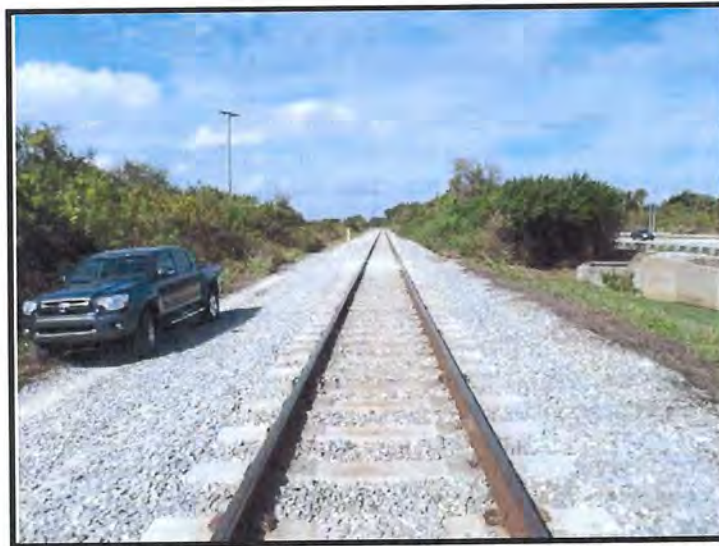
Looking North from MP 177.03A. Note Concrete Box on East Side of Track 150 feet North of Double 36" RCP. This is the Discharge for the "Unknown" 72" RCP From Canal West of FEC ROW (MP 177.03B)
