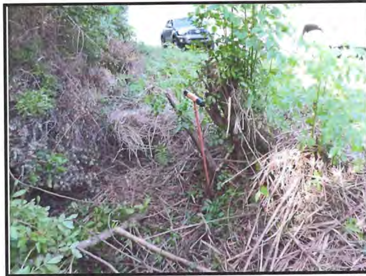
Approximate West (Upstream) End of Buried Cross Drain at MP 205.70
