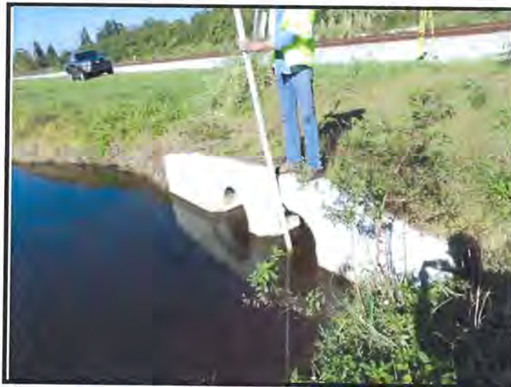
West (Upstream) End of Cross Drain MP 195.73 and West Endwall
