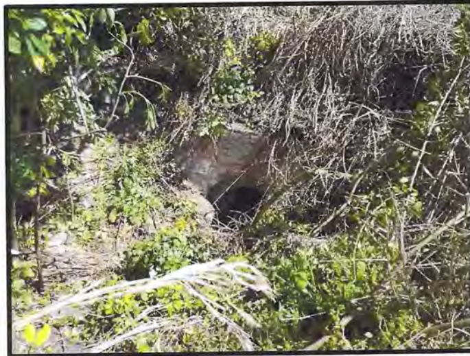
Western Headwall of 24" by 27" Oval RCP Culvert at MP 215.06
