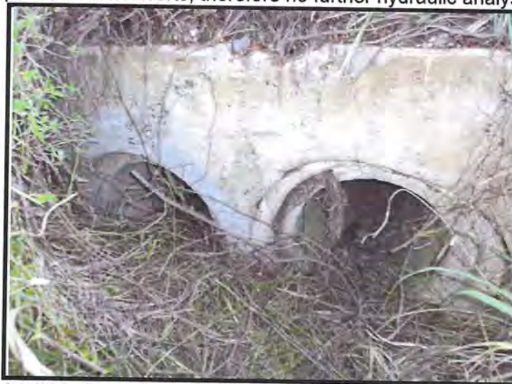
Looking at MP 230.51 West Headwall and Upstream Side of Double 24" by 27" RCP Culverts
