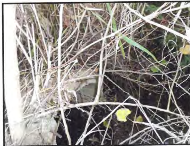
East (Downstream) End of 2 – 42" by 46" RCP Cross Drains at MP 207.80
