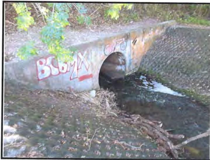
MP 190.87 West Endwall and Upstream Side of Single 72" Steel Culvert
