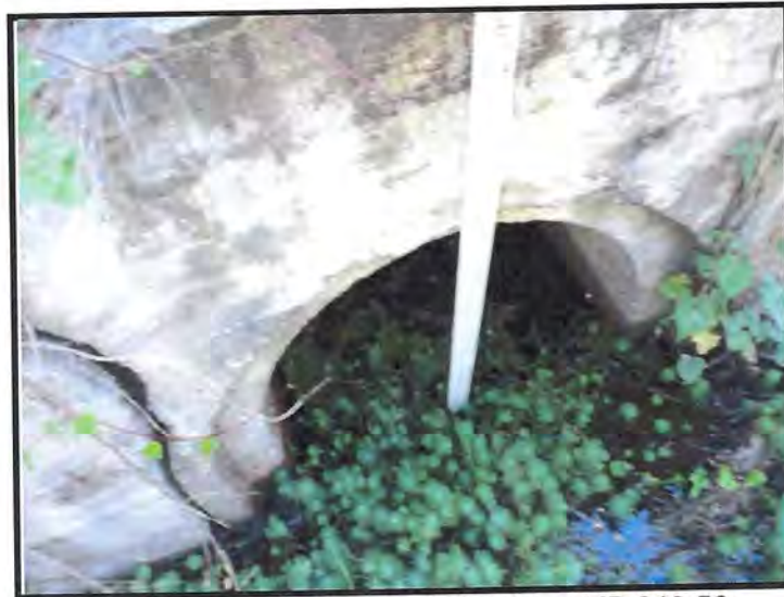
West Headwall of 42" by 46" RCP at MP 219.56
