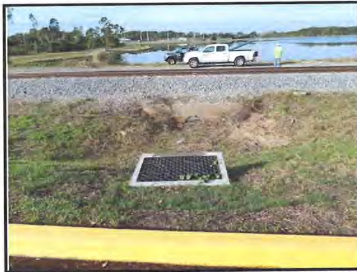
East End of Grouted Culvert and Catch Basin on Eastern FEC ROW (The 54" Steel Culvert Installed by FDOT Connects this Catch Basin with the One Below Outside of the Western ROW)
