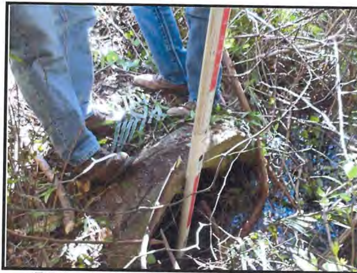
Existing West End of Cross Drain at MP 232.64
