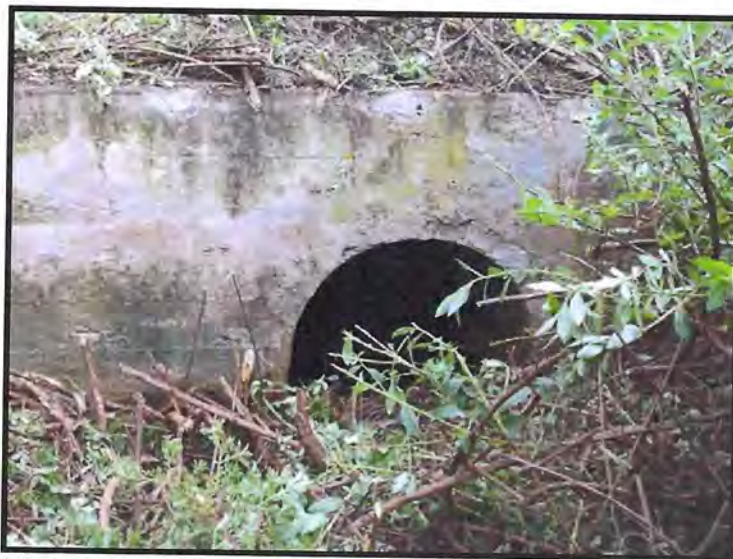
Existing Headwall on East Side of Cross Drain at MP 231.27
