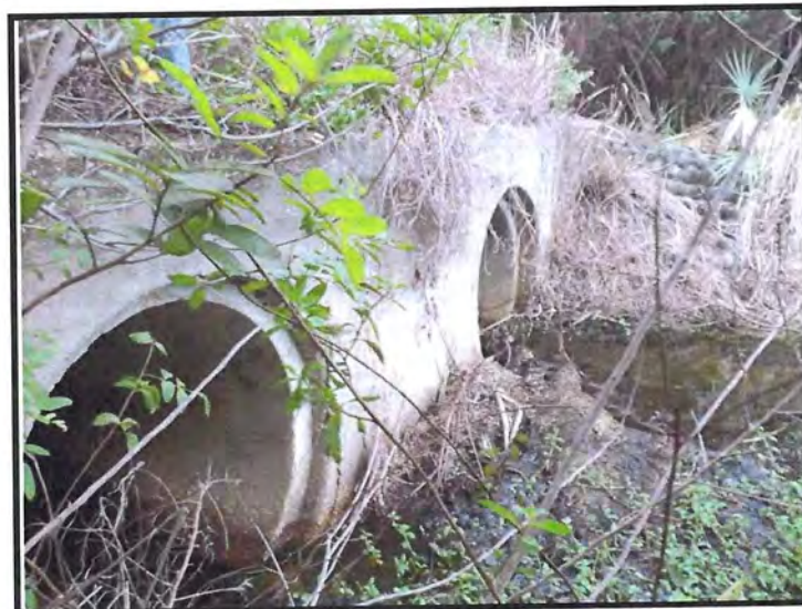
West (Upstream) End of Double 48" by 54" Culverts at MP 183.01
