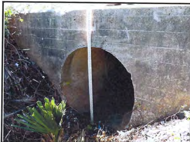
East (Downstream) Headwall at 60" RCP Cross Drain at MP 191.66
