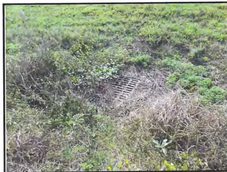
West (Upstream) Grate Inlet at MP 206.55
