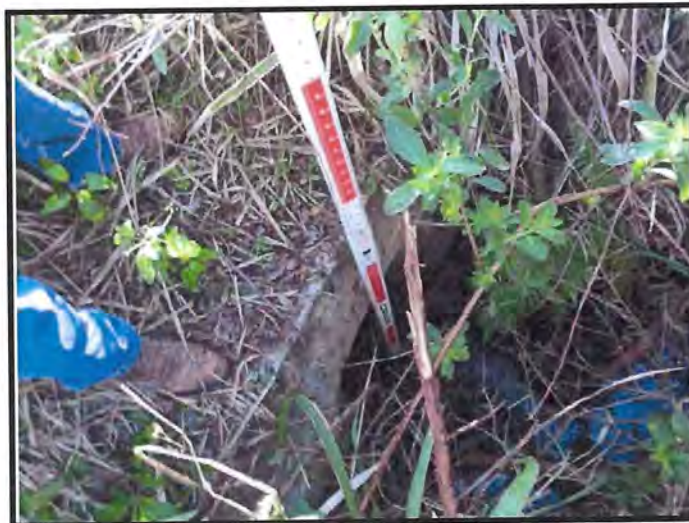
Existing West Endwall and End of Cross Drain at MP 218.56
