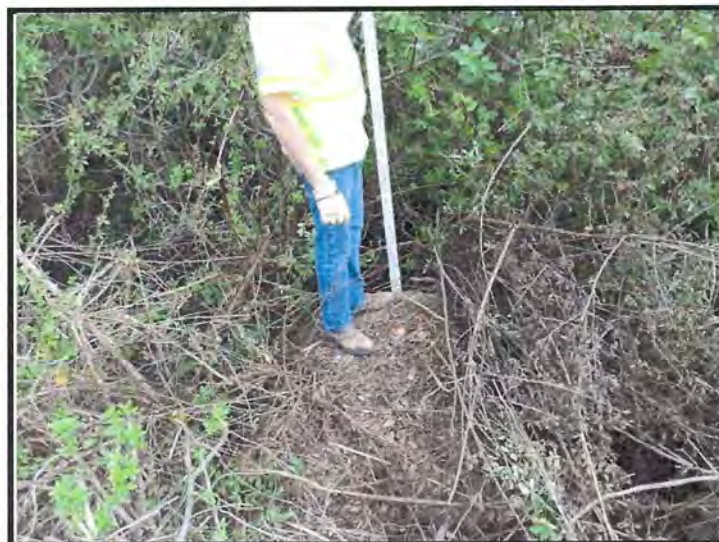
East End of Cross Drain at MP 222.88 and Adjacent Ditch
