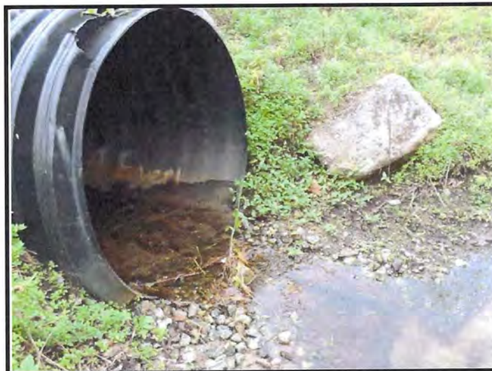
Existing 54" HDPE Draining Northward and Running Parallel to the Track on Upstream (West) End of Right of Way
