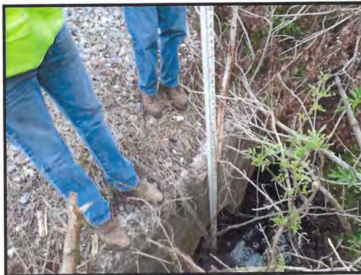
Headwall on Eastern End
