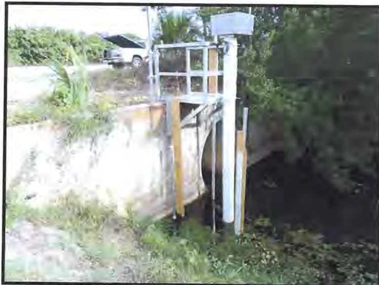
Western End of 72" RCP Culvert Showing Headwall, Staff Gauge and Monitoring Station
