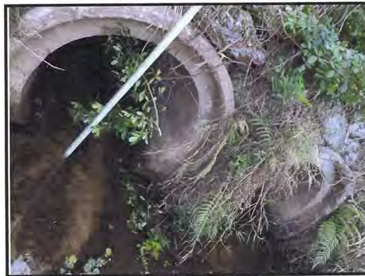
West (Upstream) End of Triple 42" by 46" Culverts at MP 184.02
