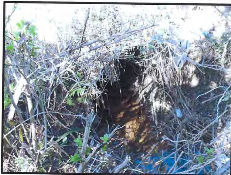
East (Downstream) End of 42" by 48" RCP at MP 211.32
