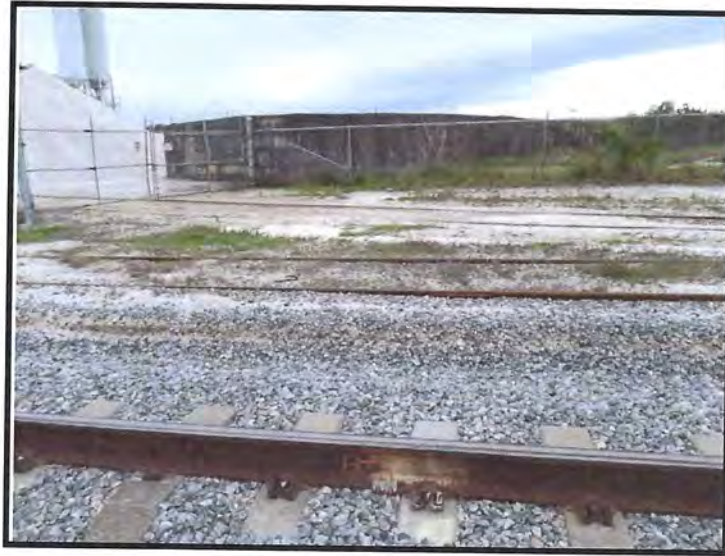
Concrete Mix Plant (West of Rail). Site of Former Ditch Draining to Cross Drain from the West
