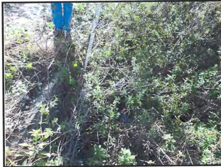
West (Upstream) Endwall and 3 - 84" by 90" RCP Cross Drains at MP 203.29
