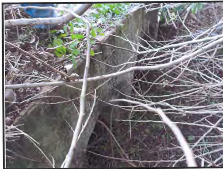
West (Upstream) End of Triple 24"x30" Culverts at MP 224.25
