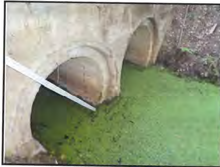
Looking at West Headwall at 2 - 54" RCP.
