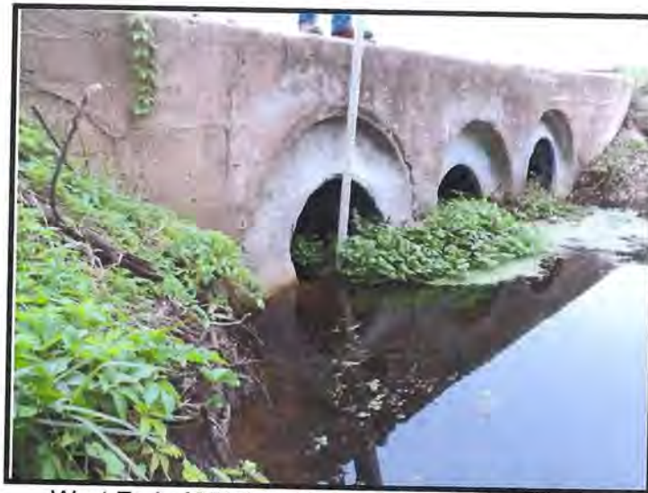
West End of MP 189.12 Cross Drain and Endwall
