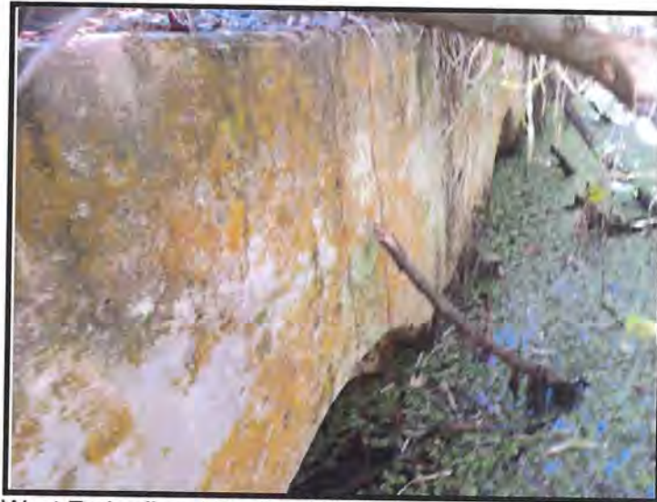
West Endwall and Double 48" RCP Culverts at MP 231.86
