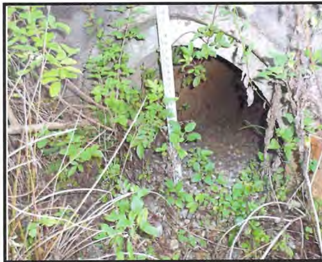
Looking at West Headwall at 42" RCP.
