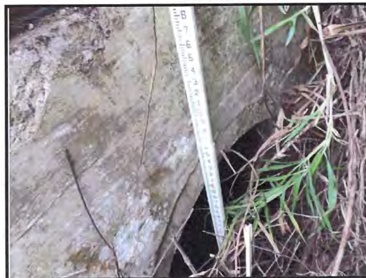
East Endwall of Double 48" RCP Culverts at MP 221.42
