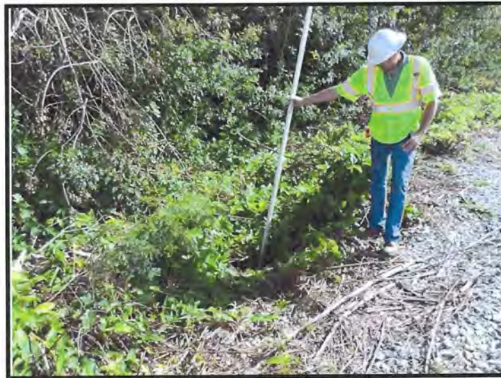
East End of Cross Drain at MP 205.40
