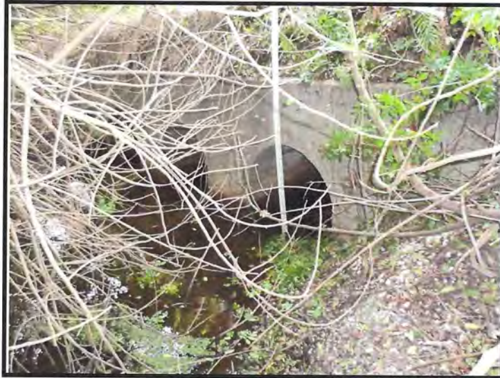
East (Downstream) End of Triple 42" by 46" Culverts at MP 184.02
