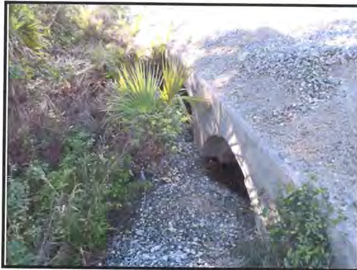
East (Downstream) Endwall and 3 - 84" by 90" RCP Cross Drains at MP 203.29
