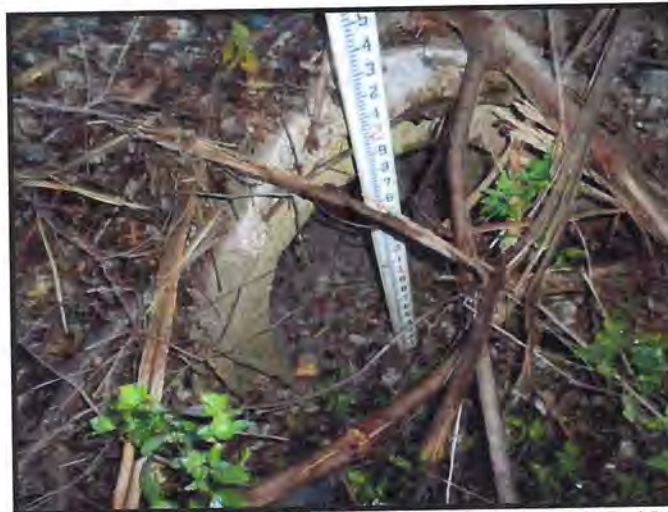
East (Upstream) End of 24" RCP Cross Drain at MP 190.17
