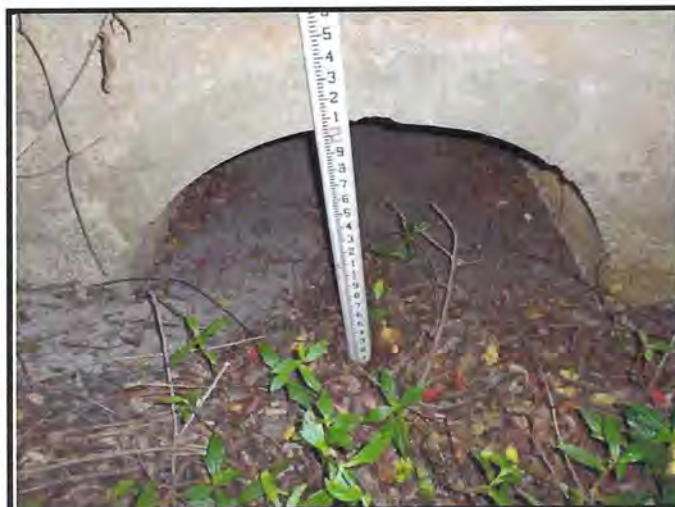
Looking at East End Headwall at 42" RCP.
