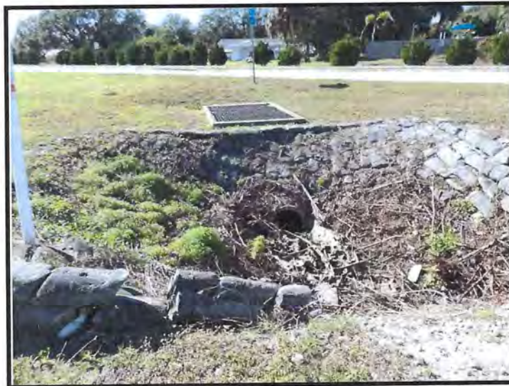
Looking Westward at Sump Area West (Upstream) of the Western End of the MP 214.85 Cross Drain. Picture Shows Junction Box and 24" RCP Discharge from CR 512 Pond System.
