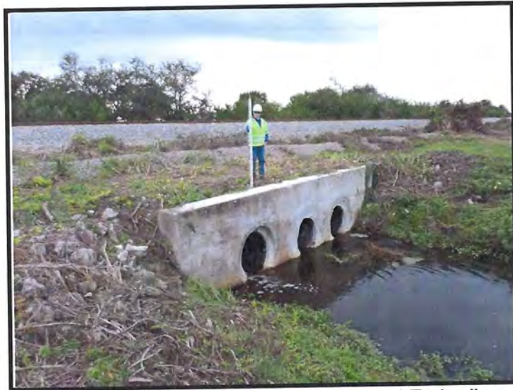
East End of MP 189.12 Cross Drain and Endwall
