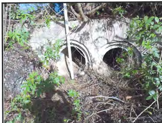
West (Upstream) Endwall of Double 24" RCP Culverts at MP 205.90
