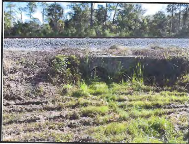
West (Upstream) Endwall and 42" by 48" RCP at MP 211.32
