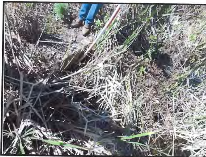
East Endwall and Double 36" RCP Culverts at MP 213.59
