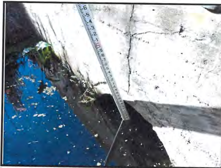
Existing Endwall and East End of Cross Drain at MP 232.64
