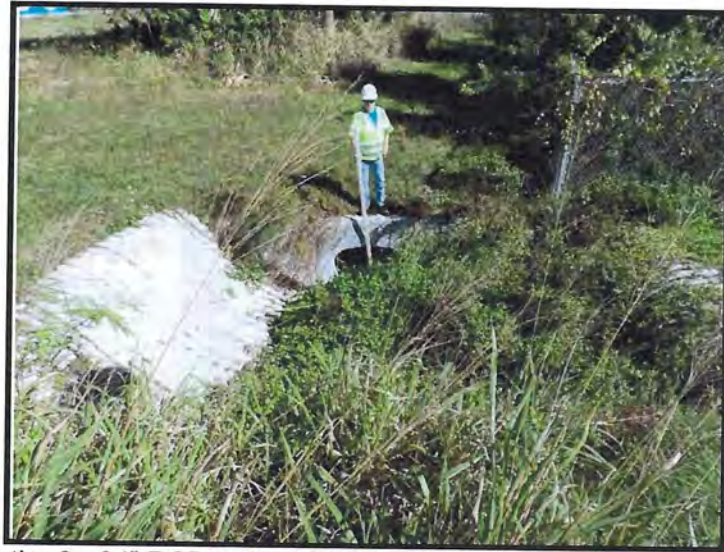
Looking East From the 3 - 24" RCP to the 36" x 54" ERCP Pipe that Carries Discharge From the Cross Drain to the East
