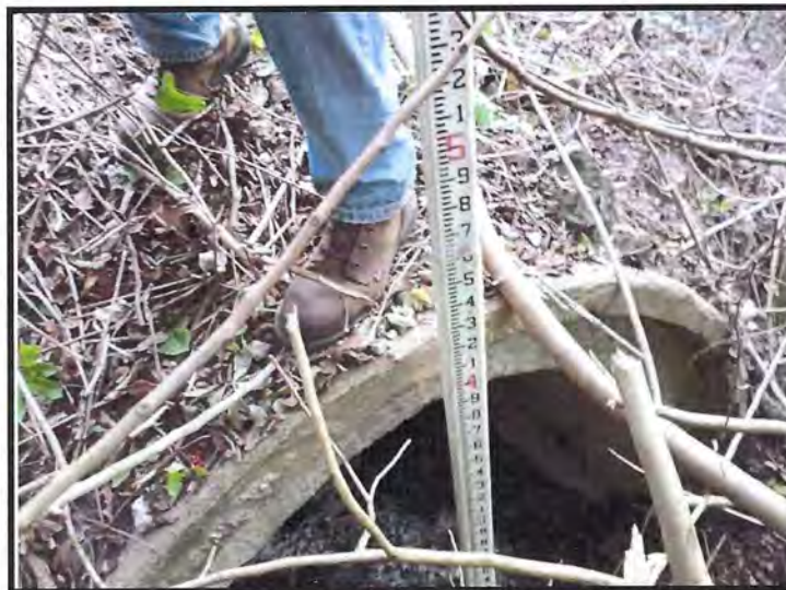
Existing West End of Cross Drain at MP 223.01
