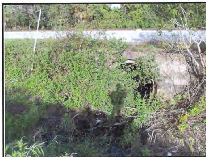
West (Upstream) Endwall and 2 - 84" by 90" RCP Cross Drains at MP 207.09
