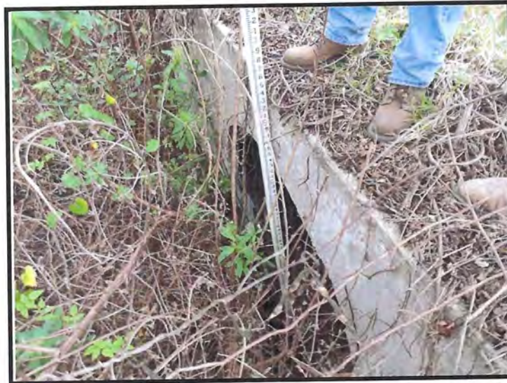
Looking at West Headwall at Southernmost 66" by 60" RCP.
