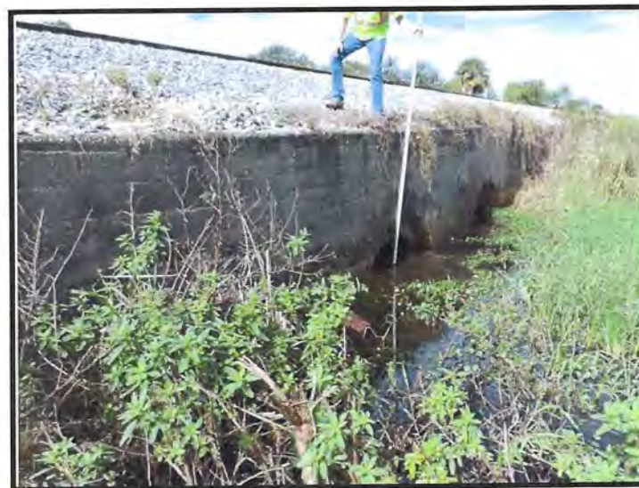
MP 205.01 East Endwall and Downstream Side of Culverts
