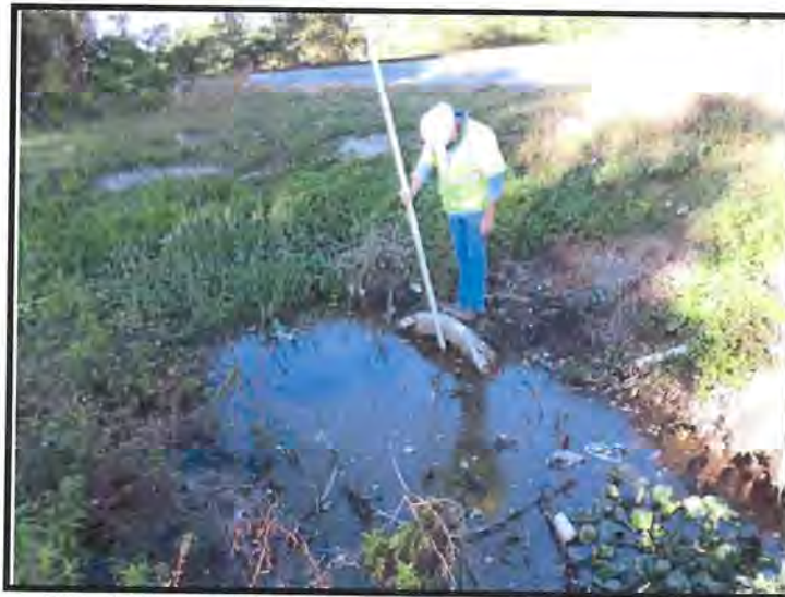
West (Downstream) End of Cross Drain MP 198.32
