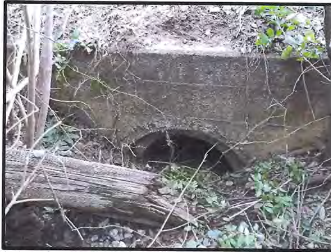
Existing Headwall West Side of Cross Drain at MP 183.22
