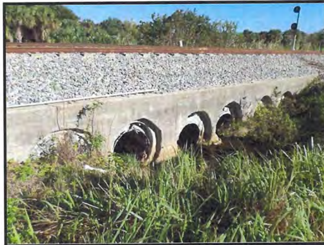
West (Upstream) Endwall and Cross Drain at MP 197.24. Note: Adjacent Capped Culverts.
