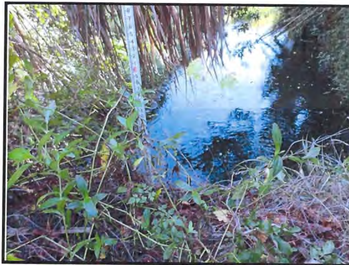
Receiving Ditch at MP 190.87 (East of FEC Rail)
