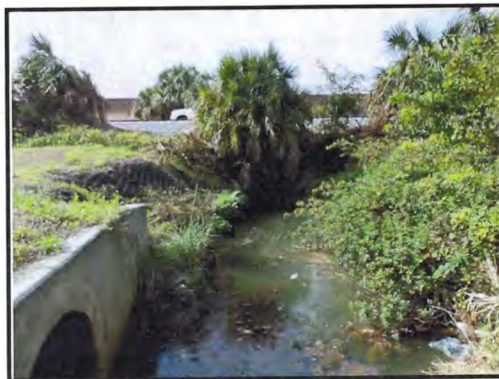
East (Downstream) Endwall and 48" RCP Cross Drain at MP 193.16
