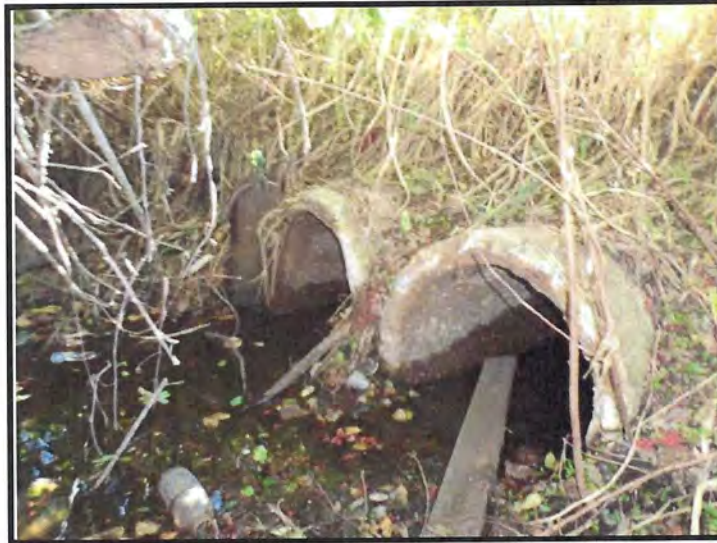
East (Downstream) End of Cross Drain MP 195.73
