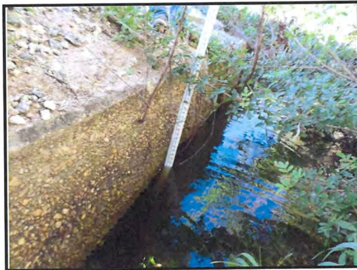
East (Upstream) End of Cross Drain MP 198.32 and Endwall
