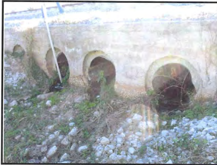
East (Downstream) Endwall and Cross Drain at MP 197.24. Note: Adjacent Capped Culverts.
