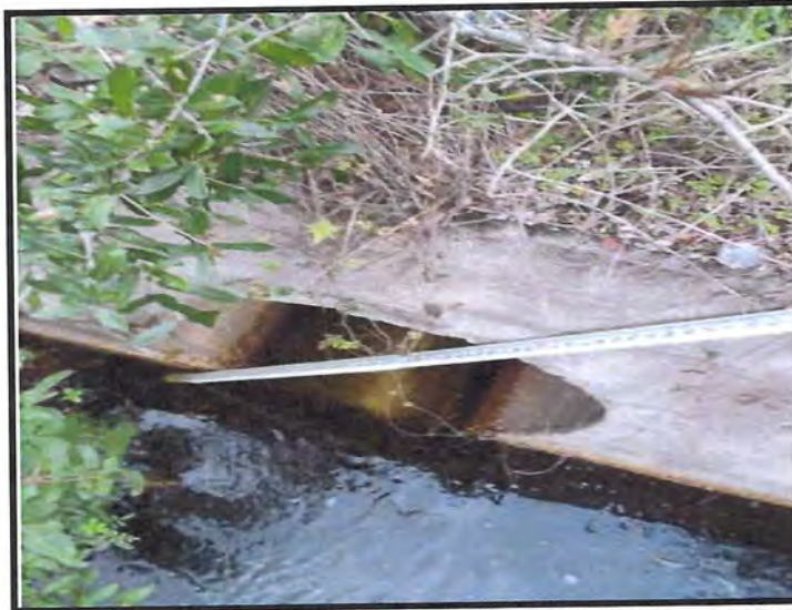
East (Downstream) End of Double 48" by 54" Culverts at MP 183.01
