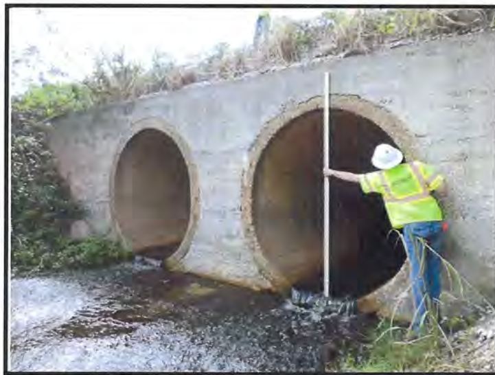
East (Downstream) Endwall and 2 - 84" RCP Cross Drains at MP 182.00
