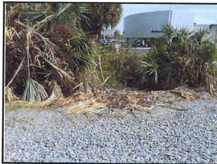
Looking East Toward Culvert Discharge Location
