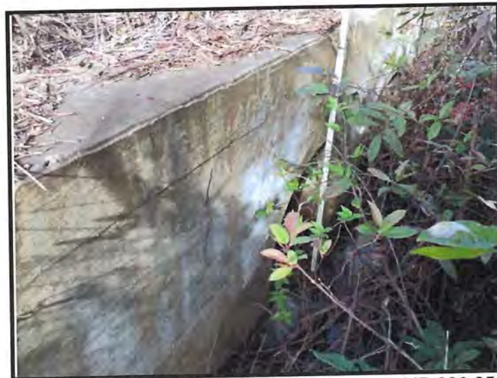
East Endwall of Double 36" RCP Culverts at MP 220.25
