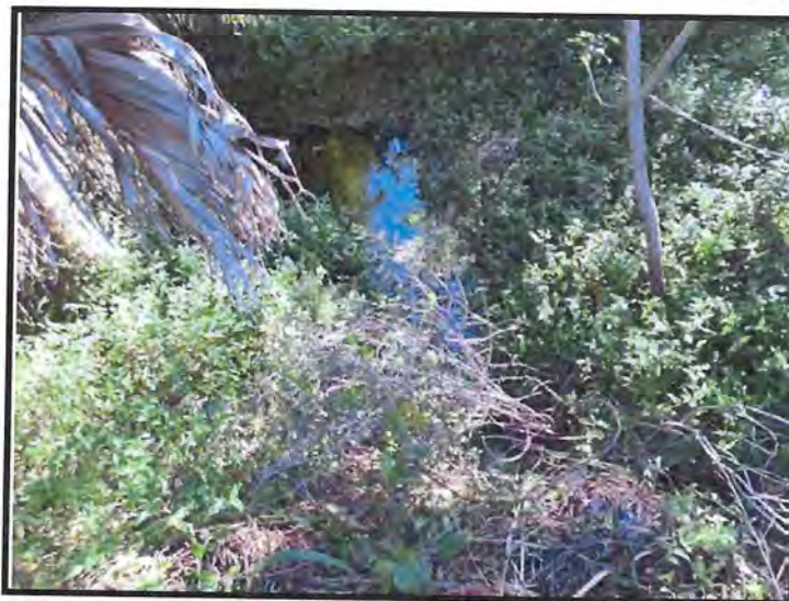
Looking East at Downstream Side of MP 230.51 Single 36" Culvert and Receiving Ditch
