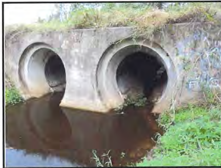
Looking at West Headwall at 2 - 72" CMP.
