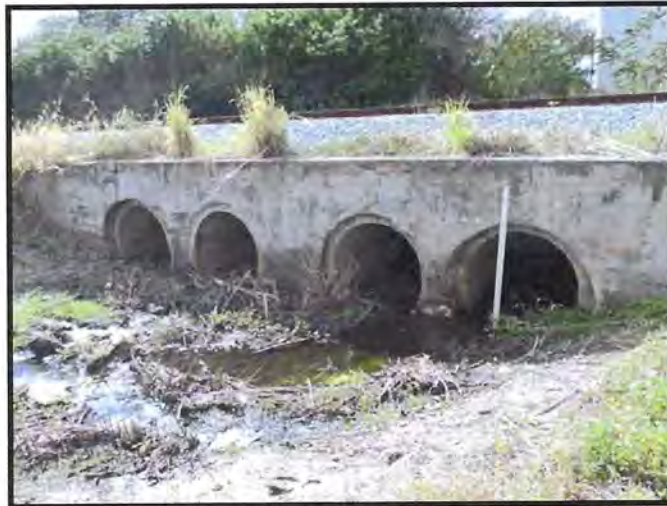
East (Downstream) End of 4-42" by 46" Culverts and Headwall at MP 224.83
