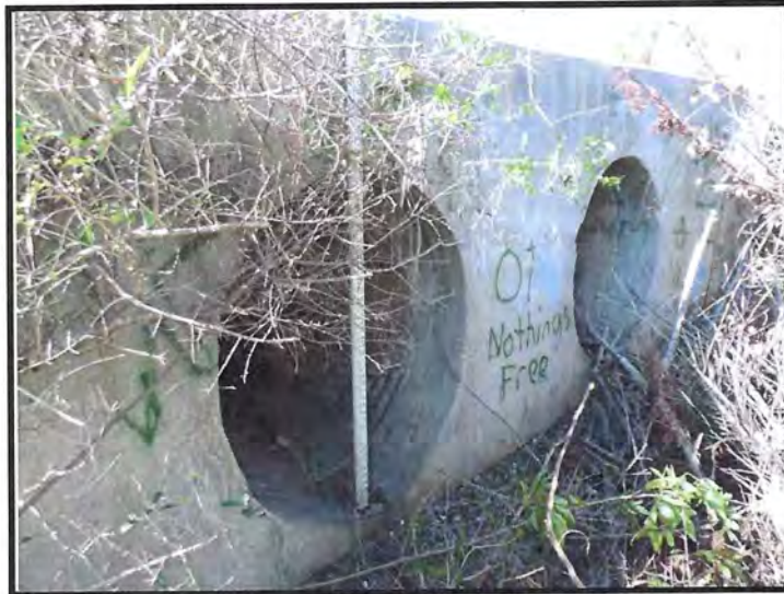
MP 193.32 East Endwall and Downstream Side of Double 48" by 54" RCP Culverts
