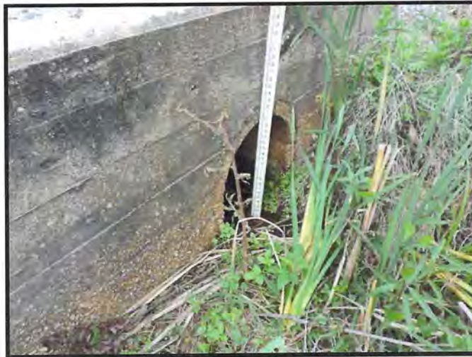
Looking at East Headwall of the 24" RCP.
