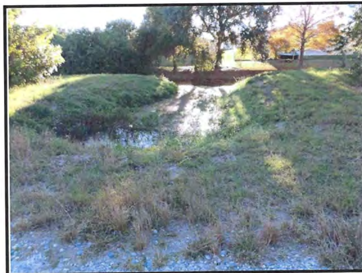
Looking West at Receiving Ditch System
