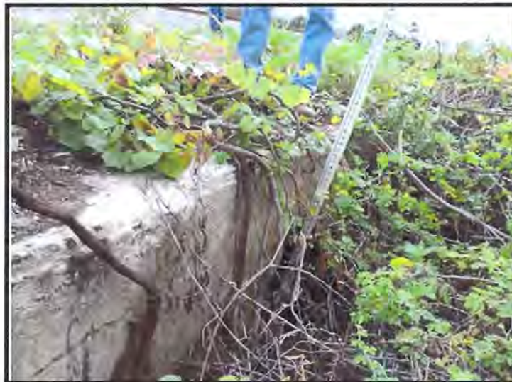
West (Upstream) End of Single 24" by 28" RCP Culvert and Headwall at MP 180.14
