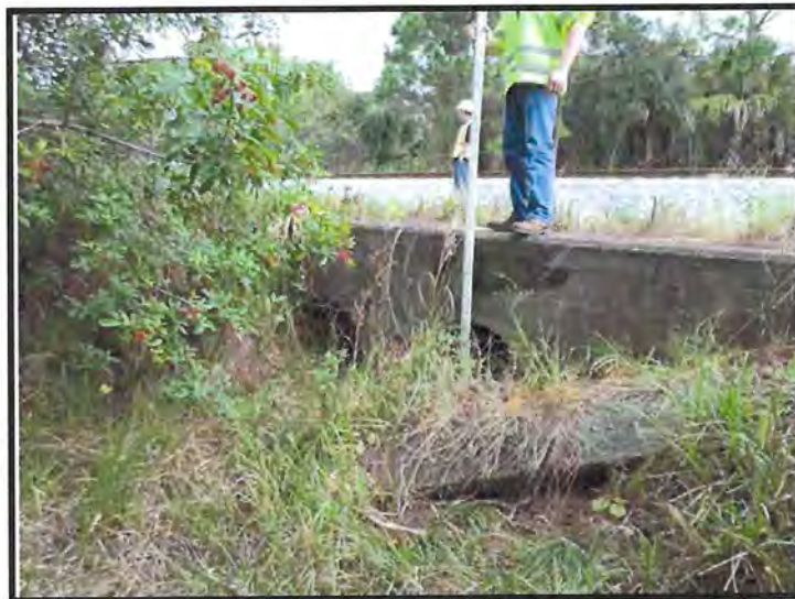
Western End of Existing Headwall and Double 36" by 40" RCP
