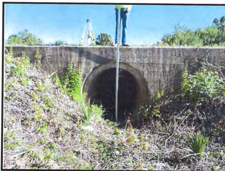
West (Upstream) Headwall at 60" RCP Cross Drain at MP 191.66
