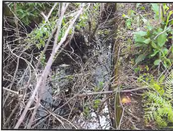
East (Downstream) Endwall and Double 30" x 40" RCP Drain at MP 201.22
