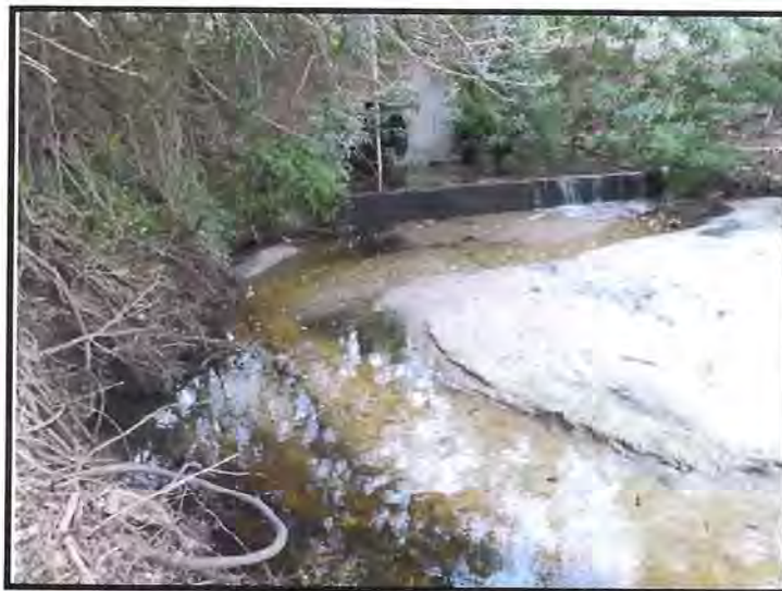
Existing East (Downstream) End of Cross Drains Showing Weir Structure
