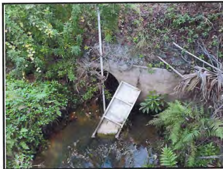
West (Upstream) Endwall and 48" RCP Cross Drain at MP 193.16
