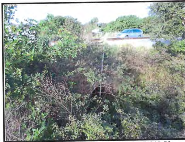
East Headwall of 42" by 46" RCP at MP 219.56
