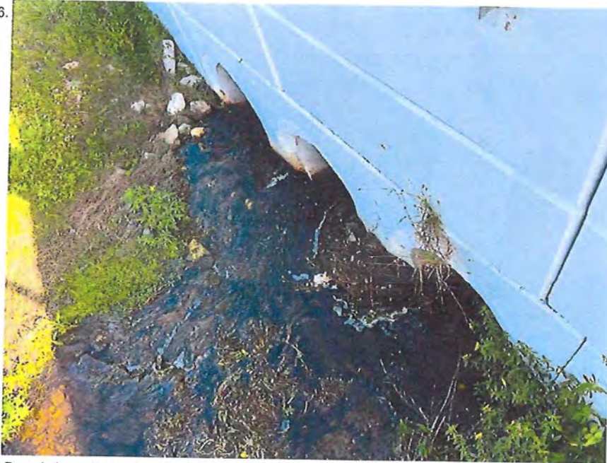
Description: Face of headwall West side (IMG_4350.jpeg)
