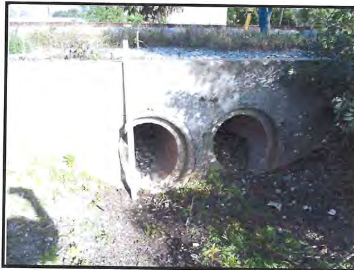
Existing West End of Cross Drain at MP 228.13
