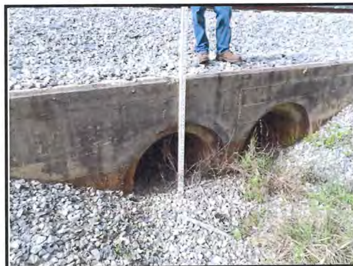
Eastern End of Existing Headwall and Double 36" by 40" RCP
