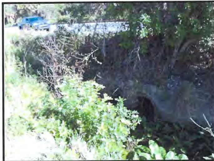
West (Upstream) Endwall of Double 30" RCP Culverts at MP 204.30
