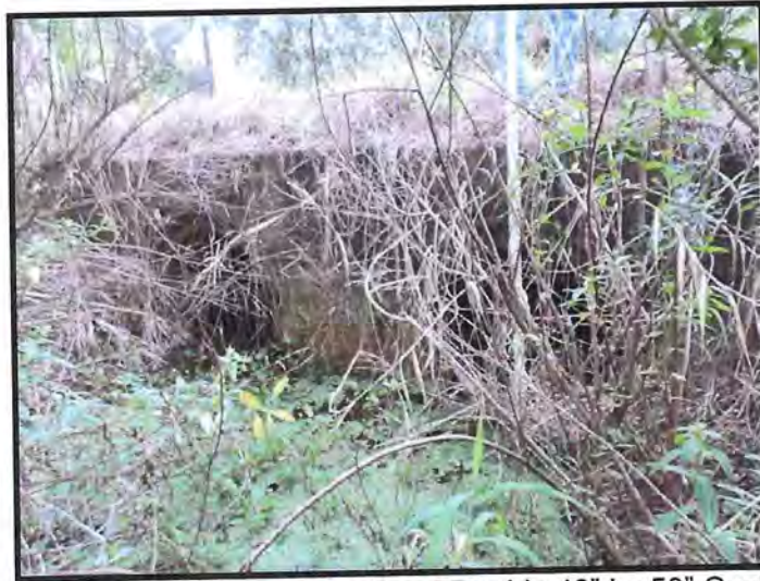
Western End of Existing Endwall and Double 48" by 53" Oval RCP.
