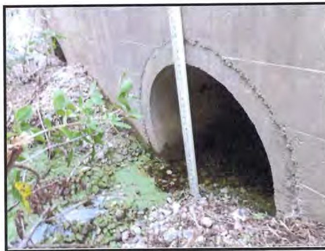
East (Downstream) Endwall and Double 36" RCP Culverts at MP 187.69
