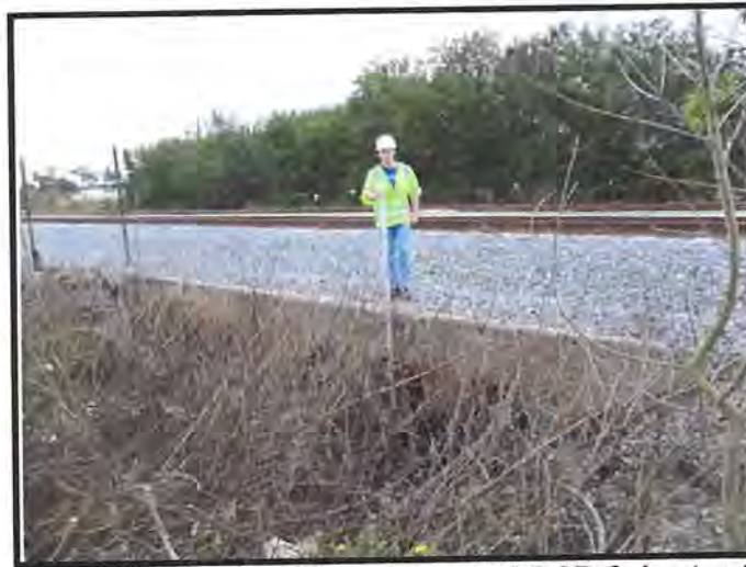
East (Downstream) Endwall and Five 30" by 33" RCP Culverts at MP 179.50
