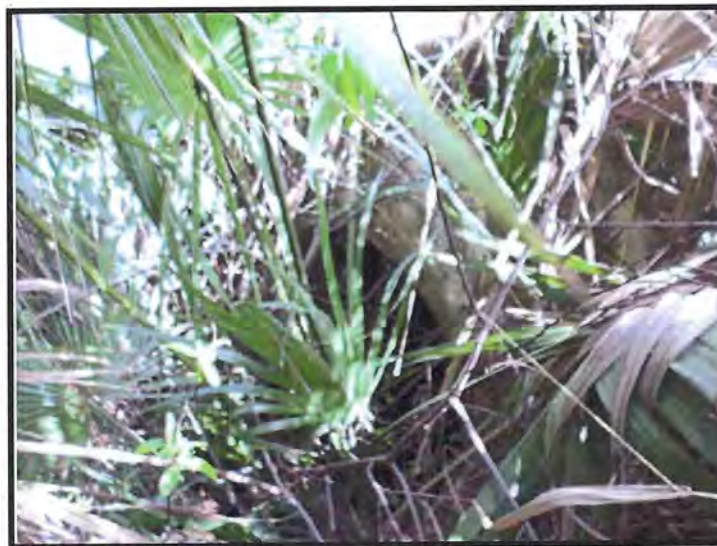
West End of Double 48" RCP at MP 221.42
