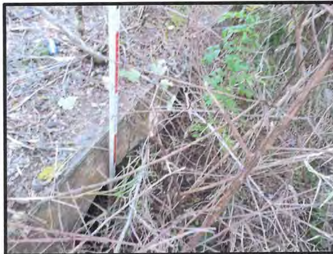
West (Upstream) End of 4-42" by 46" Culverts and Headwall at MP 224.83
