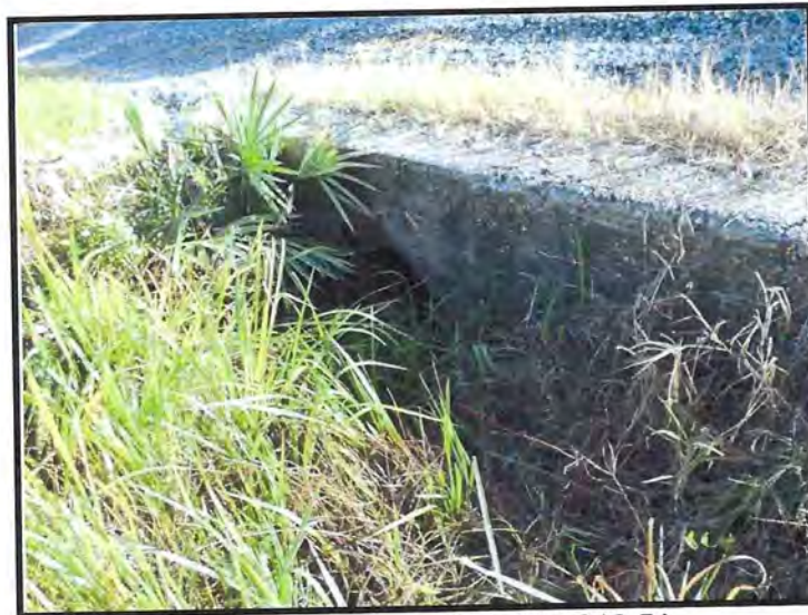
West End of Cross Drain MP 210.51
