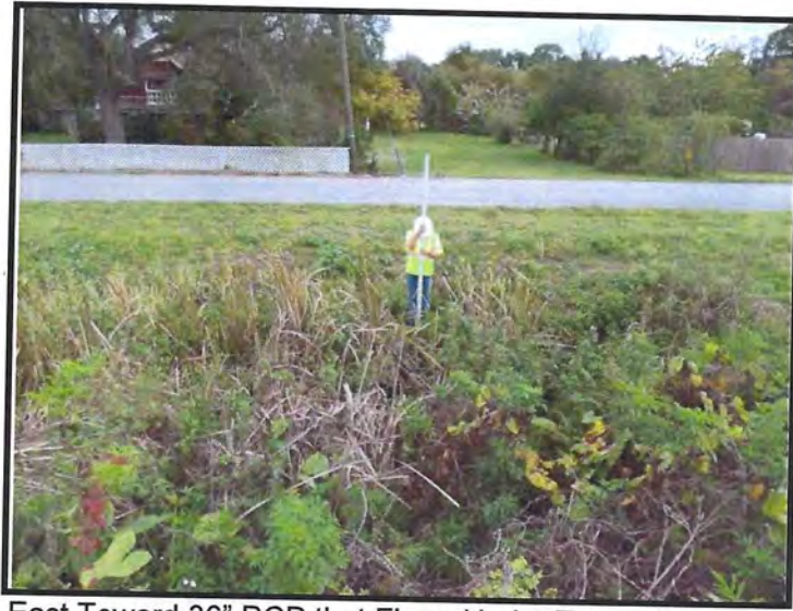
Looking East Toward 36" RCP that Flows Under Turner Rd. at MP 182.47.
