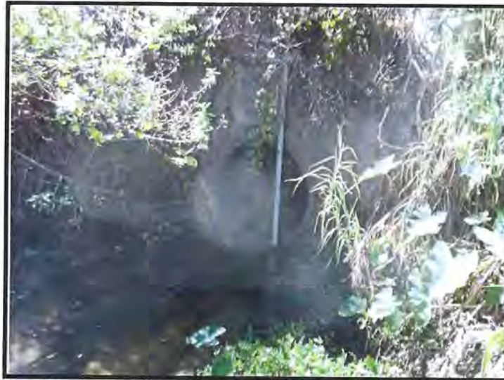
MP 193.32 East Headwall and Downstream Side of Single 48" RCP Culvert
