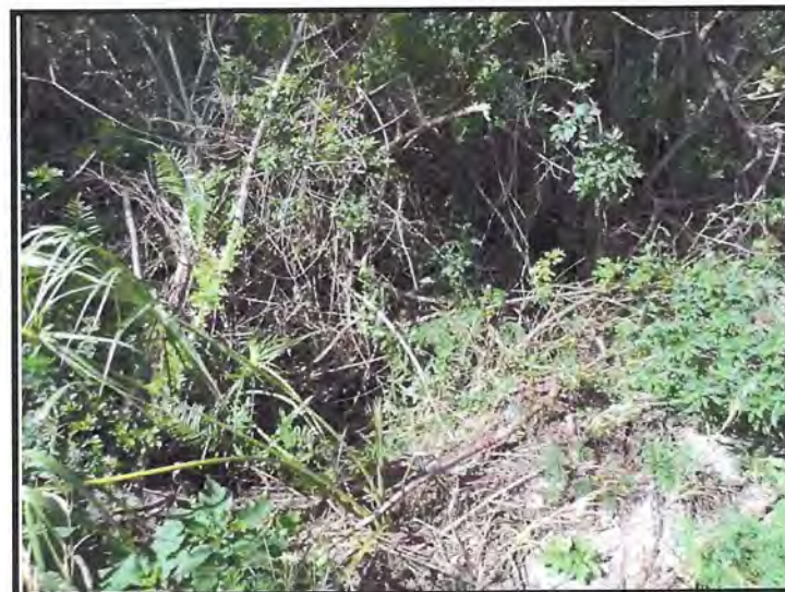
West End of Cross Drain at MP 205.40
