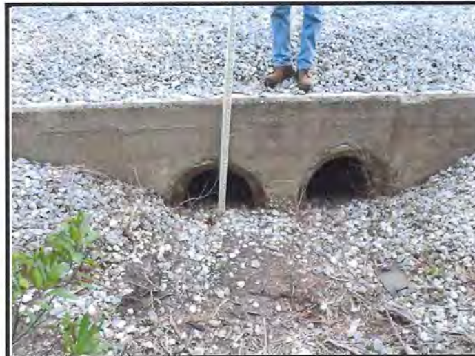
Looking at Upstream (West) End of MP 180.60 Cross Drain and Endwall
