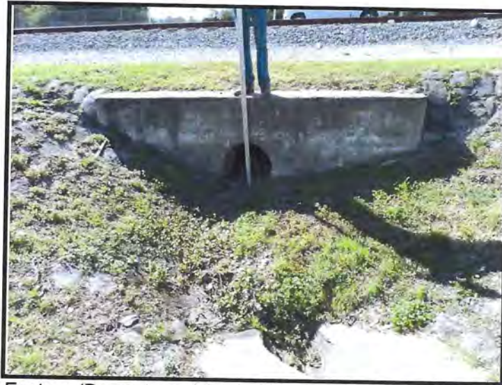
Looking West at Eastern (Downstream) End of MP 214.85 Cross Drain and Headwall. The Mitered End Section at the Bottom of the Photo is the 18" RCP (That was permitted to be a 24") Discharge from the Receiving Sump Draining to the Exfiltration Trench and Storm Sewer to the North
