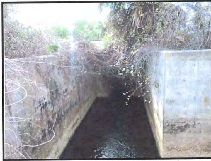
Eastern End (Downstream) of 72" RCP Culvert at Concrete Box Structure Directing Flow Northward Along US 1 (SR 5)
