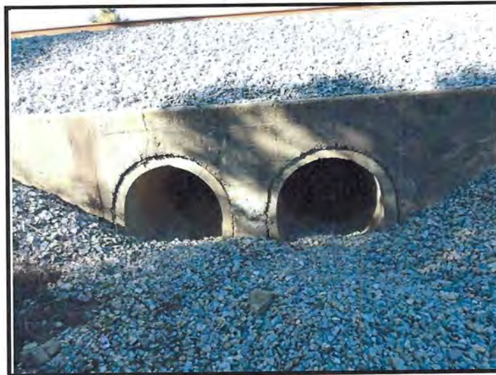
Looking at East (Downstream) Endwall and Double 42" Culverts at MP 191.17
