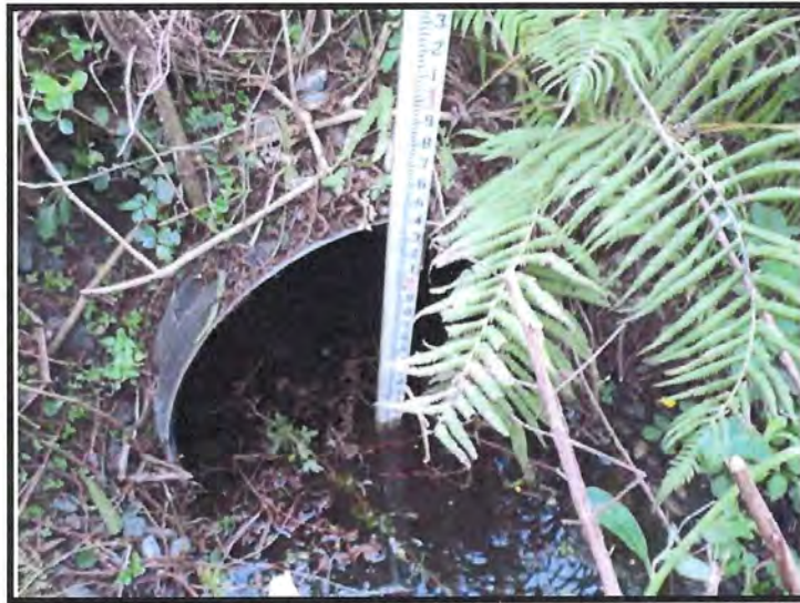
East (Downstream) End of Single 30" CMP Culvert at MP 180.14
