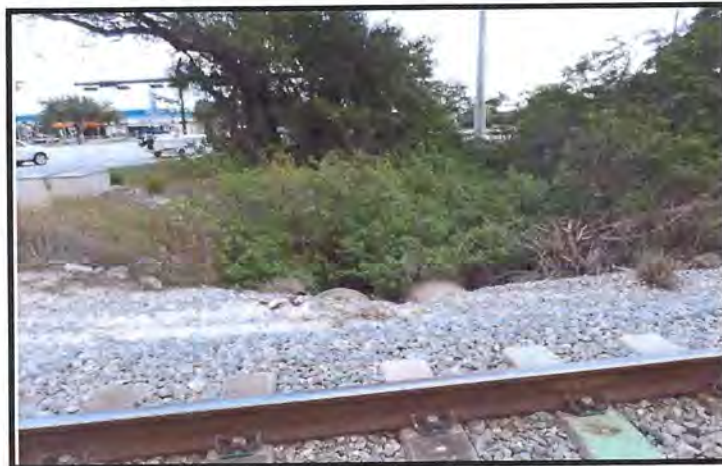
East Receiving Ditch of MP 229.76 Culvert System (Conveys Drainage to South Relief Canal)
