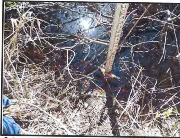
Submerged West End of Double 36" RCP at MP 213.59
