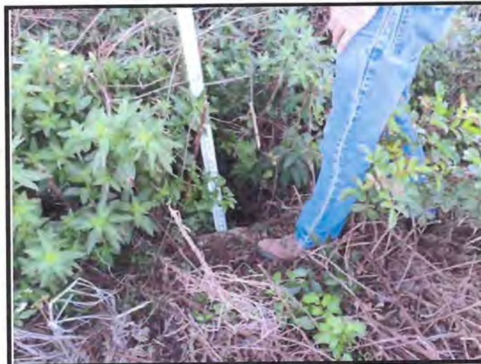
East (Downstream) End of 24" RCP Culvert at MP 203.88.
