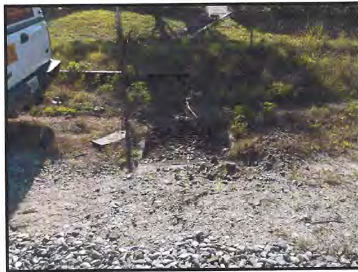
Existing Inlet on West Side of Existing Track
