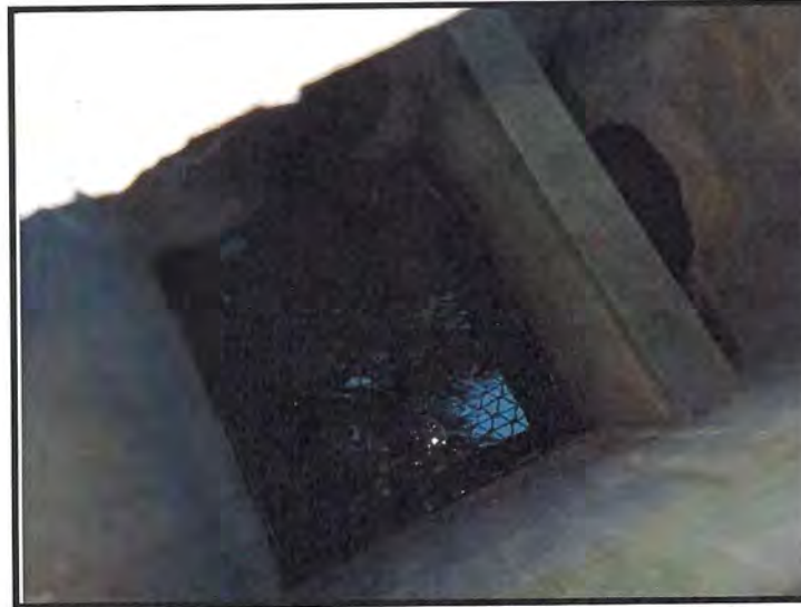
Inside of Catch Basin at East End of Cross Drain
