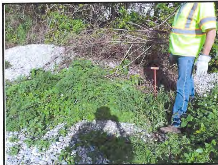
Approximate East (Downstream) End of Buried Cross Drain at MP 205.70
