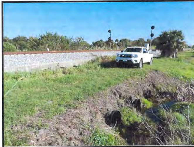
Triple 30" HDPE Culverts (Upstream of MP 197.24 Cross Drain)
