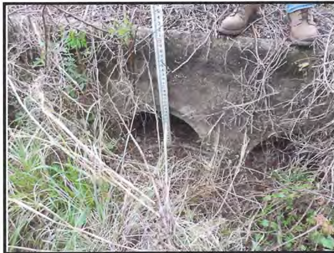
Looking at Downstream (East) End of MP 180.60 Cross Drain and Endwall
