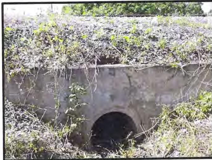
Eastern Headwall of 24" by 27" Oval RCP Culvert at MP 215.06
