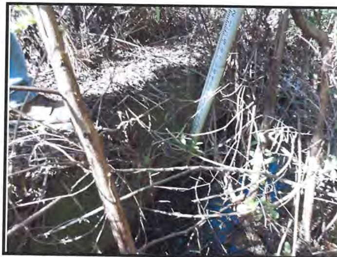
East End of MP 212.93 Cross Drain and Endwall
