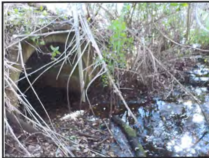
Existing West End of Cross Drain at MP 222.88
