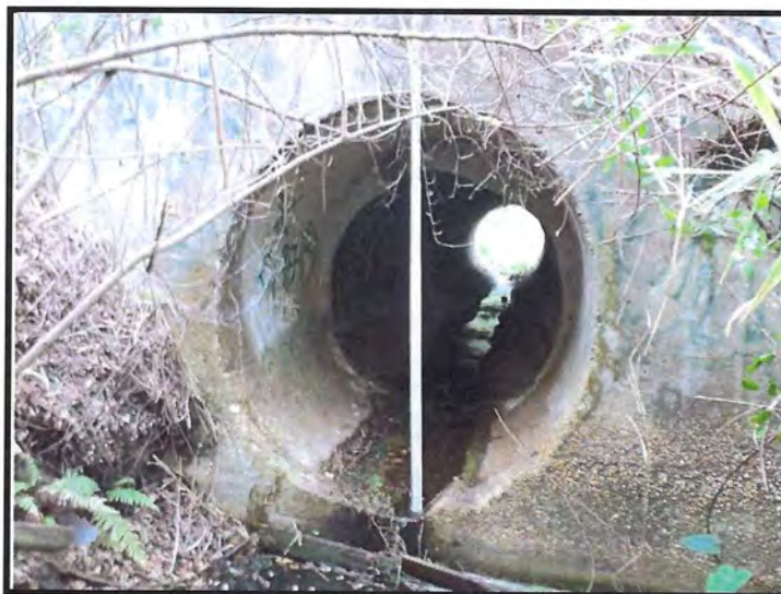
Looking at East Headwall at Southernmost culvert of 2 – 72" CMP.
