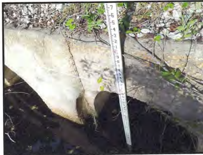
West (Upstream) Endwall and 2 – 42" by 46" RCP Cross Drains at MP 207.80
