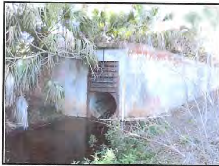
Existing West End of Cross Drain with Sluice Gate
