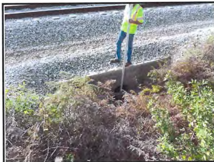
East (Downstream) Endwall of 24" RCP Culvert at MP 206.55.
