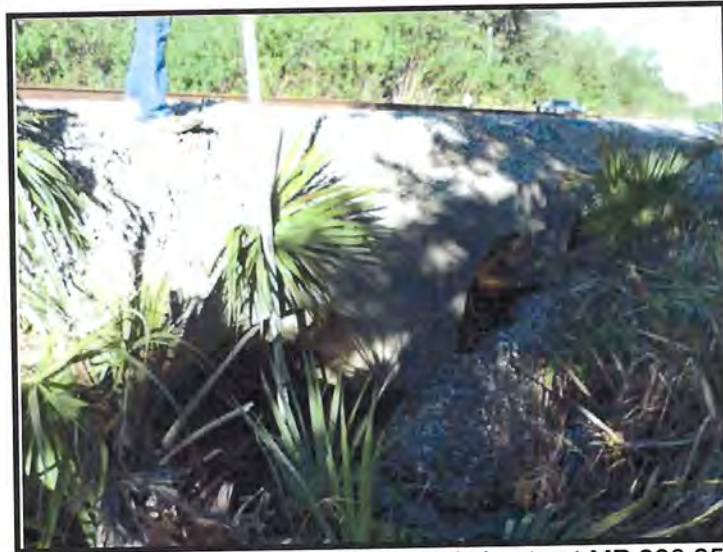
West Endwall of Double 36" RCP Culverts at MP 220.25
