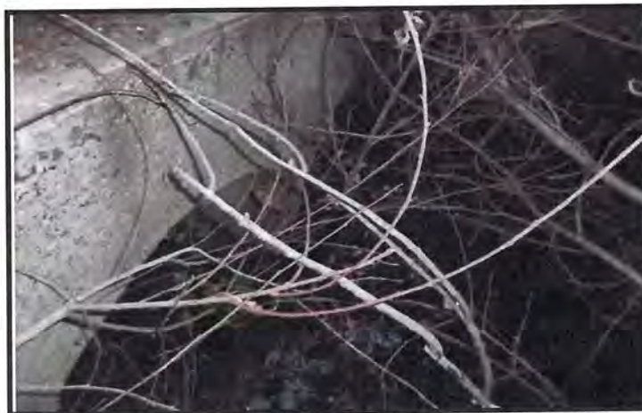
West End of MP 229.76 Culverts and Endwall
