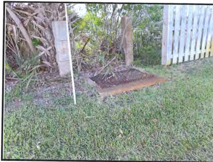
Catch Basin at East End of Cross Drain at MP 228.13
