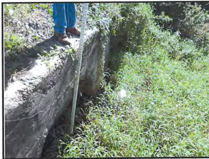
MP 205.01 West Endwall and Upstream Side of Culverts
