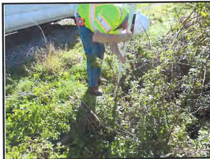
West (Upstream) End of 24" RCP Culvert at MP 203.88.
