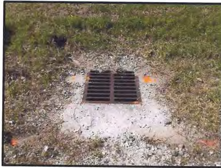
Existing Inlet on West Side of Existing Track
