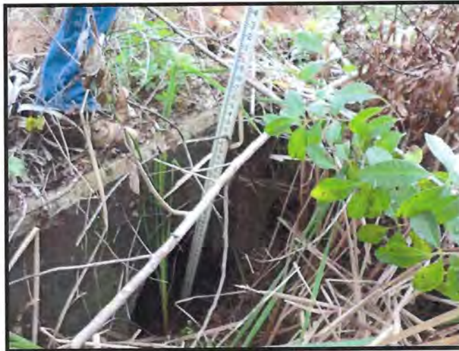
Looking at West Headwall of the 24" RCP.
