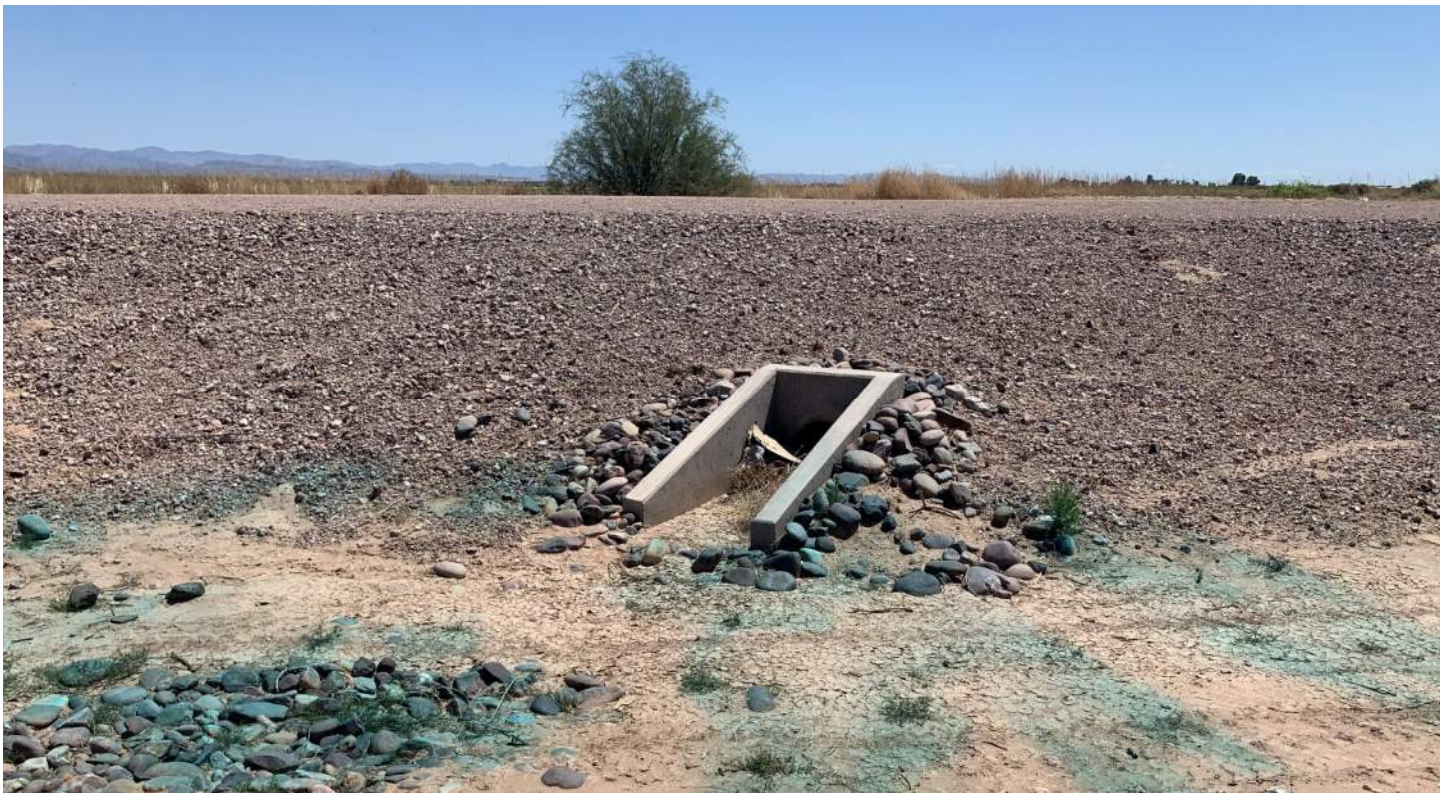
PHOTO 33: View of culvert in Ellsworth Channel at UPRR sta. 157+22, looking east.
