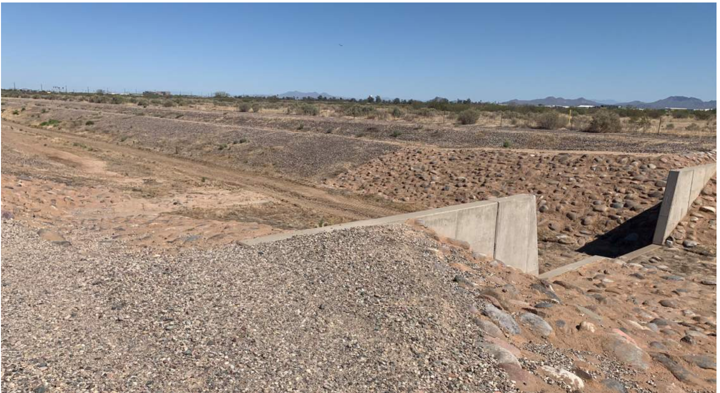
PHOTO 4: Rittenhouse Channel near UPRR sta. 1500+00, looking northwest.
