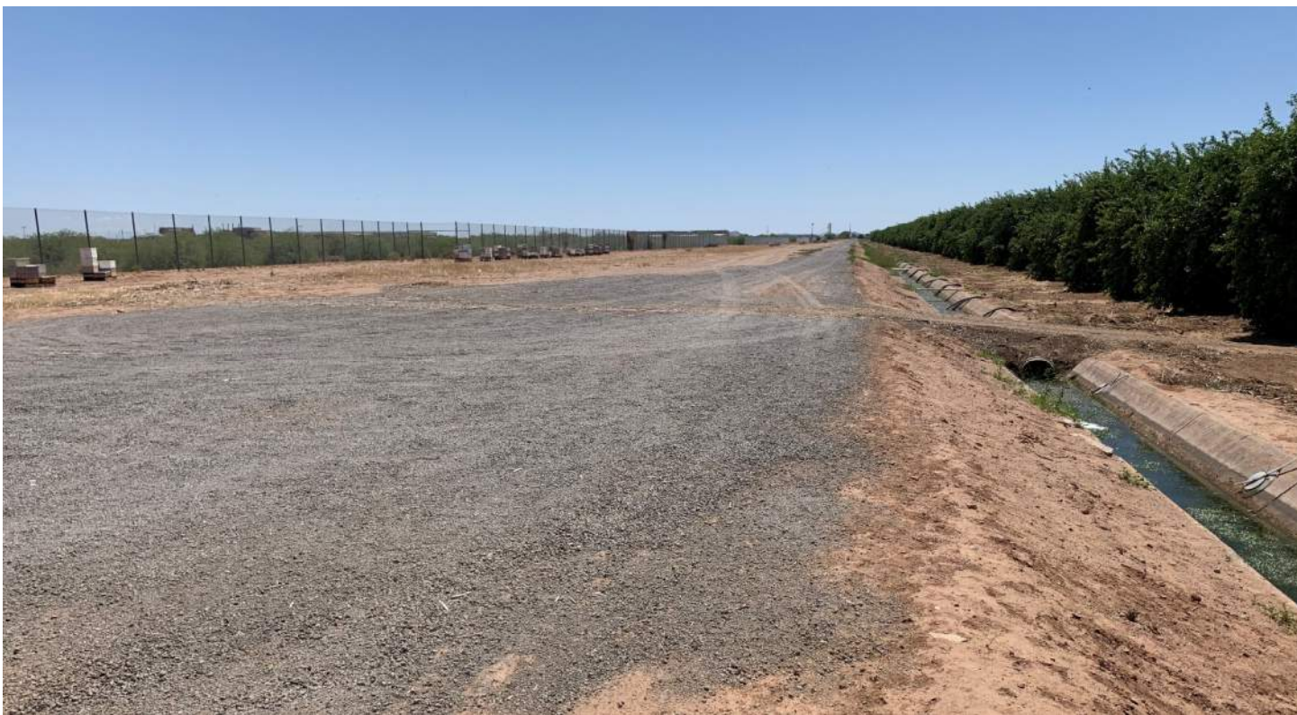
PHOTO 48: View from Signal Butte Road, looking south.
