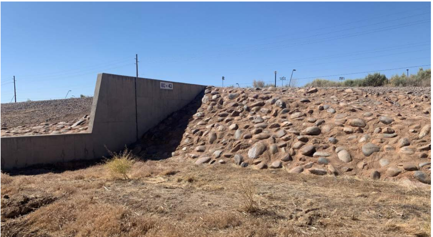
PHOTO 6: Typical Rittenhouse channel armoring, looking southeast.
