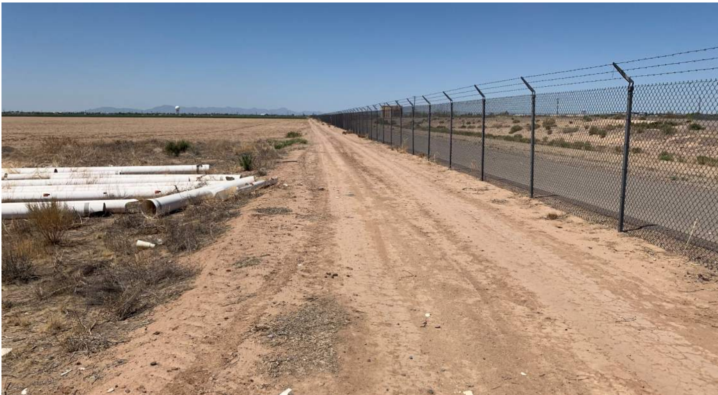
PHOTO 27: Near UPRR sta. 99+00, looking west.
