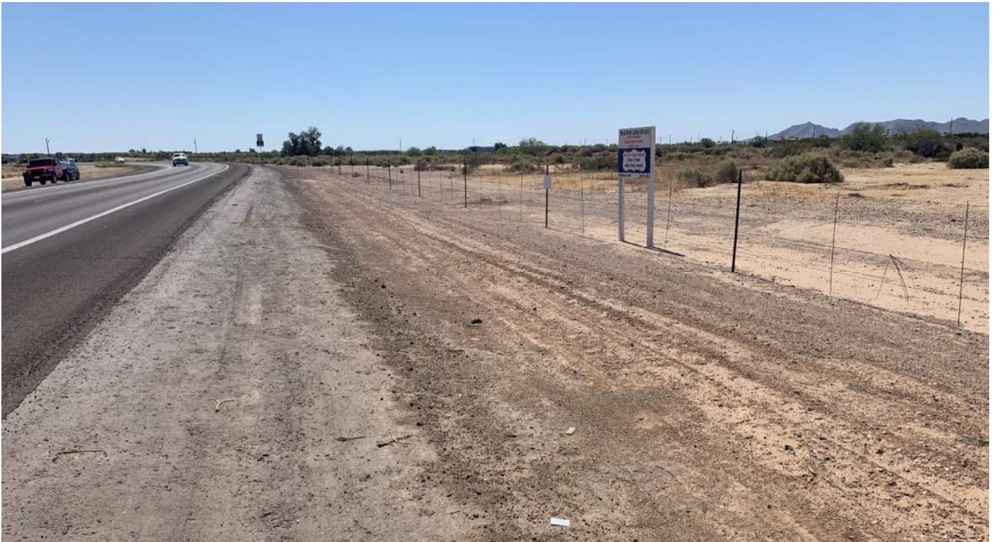
PHOTO 17: Downstream side of Pecos Road, UPRR sta. 24+00, looking southeast.
