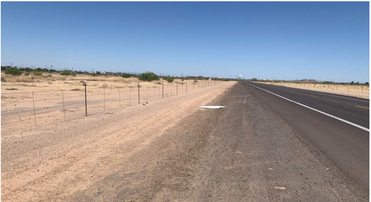
PHOTO 15: Downstream side of Pecos Road, UPRR sta. 24+00, looking northwest.
