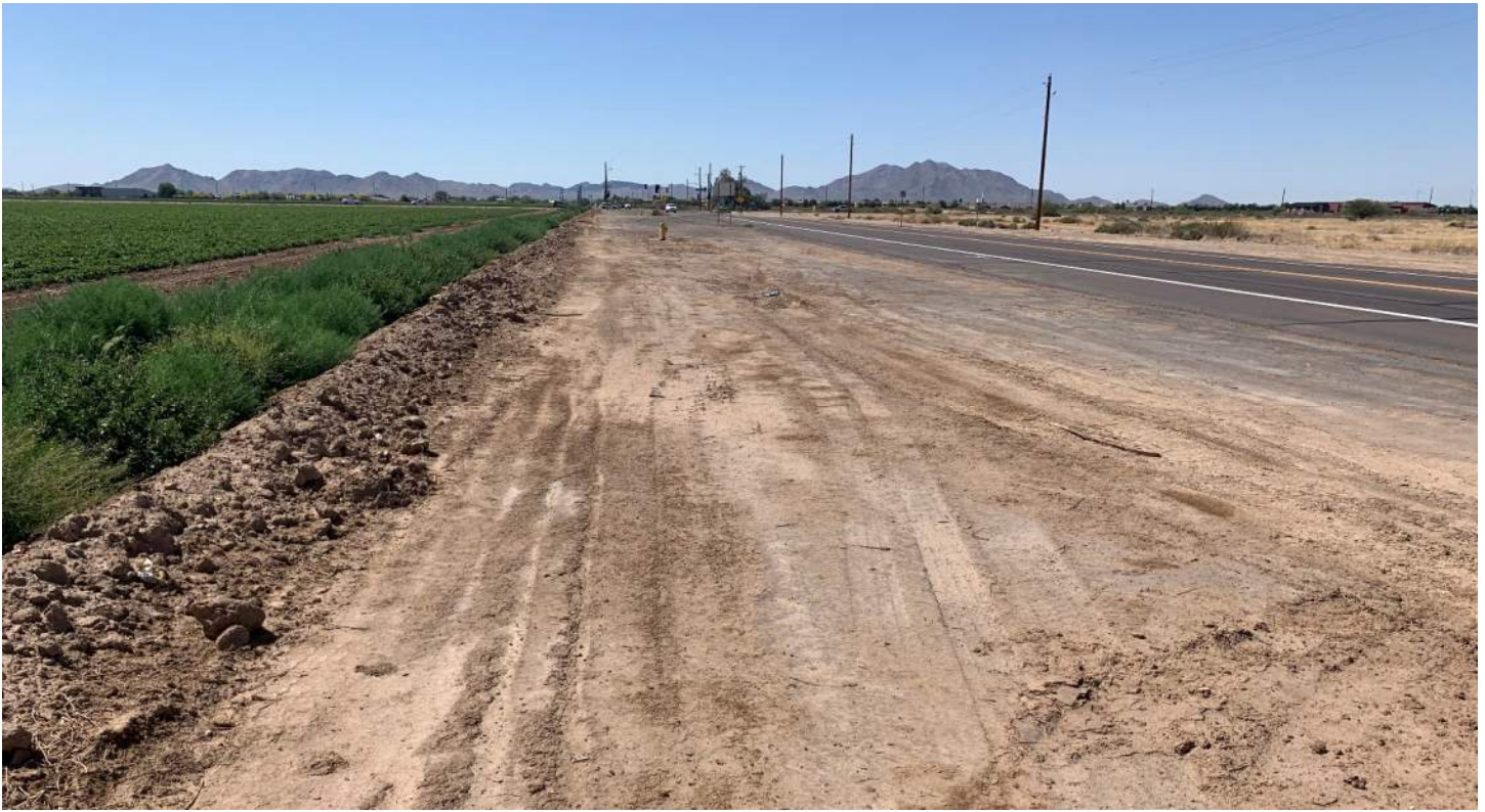
PHOTO 21: Upstream side of Sossaman Road, UPRR sta. 39+00, looking south.
