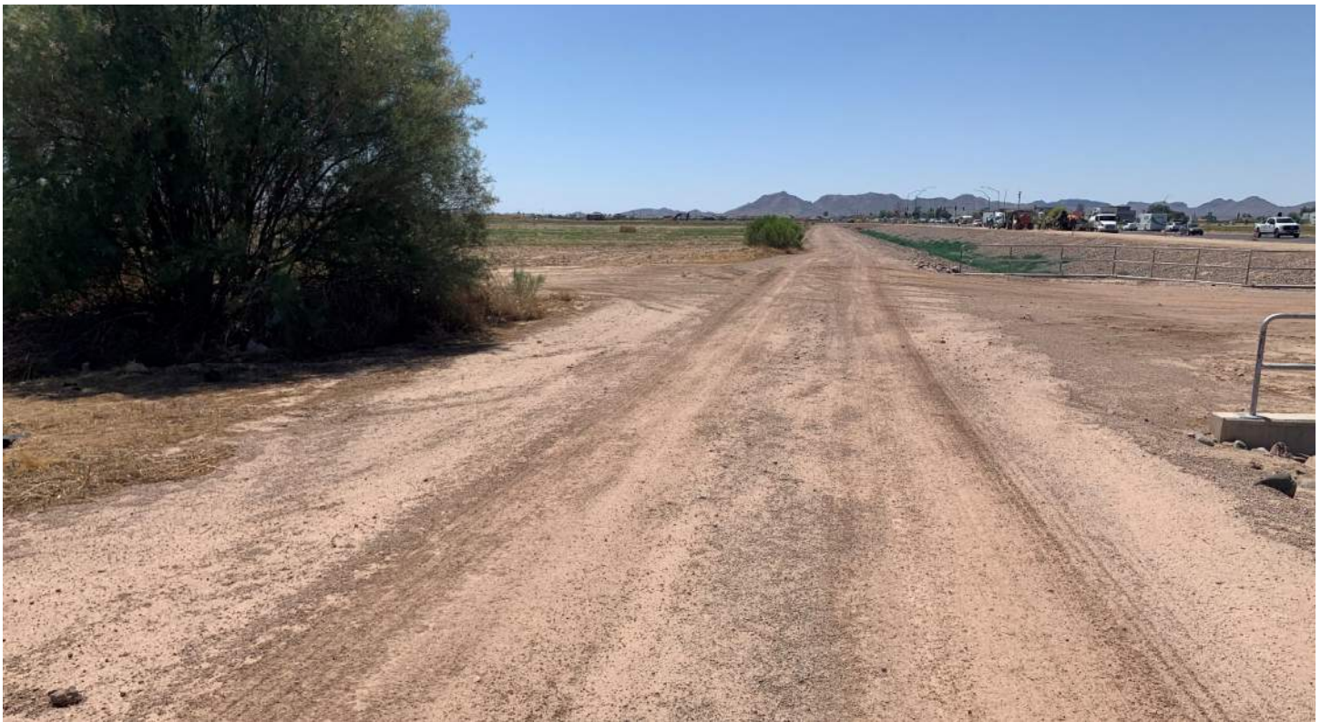
PHOTO 41: Top of access road culvert, looking east.
