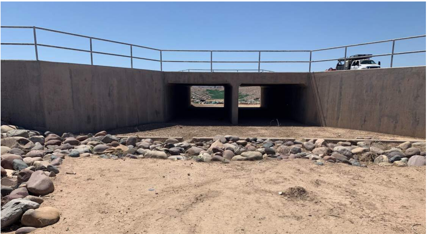
PHOTO 36: Upstream Ellsworth Channel culvert under private access road, looking south.
