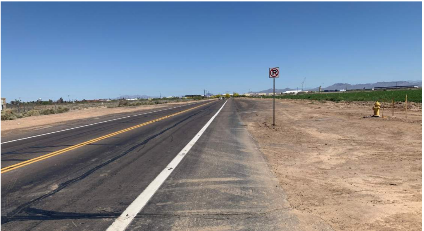
PHOTO 18: Upstream side of Sossaman Road, UPRR sta. 40+00, looking north.
