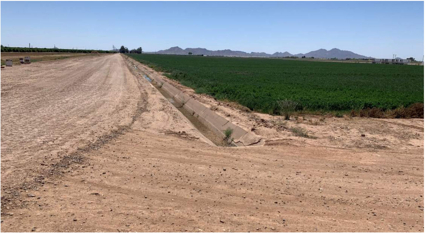
PHOTO 45: View from Pecos Road and Merrill Road, looking south.
