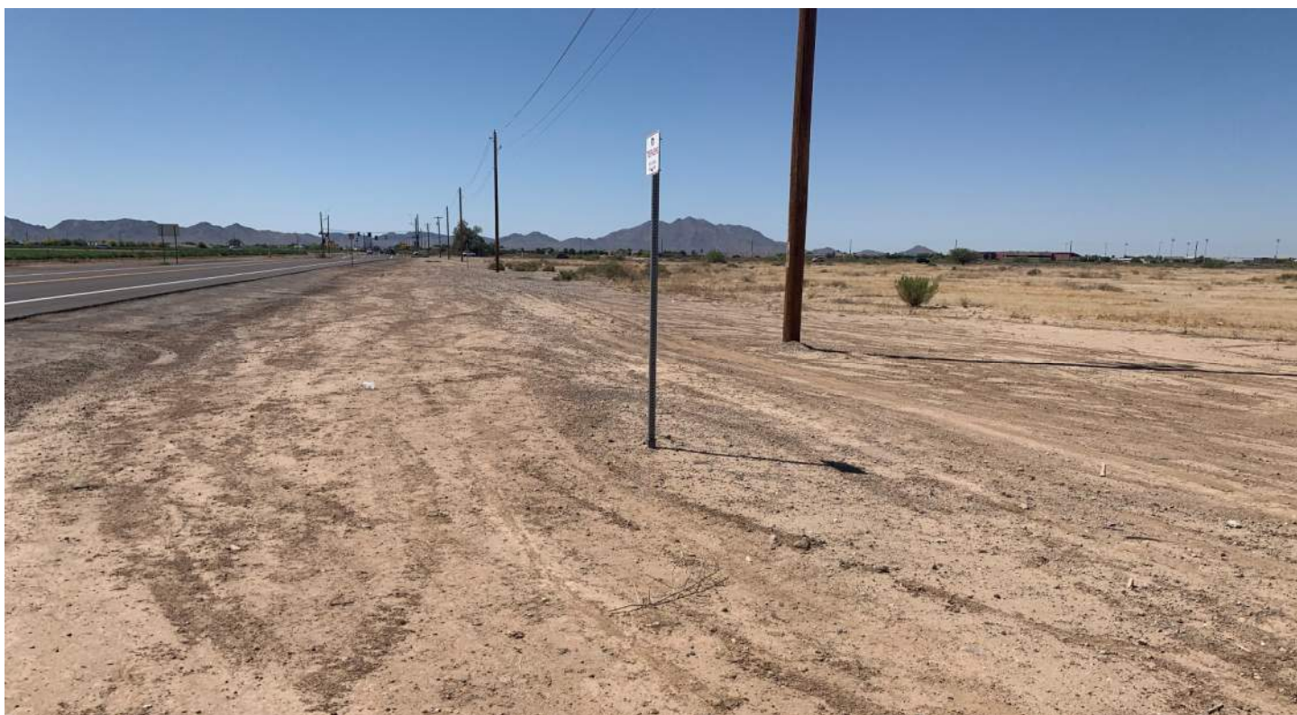
PHOTO 24: Downstream side of Sossaman Road, UPRR sta. 39+00, looking south.
