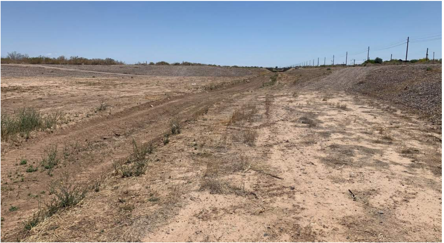
PHOTO 9: Upstream view of Rittenhouse Channel at E. Pecos Road, looking southeast.
