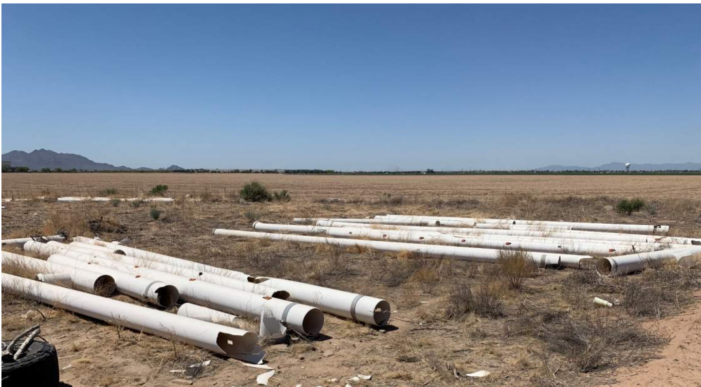
PHOTO 28: Near UPRR sta. 99+00, looking southwest.
