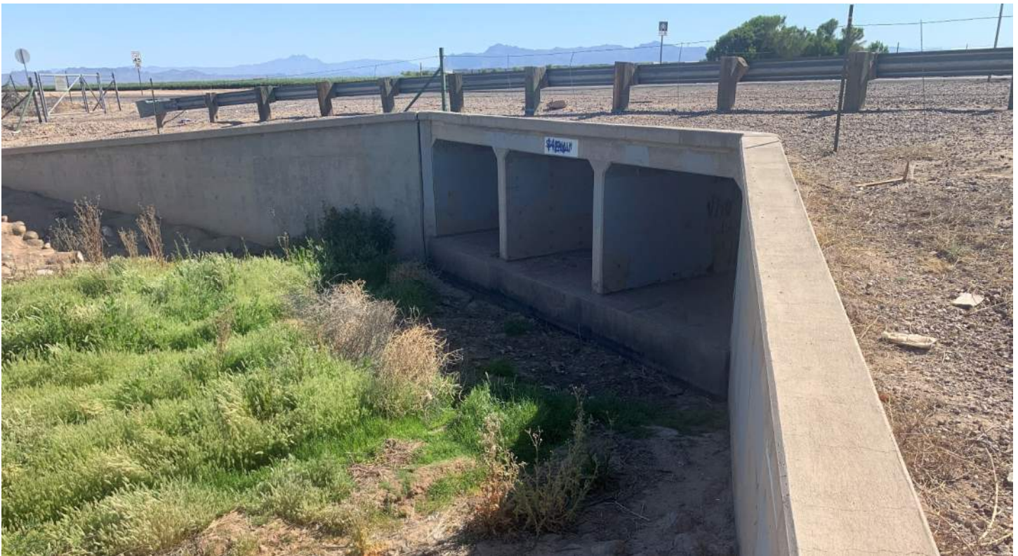
PHOTO 8: Downstream face of Rittenhouse Channel culvert at S. Sossaman Road, looking northeast.
