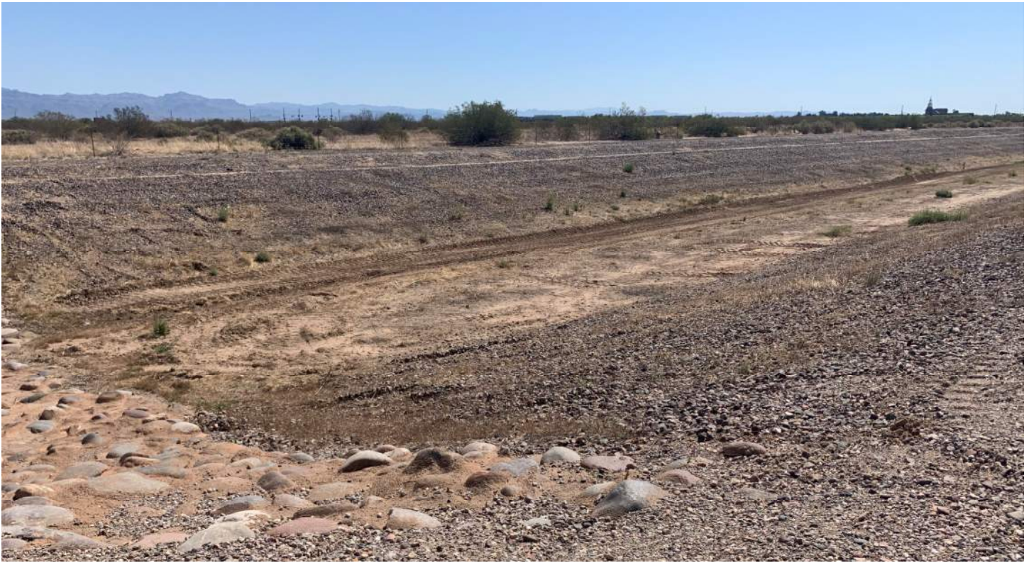
PHOTO 3: Rittenhouse Channel near UPRR sta. 1500+00, looking northeast.
