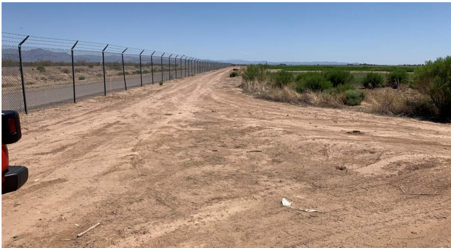
PHOTO 31: Near UPRR sta. 99+00, looking east.
