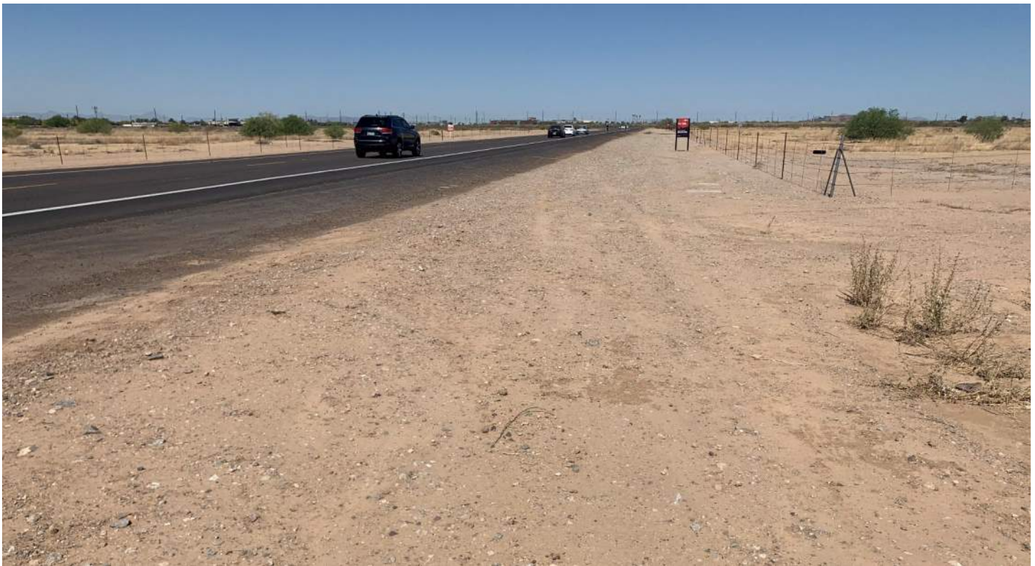
PHOTO 11: Upstream side of Pecos Road, UPRR sta. 24+00, looking northwest.
