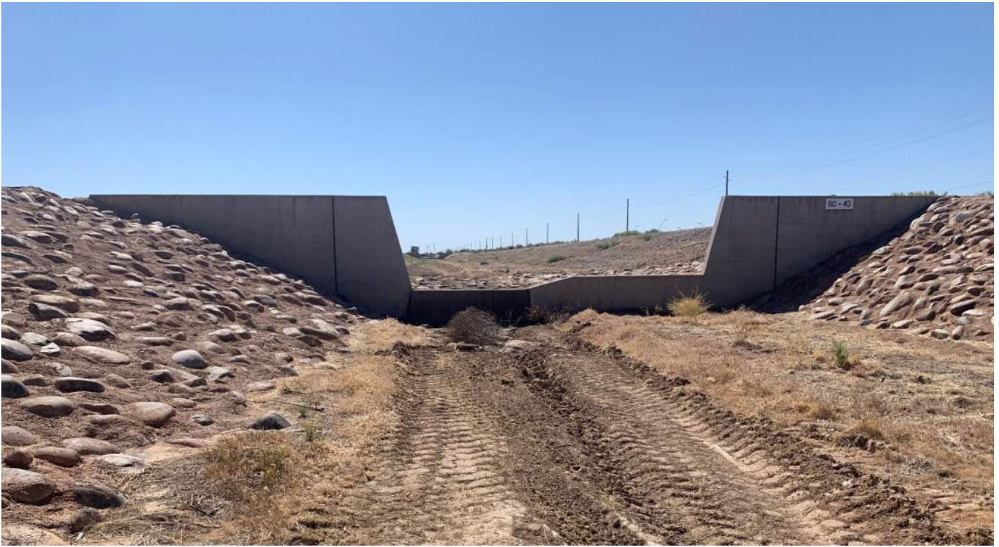
PHOTO 1: Rittenhouse Channel and weir, looking upstream near proposed Wye track.
