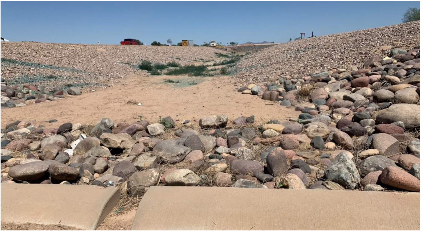
PHOTO 37: Looking downstream from private access road culvert, looking north.
