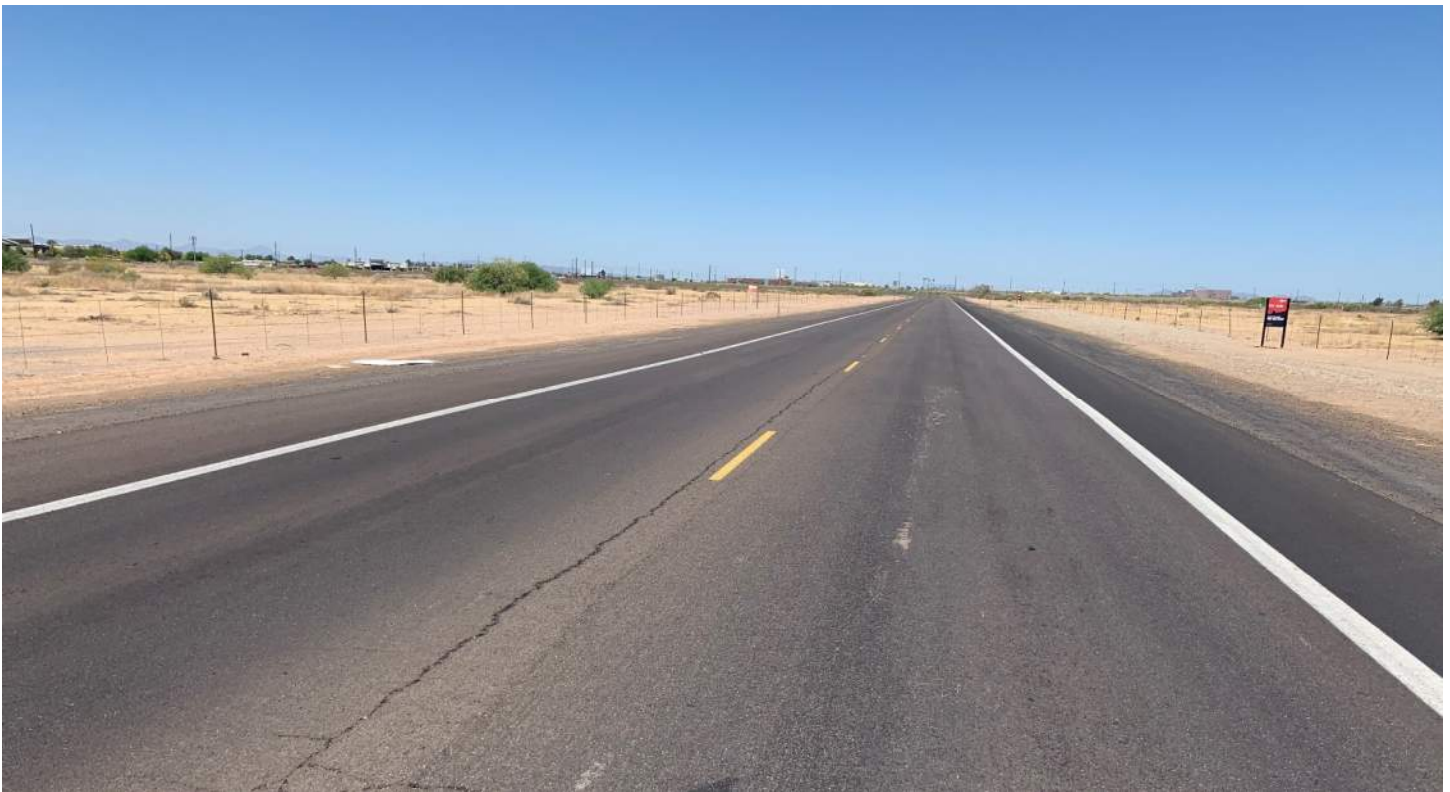
PHOTO 14: Top of Pecos Road near proposed track crossing, UPRR sta. 24+00, looking northwest.
