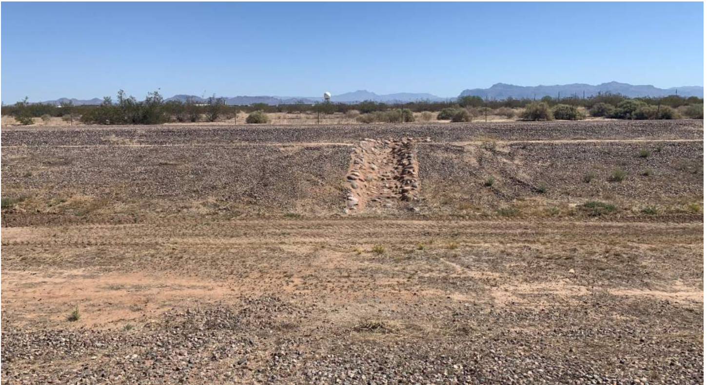
PHOTO 5: Armored drainage swells into Rittenhouse Channel near UPRR sta. 1500+00, looking northeast.
