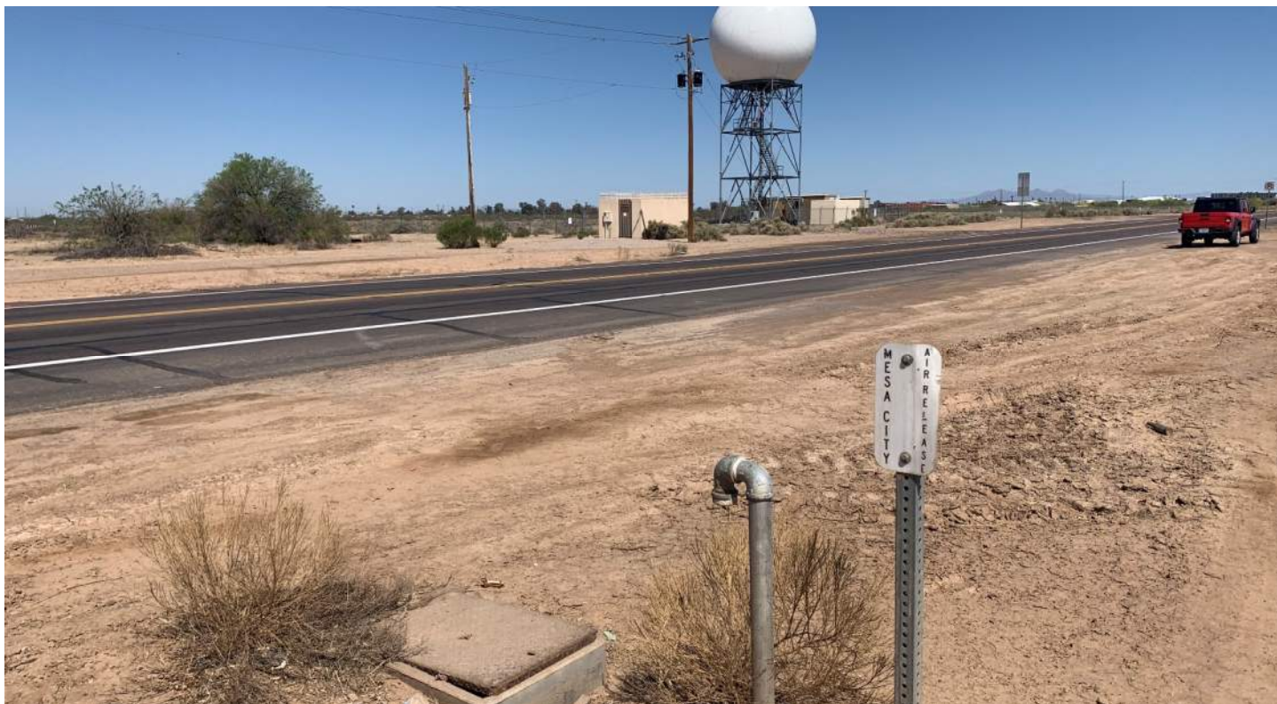
PHOTO 25: Looking northwest at Doppler and water line air release standpipe, UPRR sta. 40+00.
