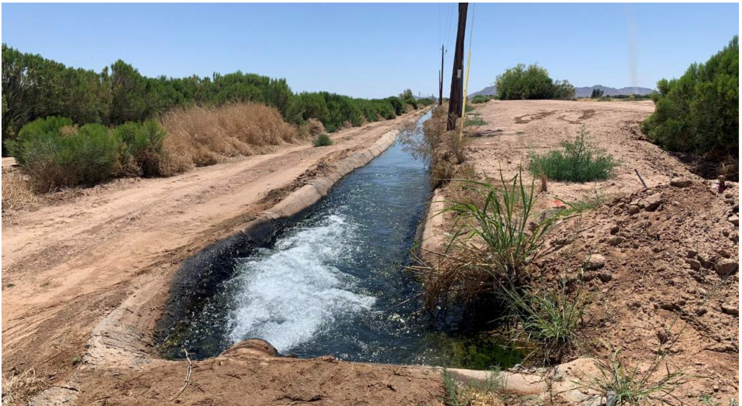
PHOTO 43: Irrigation flume on east side of Crismon Road, looking south.
