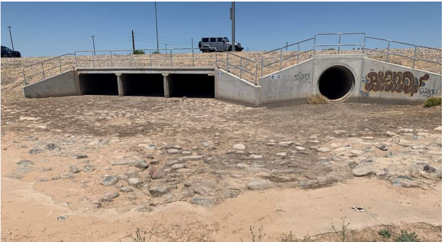
PHOTO 10: Upstream face of Rittenhouse Channel culvert at E. Pecos Road, looking northwest.
