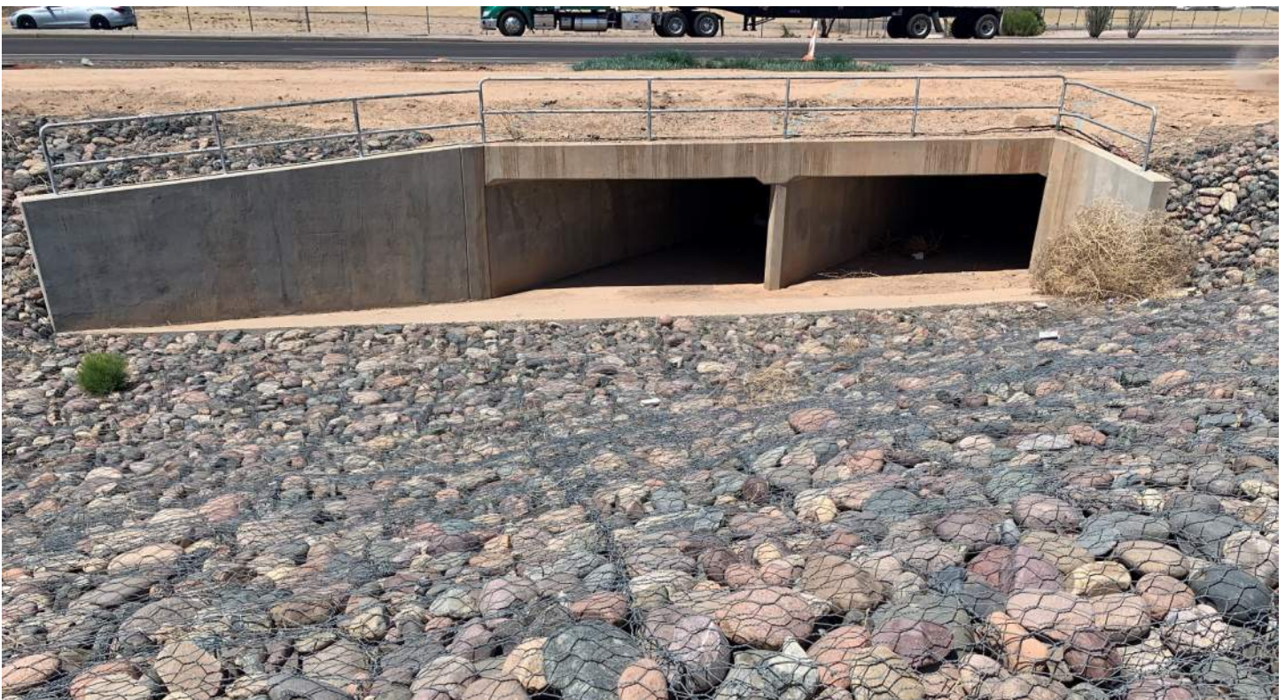
PHOTO 38: Downstream Ellsworth Channel culvert under Ellsworth Road, looking west.
