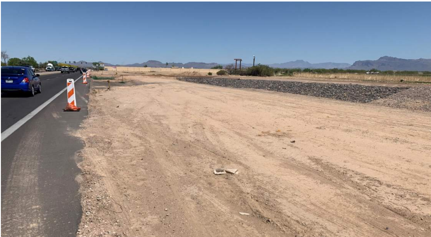
PHOTO 39: Edge of Ellsworth Road near proposed track crossing, looking north.
