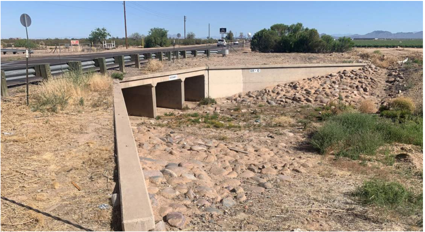
PHOTO 7: Upstream face of Rittenhouse Channel culvert at S. Sossaman Road, looking northwest.
