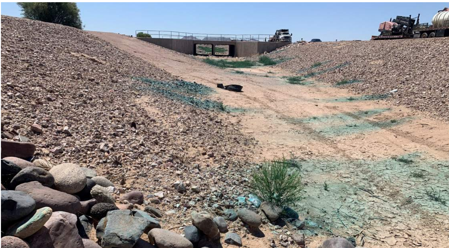
PHOTO 34: Upstream view of Ellsworth Channel at UPRR sta. 157+22, looking south.
