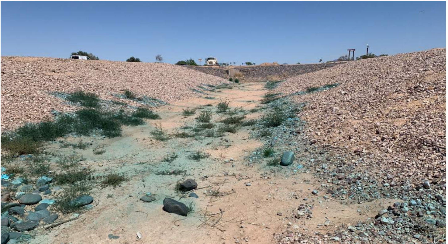
PHOTO 35: Downstream view of Ellsworth Channel at UPRR sta. 157+22, looking north.
