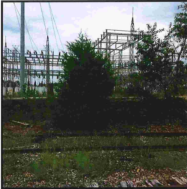
Photograph No. 7: Utilities along the project corridor, at Duke Street.
