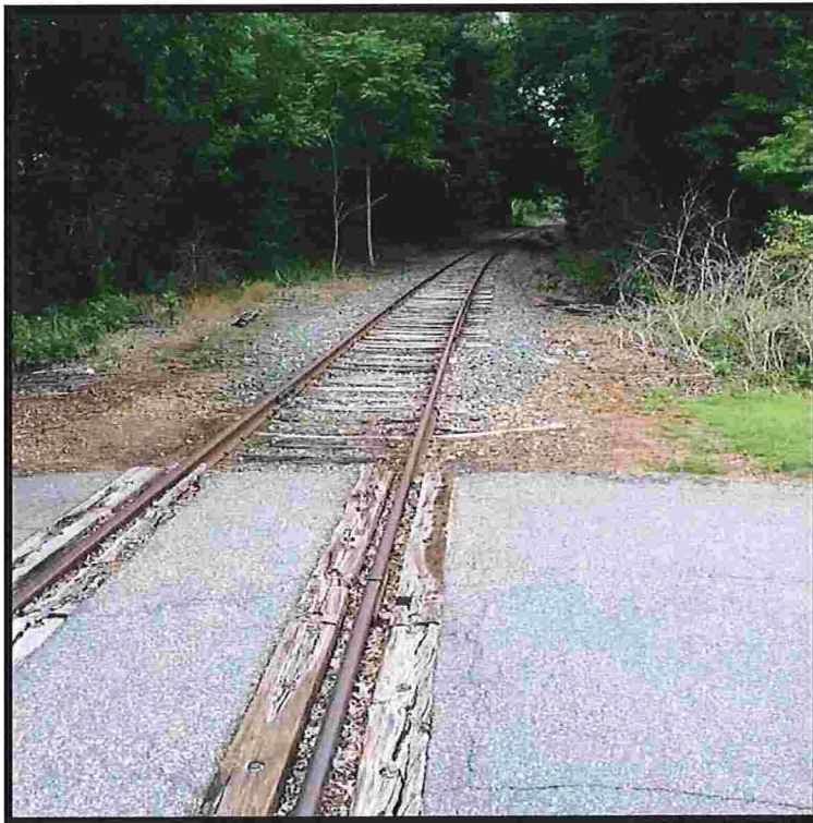
Photograph No. 6: Portion of the project corridor.
