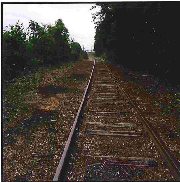
Photograph No. 2: Northern portion of project corridor, looking south east from northern terminus.
