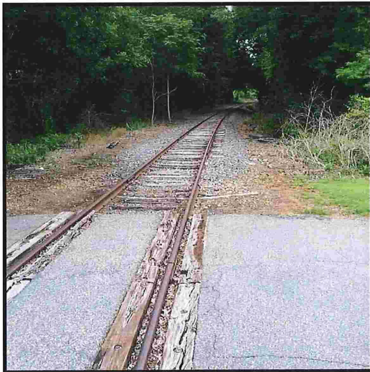
Photograph No. 6: Portion of the project corridor.
