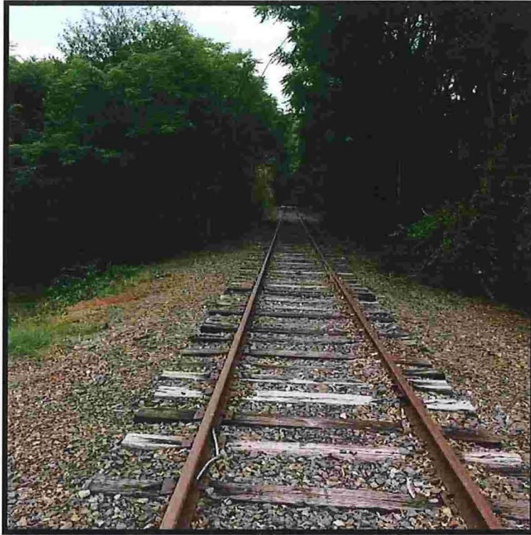
Photograph No. 9: Portion of the project corridor adjacent to the West Main Street Historic District.
