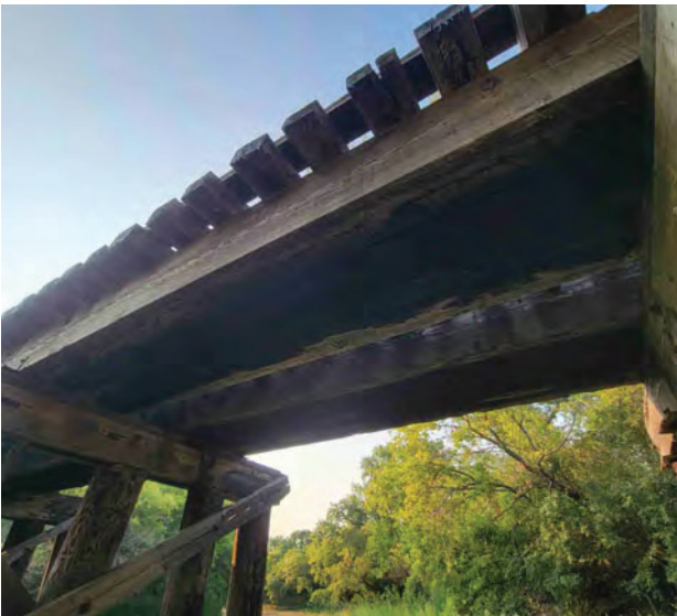
Bridge 11.0 Typical Span
