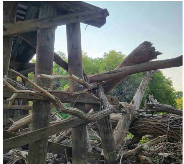
Bridge 11.0 Bent 6 Pile 1
