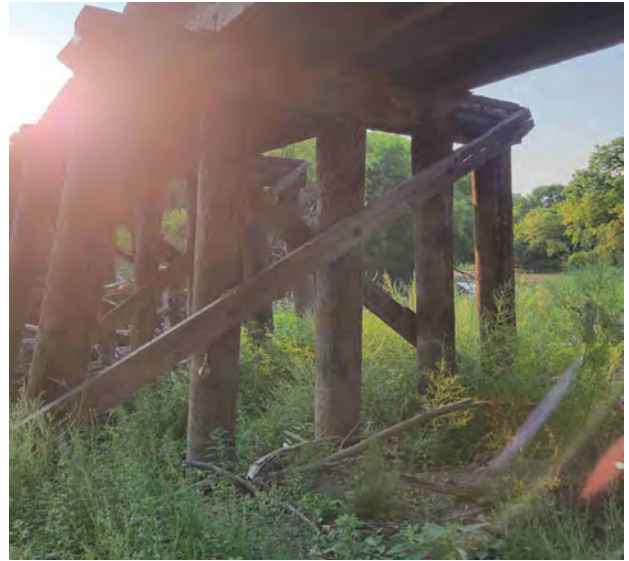
Bridge 11.0 Typical Bent
