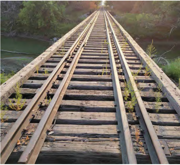
Bridge 11.0 Deck View
