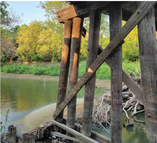
Bridge 11.0 Bent 4 Pile 1
