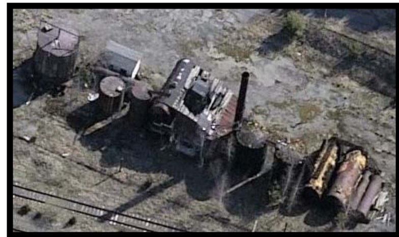
Rear View before demolition
