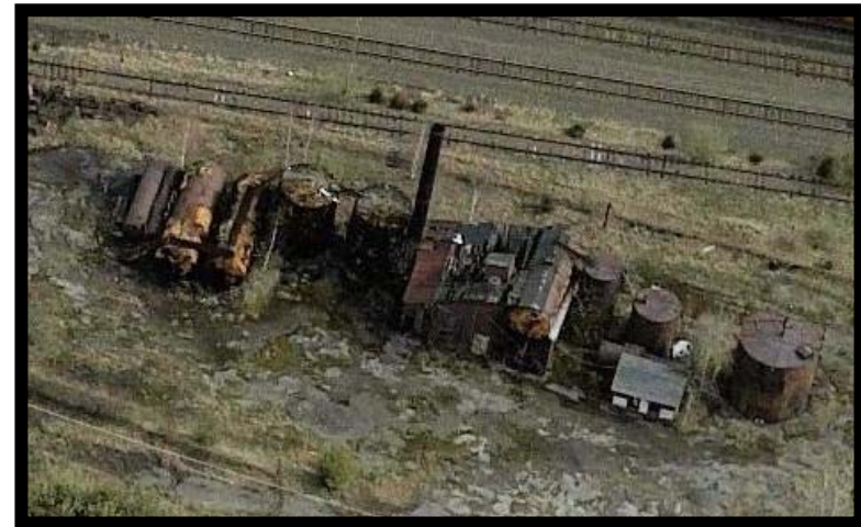
Front View before demolition
