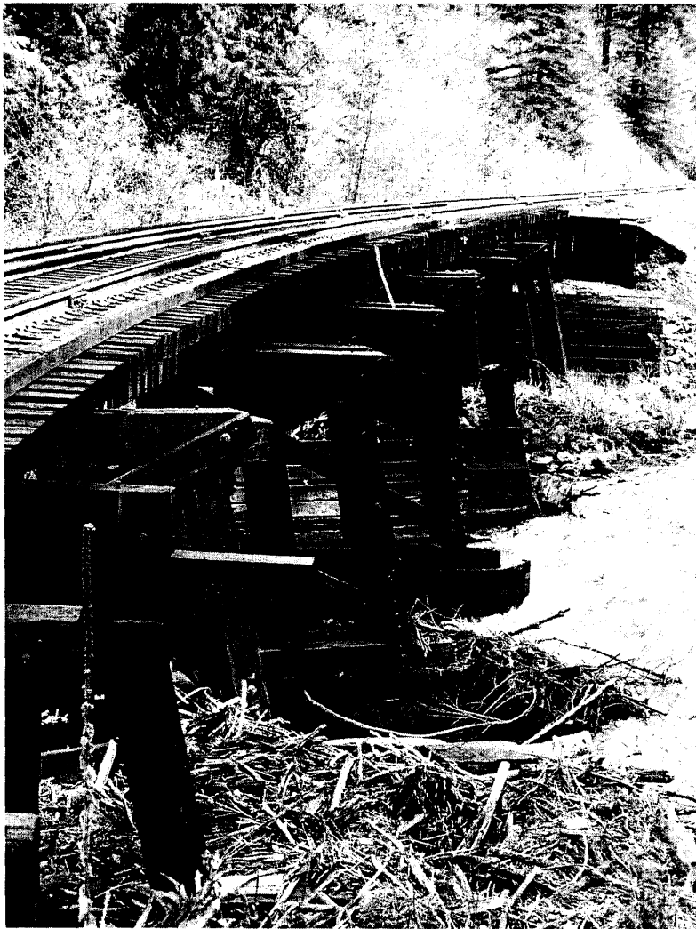
Trestle # 11 Side View
