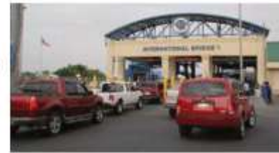
Eagle Pass International Bridge I (IB1)
