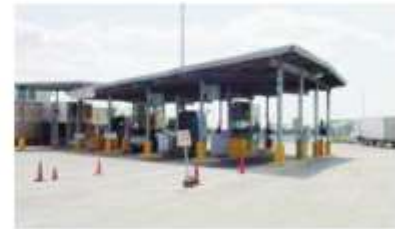
Camino Real International Bridge (IB2) (a.k.a. Eagle Pass-Piedras Negras International Bridge II)
