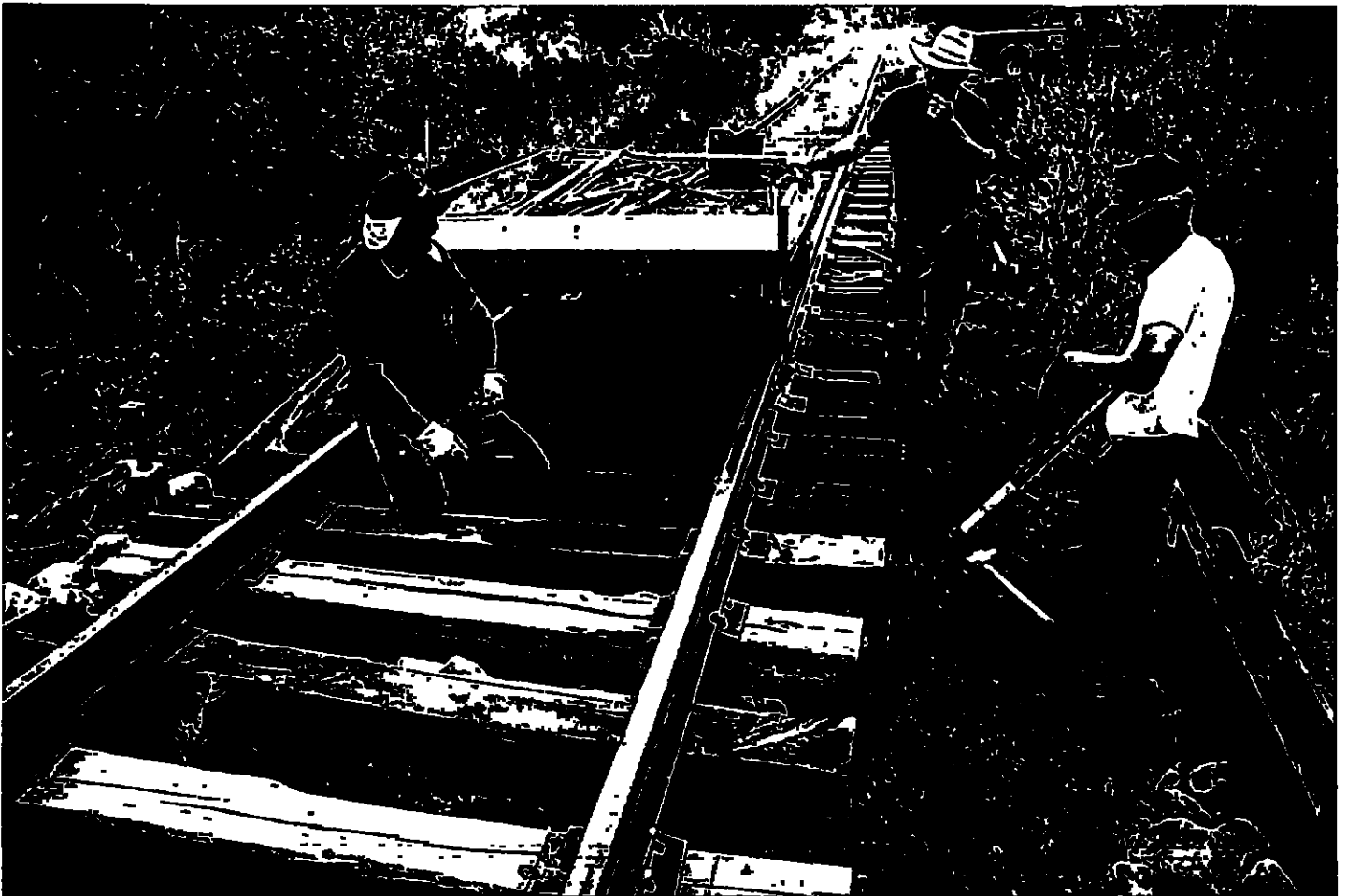
replacement of ties, spiking, leveling, gauging and filling with ballast .....
