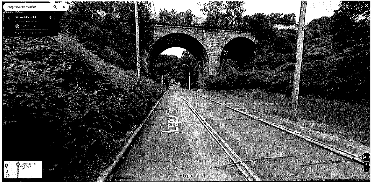
Viaduct over Leech Farm Road 1b
