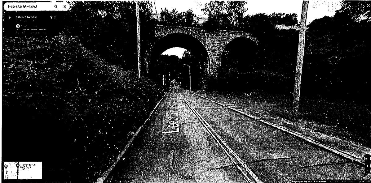
Viaduct over Leech Farm Road 1b
