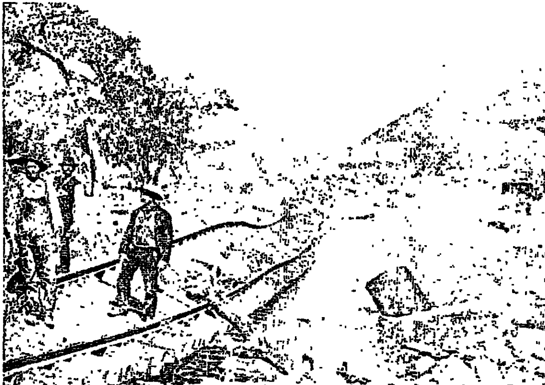
Figure 7. Track Washout at Eccles, east of Caliente, 1907.
