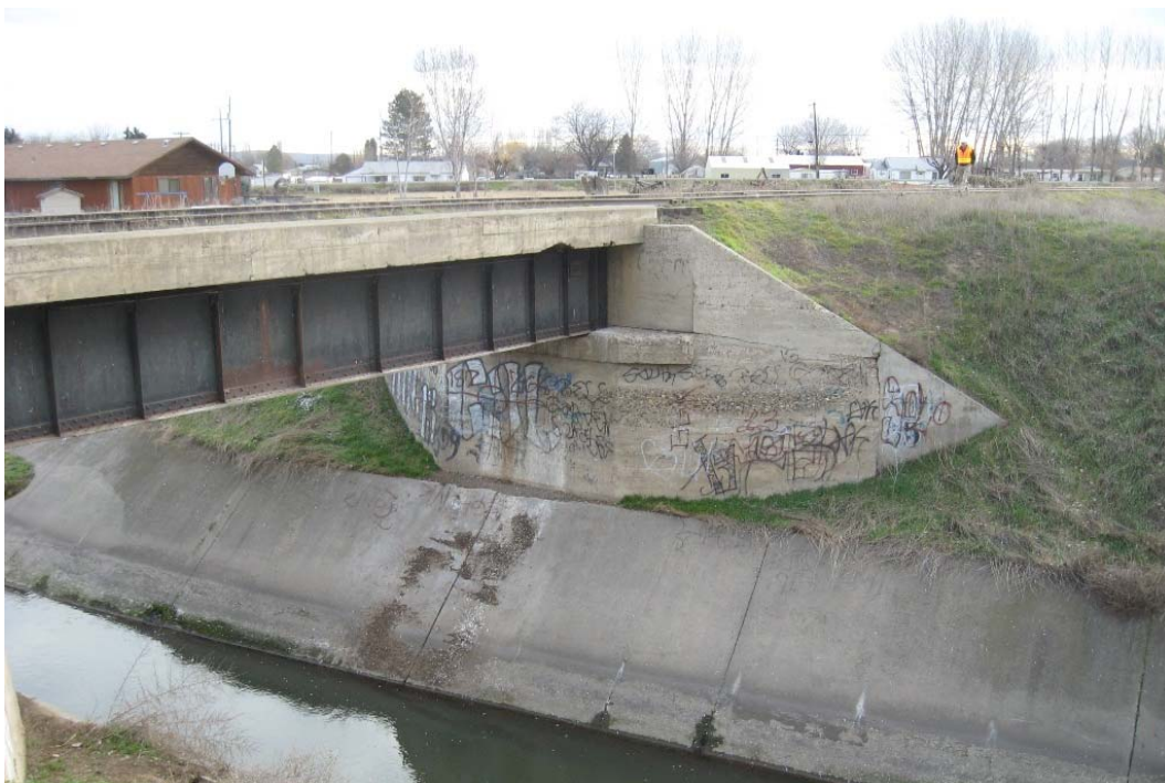
Figure 14. Bridge over Sulphur Creek Wasteway, looking northeast
