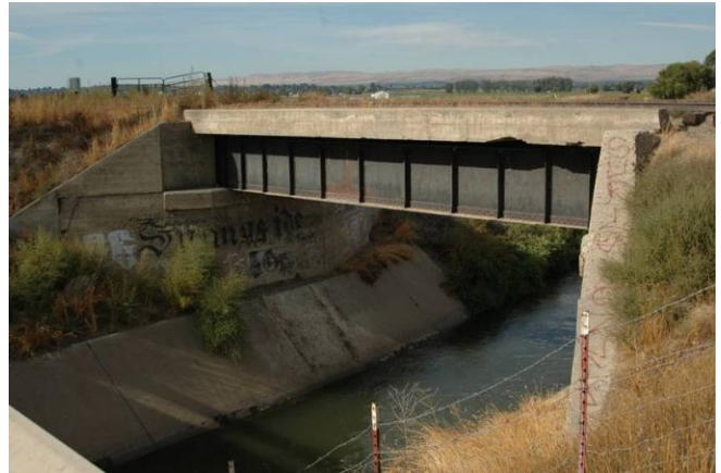
Railroad bridge over irrigation ditch, Midvale, looking northwest. 2010
