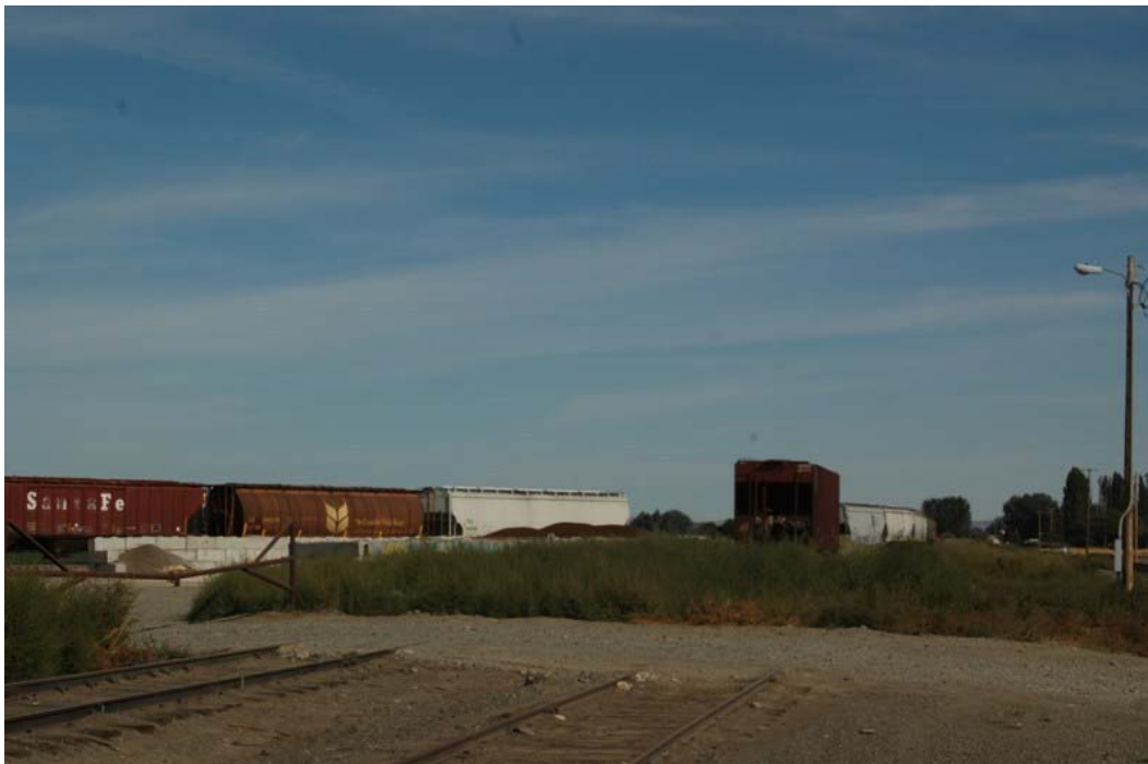
Figure 10. Railroad corridor at Sunnyside Branch, Midvale, looking east.
