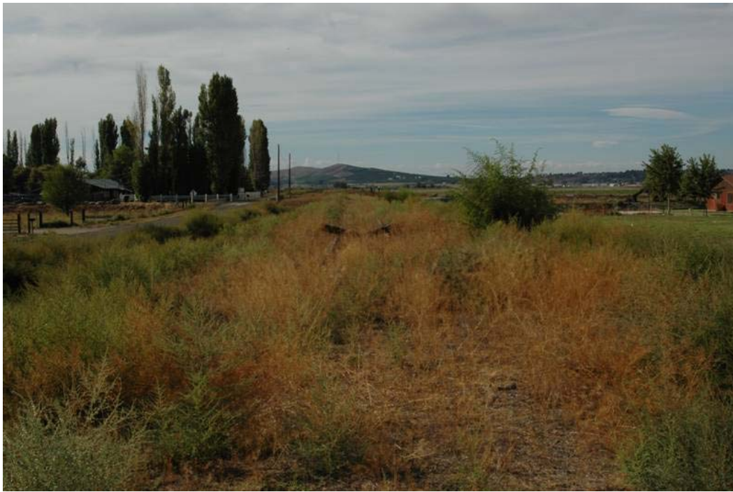
Figure 3. Railroad corridor at beginning of project area at MP 62.75, Midvale, looking west.
