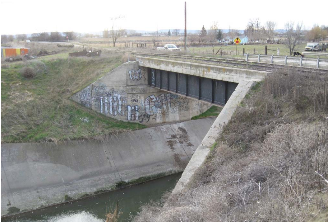
Figure 12. Bridge over Sulphur Creek Wasteway, looking southeast.
