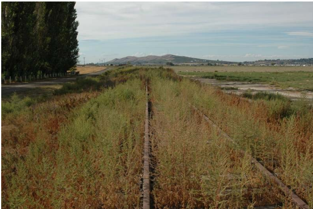
Figure 4. Railroad corridor at MP 63, Midvale, looking west.
