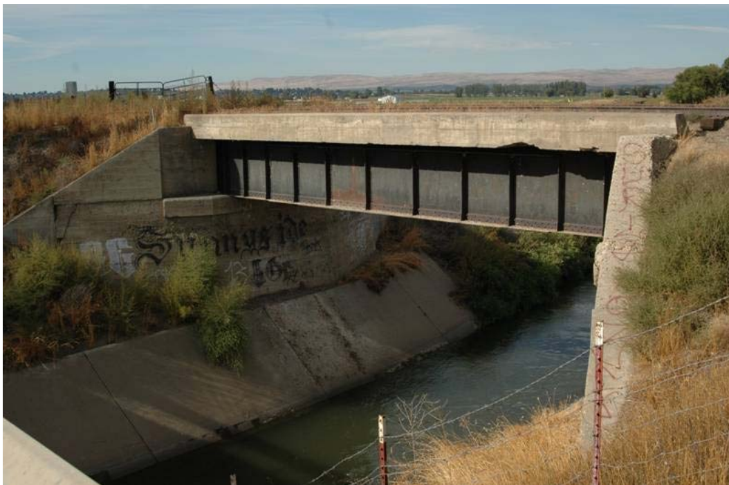
Figure 13. Bridge over Sulphur Creek Wasteway, looking northwest
