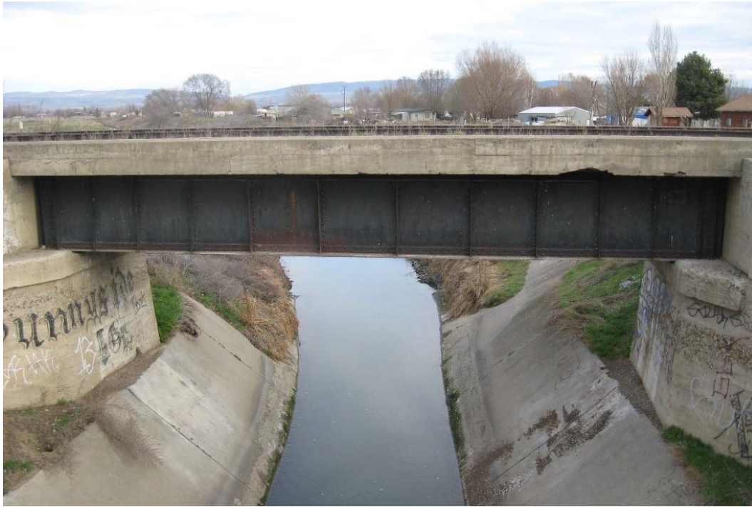
Figure 11. Bridge over Sulphur Creek Wasteway, looking north.
