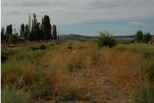
Railroad corridor at beginning of project area at MP 62.75, Midvale, looking west. 2010
