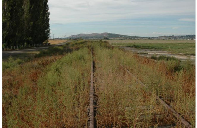
Railroad corridor at MP 63, Midvale, looking west. 2010
