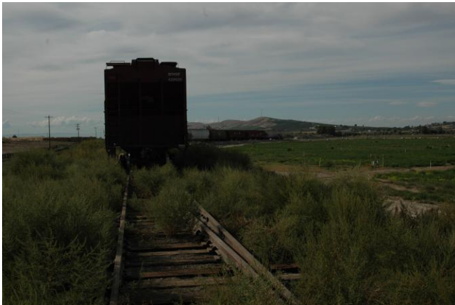
Railroad corridor at Sunnyside Branch, Midvale, looking west. 2010
