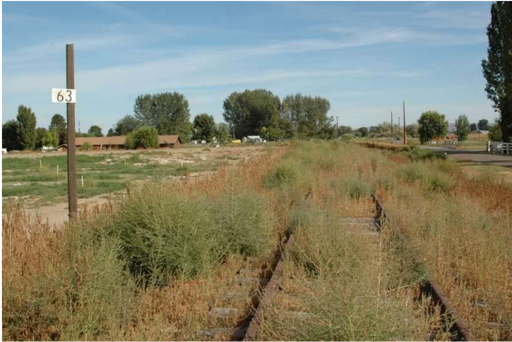
Figure 5. Railroad corridor at MP 63, Midvale, looking east.
