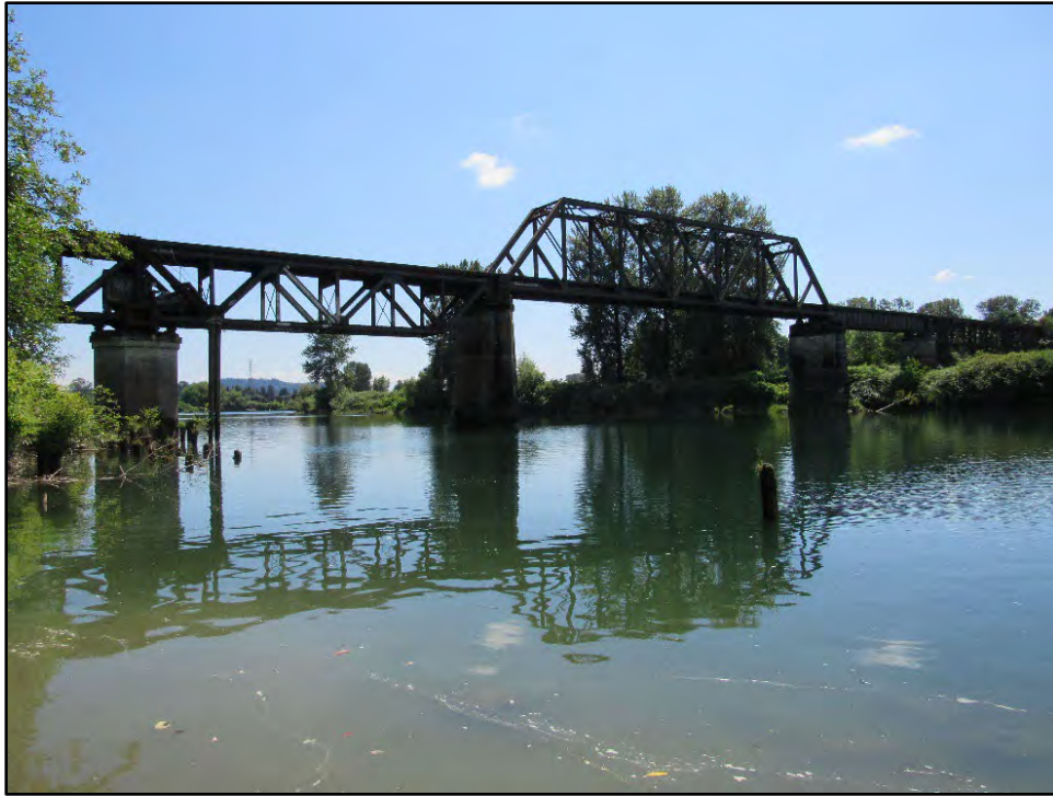
Figure 2: The Snohomish River Bridge, view facing south.
