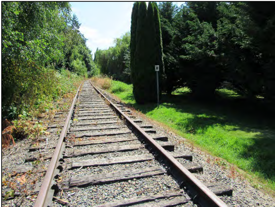
Figure 1: SLS&E Snohomish Segment south of milepost 34.3 showing typical standard-gauge rails with pressure-treated replacement wood ties and a typical whistle stop sign at right.
