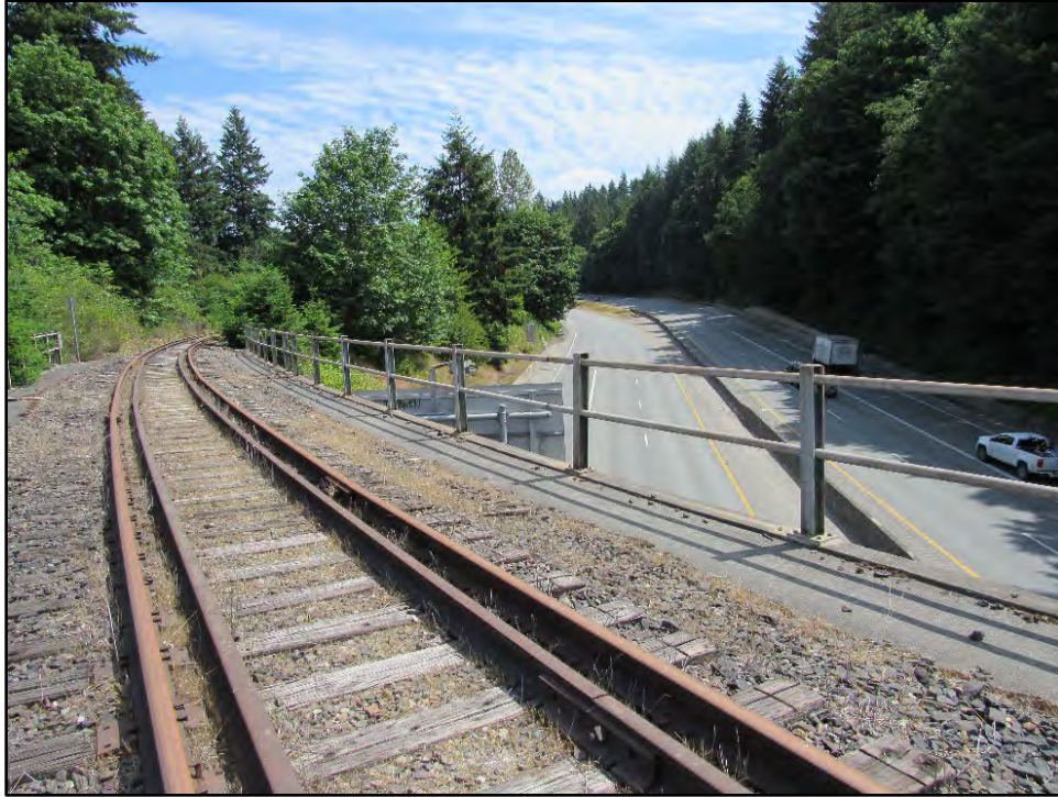
Figure 3: The State Route 522 Rail Overcrossing, view facing northeast.
