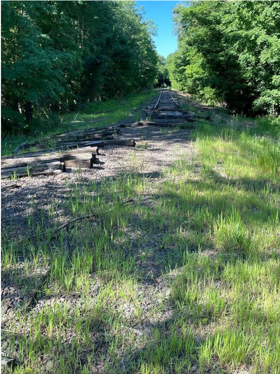
MP 12.0 approximately 300' of track removed
