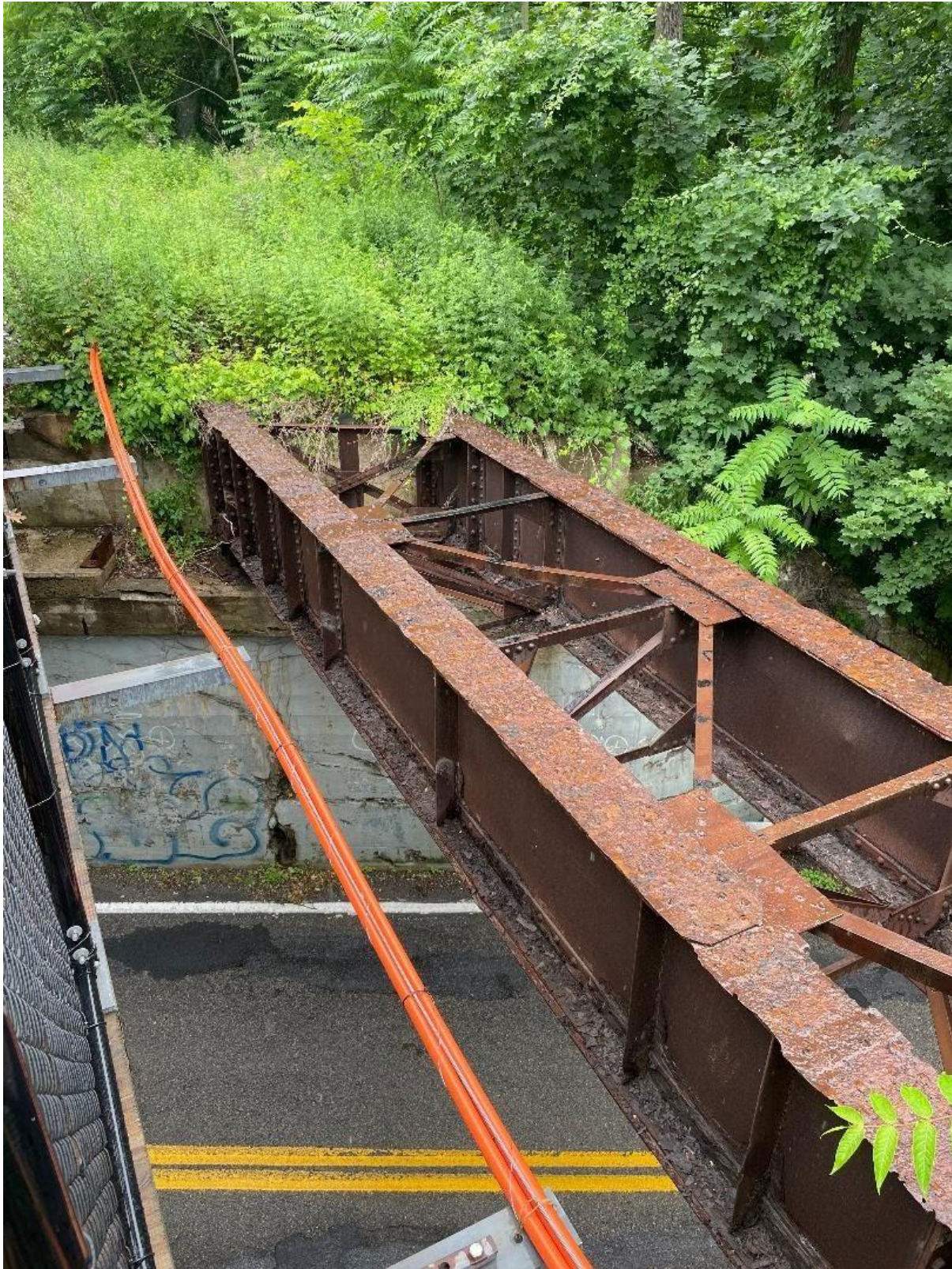
Bridge MP 31.03 NY-164 UG
