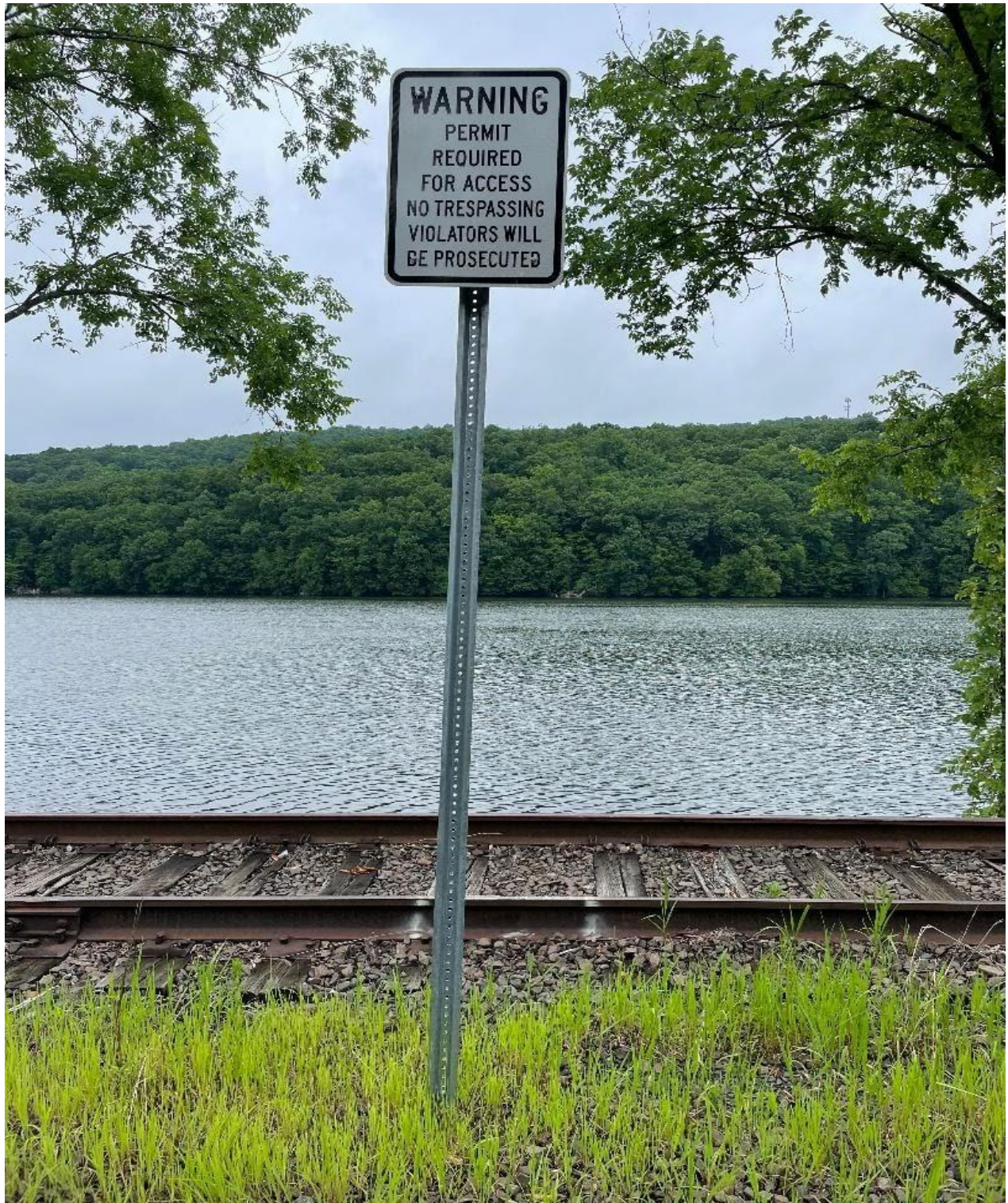
Signage in the Brewster area, too close to track.
