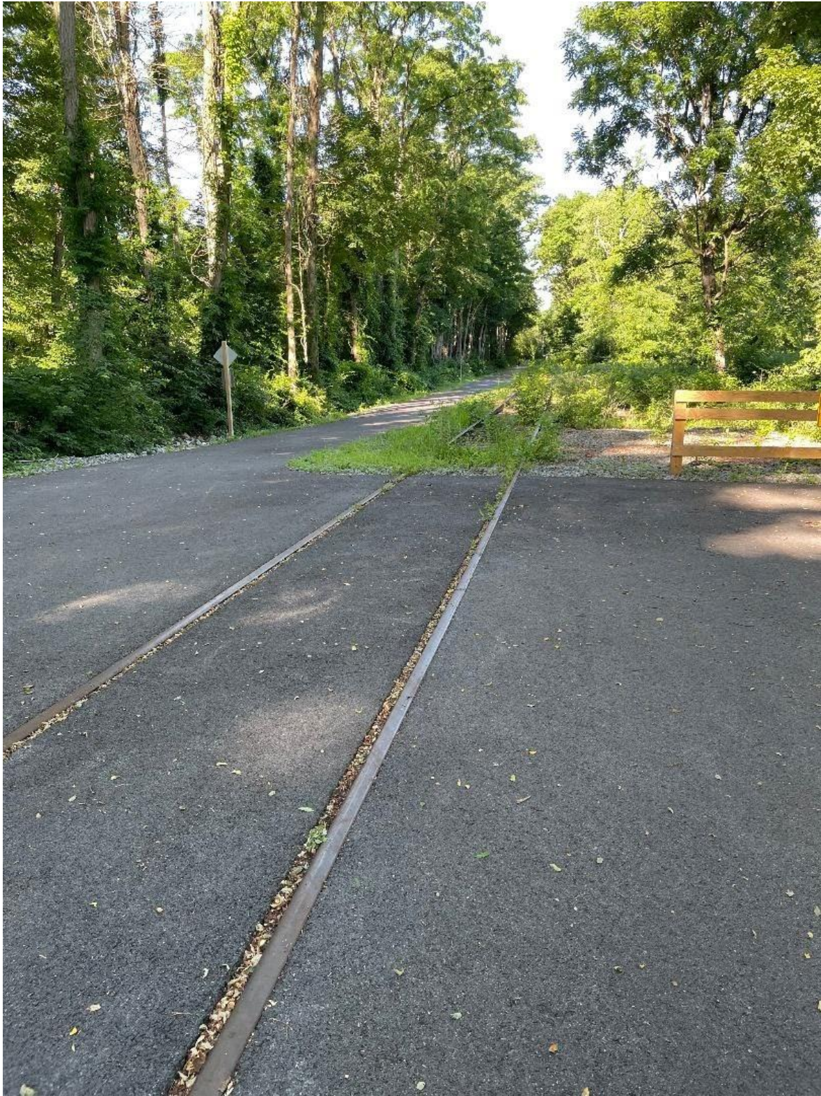
West side of Stormville, new crossing installed for path.
