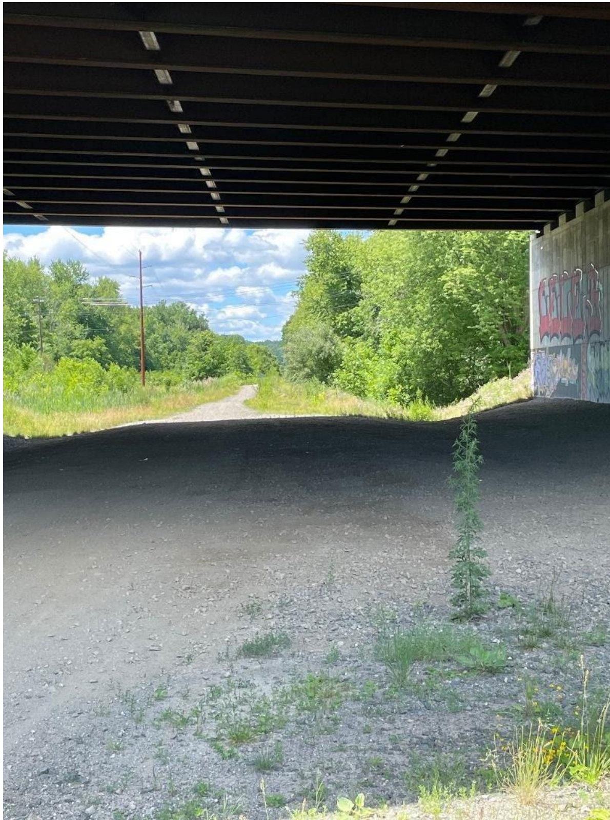
MP 5.50-5.40 Rail and bed removed under I-84 at least 400'
