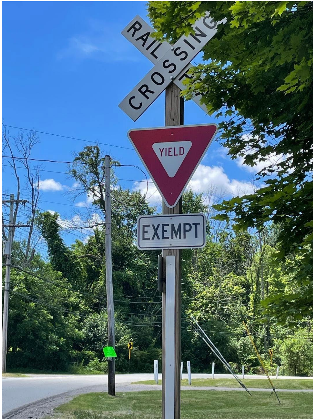
Example of what every crossing has for crossing protection along the Beacon Line
