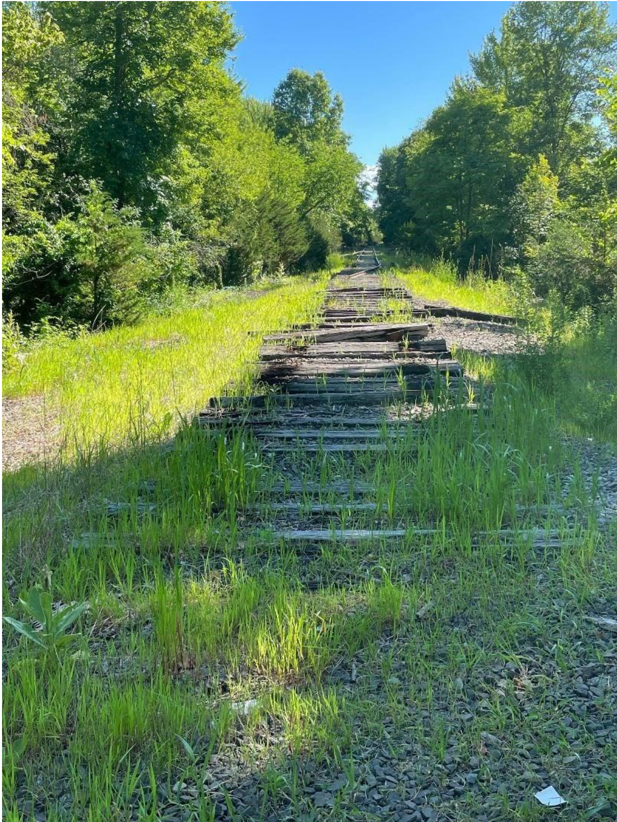
MP 12.0, Track removed approximately 300'
