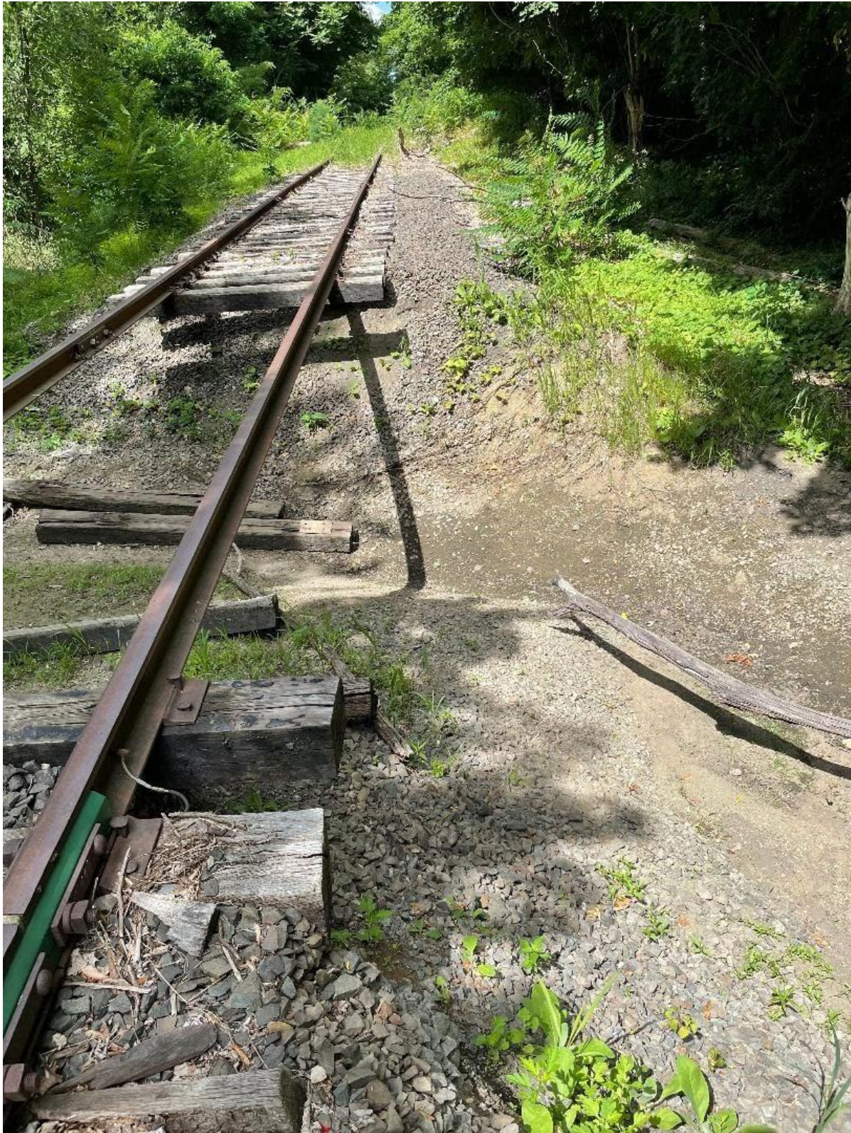
Wash MP 6.62, culvert
