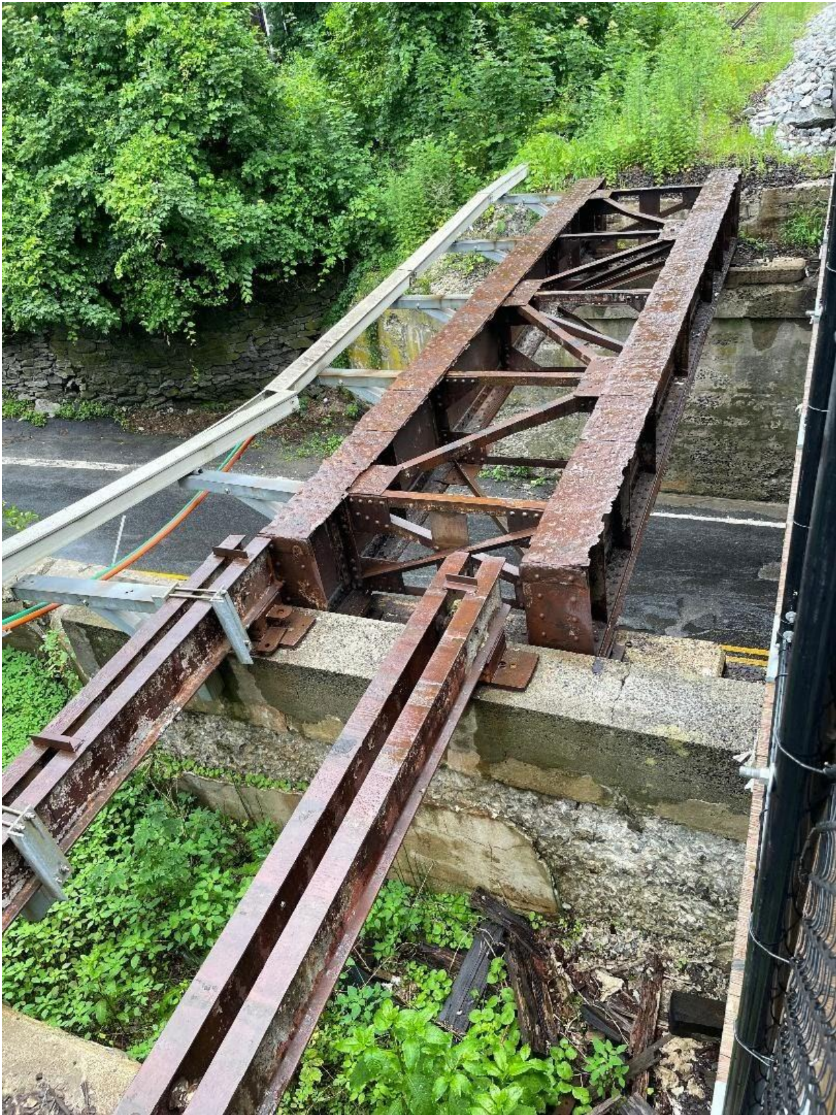
Bridge MP 30.02 NY-311
