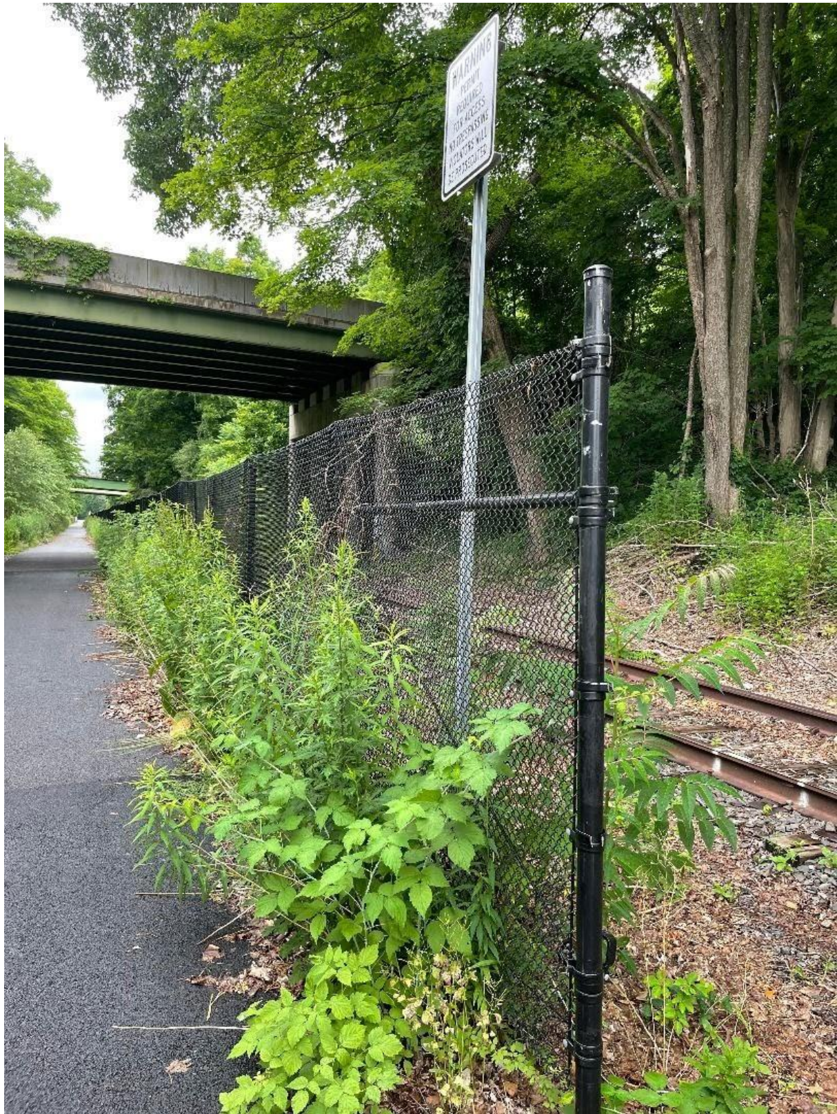
Most of the area Brewster area has a fence between path and tracks.
