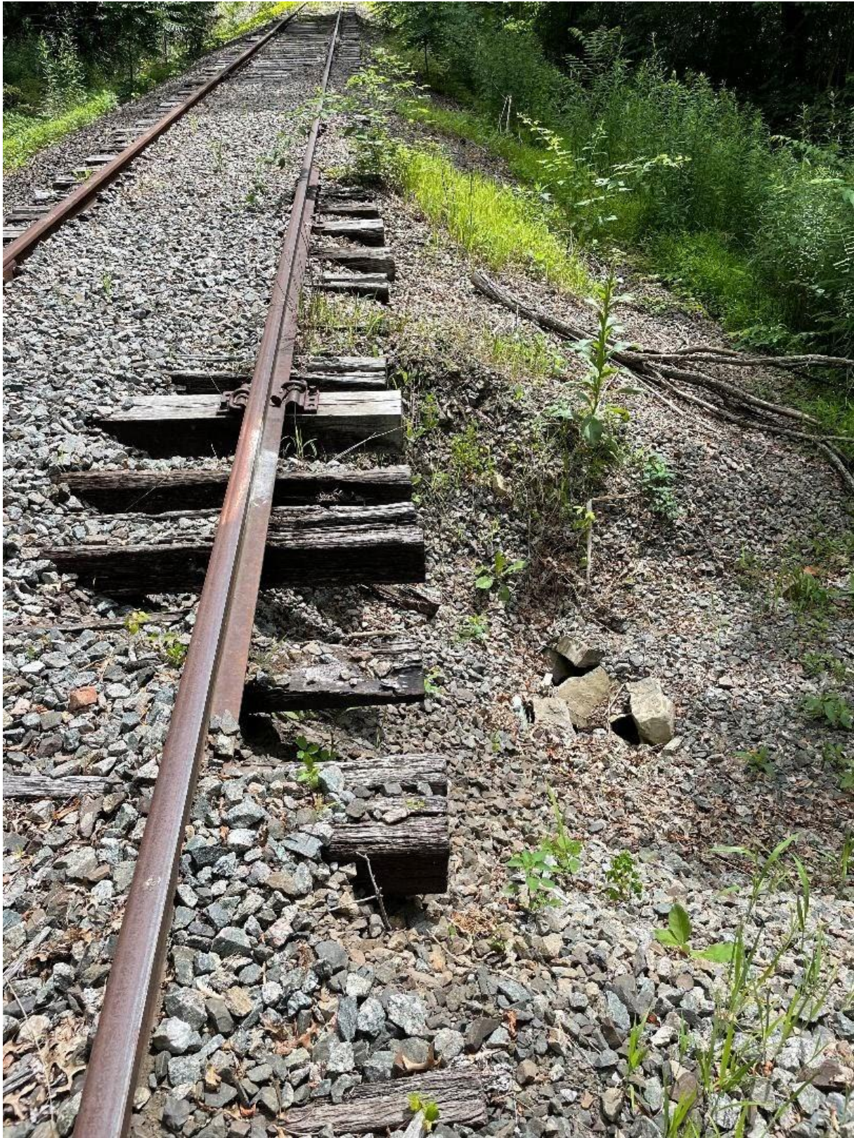
Wash MP 6.71, culvert
