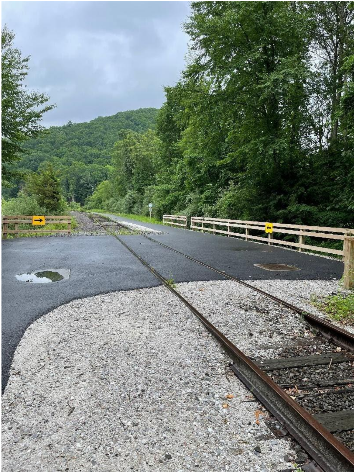
Dykeman's facing west, new crossing and fence.
