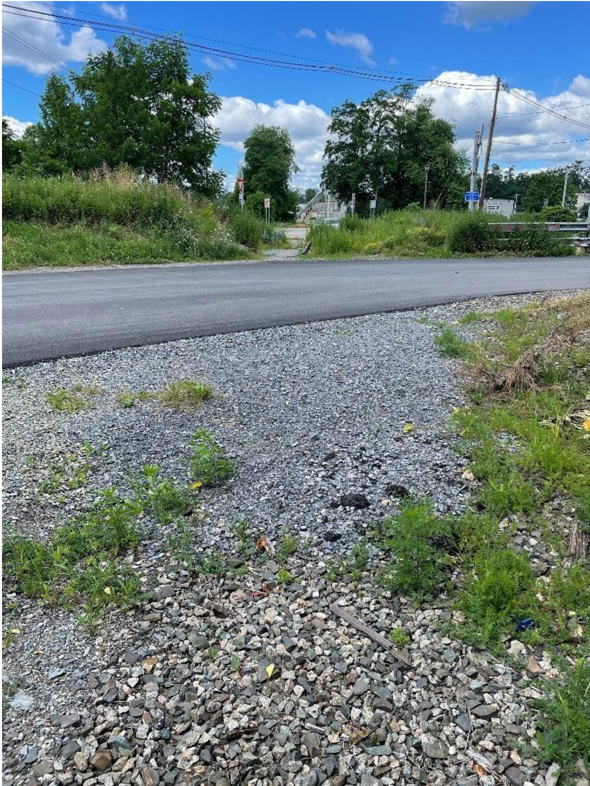
MP 6.48 Crossing removed, facing west at RT 9 which also will require work.
