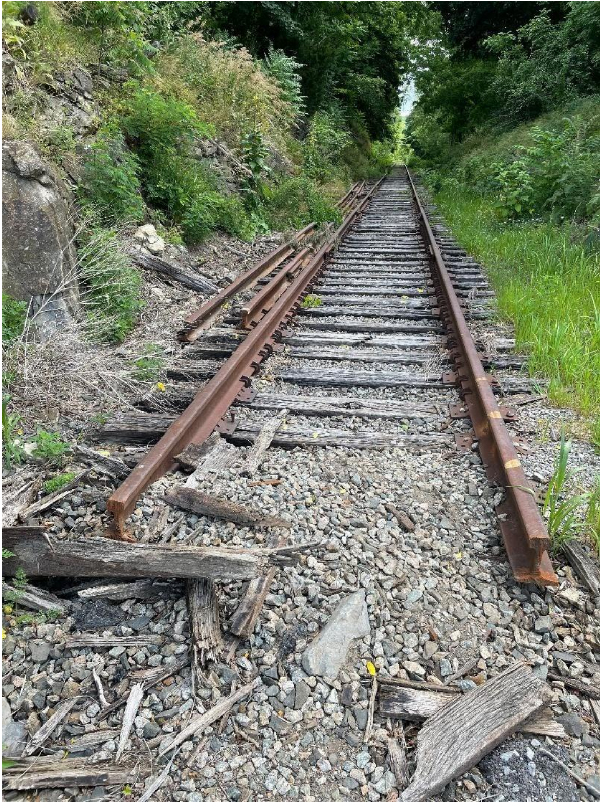
MP 6.48 crossing removed
