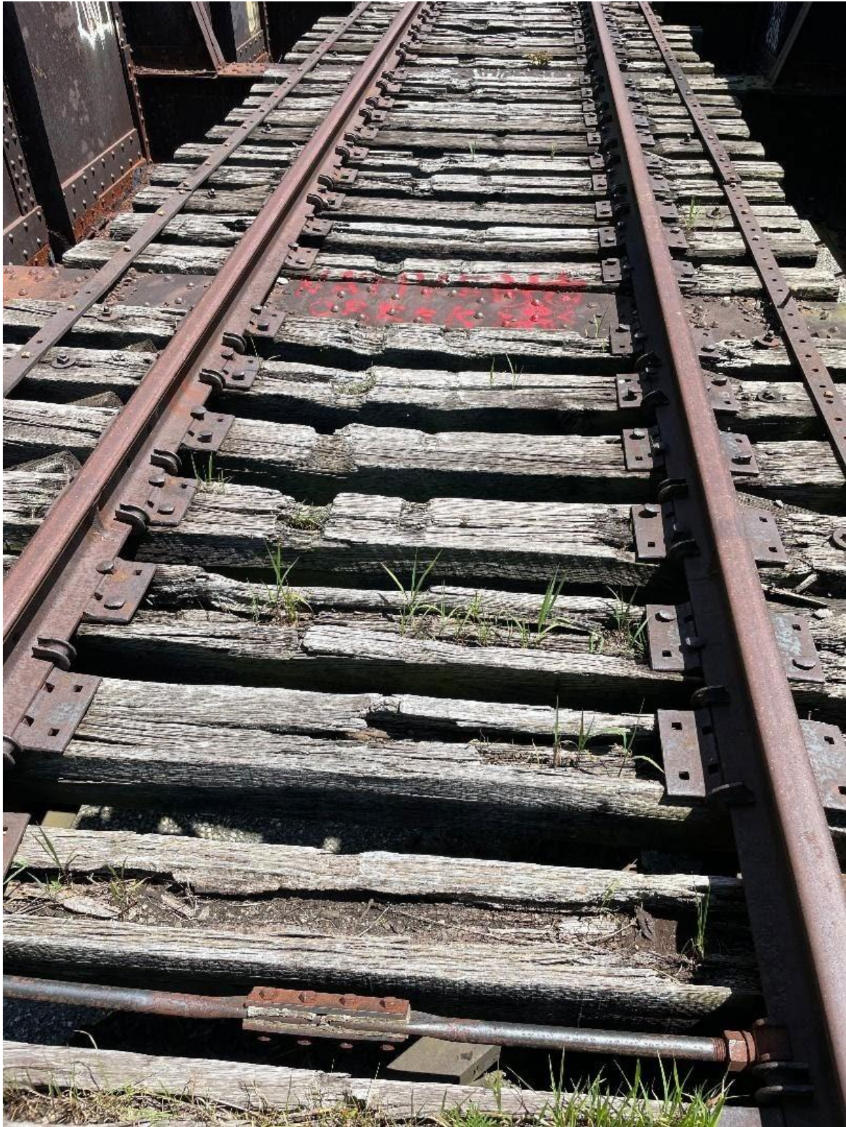
MP 0.63 Bridge Hudson Line.
