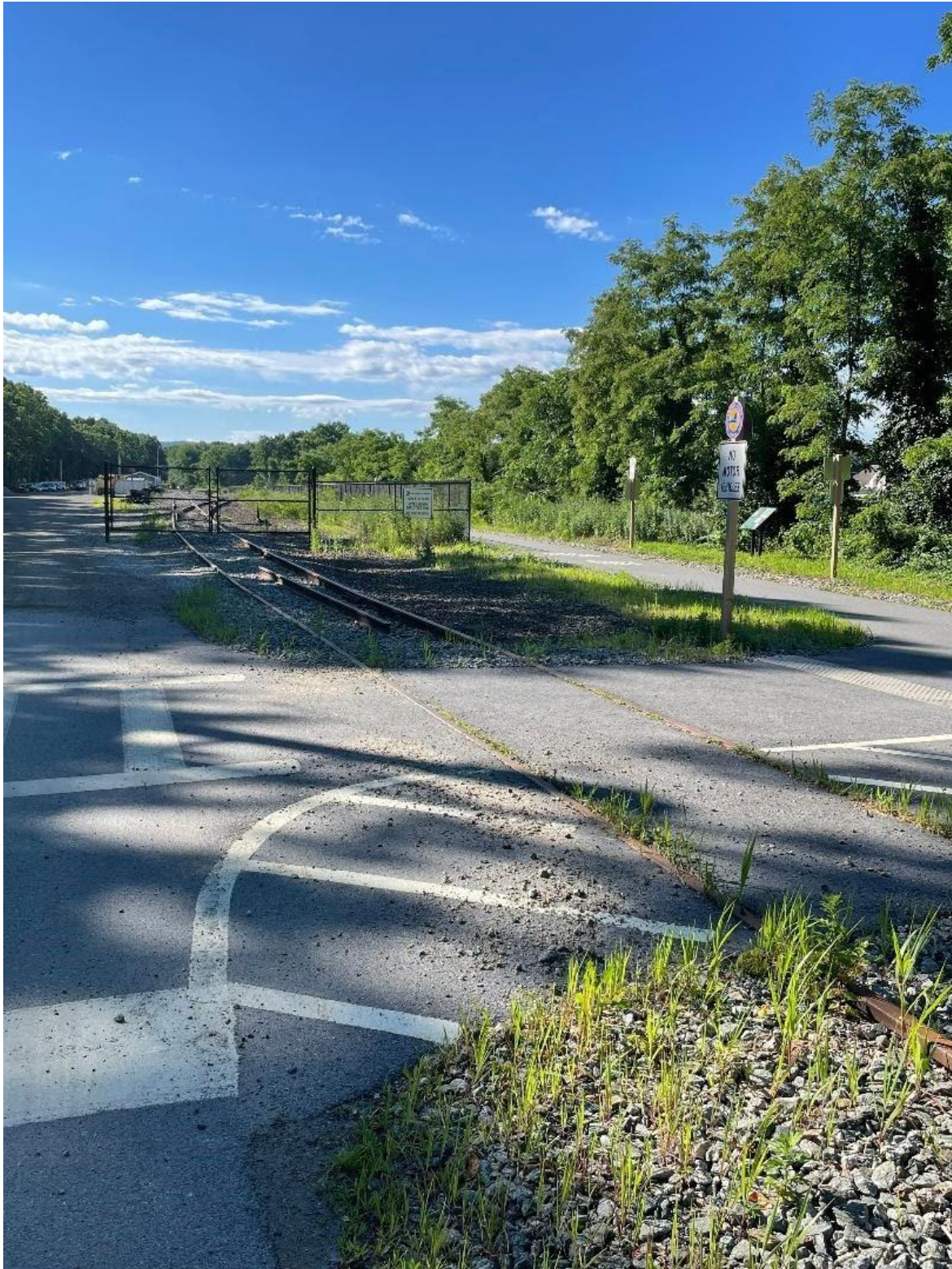
West end Hopewell Yard, track gated and crossing installed for path
