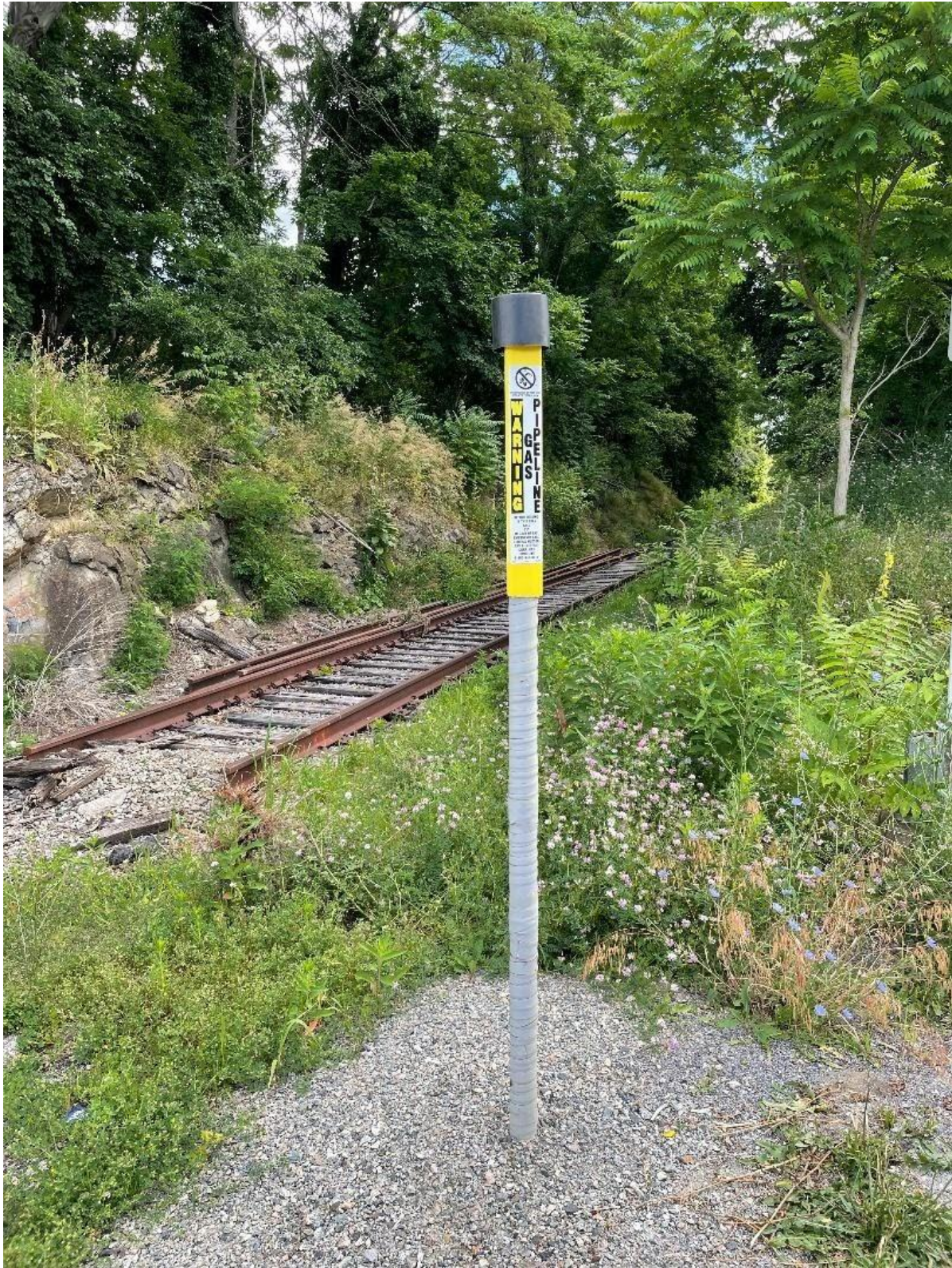
New Utility marker at MP 6.48 crossing, possibly reason for crossing removal.
