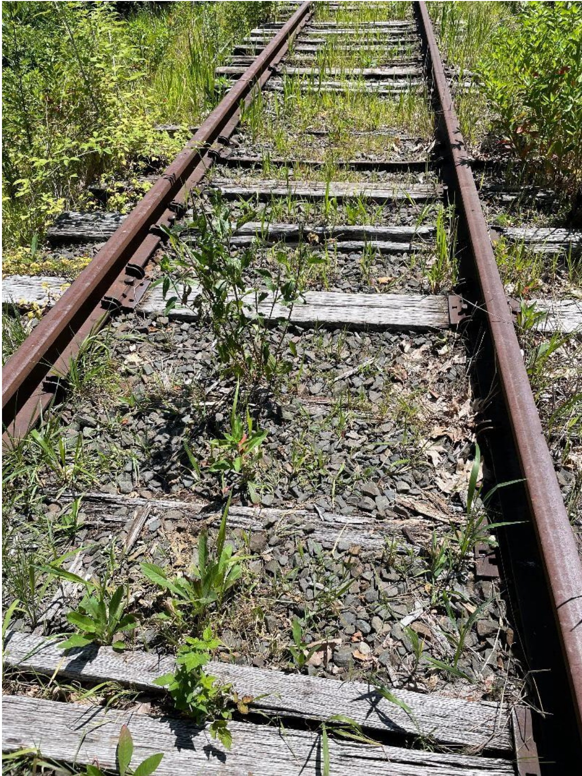
Example of tie condition, worse west of Hopewell
