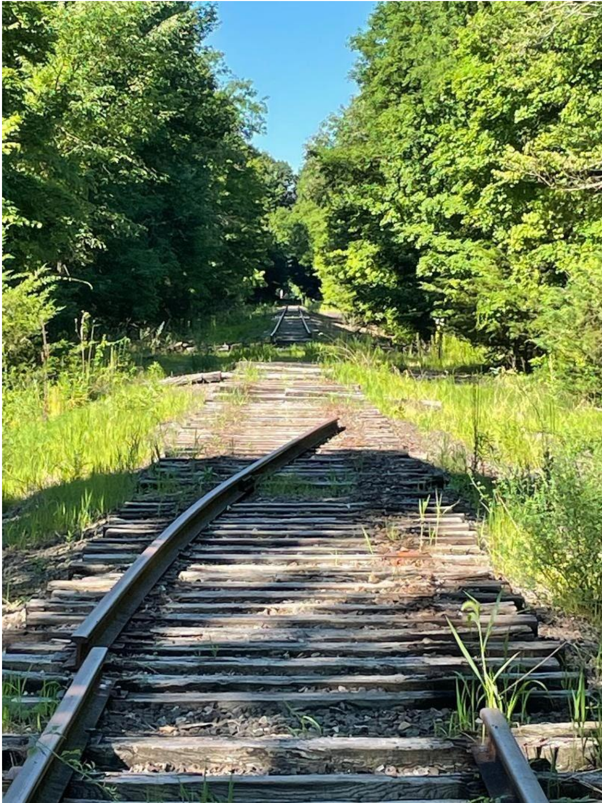
MP 12.0, approximately 300' of rail removed.
