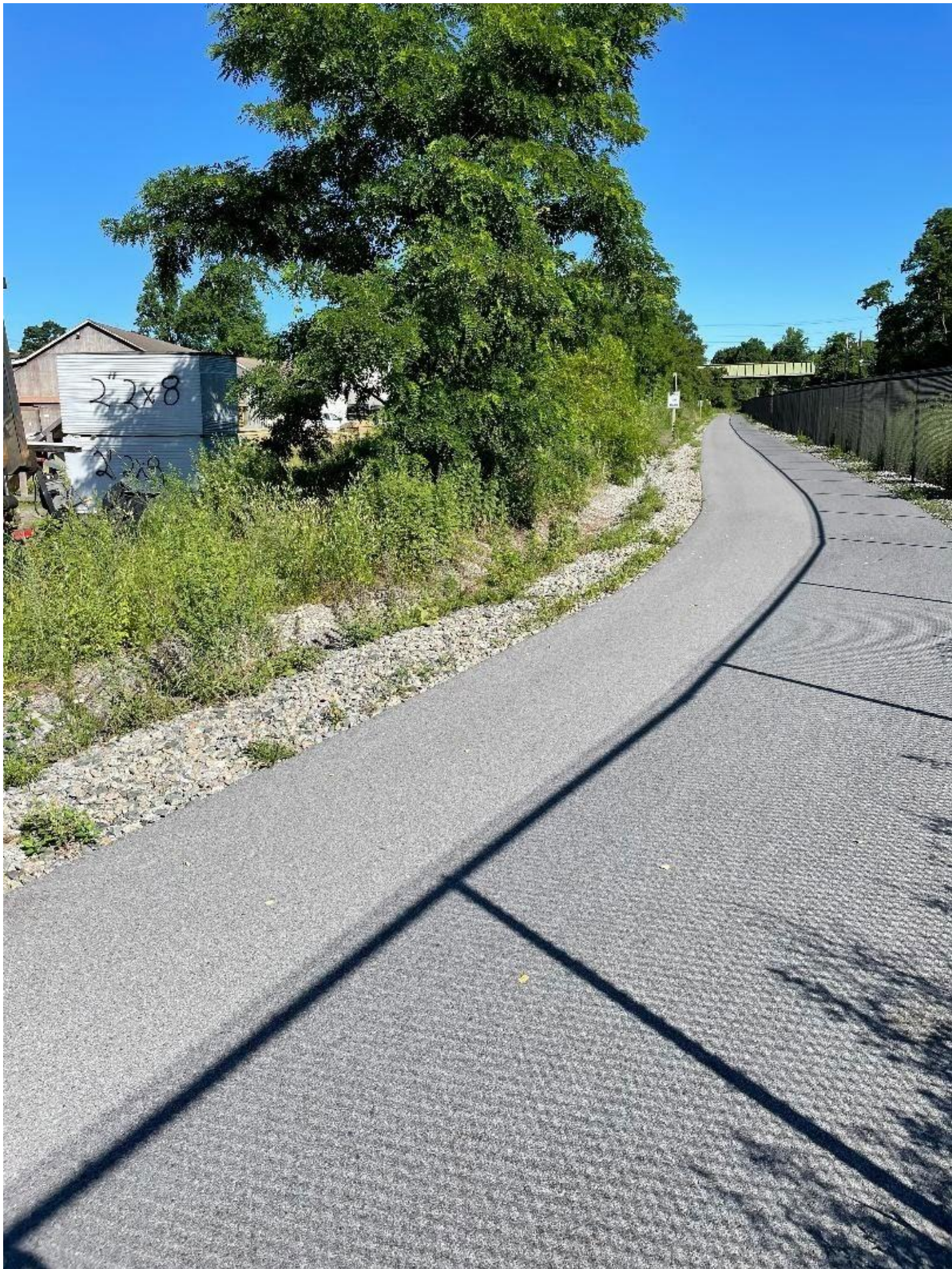
Hopewell Yard, Track lead to customer side of yard removed for path.
