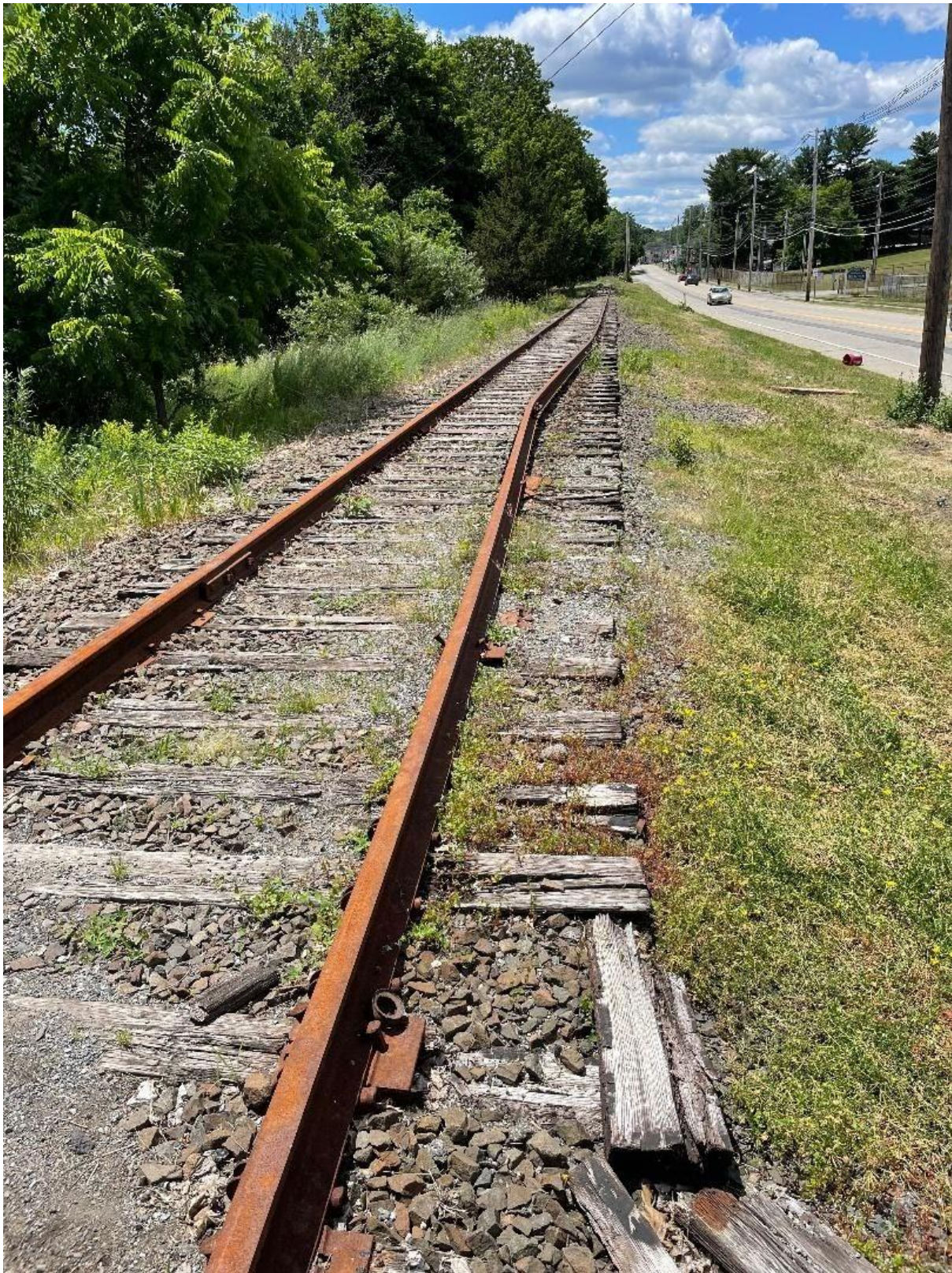
MP 3.45, rail not seated and plates missing.
