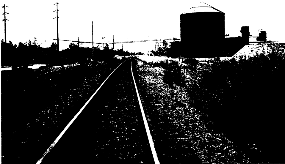
16 July 2003 Warroad, MN Standing on CN main track, facing South (timetable east), former location of West CN side track switch. Side track (disconnected) is to right, hidden in vegetation, but apparently intact, except for switch to main track. Note, that main track rail at this location is CWR.
