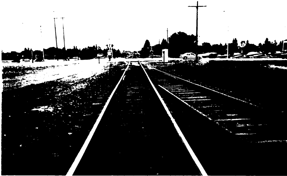
Photo #1 - Location: Warroad, MN standing on CN Main - facing South at East Transfer Track switch.
