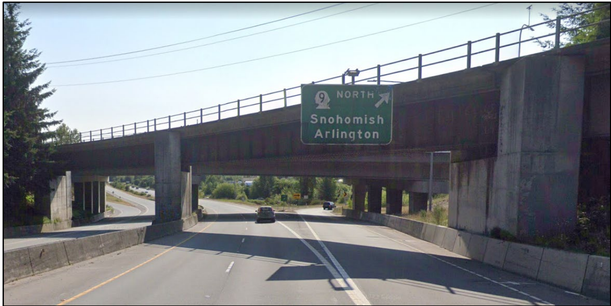
Figure 4: The State Route 522 Rail Overcrossing, view facing southwest from State Route 522 (Google Maps July 2023).
