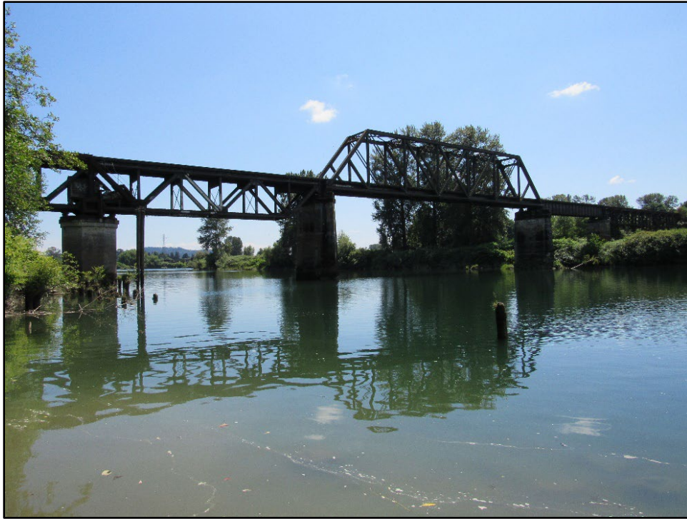
Figure 2: The Snohomish River Bridge, view facing south.
