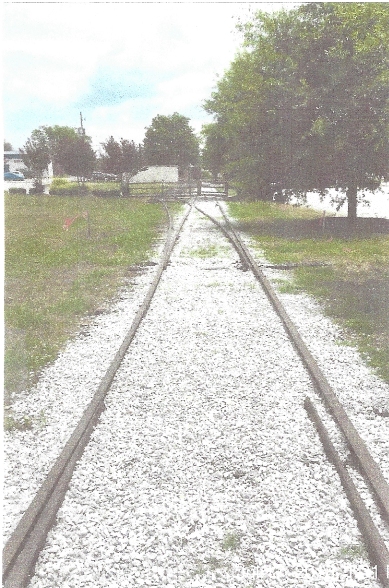
GWRC Photograph 6 Refurbished mainline track facing east from just beyond eastern side of Chandler Street dated July 20, 2018.
