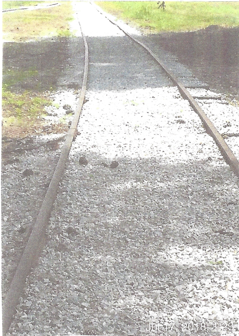
GWRC Photograph 7 Refurbished mainline track facing east from a point west of the point at which locomotive is parked in GWRC photograph 5. turntable track at top left of the photograph. Dated July 17, 2018.
