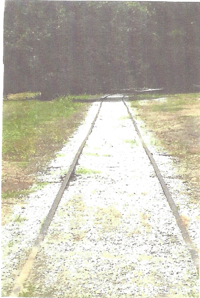
GWRC Photograph 8 Refurbished mainline track facing west from a point that is to the west of the point at which locomotive is parked in GWRC photograph 5. Dated July 17, 2018.
