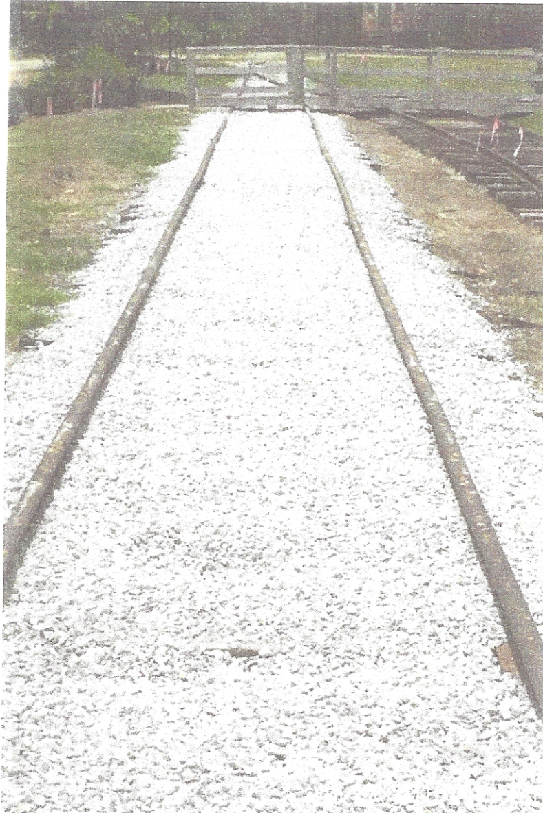
GWRC Photograph 4 Refurbished mainline track and partially refurbished runaround track west from South Webb Street dated July 17, 2018
