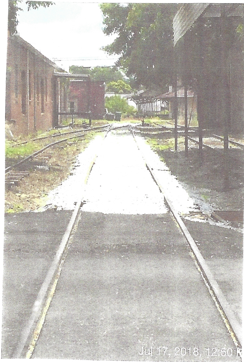
GWRC Photograph 3 Refurbished mainline track and start of runaround track facing east from South Webb Street to Jackson Street dated July 17, 2018
