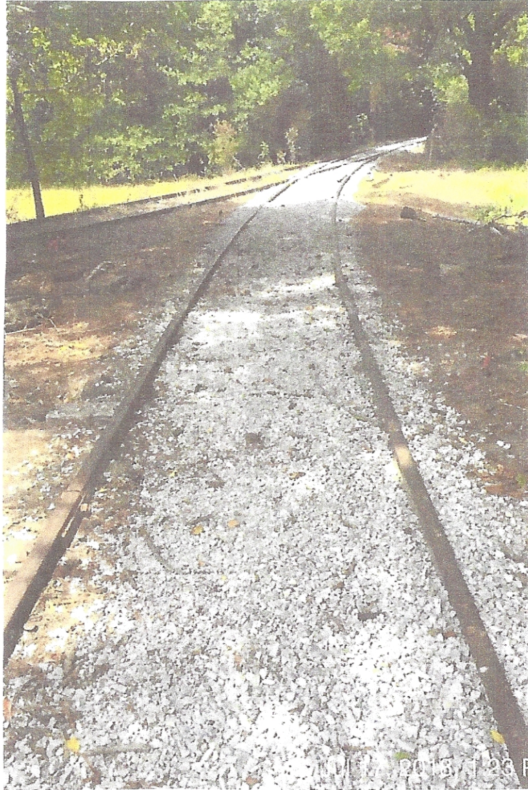
GWRC Photograph 9 Refurbished mainline track facing west from point located on photograph 8. Dated July 17, 2018.
