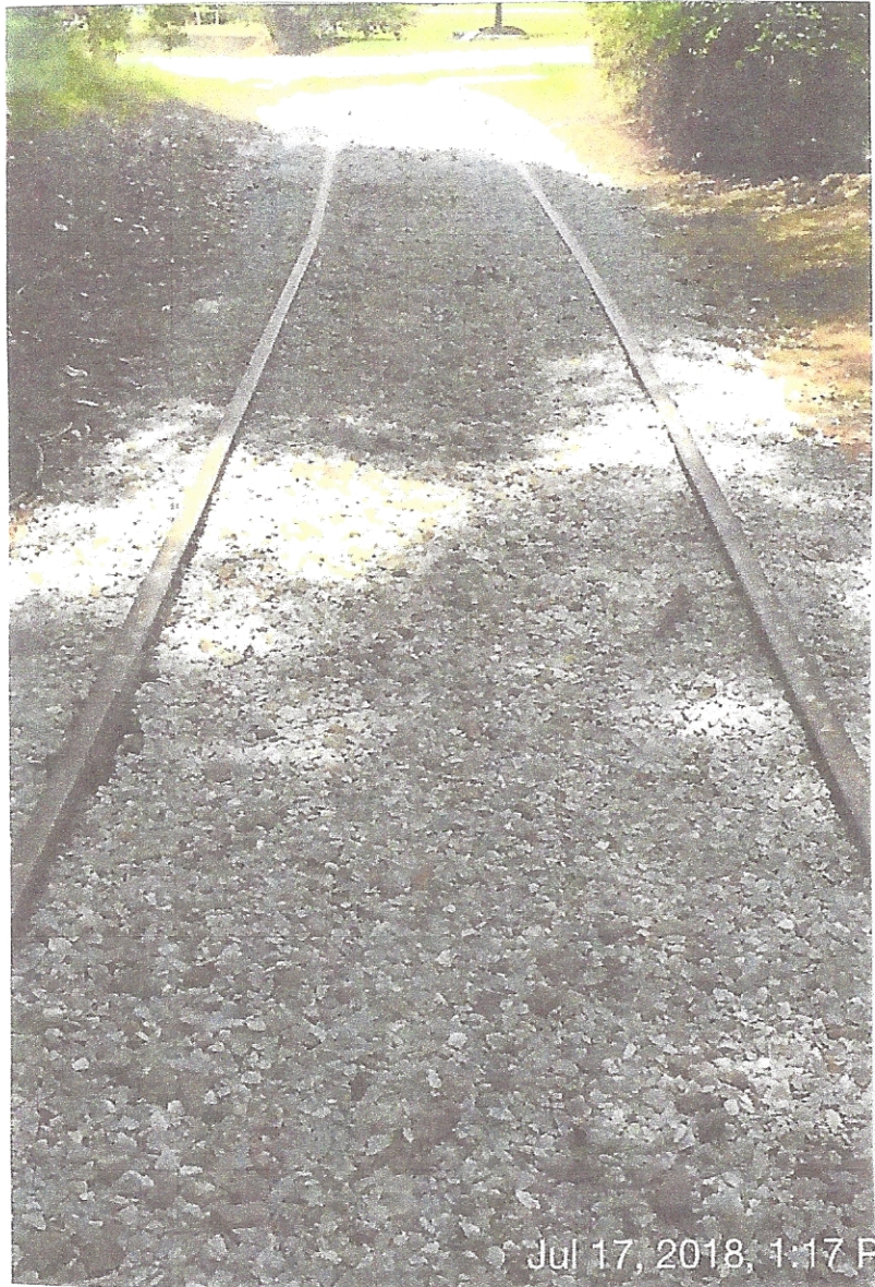
GWRC Photograph 11 Refurbished mainline track facing further west and showing the crossing at Athens Street. Dated July 17, 2018.
