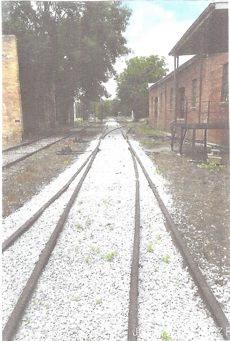
GWRC Photograph 2 Refurbished mainline track and start of runaround tracks facing west from Jackson Street to South Webb Street dated July 17, 2018
