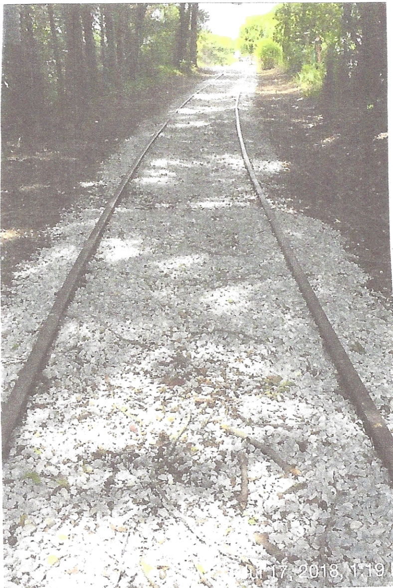
GWRC Photograph 10 Refurbished mainline track facing further west toward Athens Street. Dated July 17, 2018.
