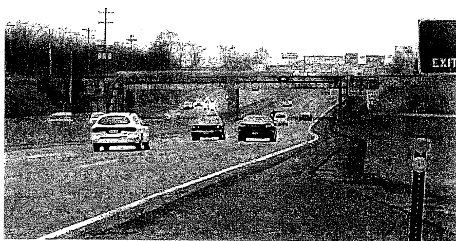
Bridge Viewed From I-75 - Looking South
