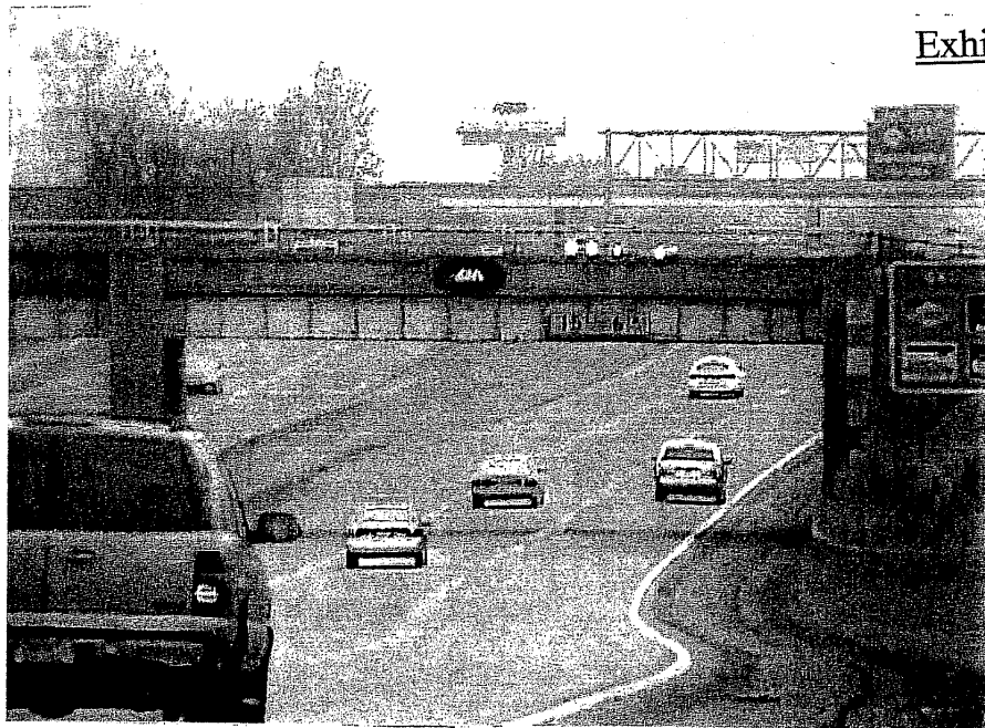
Bridge Viewed From I-75 - Looking South
