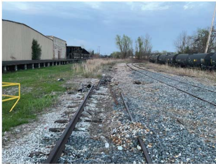
Frame 110. Looking northeasterly from the north side of the crossing at East Scott Street. Photographed by Charles W. Rex IV, MAI, AI-GRS on March 3, 2023.
