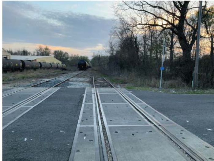
Frame 109. Looking southwesterly at the crossing at East Scott Street. Photographed by Charles W. Rex IV, MAI, AI-GRS on March 3, 2023.
