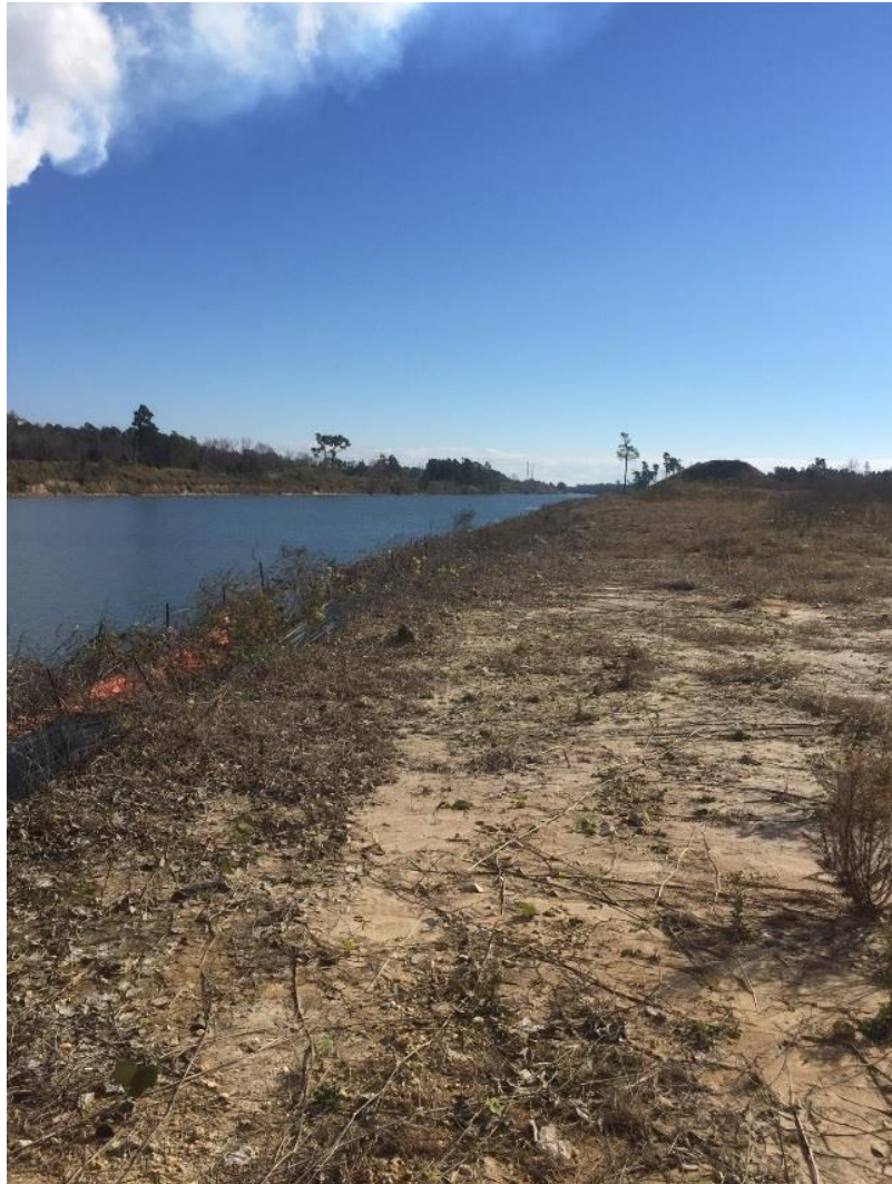
Photograph 1 Diversion Canal, View North.
