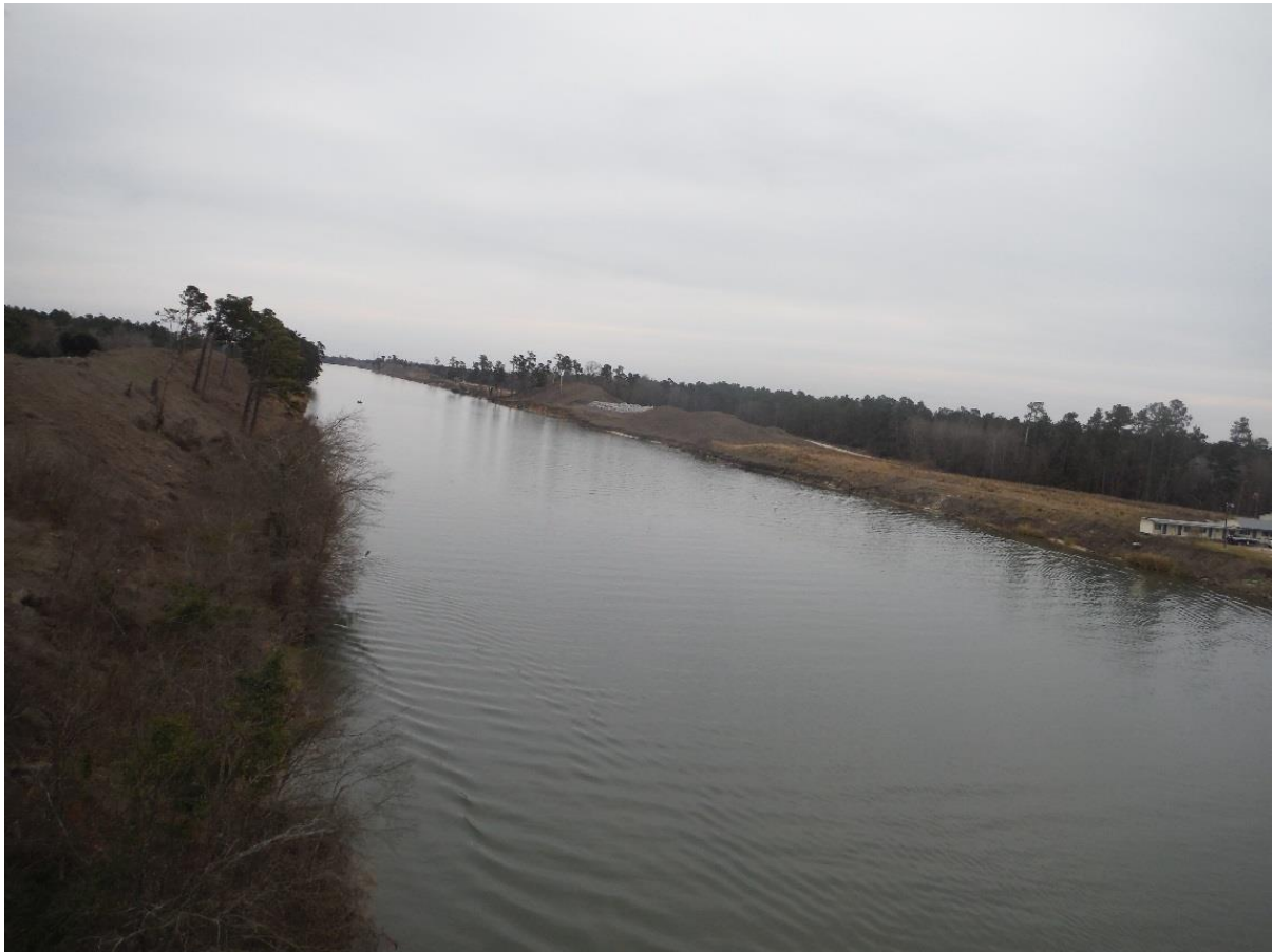
Photograph 2 Diversion Canal, view southeast
