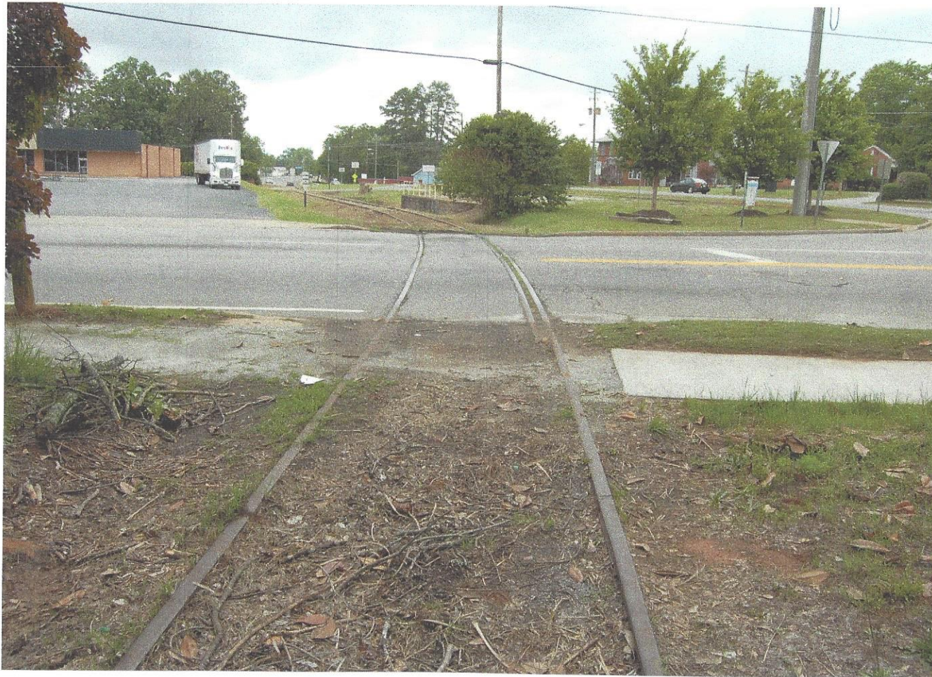
Photograph 23: GWRC Mainline Crossing Athens Street and extension of Mainline on the West Side of Athens Street
