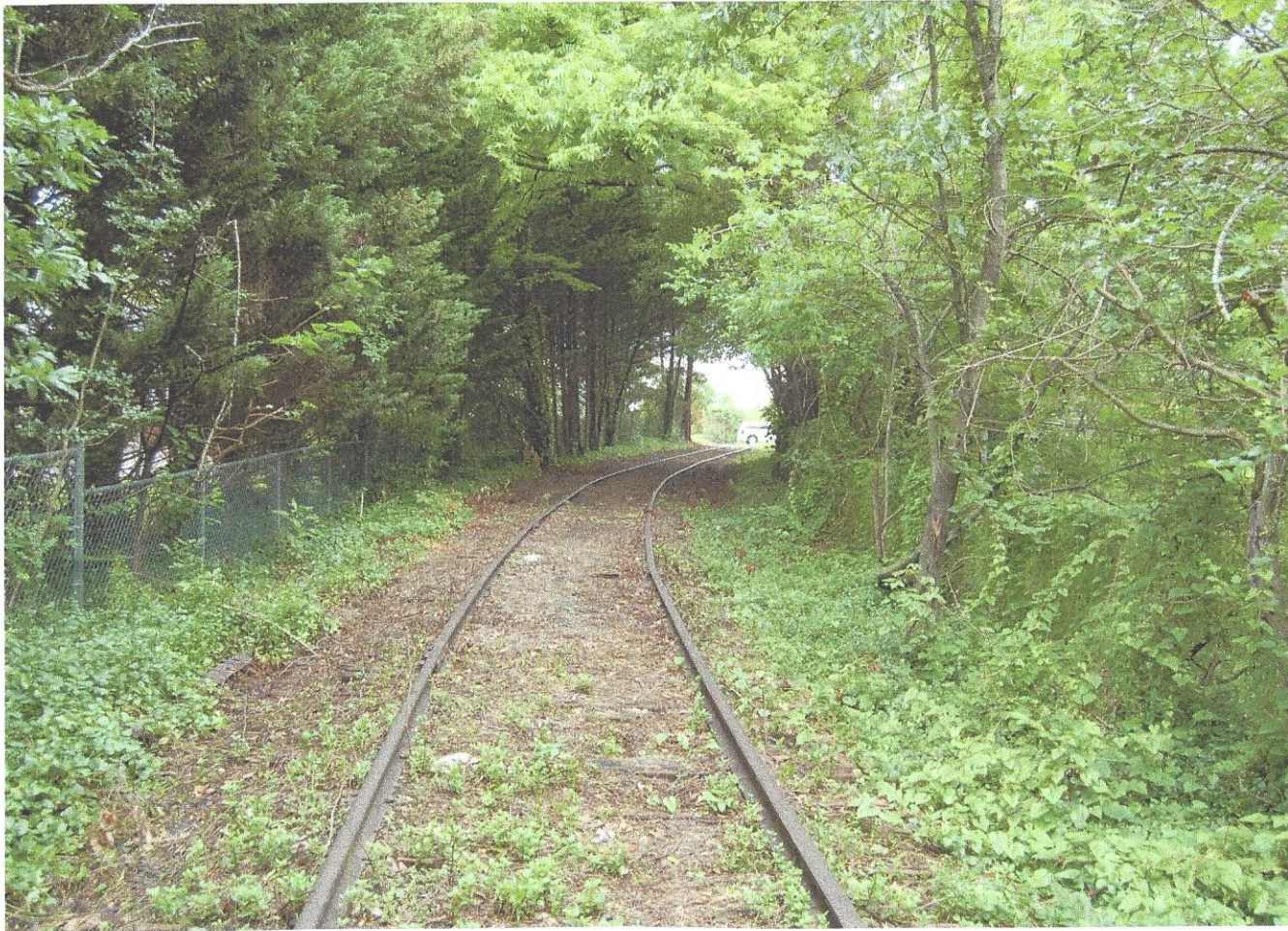
Photograph 19: GWRC Mainline Track with car passing over Mainline Track at Athens Street to the West
