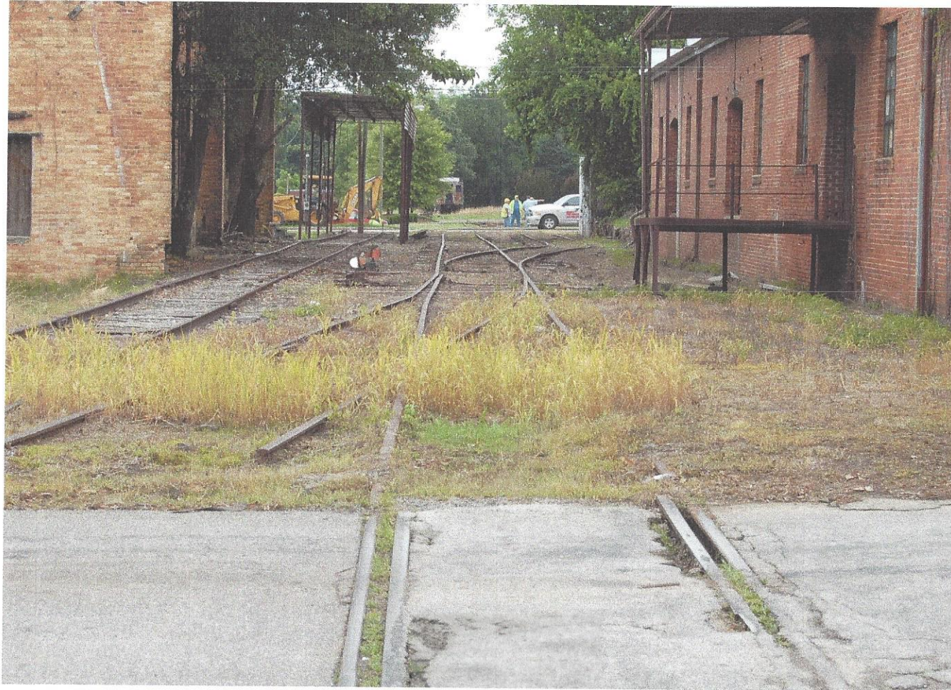
Photograph 1: GWRC Mainline at Jackson Street Intersection along with Industry Track to Left and intersection with Runaround Track to the Right
