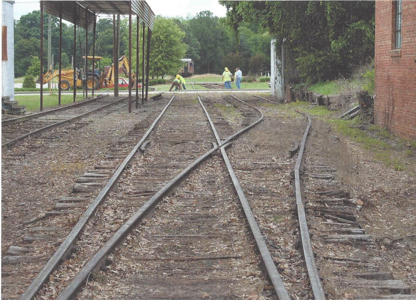
Photograph 3: GWRC Mainline and Runaround Track Intersection Between Jackson Street and Webb Street
