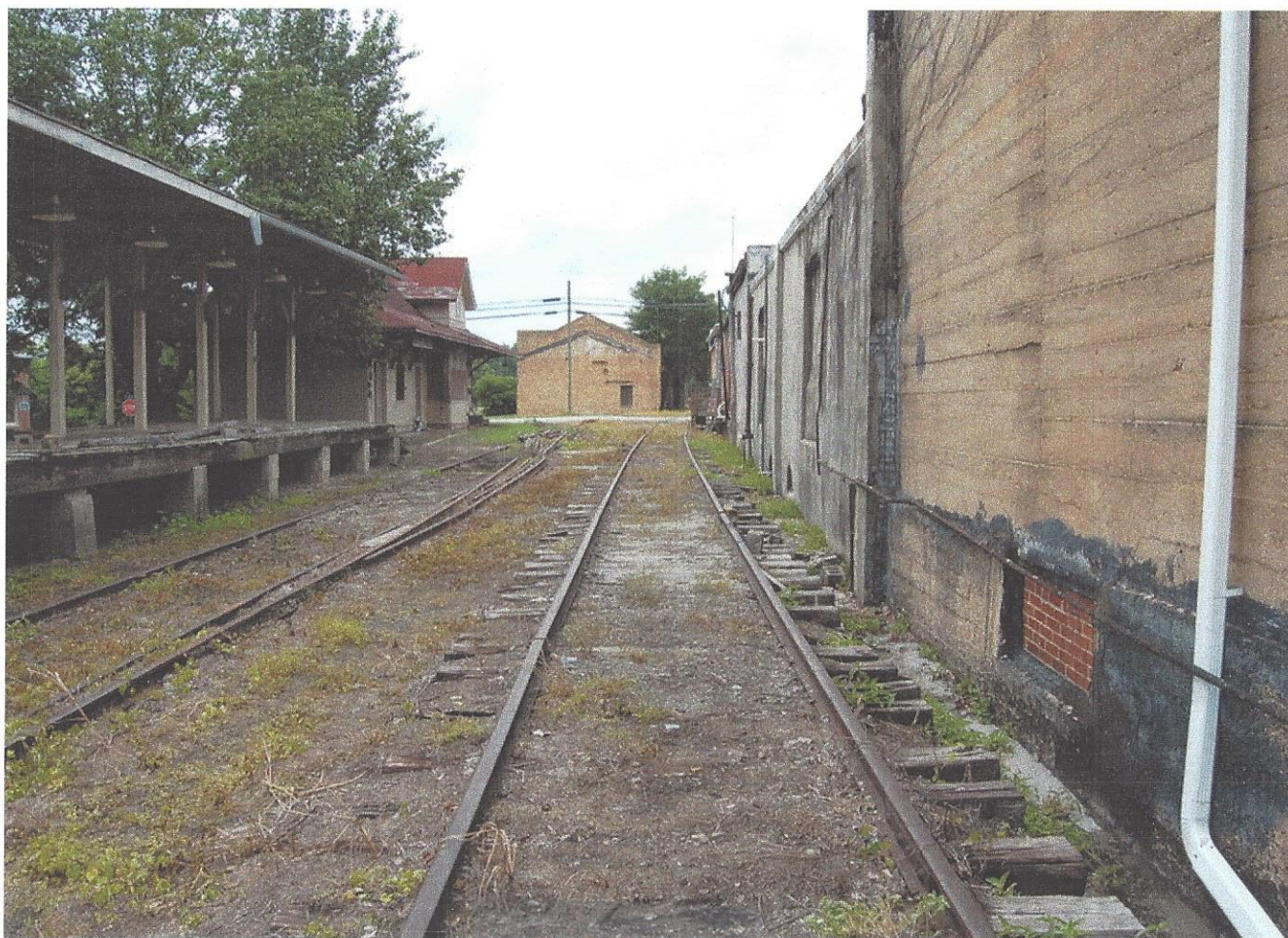
Photograph 0: GWRC Mainline looking westward from the east side of Jackson Street Reflecting historic loading platform and the Hartwell Depot on the left
