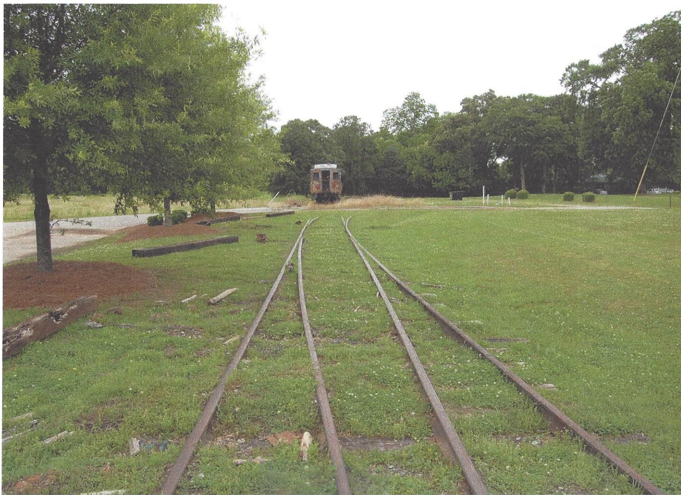
Photograph 9: Intersection of GWRC Mainline and parallel Runaround Tracks reflecting Rails laid prior to June 30, 1916
