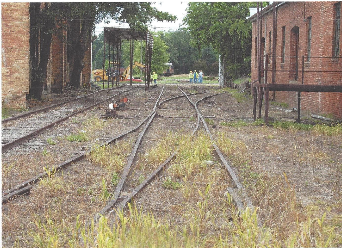
Photograph 2: GWRC Mainline and Runaround Track Between Jackson Street and Webb Street
