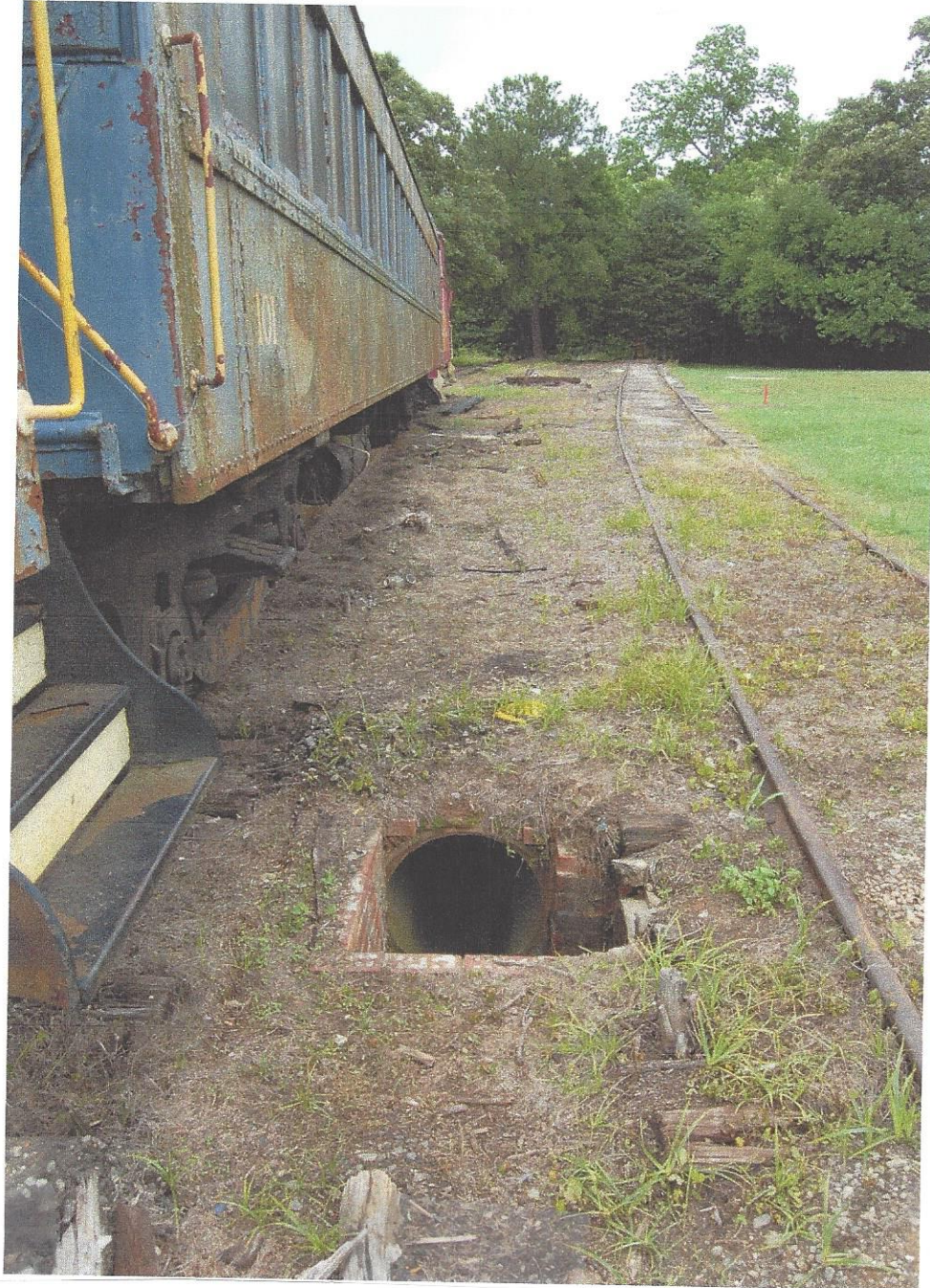
Photograph 13a: Drainage system reflecting culvert running parallel to Main Track
