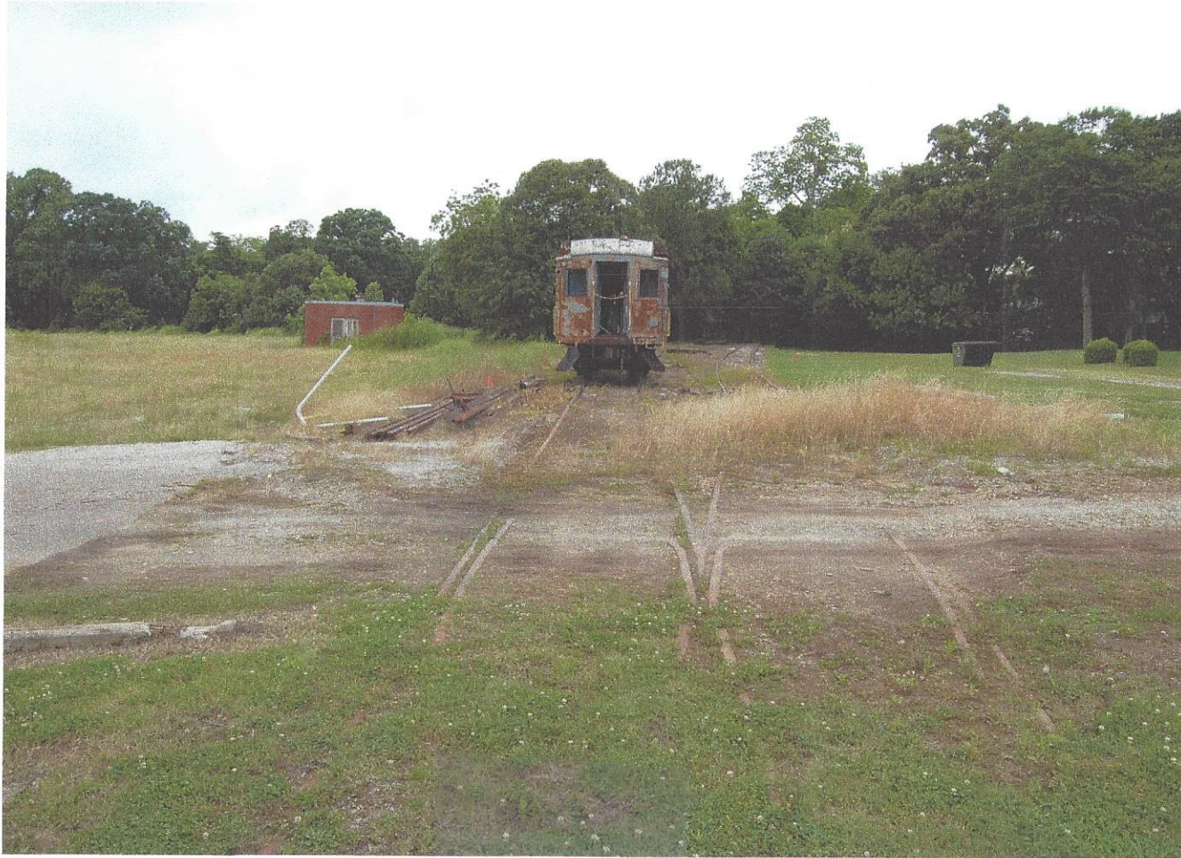
Photograph 11: GWRC Mainline and Turntable Spur at intersection of extension of Chandler Street Partially obscured by gravel temporarily placed by Hartwell First
