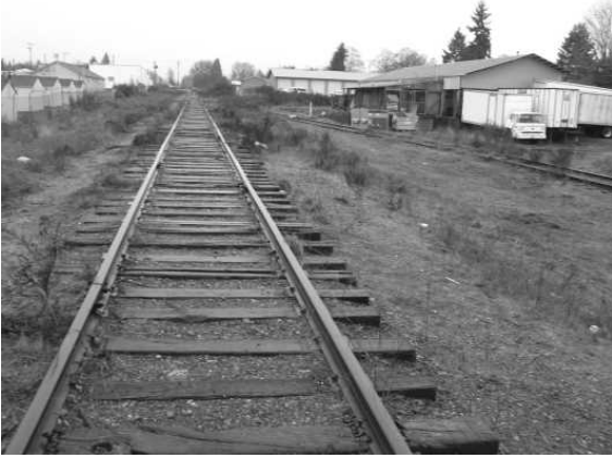
Mainline segment, view southwest
