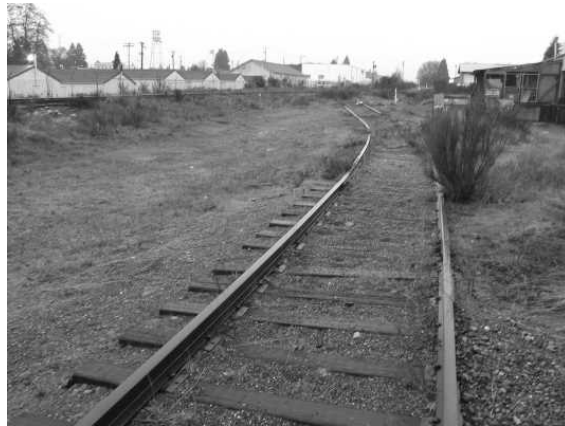
Siding track, view southwest
