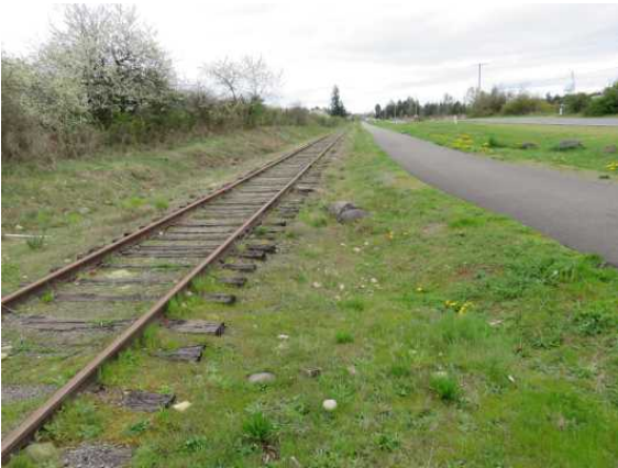
Northern Pacific Railway/Yelm Railroad
