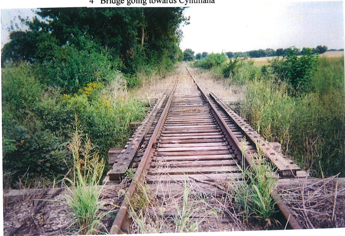
4 th Bridge going towards Cynthiana
