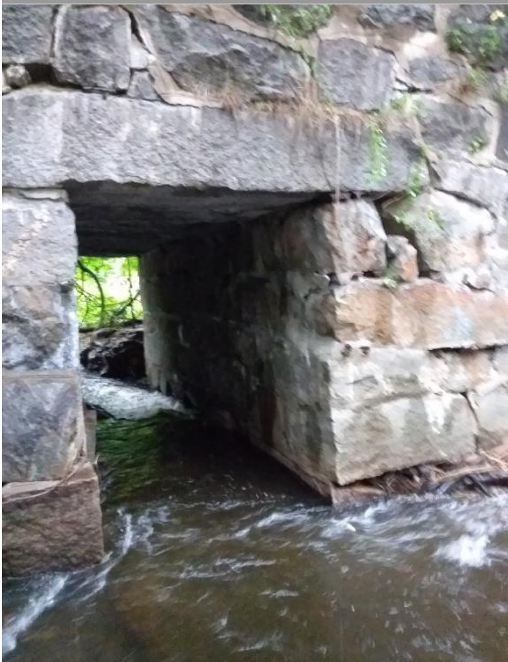
Bridge Structure at milepost QBU 4.52
