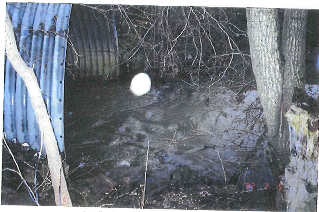
Ludington Ditch near Proposed Site
