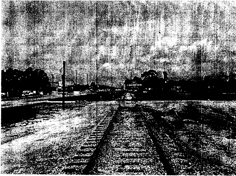
(3) FLORIDA POWER & LIGHT CROSSING LOOKING WEST
