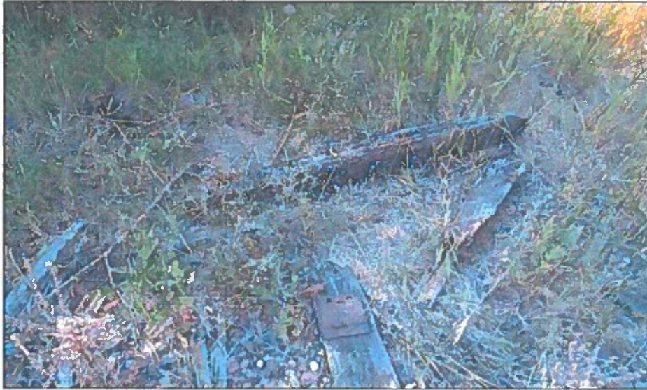
Figure 9. Broken railings and ties near south end, plan view.
