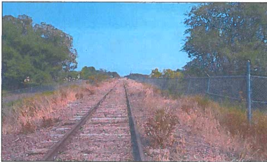
Figure 6. Northwest end of project area, view to the east.
