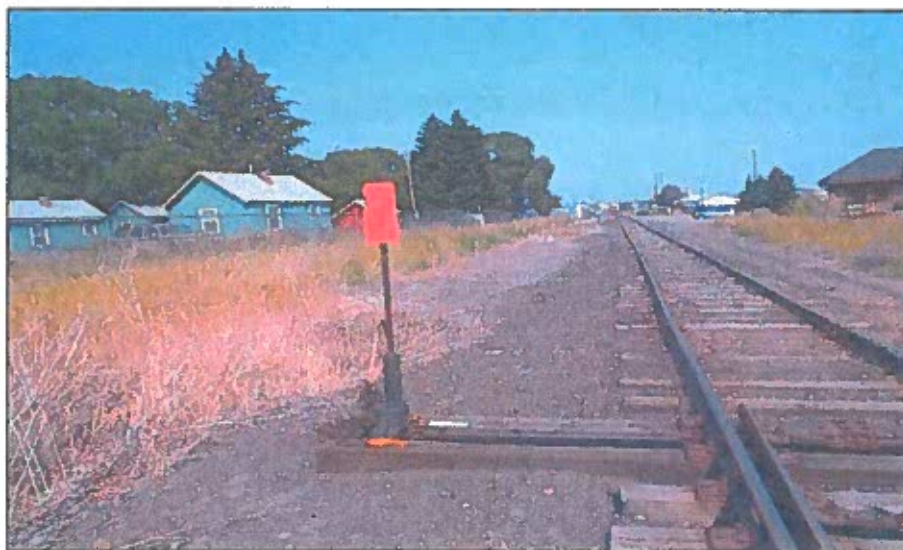
Figure 15. Railroad switch near northeast end of project area, view to the east/northeast.
