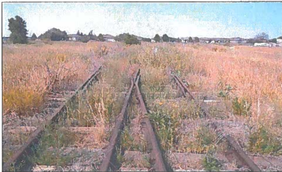
Figure 12. Southern junction, overgrown, view to the north.
