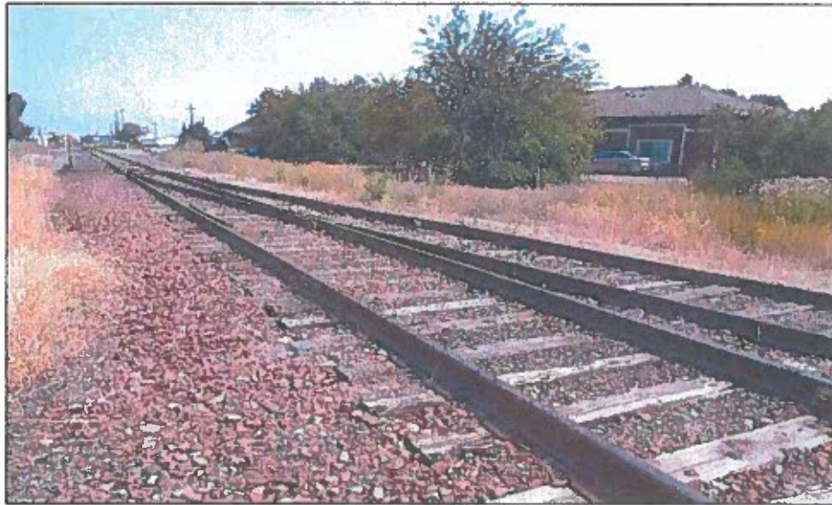
Figure 5. Northeast end junction of Kalispell-Somers spur line, view to the southeast.
