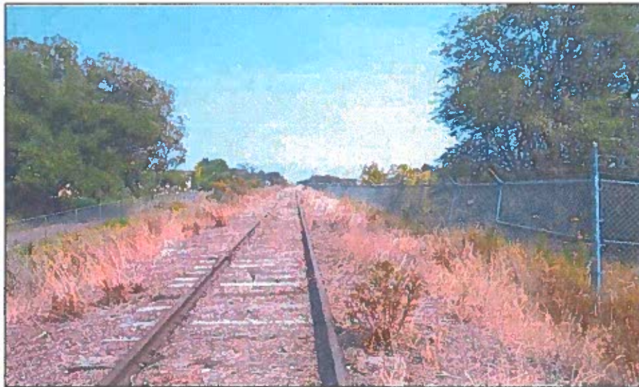
Figure 8. Northwest end of project area, view to the east.
