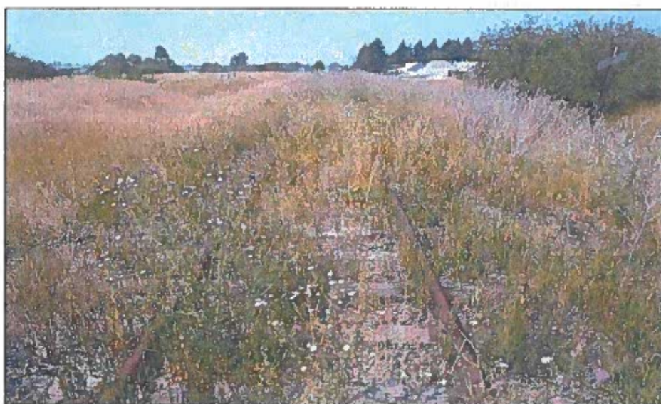
Figure 10. South end of project area, heavily overgrown, view to the north.
