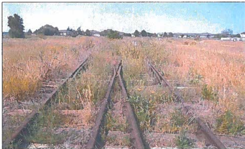
Figure 14. Southern junction, overgrown, view to the north.
