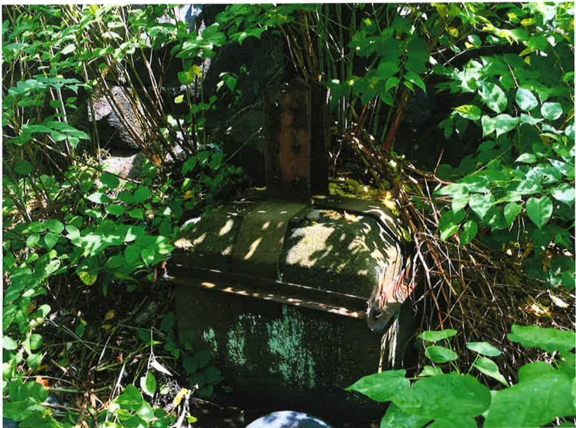
Photo 11. Catenary foundation block with cut-off, riveted iron beam on the north side.
