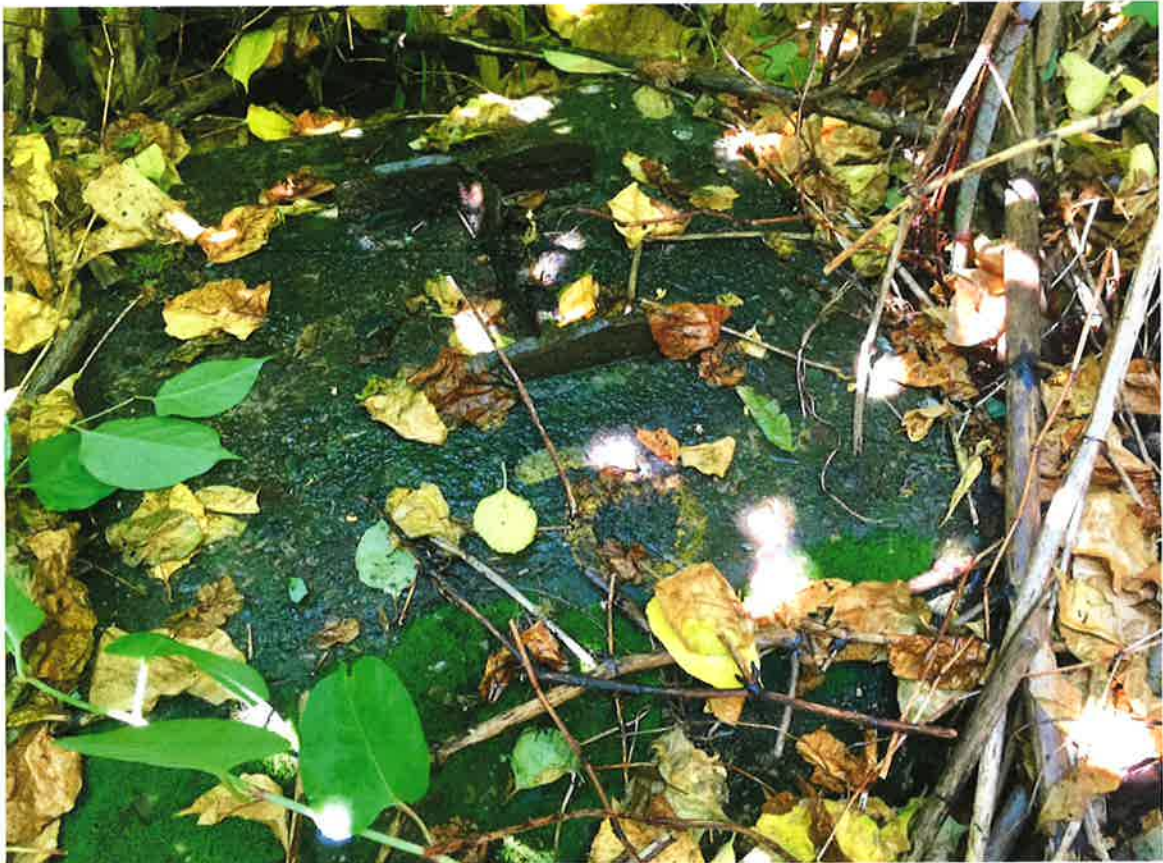
Photo 5. Third set of catenary pole foundation blocks. This one is on the south side.
