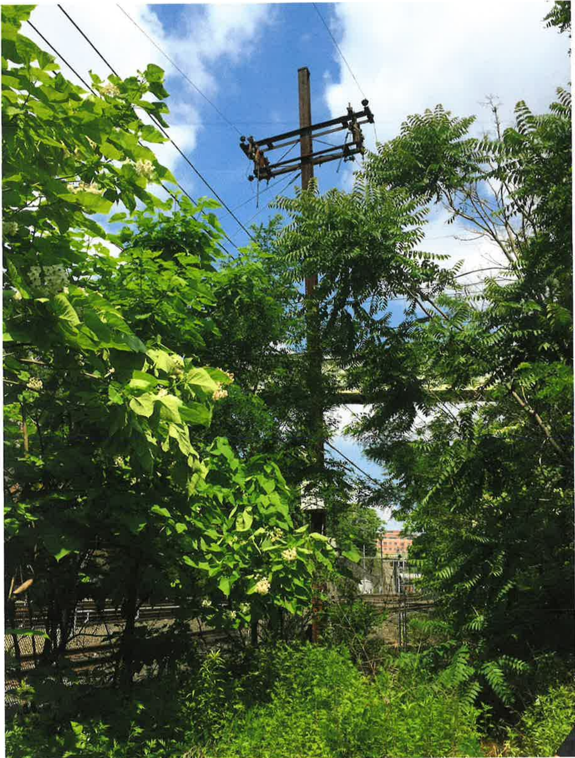
Photo 10. A complete catenary pole and foundation block at the western end of the Harsimus Branch.
