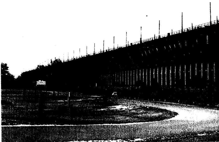
Ashland Ore Dock, west side, facing northeast
