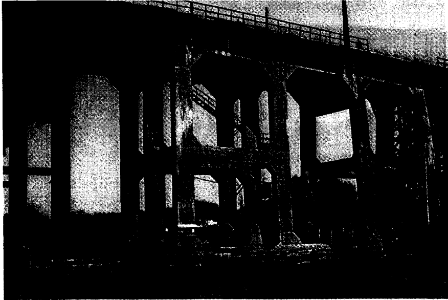
Ashland Ore Dock west side concrete trestles, detail
