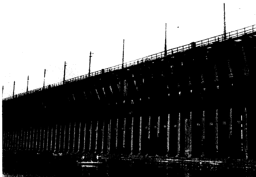
Ashland Ore Dock, west side, facing northeast
