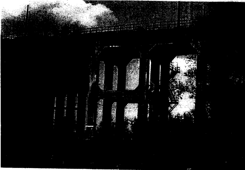
Ashland Ore Dock, concrete trestle, west side, facing east
