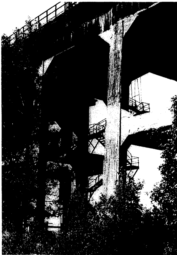
Ashland Ore Dock, concrete trestle detail, west side
