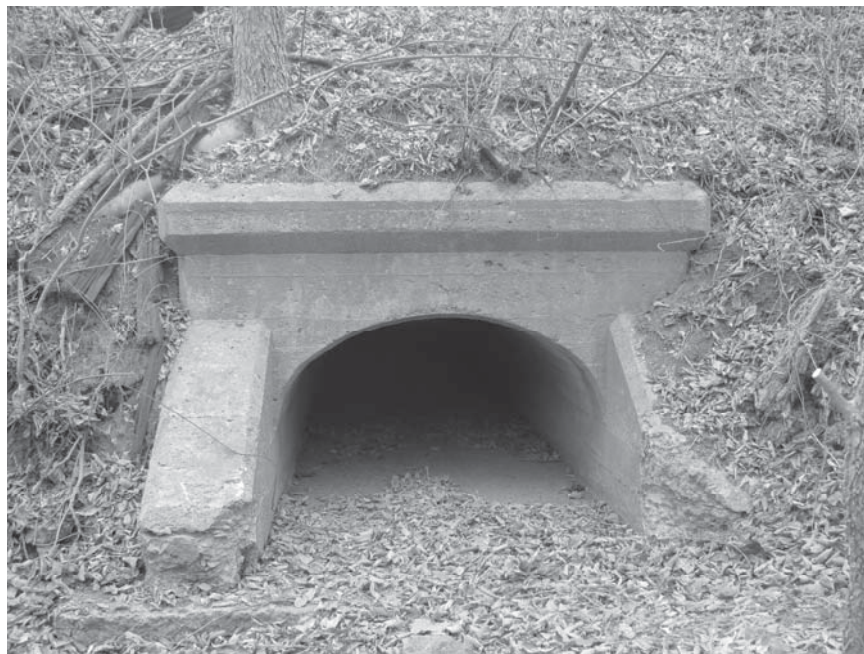
Photo 0033.jpg. North face of culvert #2047.
