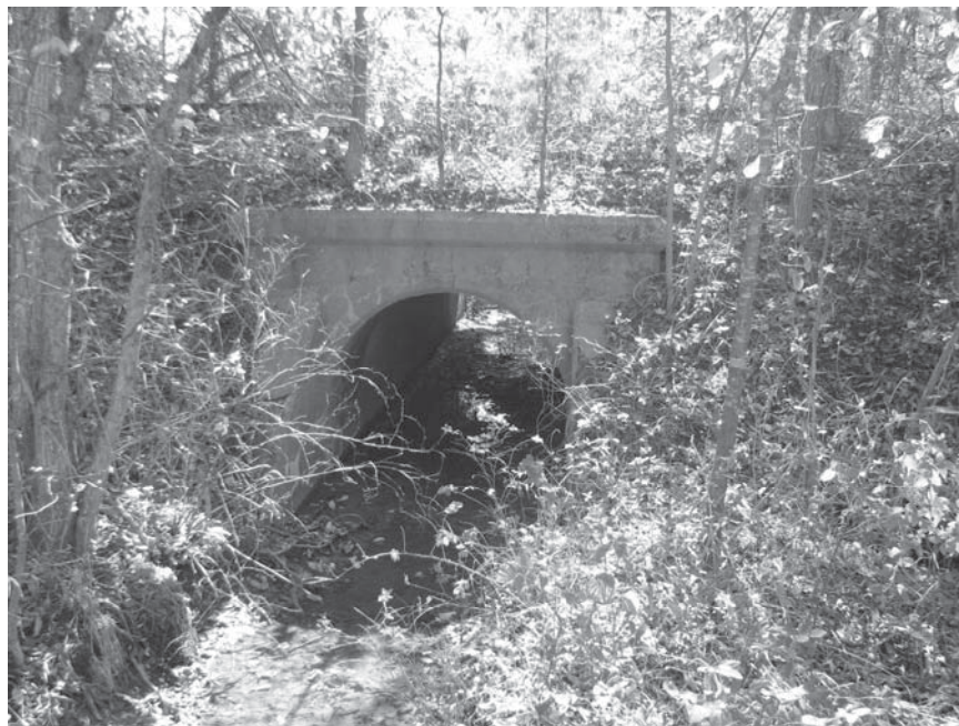
Photo 0075.jpg. North face of culvert #1013.
