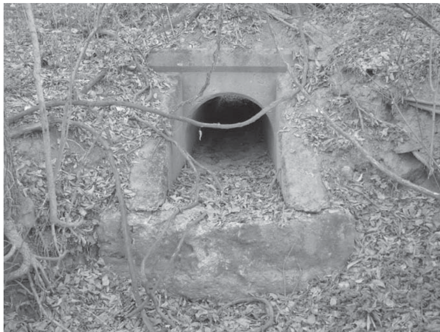
Photo 0058.jpg. North face of culvert #1104.
