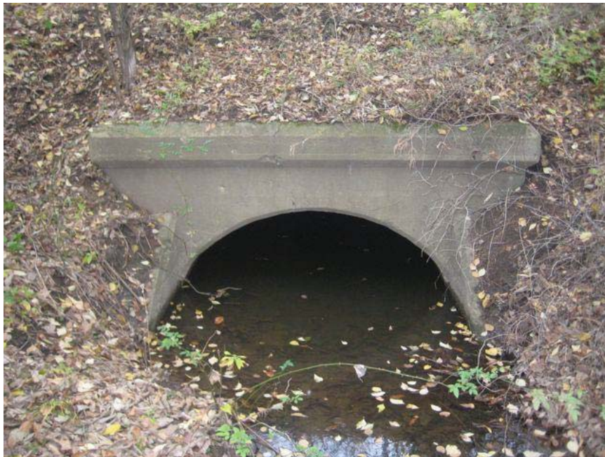
Looking upstream (north) at south end of culvert #1049.
