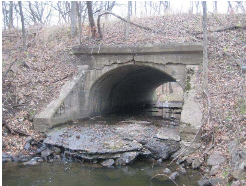
Looking upstream (north) at south end of culvert #1044.
