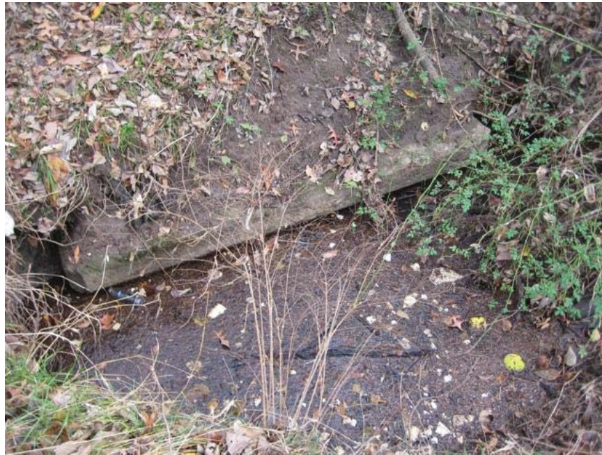
IMG_5374.jpg. South face of culvert #2090.
