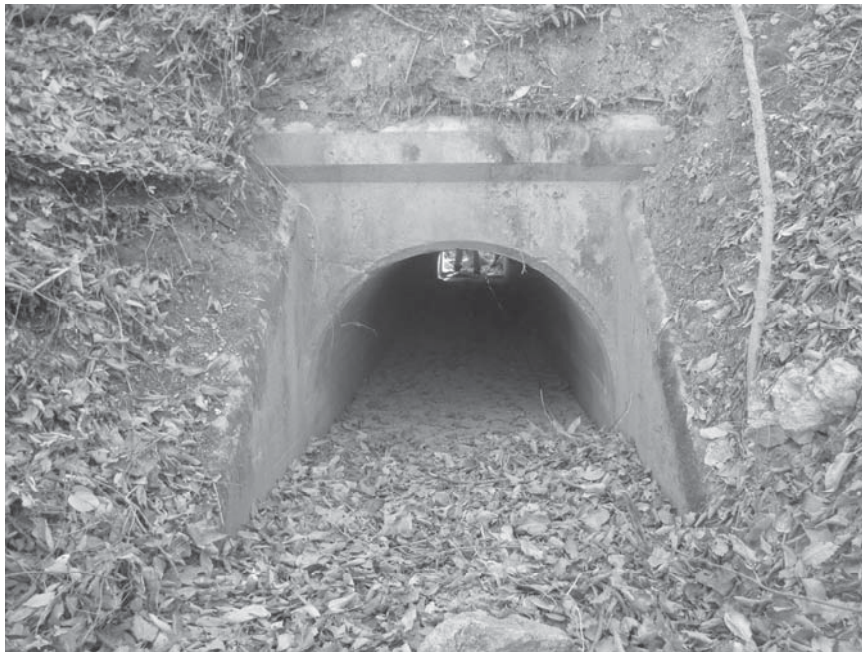
Photo 0044.jpg. North face of culvert #1150.
