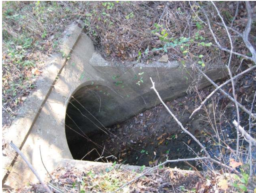
IMG_4373.jpg. South face of culvert #1013.
