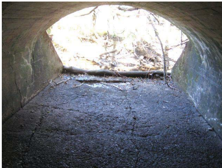
Looking upstream (north) from culvert #2032.
