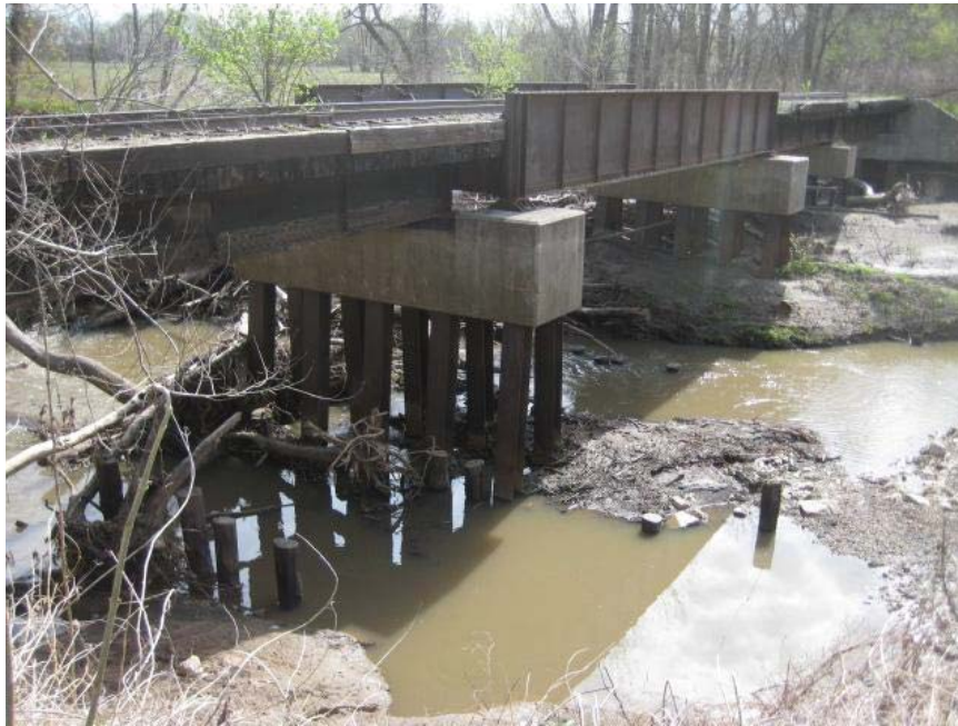
Looking east along south side of bridge across creek of bridge #3031.
