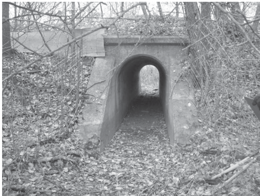
Photo 0042.jpg. North face of culvert #2003.
