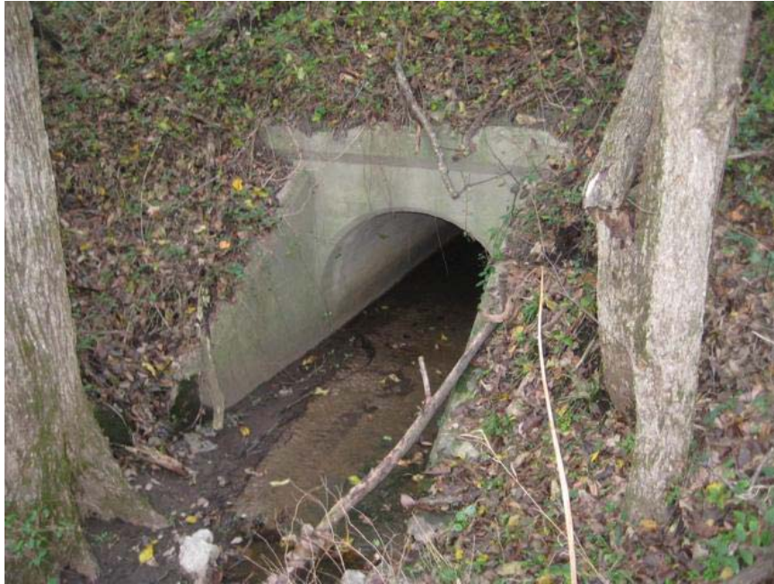
IMG_4821.jpg. South face of culvert #1150.
