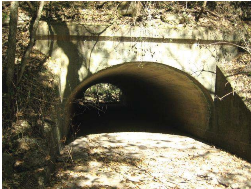
Looking upstream (north) through culvert #2032.
