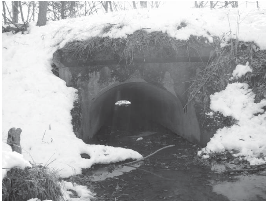
Culv 1Photo 030. Culvert #970.
