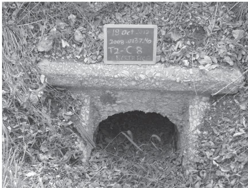
Photo 0017.jpg. North face of culvert #2132.
