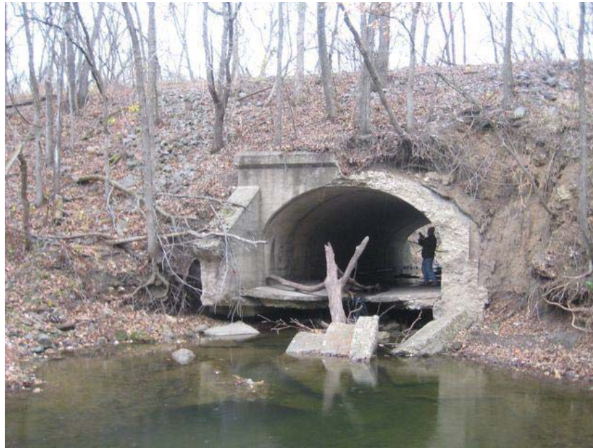
Looking upstream (north) at south end of culvert #1046.
