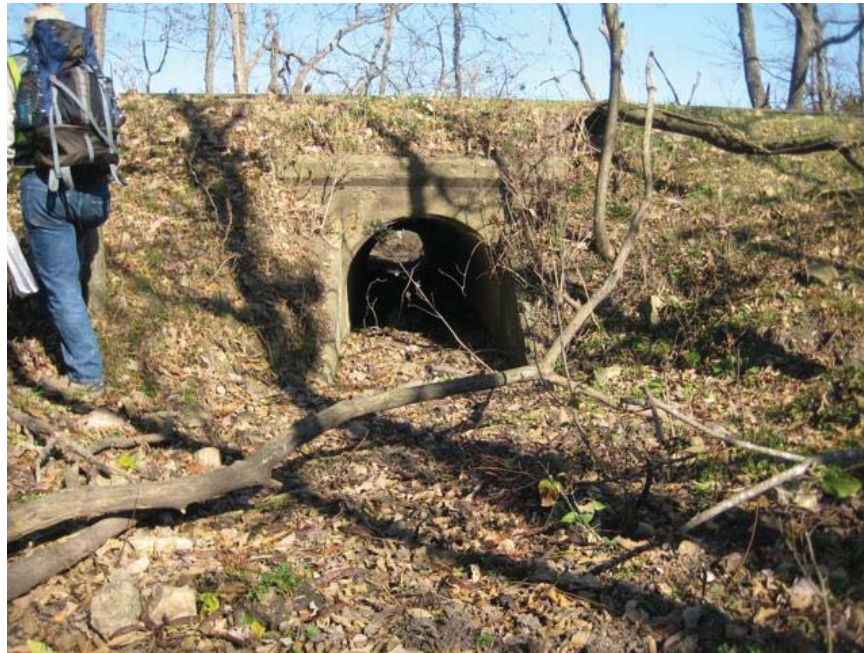
IMG_4535.jpg. South face of culvert #1060.
