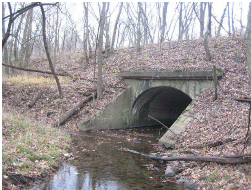
Looking downstream (southeast) at north end of culvert #1044.
