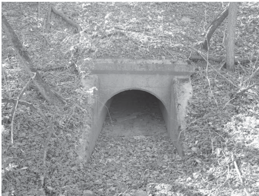
Photo 0047.jpg. North face of culvert #1144.
