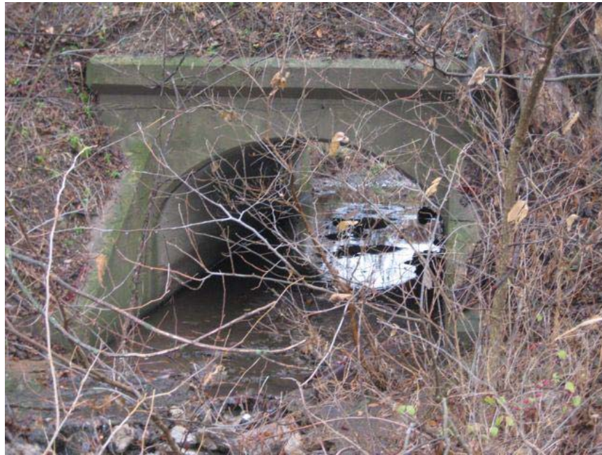
Looking upstream (north) at south end of culvert #2014.
