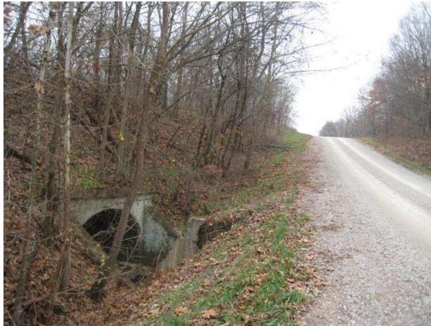
Looking west along County Road at adjacent culvert #1053.
