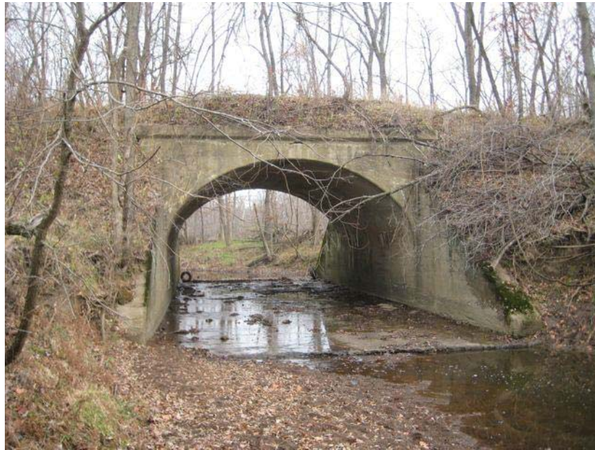
Looking upstream (north) at south end of culvert #1025.
