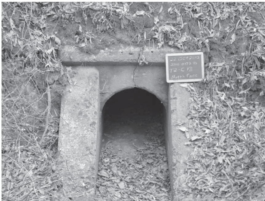
Photo 0022.jpg. North face of culvert #2113.
