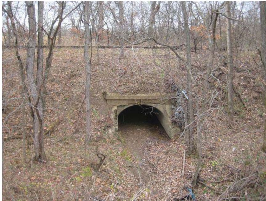
Looking upstream (north) at south end of culvert #1065.
