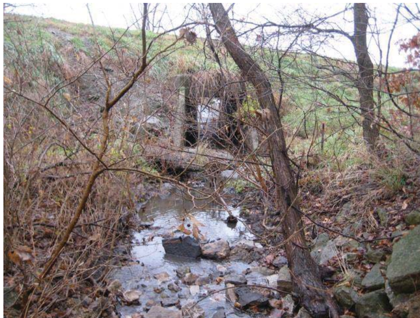
Looking downstream (south) of culvert #2014 towards downstream concrete box culvert under adjacent road embankment.
