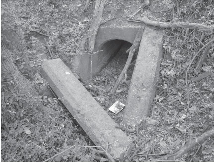
C 2095.jpg. Culvert #2095.
