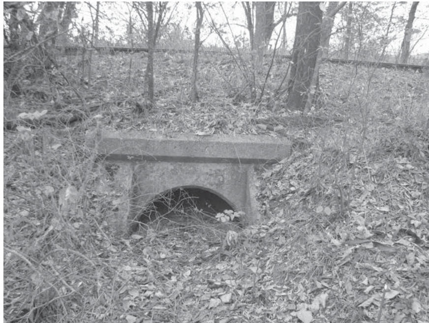
Photo 0063 C18 068.jpg. Culvert #1074.
