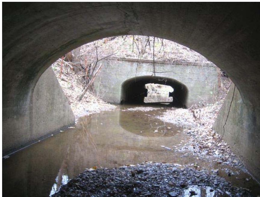
Looking north through culvert #1099 downstream.
