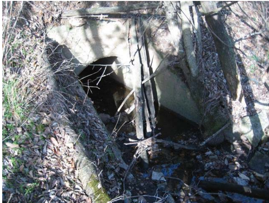
IMG_4804.jpg. South face of culvert #1145.
