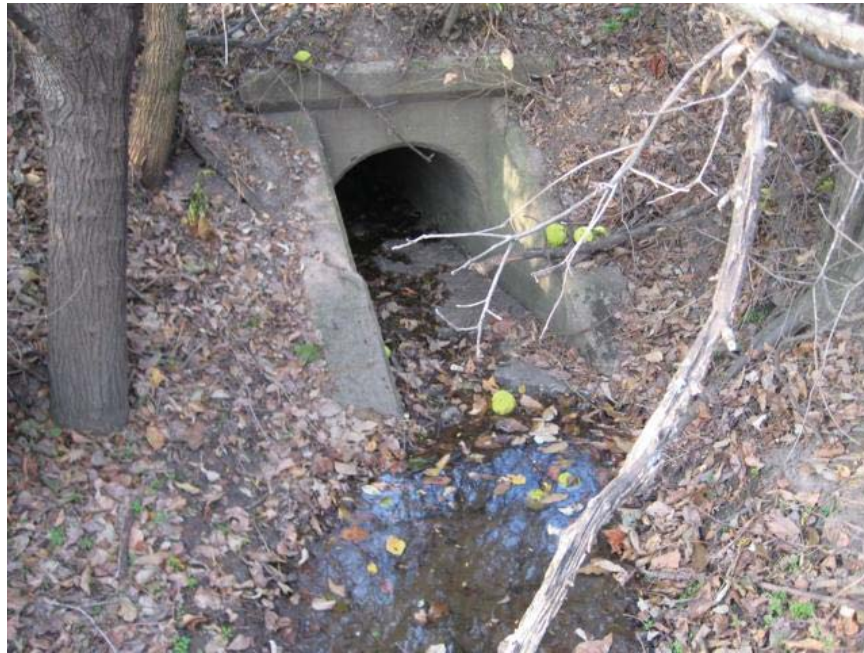
IMG_4672.jpg. South face of culvert #1104.
