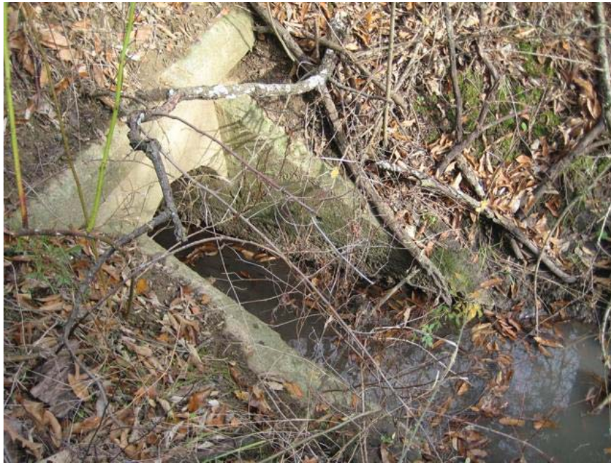
IMG_5510.jpg. South face of culvert #2113.
