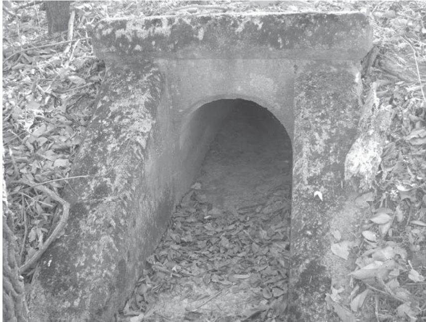
Photo 0055 C51 T2 1133.jpg. Culvert #1117.
