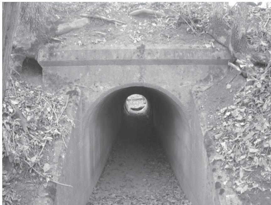
C 1162.jpg. North face of culvert #1162.
