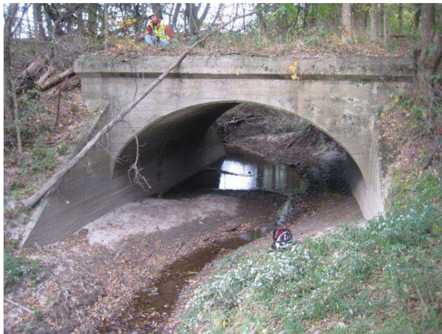
Looking upstream (north) at south culvert face of culvert #3000.
