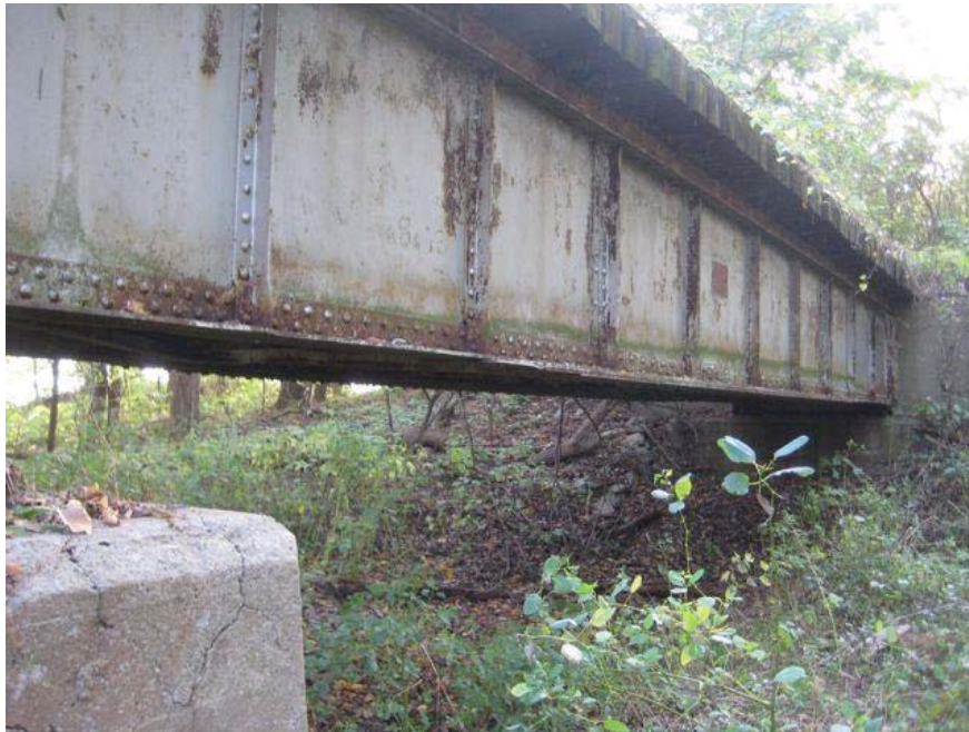
Looking northeast along south side of east span of bridge #3021.
