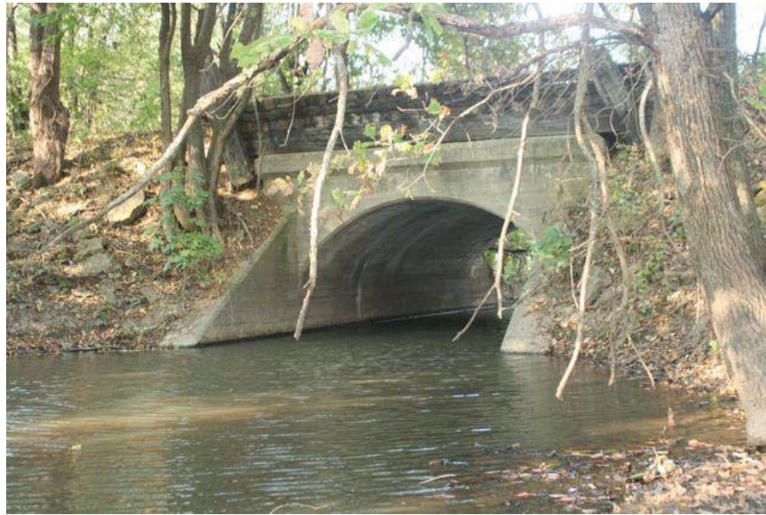
Looking upstream (north) at south culvert face of culvert #3016.
