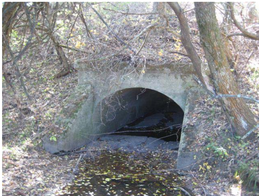
Looking downstream (south) at north end of culvert #2029.
