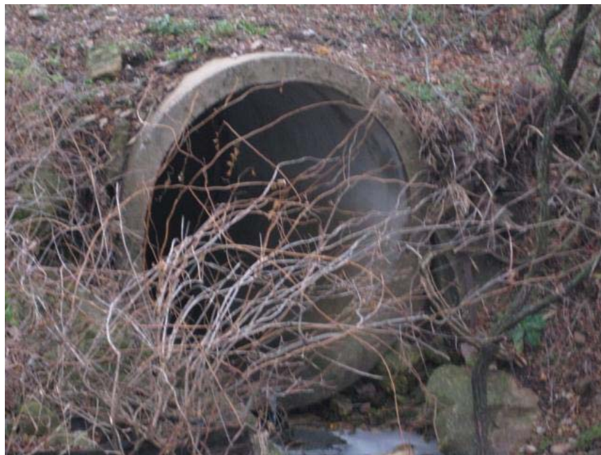
Picture 645.jpg. Culvert #2021.
