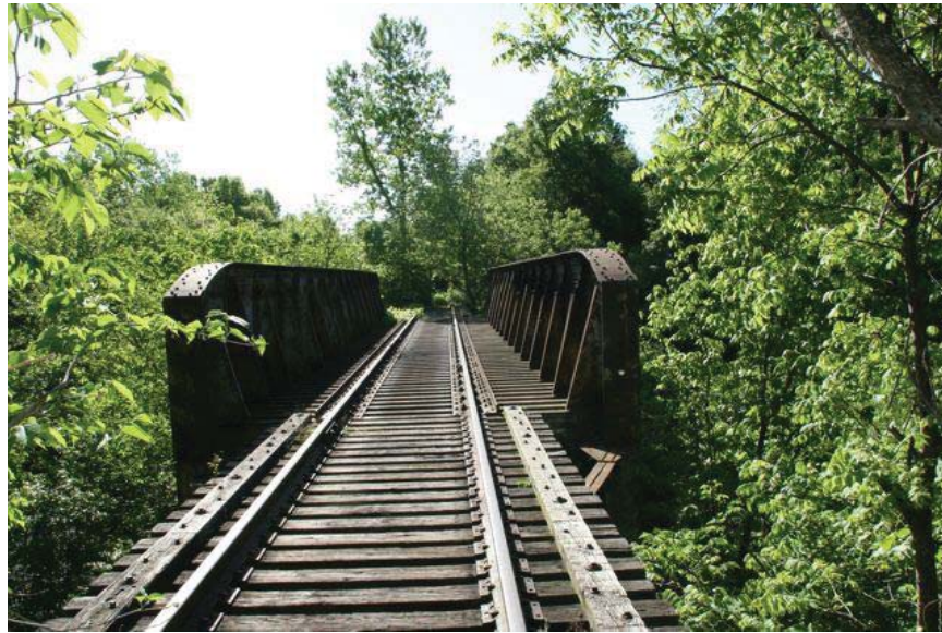
Looking east across bridge #2141 at center through-girder span of three-span bridge.
