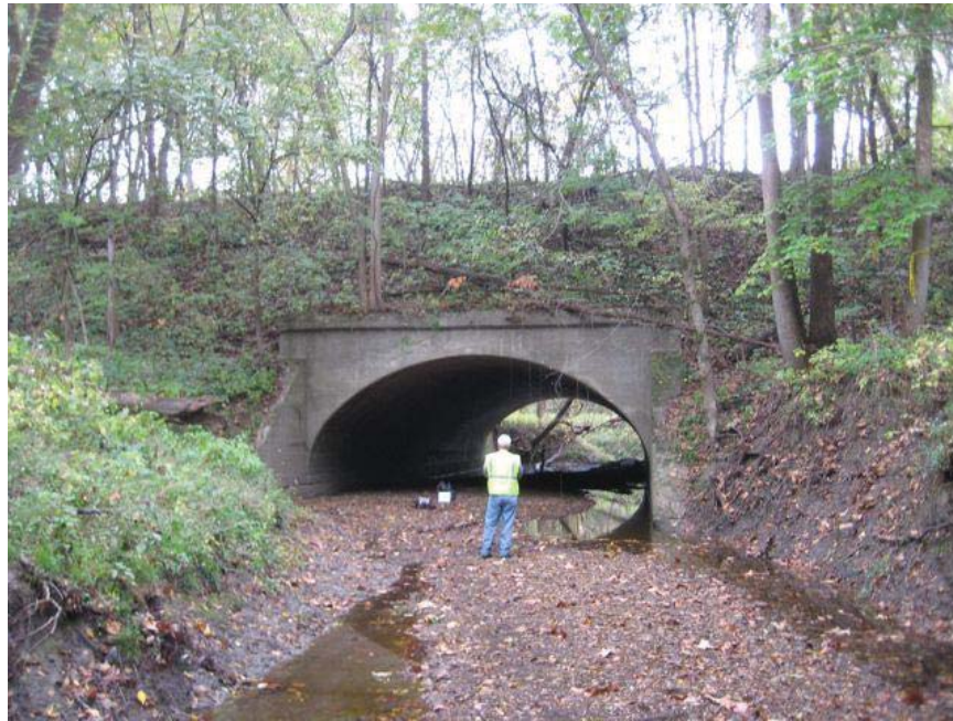
Looking upstream (north) at south end of culvert #2055.
