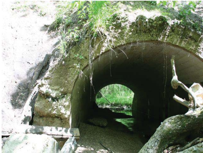
Looking upstream (north) of culvert #1057.
