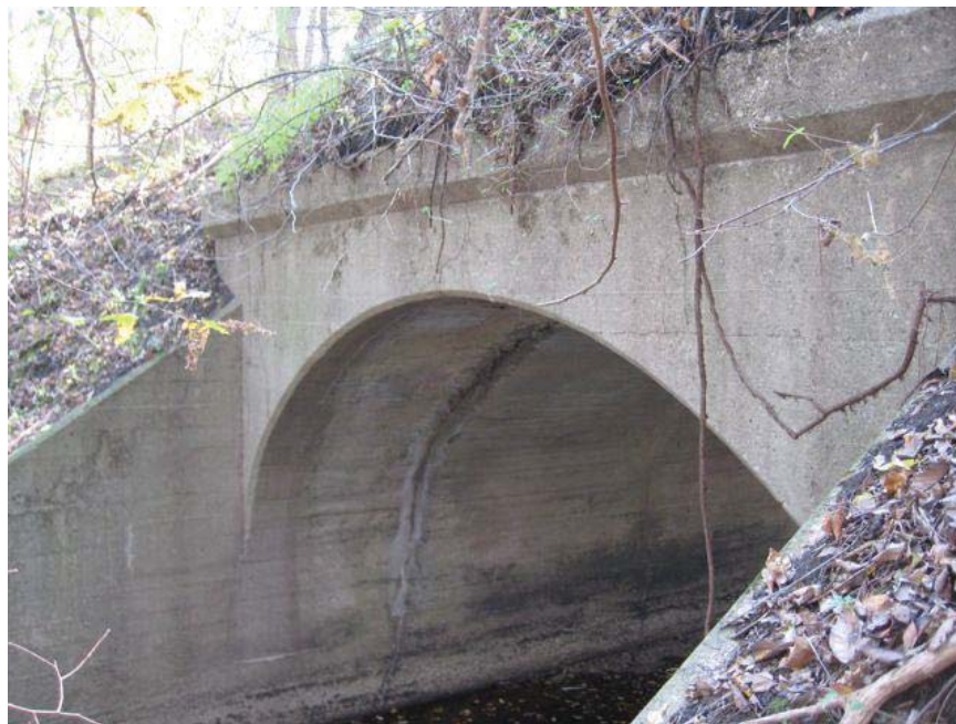
Looking southeast at north headwall of culvert #2122.
