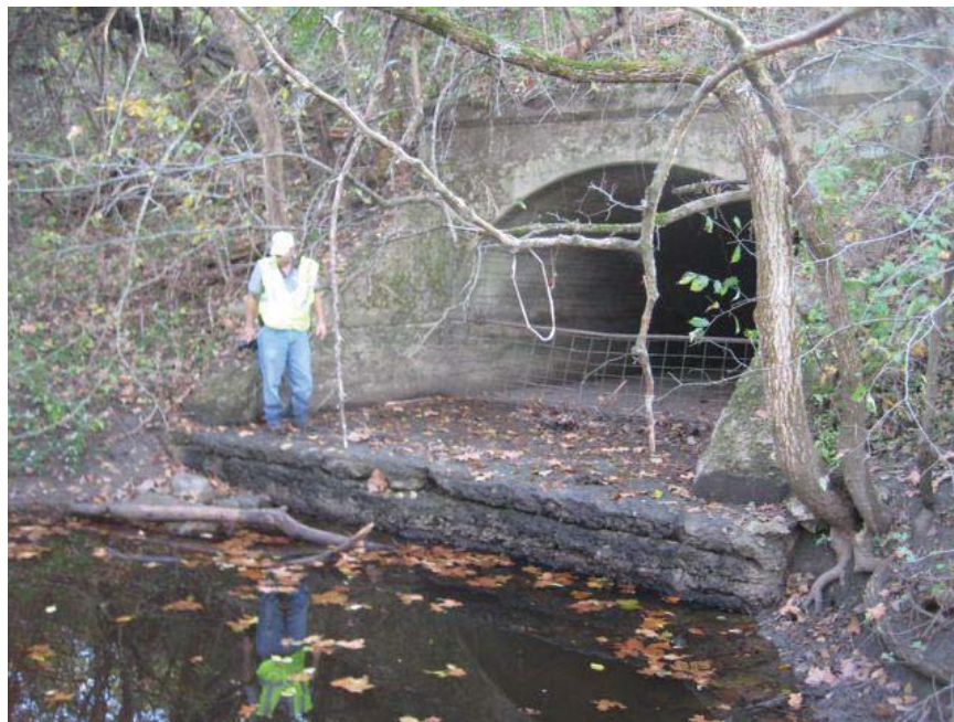
Looking northwest (upstream) towards culvert #2070.
