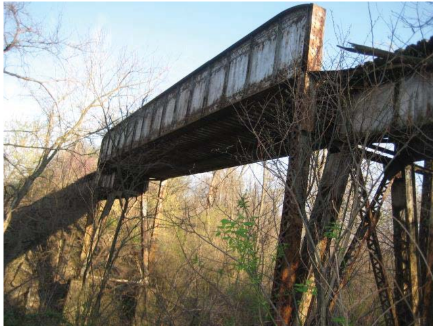
Looking southeast at bridge with center through-girder and plate girder of bridge #2141.
