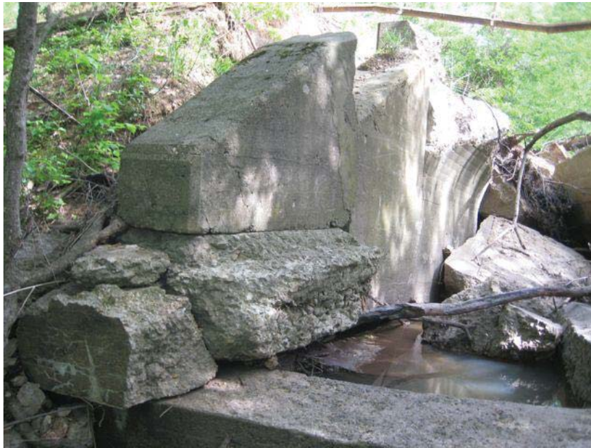
Looking north at culvert #2018.
