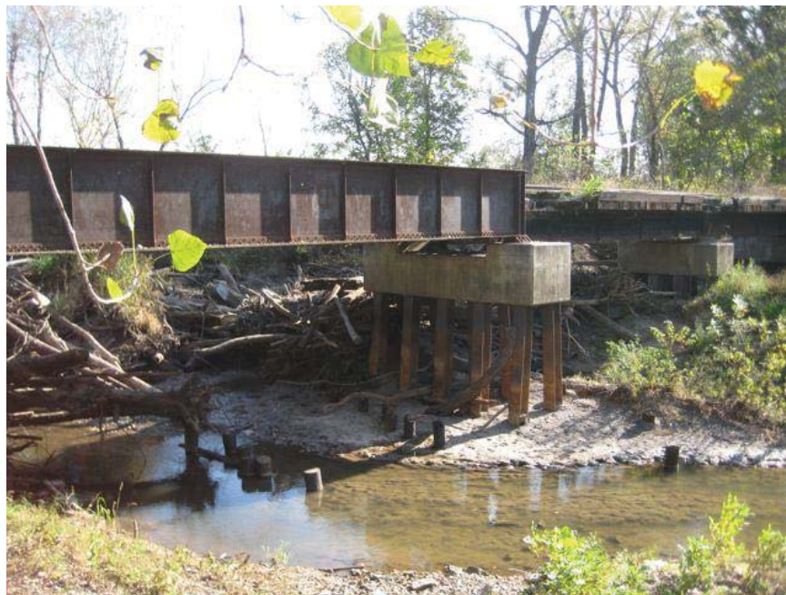
Looking northeast at center spans of bridge #3031.
