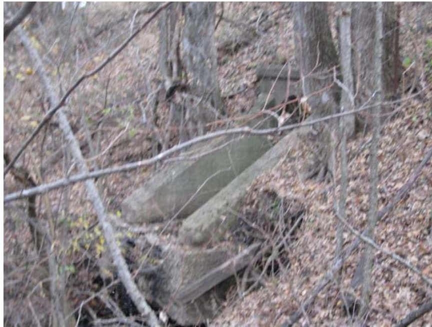
IMG_5498.jpg. South face of culvert #2111.
