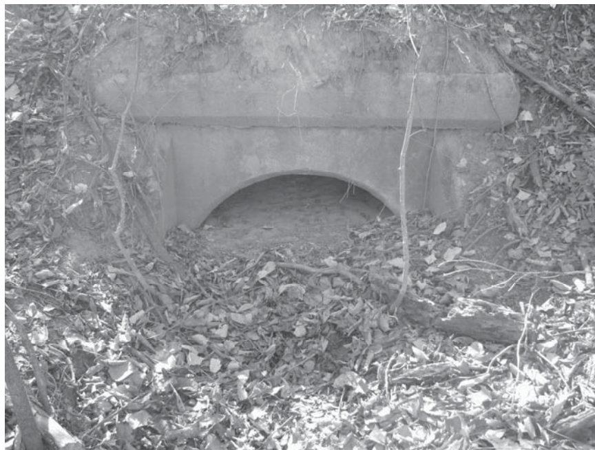
Photo 0054.jpg. North face of culvert #1126.
