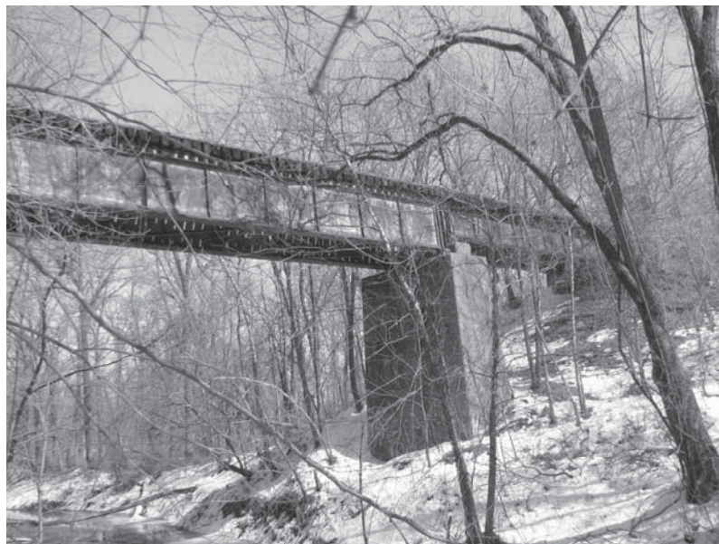
Looking along north face of bridge #960.
