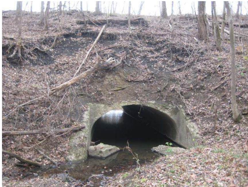
Looking downstream (south) at north end of culvert #1069.
