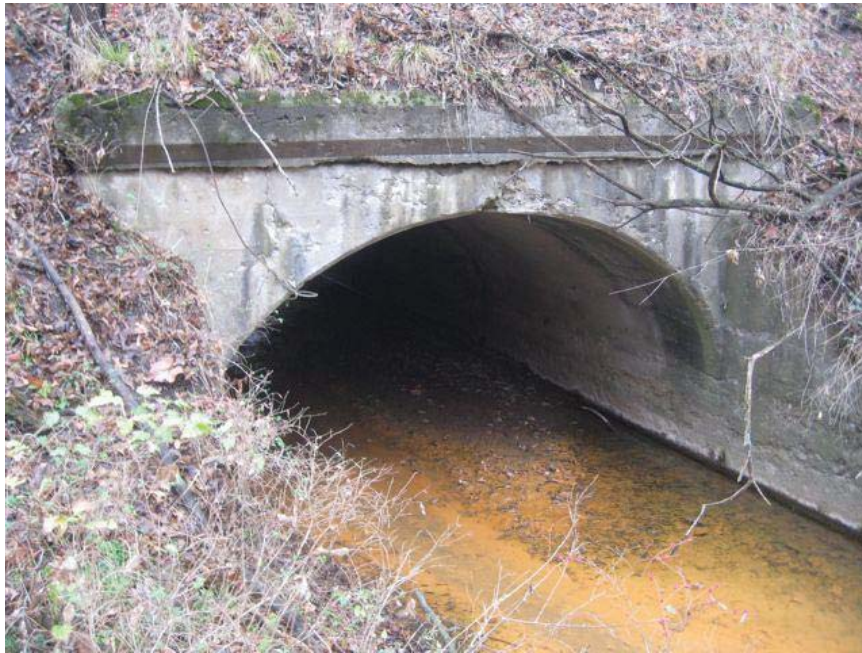
Looking upstream (north) at south end of culvert #1038.
