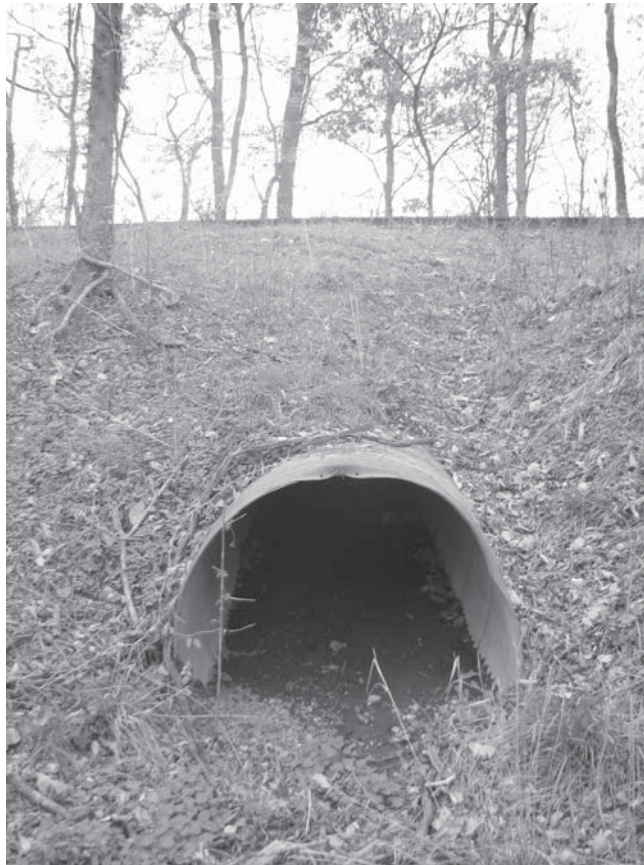
C 1060.jpg. North face of culvert #1060.
