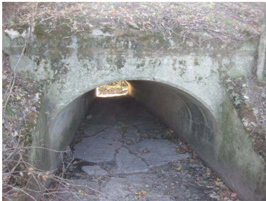
Looking downstream (south) at north end of culvert #2023.
