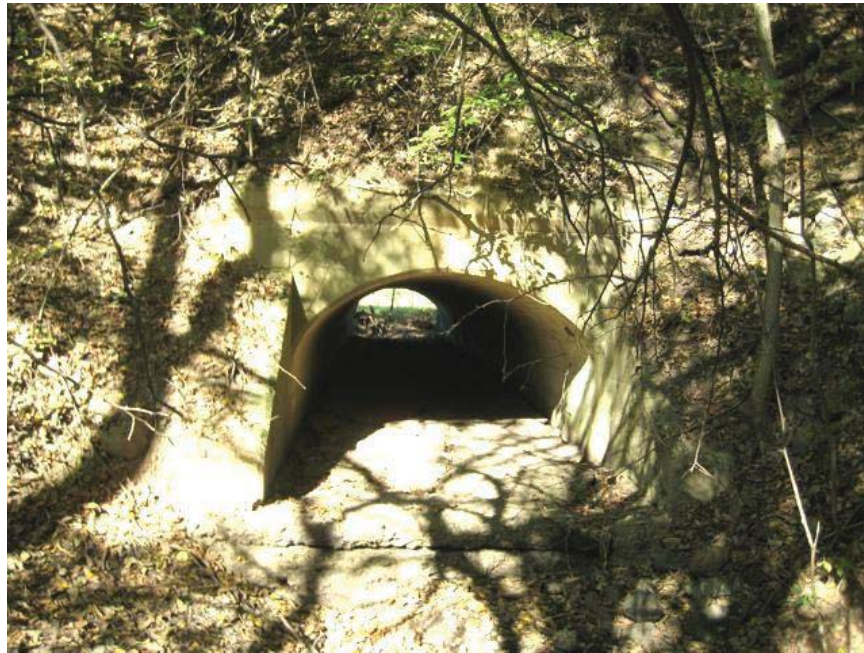
Looking north at south end of culvert #2023.
