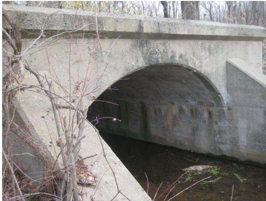
Looking downstream (northeast) at south end of culvert #1138.
