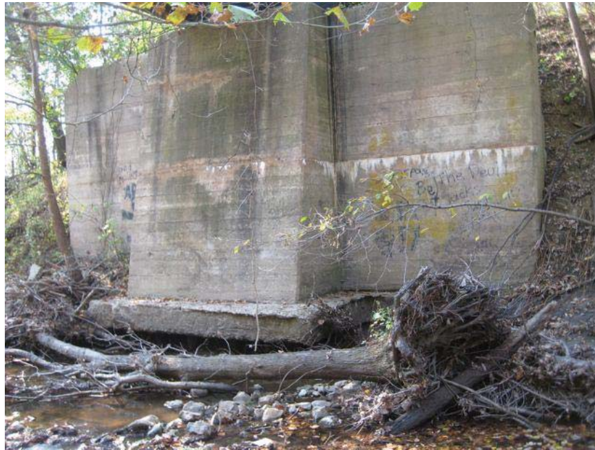
Looking southwest at west intermediate pier of bridge #2152.
