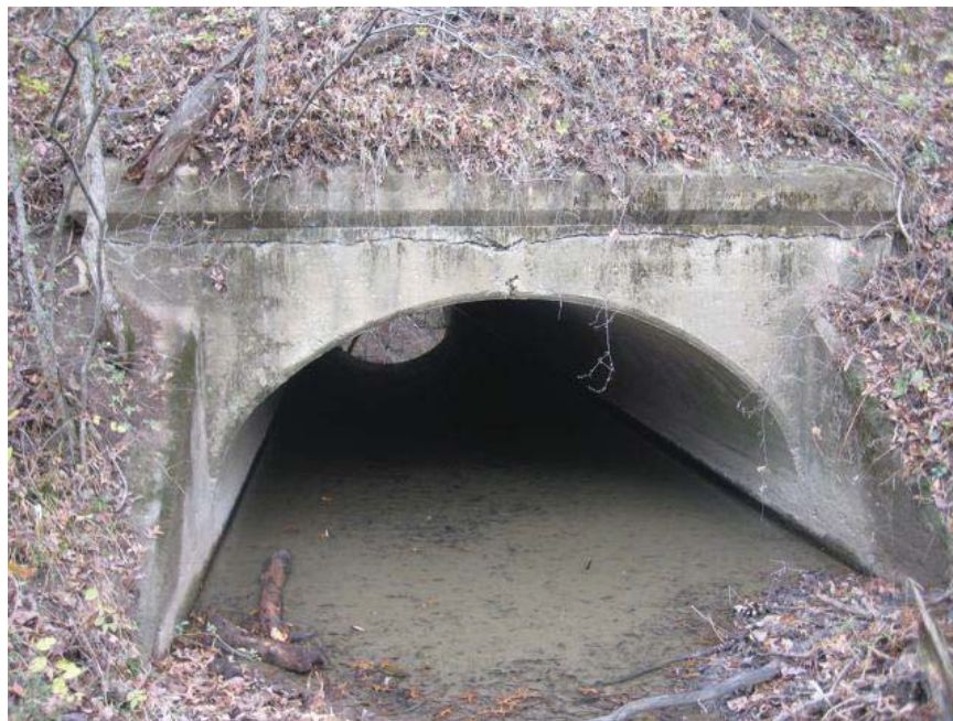
Looking upstream (north) at south end of culvert #1028.
