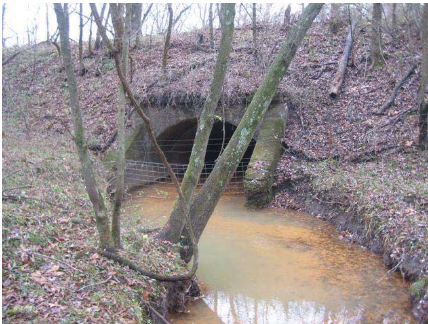
Looking upstream (north) at north end of culvert #1038.
