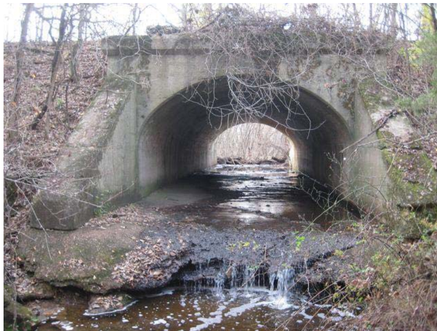
Looking upstream (south) at north end of culvert #1138.
