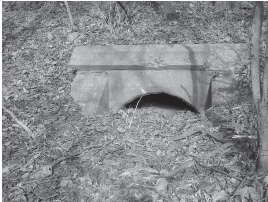
Photo 0048 C45 T2 954.jpg. Culvert #1139.
