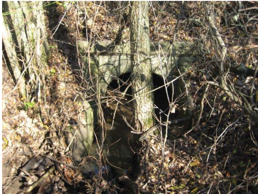
IMG_4741.jpg. South face of culvert #1126.
