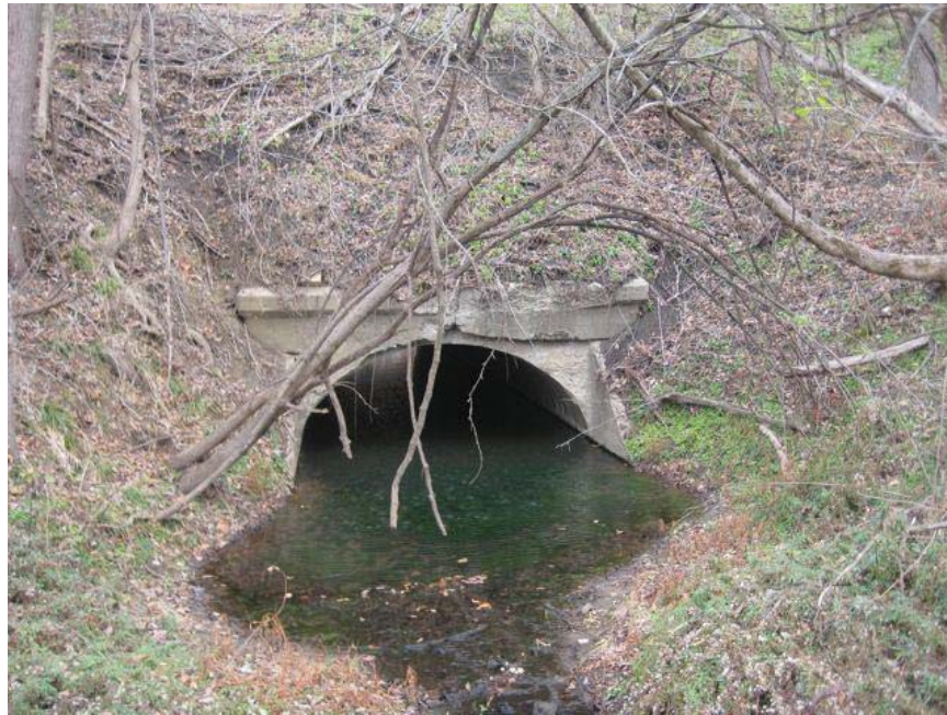
Looking upstream (north) at south end of culvert #1069.
