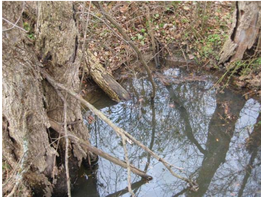
IMG_5606.jpg. South face of culvert #2132.
