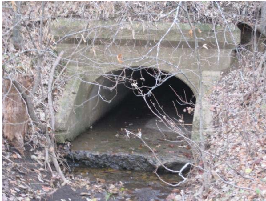
IMG_5139.jpg. South face of culvert #2047.
