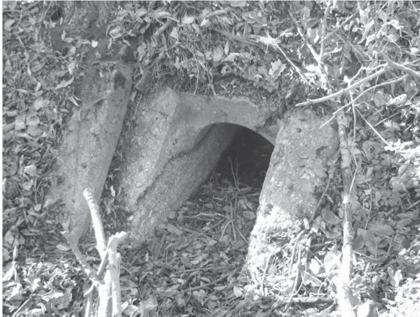
C 1047.jpg. Culvert #1047.
