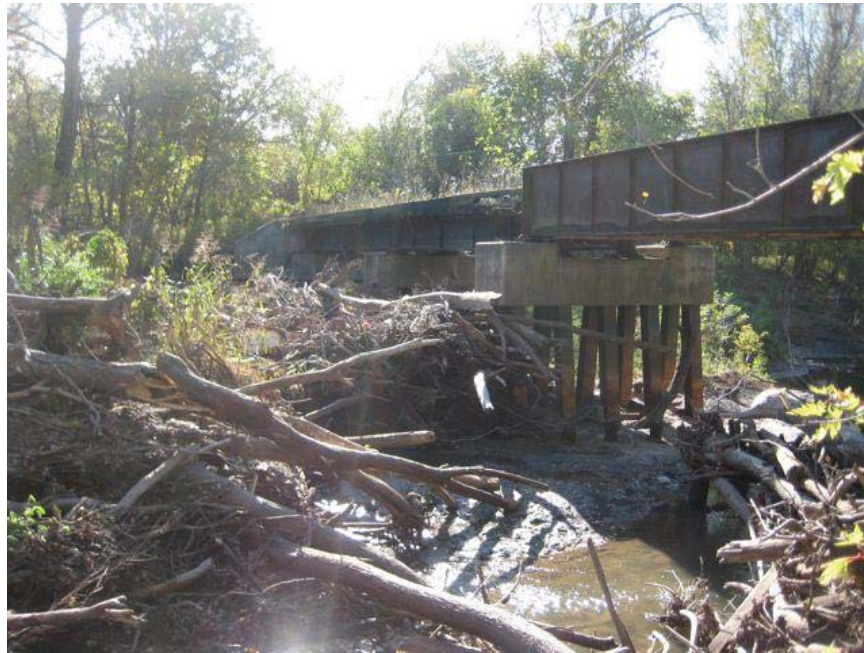
Looking southwest at center bridge spans of bridge #3031.
