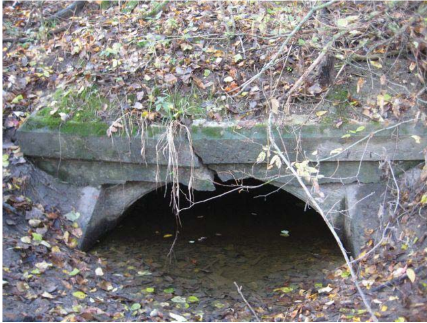
Looking at downstream (north) end of culvert #2086.
