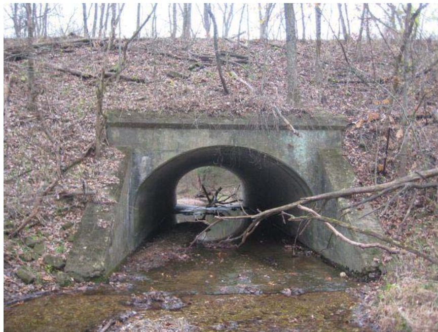
Looking downstream (south) at north end of culvert #1046.
