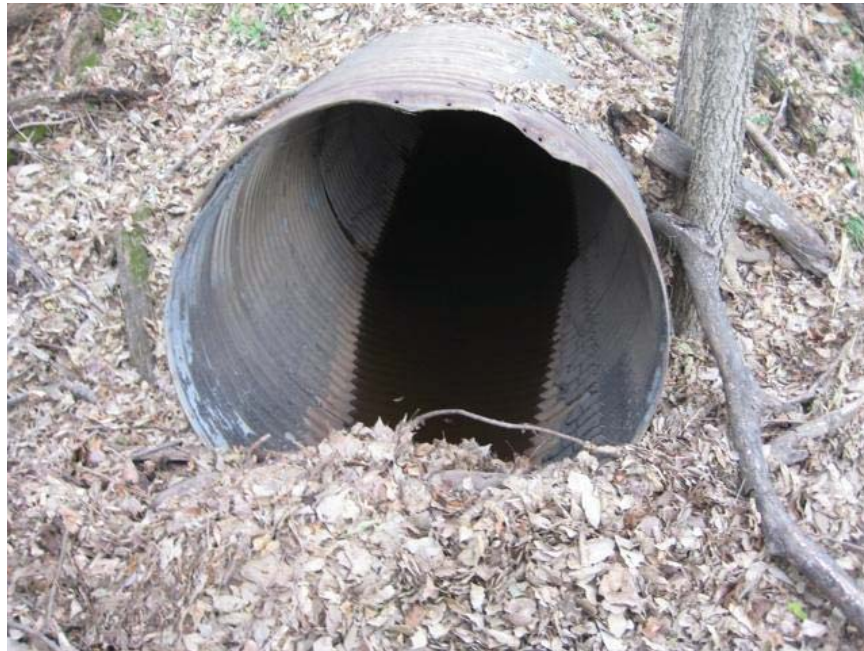
IMG_4855.jpg. South face of culvert #1162.
