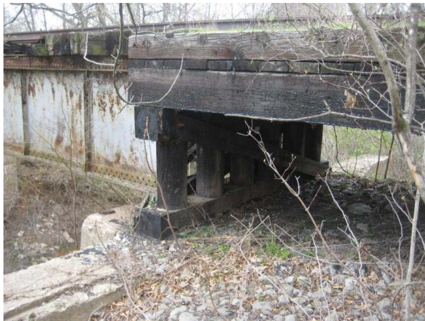
Looking northwest at east end timber span and east end of steel girder center span of bridge #2152.
