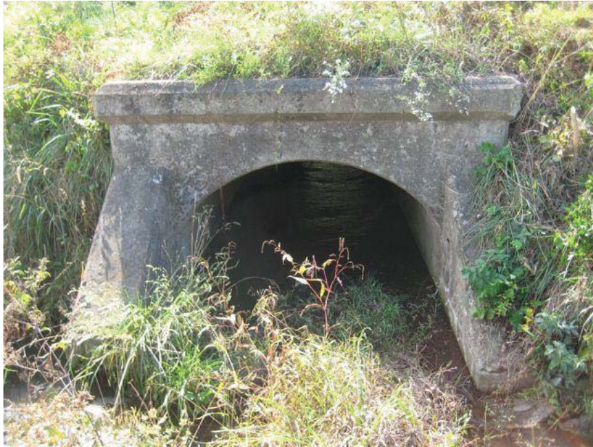
Looking downstream (south) at culvert #2042.
