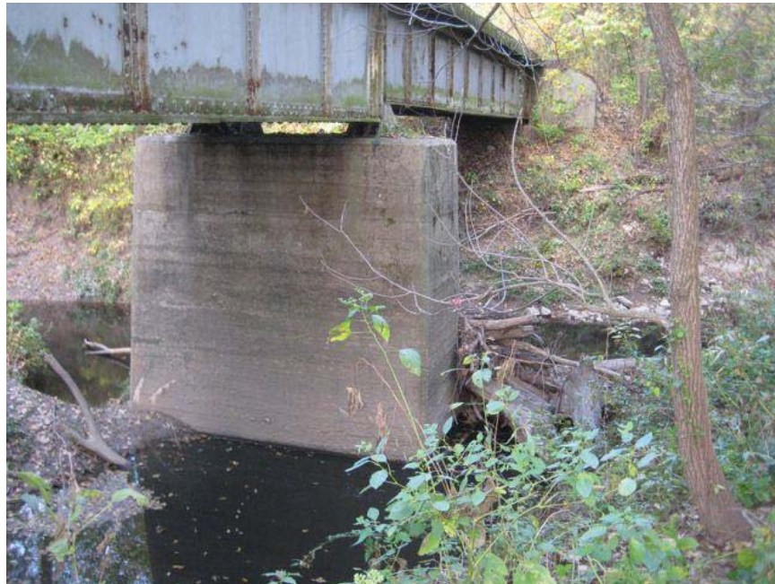
Looking southwest at taller west intermediate pier of bridge #3021. Note most of normal stream flow through west end span.
