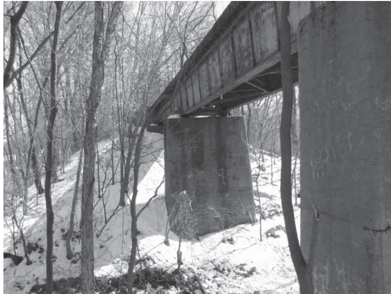
Looking along south face of bridge #960.
