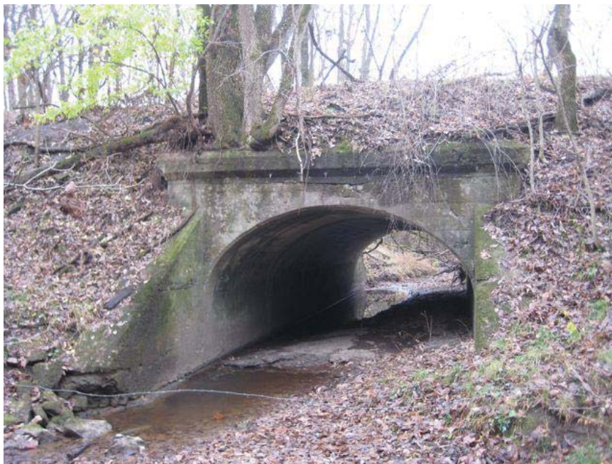
Looking downstream (south) at north end of culvert #1033.
