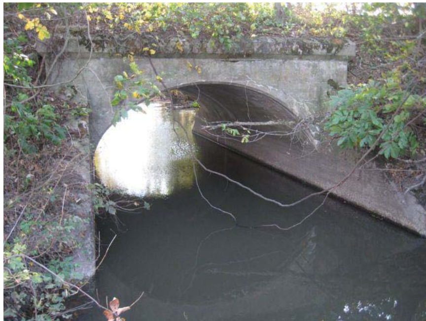
Looking downstream (south) at north culvert face of culvert #3016.
