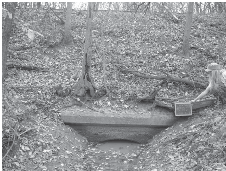
Photo 0026.jpg. North face of culvert #2090.
