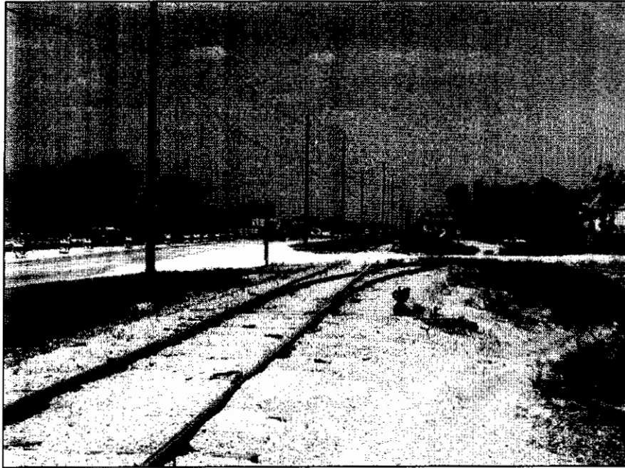
Schwab Redi-Mix Concrete Plant Switch (Looking East)
