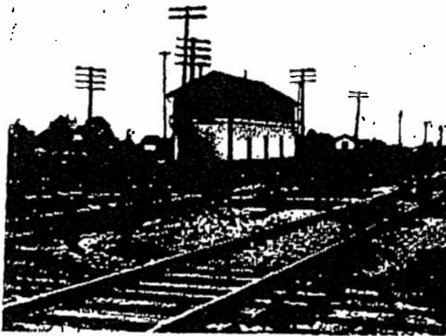
Riverdale Tower, Circa 1915. This tower which controlled the IC, PRR, B&OCT crossing was no longer of use to the IC after elevation. However the structure continued to control the crossing of the PRR and B&OCT and be manned by an IC leverman. Courtesy the Smoke Abatement and Electrification of Railway Terminals in Chicago, 1915
