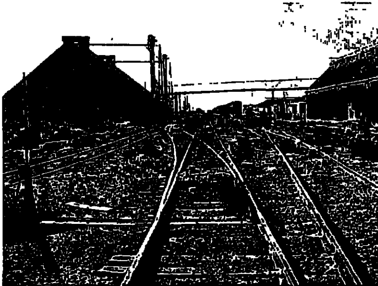
July 23, 2007 West End SAW Yard TEAM No 9298 (SAW Main Line) at West Switch Yard Track 5
