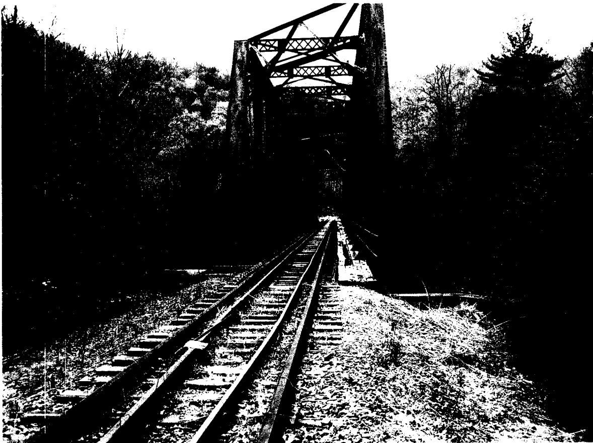
Bridge No. MP 57.81 South
