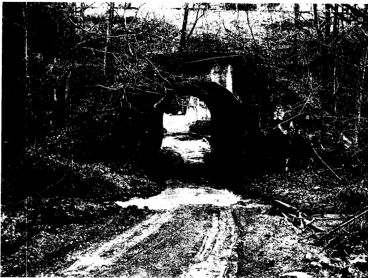
Arch 15' MP 43.59 West
