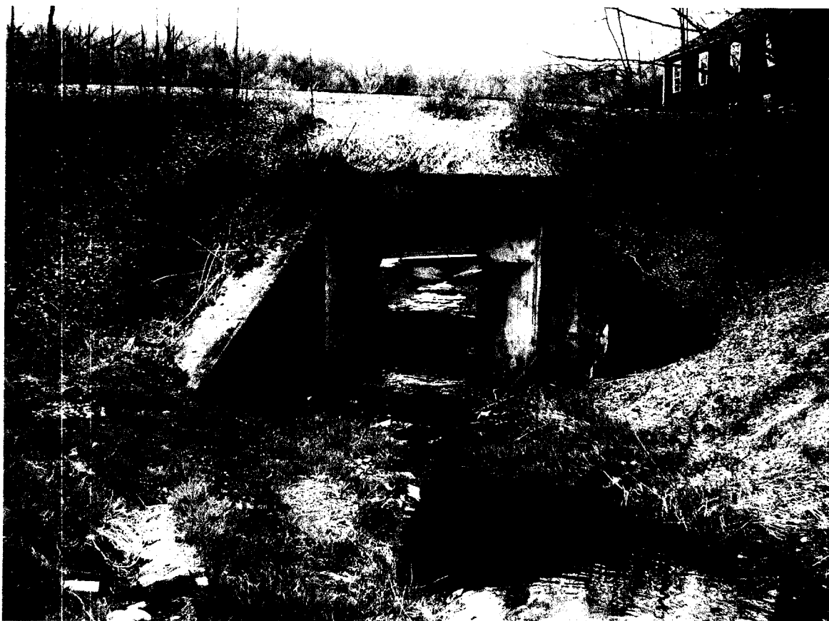
Arch 15' MP 44.57 West
