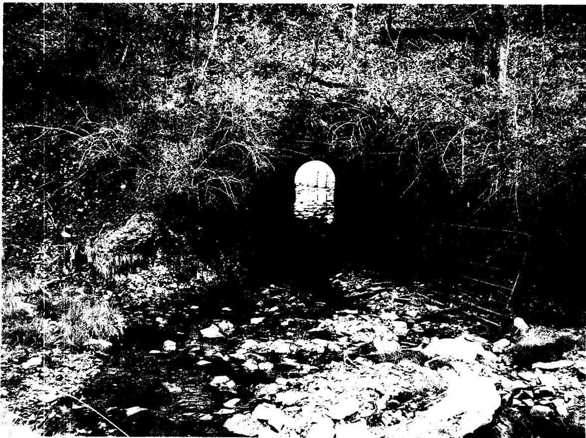
Arch 8' MP 43.16 West
