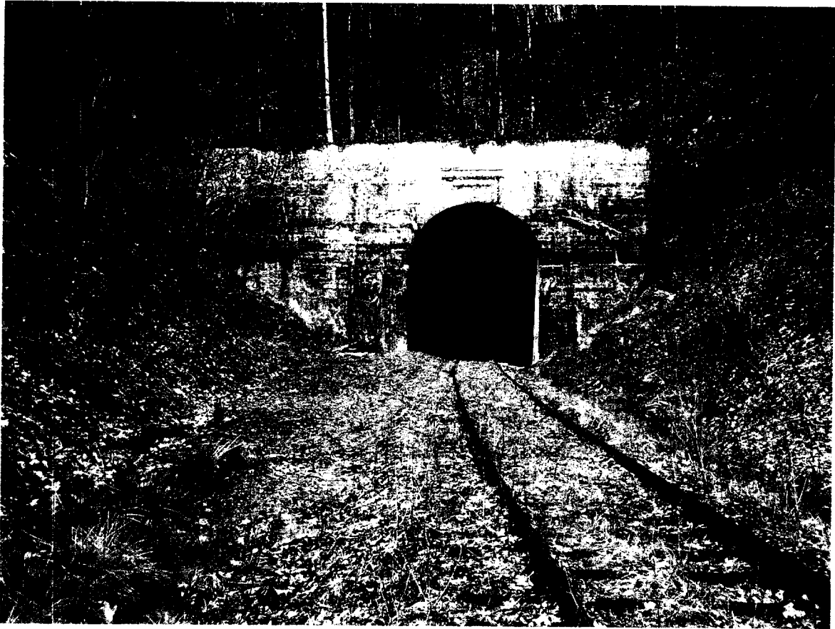
Coulter Tunnel South End looking North 35.73
