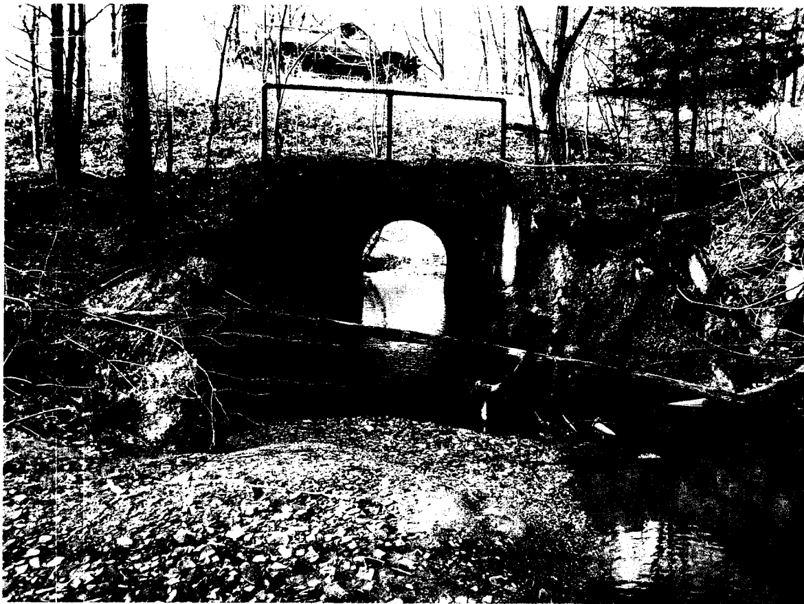
Arch 12' MP 45.09 West
