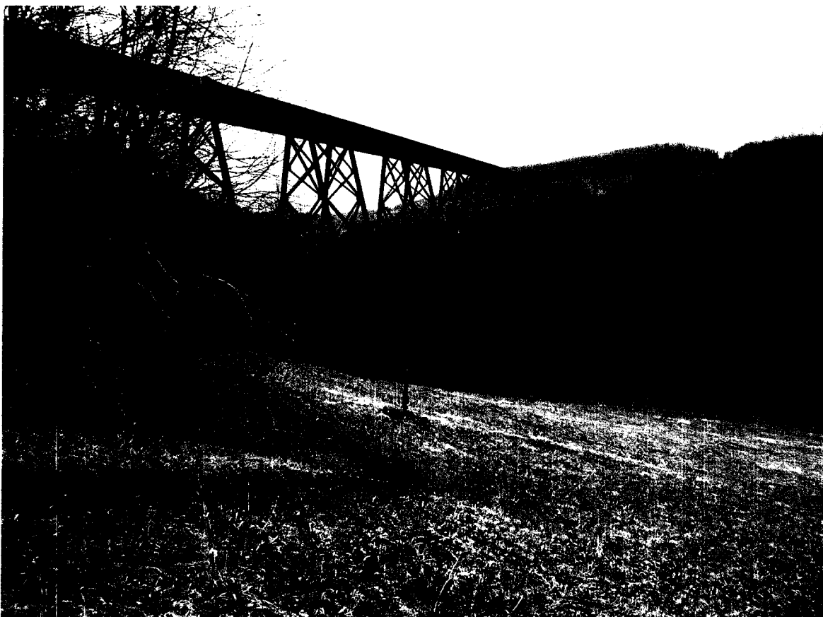
Bridge No. 33.71 East Side of South End looking North
