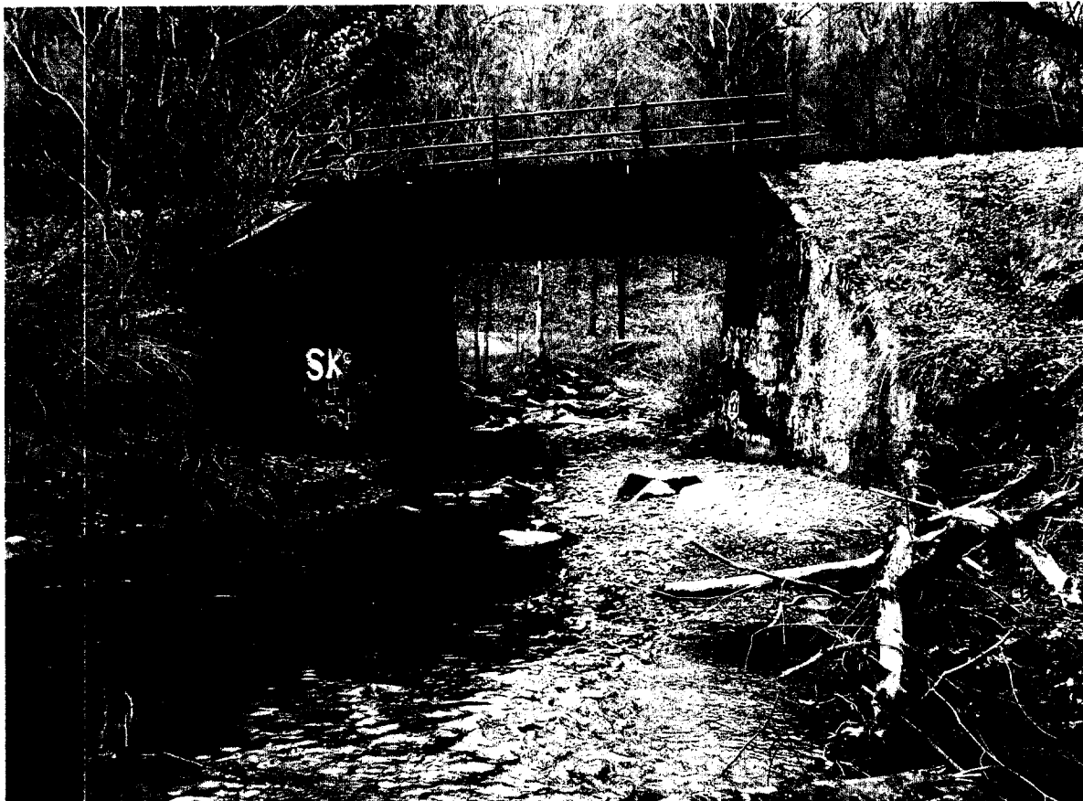
Bridge No. MP 59.21 East
