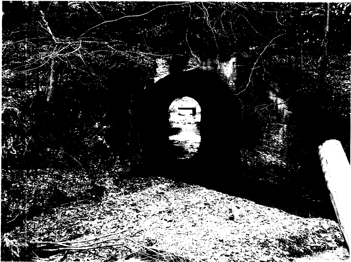
Arch 12' MP 42.86 West
