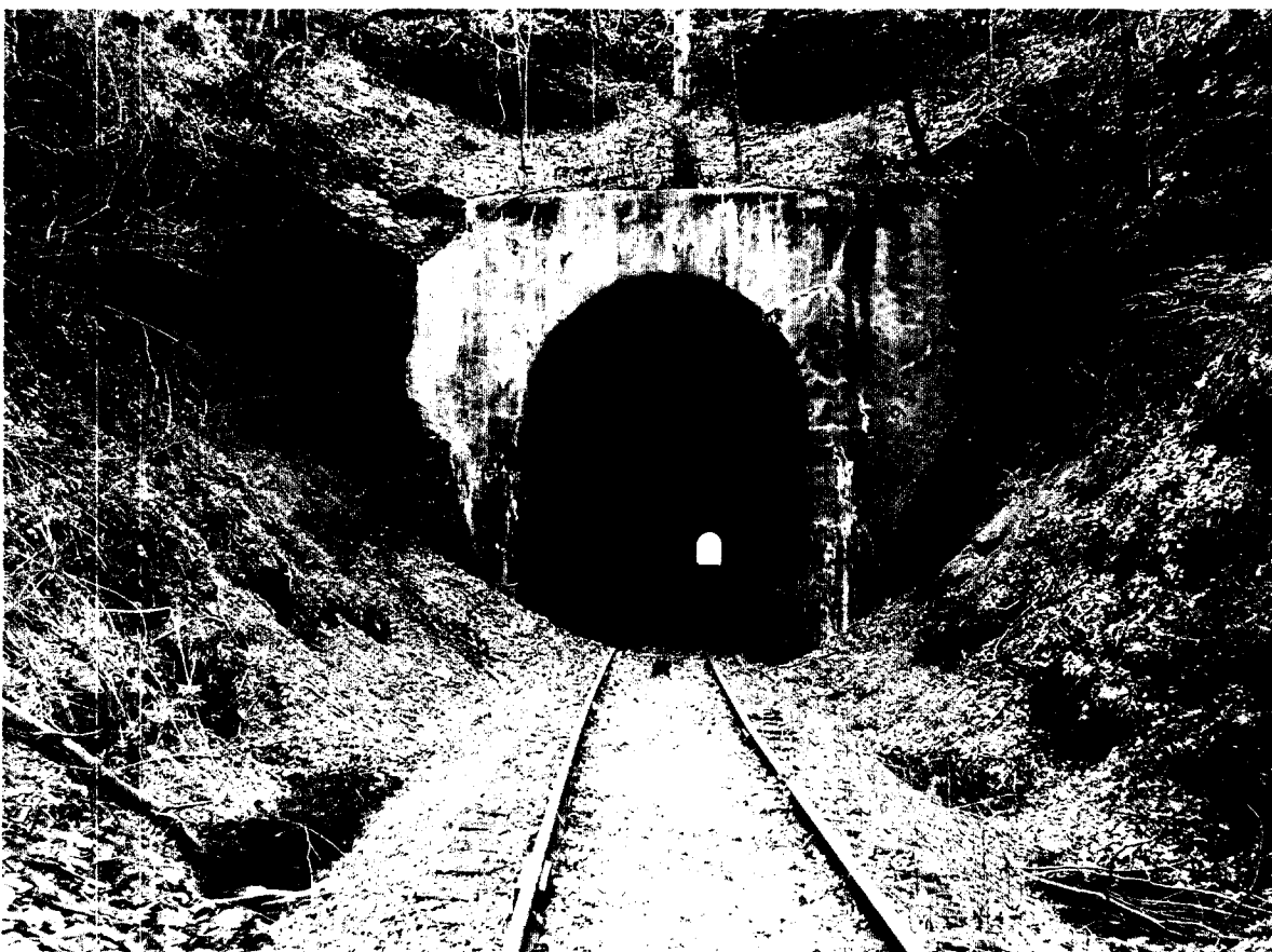
Mack Tunnel MP 56.73 South End looking North
