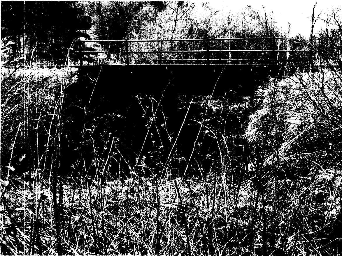
Bridge No. MP 45.95 West
