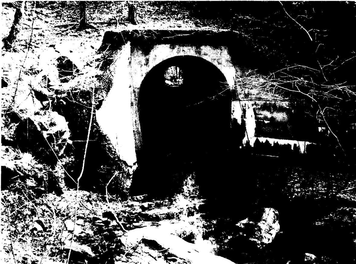
Arch 8' MP 50.49 East
