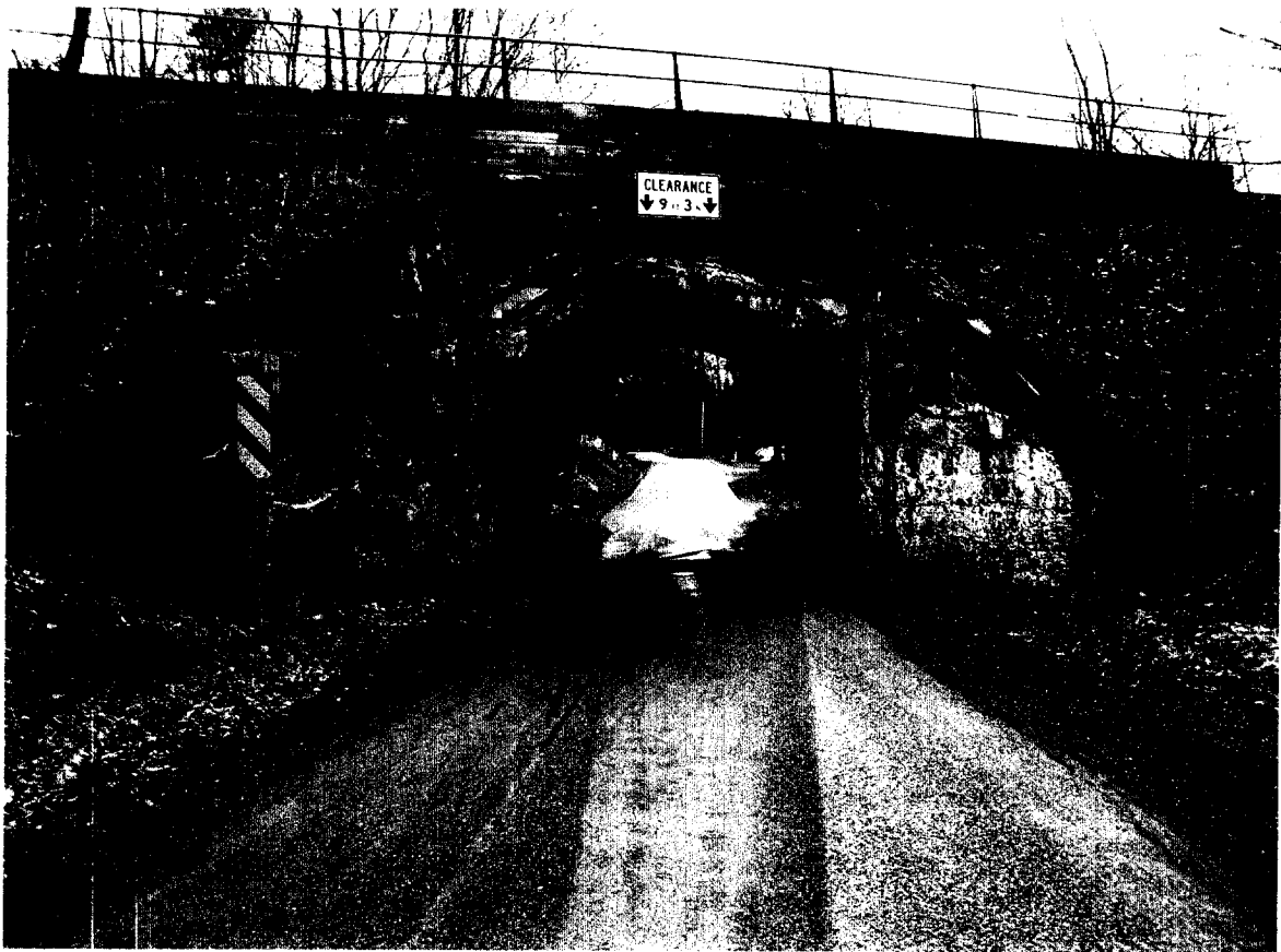
Arch 16' MP 29.11 West
