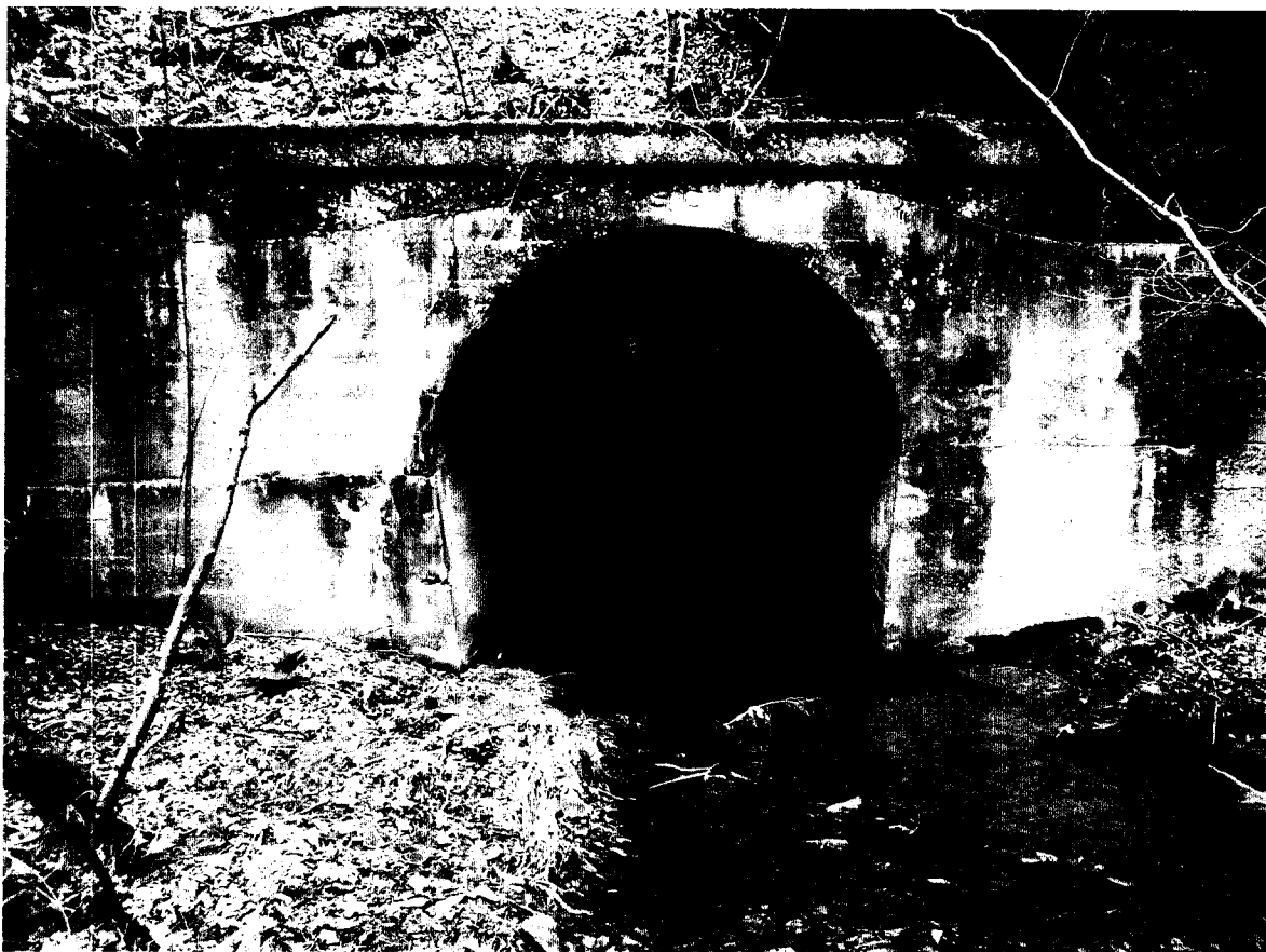
Arch 10' MP 47.92 East
