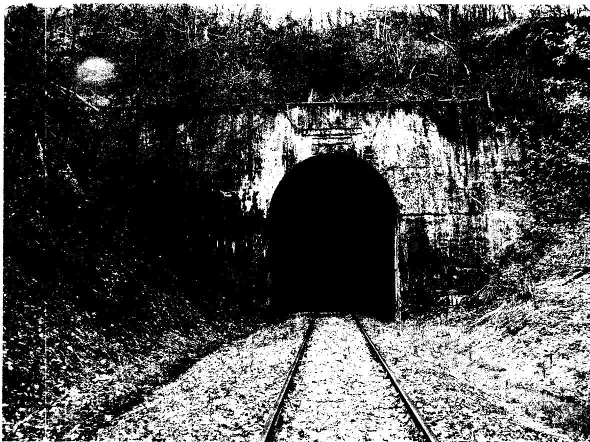
Coulter Tunnel North End looking South 35.73
