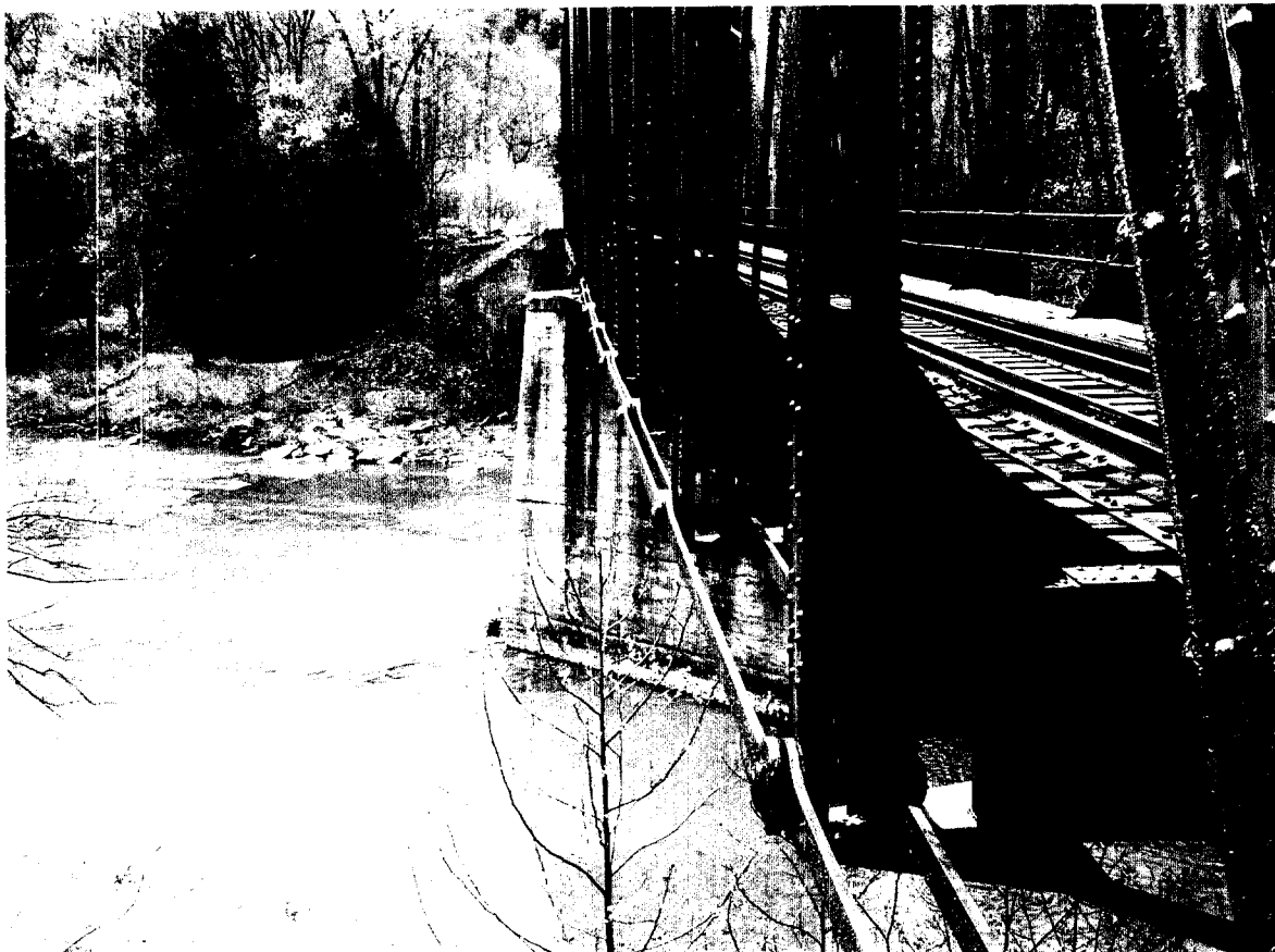
Bridge No. MP 57.81 East
