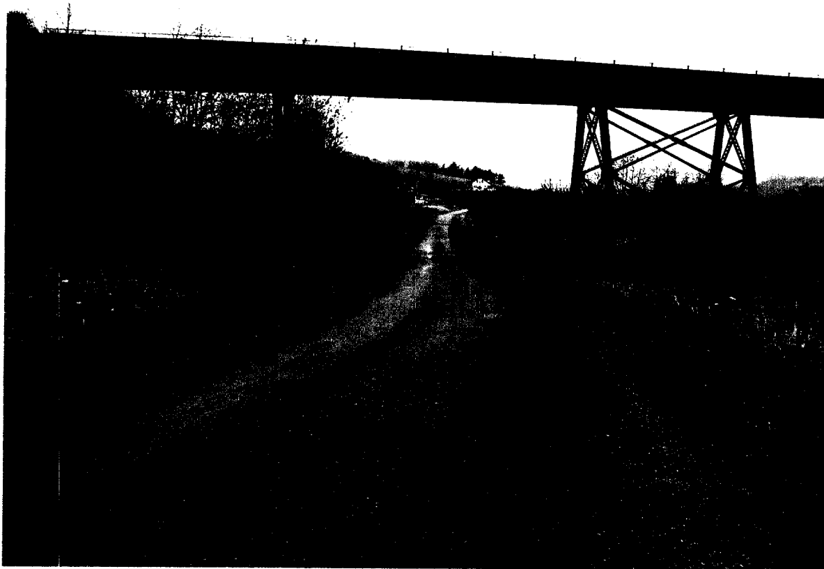
Bridge No. 38.4 East Side of South End
