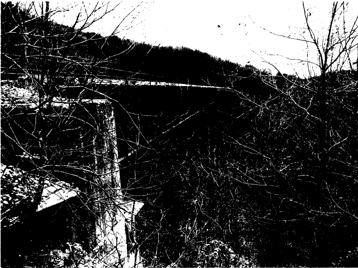
Bridge No. MP 51.23 South End East Side looking North
