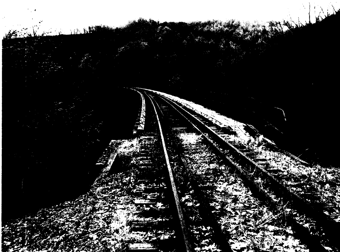
Bridge No. MP 51.86 North End looking South
