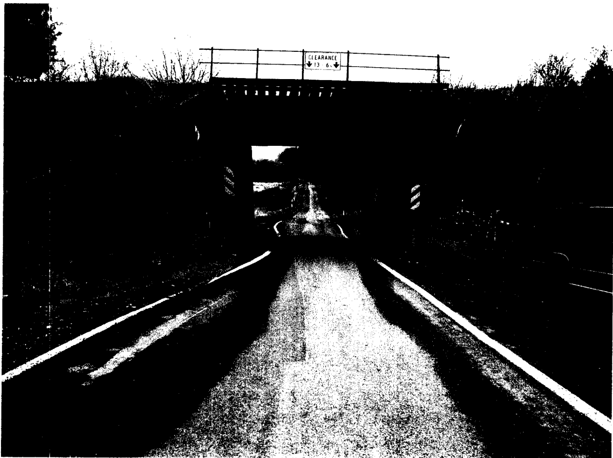
Bridge No. 42.34 East
