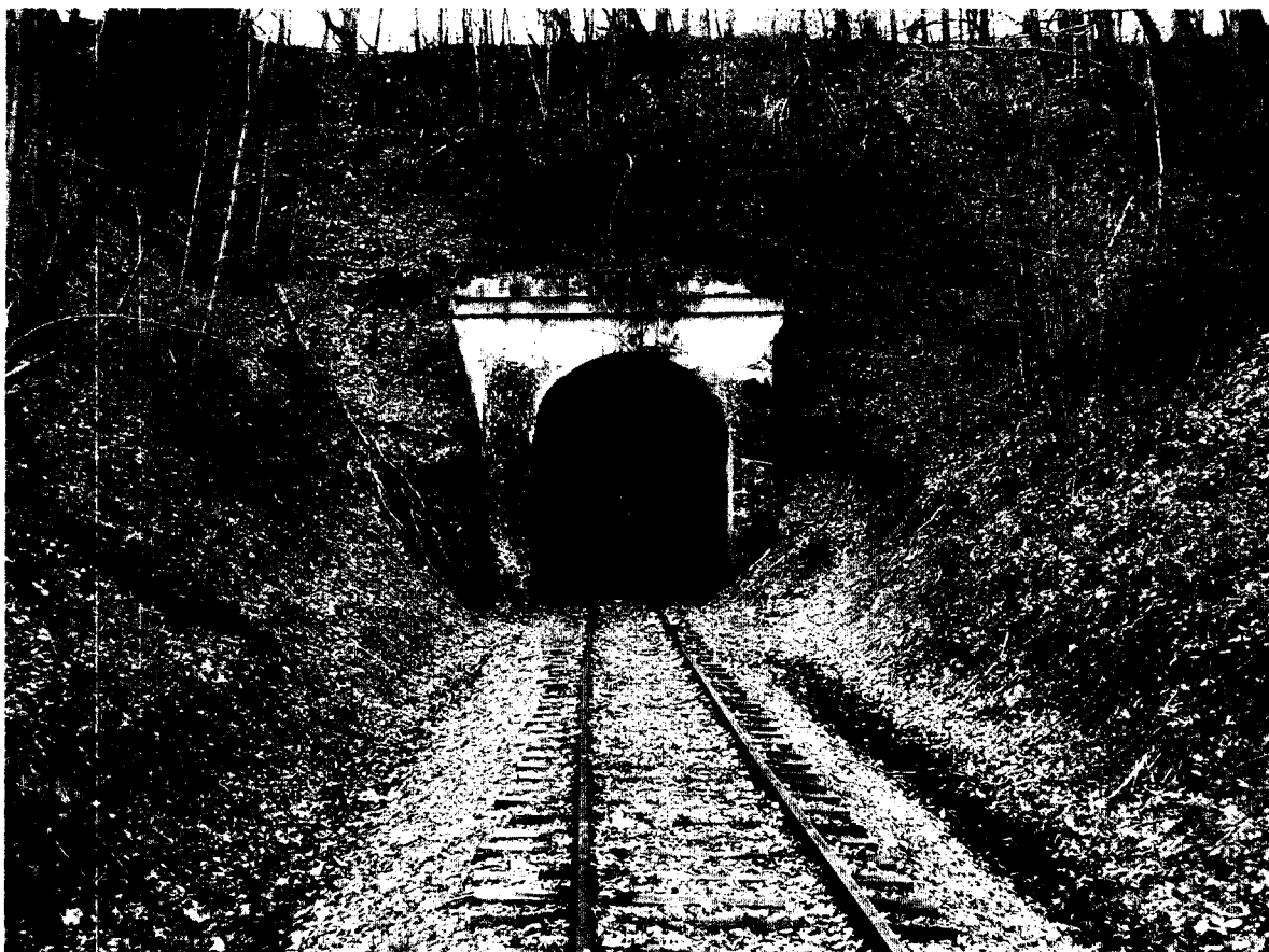
Mack Tunnel MP 56.73 North End looking South
