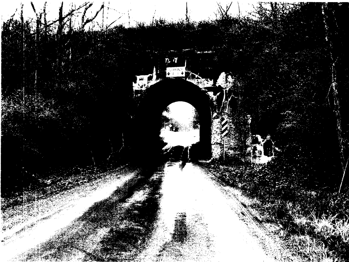
Arch 16' MP 28.02 East
