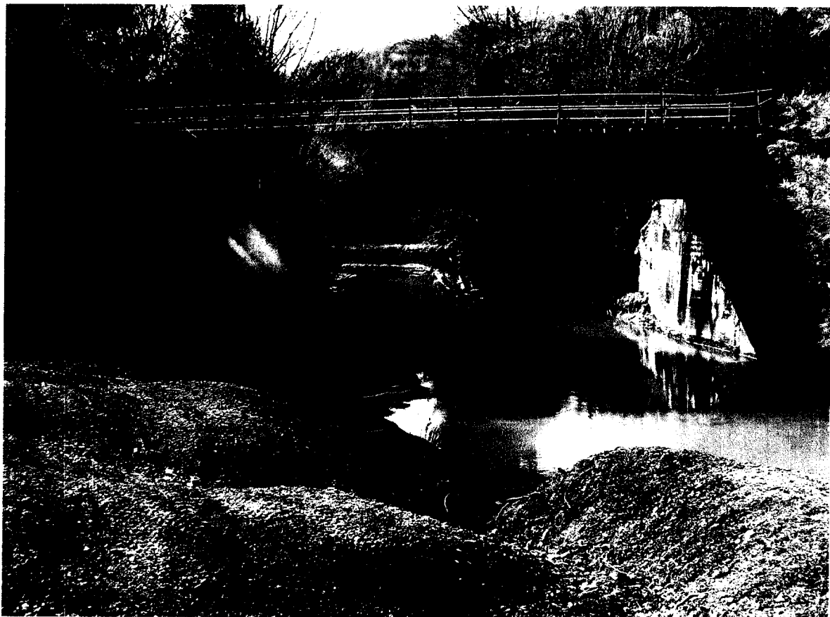
Bridge No. MP 45.60 West
