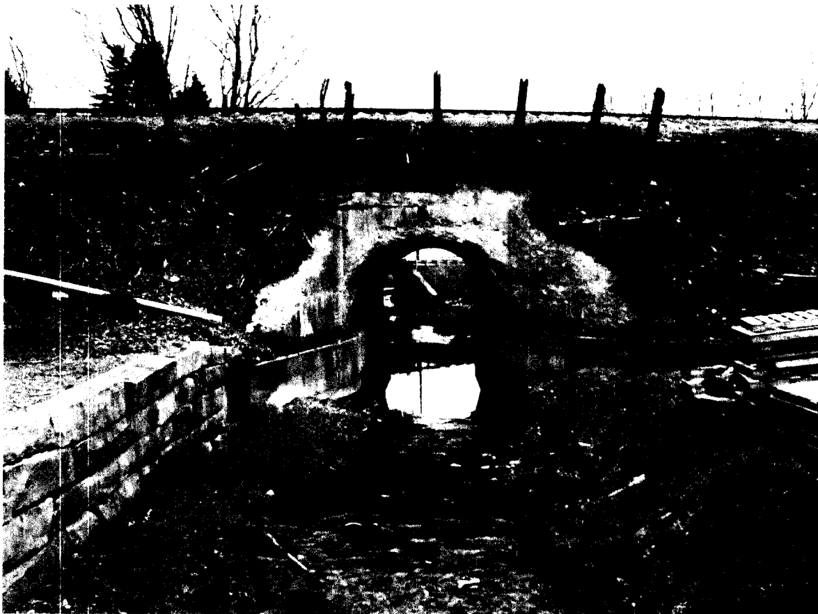
Arch 15' MP 44.57 East
