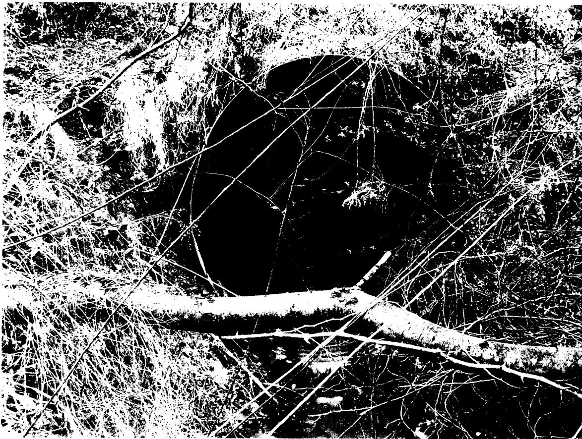
Arch 16' MP 42.39 East
