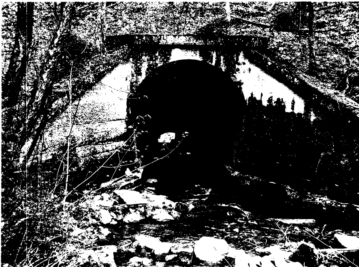
Arch 10' MP 52.69 West
