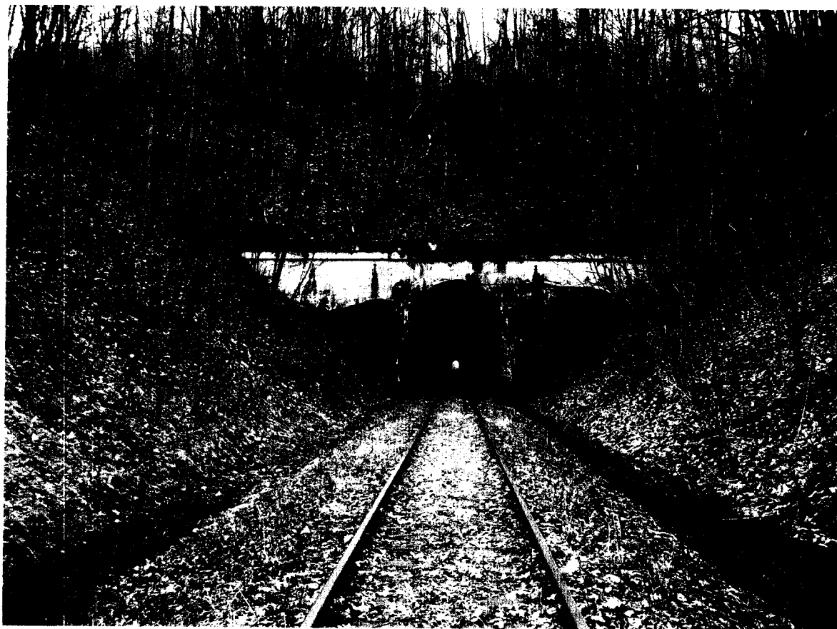
Mauk Tunnel MP 40.0 North End looking South
