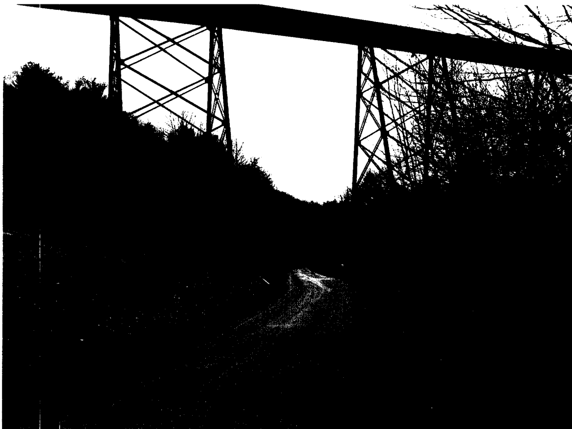
Bridge No. 33.71 East Side of South End
