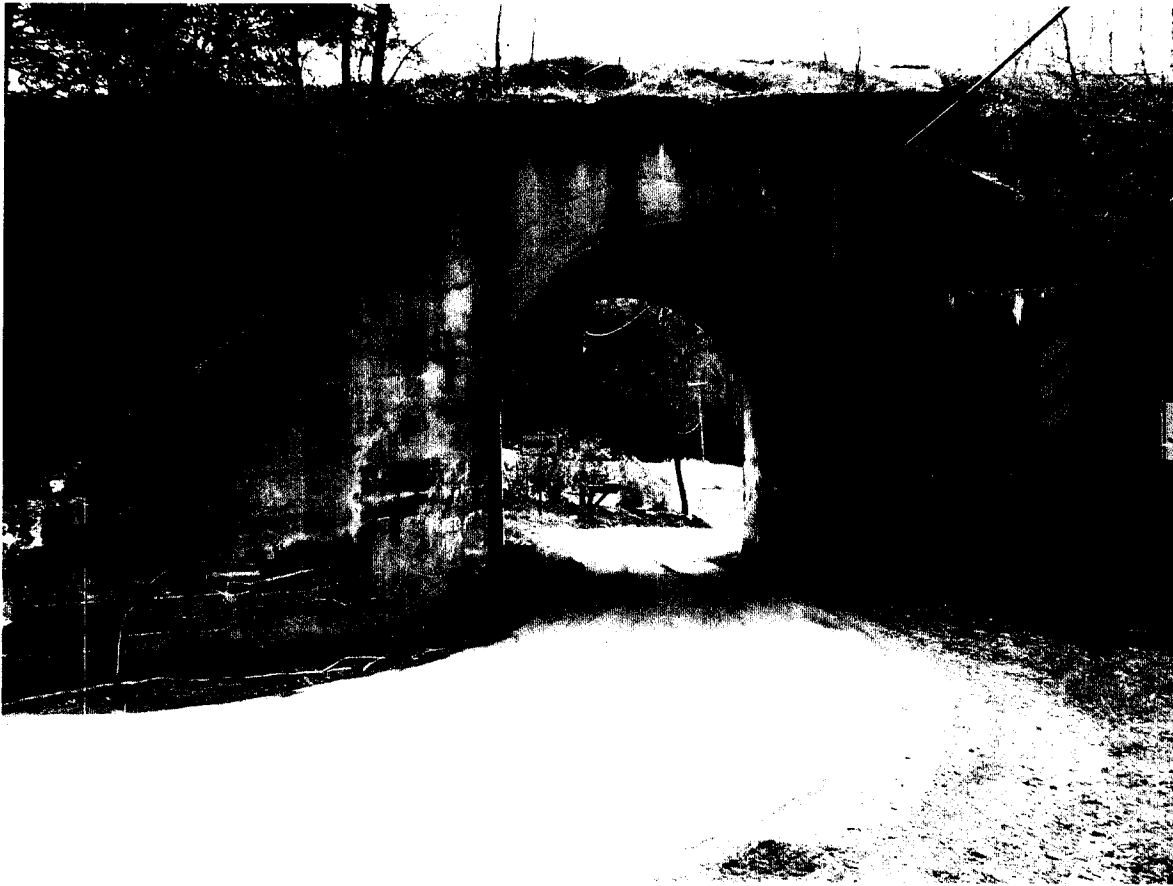
Arch 16' MP 48.92 West
