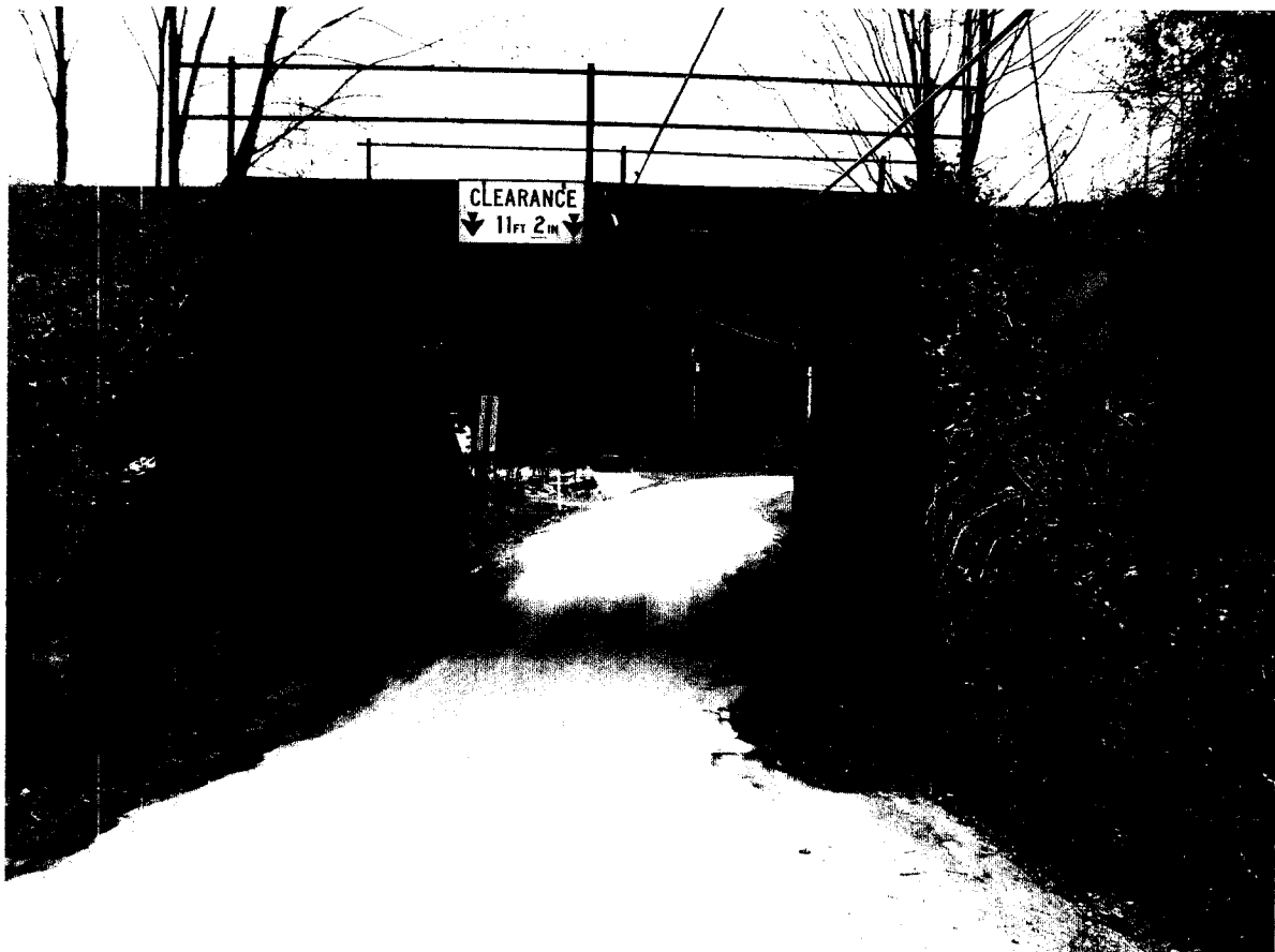
Bridge No. MP 52.75 West
