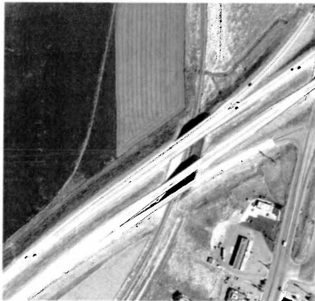
MP 708.75 under I-15 and ramp
