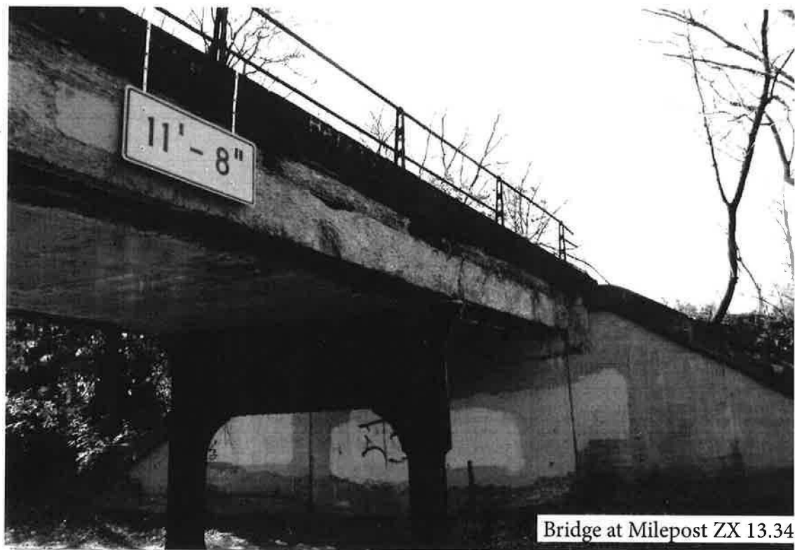
Bridge at Milepost ZX 13.34
