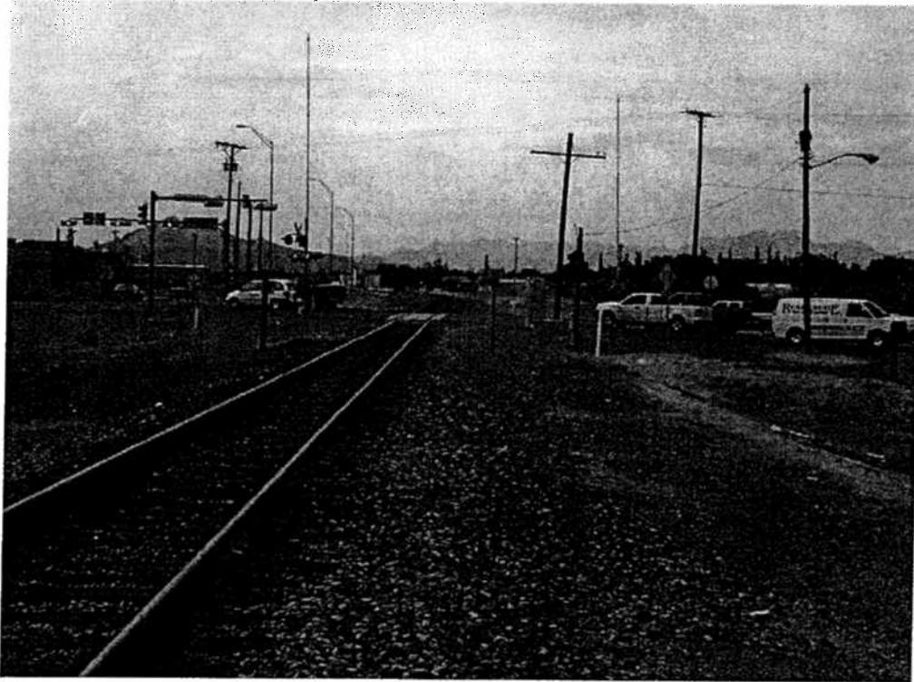
Figure 2F. – BNSF railway in El Paso, Texas
