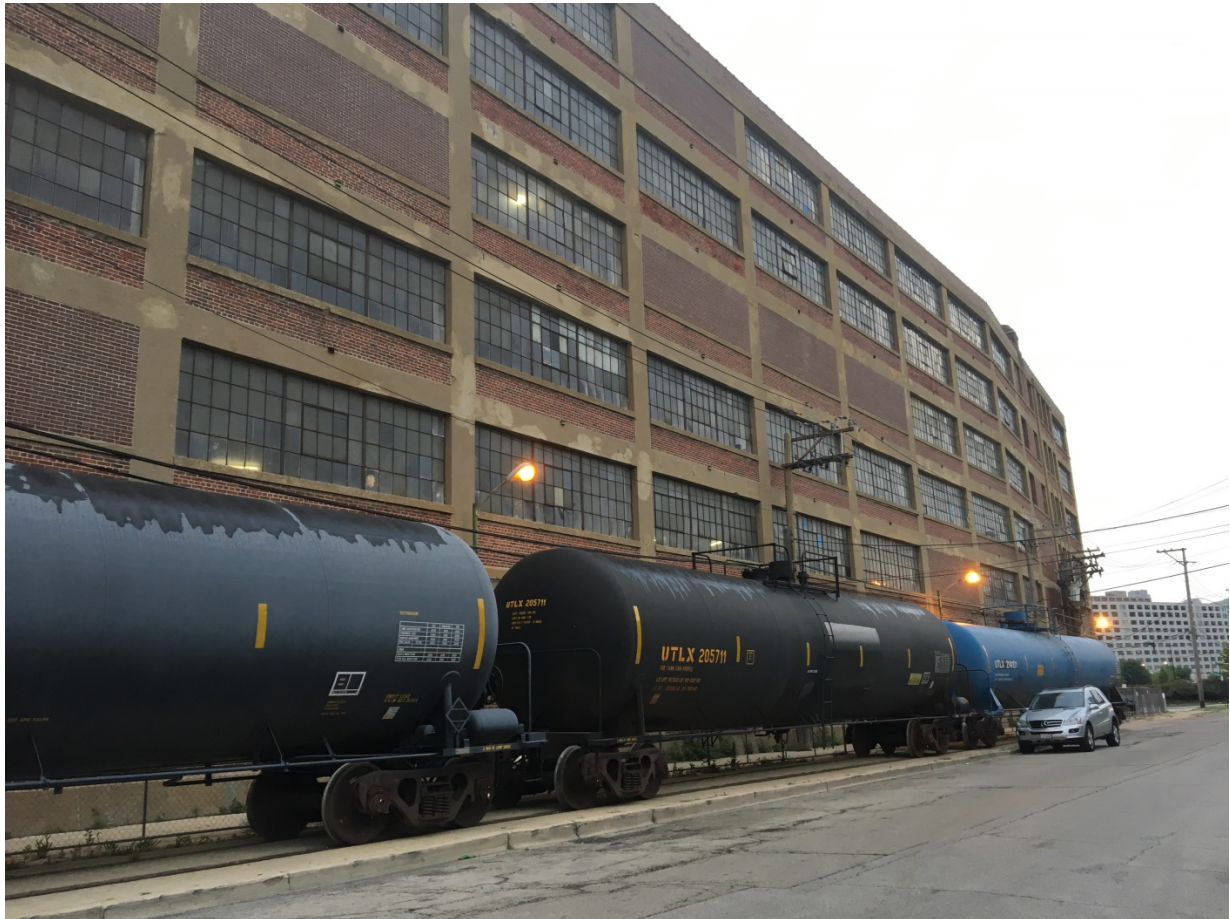
NORTH NORTH BRANCH STREET AT WEST BLISS STREET LOOKING SOUTHEAST AUGUST, 2017
