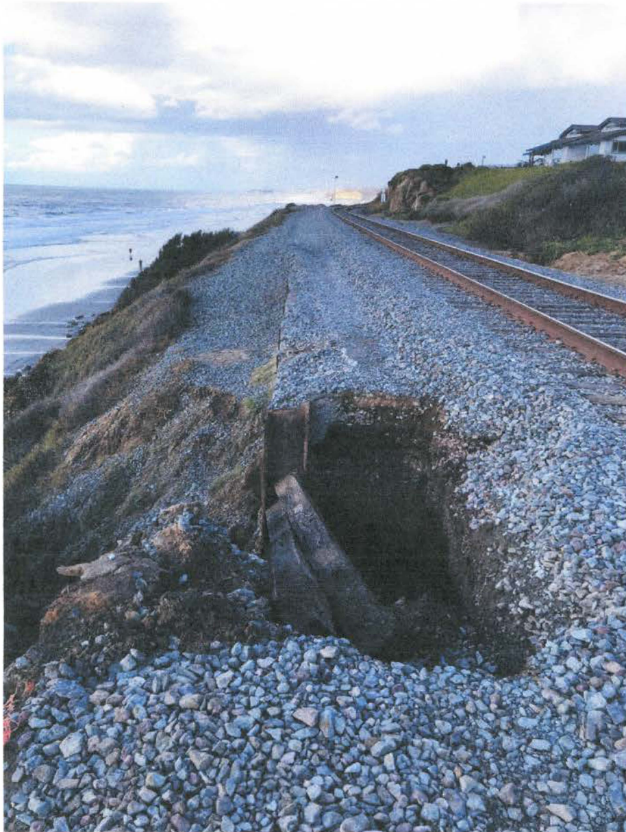
Photo 1 : Pre-construction view (looking north) of Component 1
