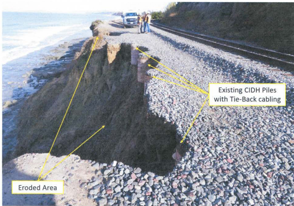
Photo 7 : Pre-construction view (looking north) of Component 2
