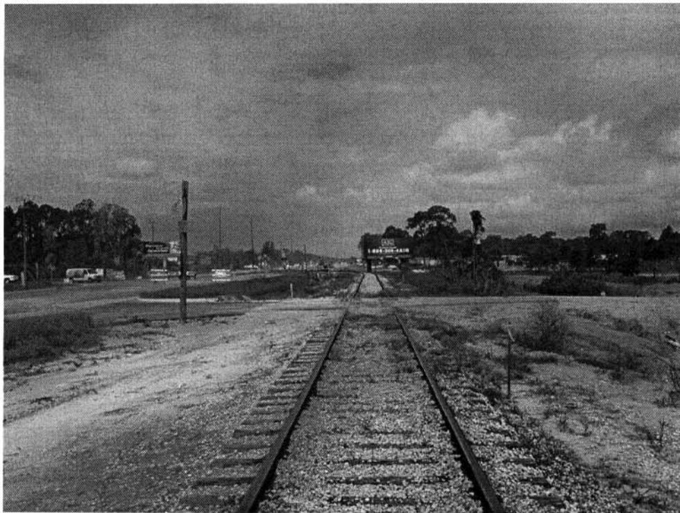
(3) FLORIDA POWER & LIGHT CROSSING LOOKING WEST
