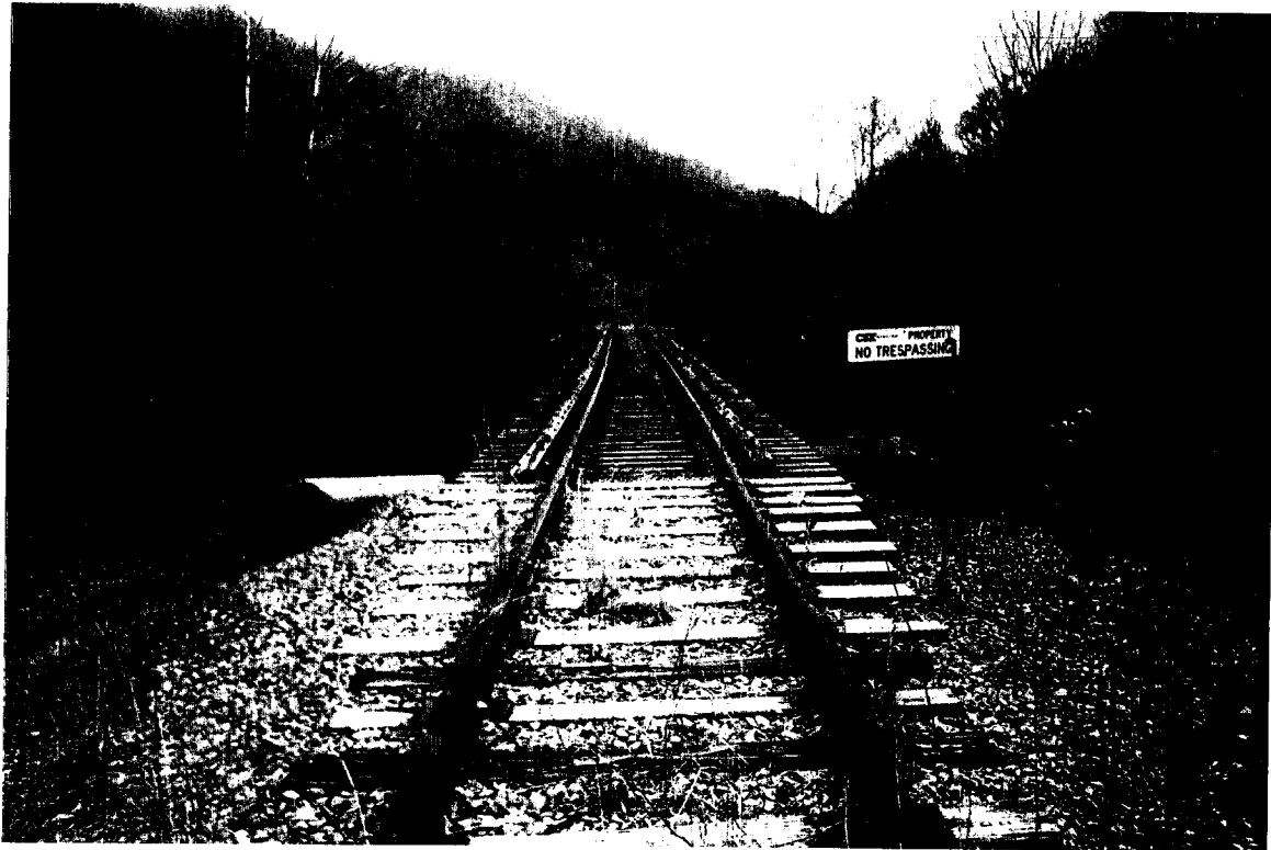
CSXT Bridge No. 15 (view 1)
