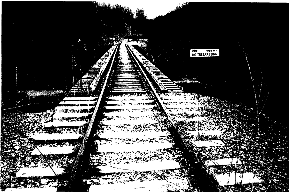
CSXT Bridge No. 15 (view 2)
