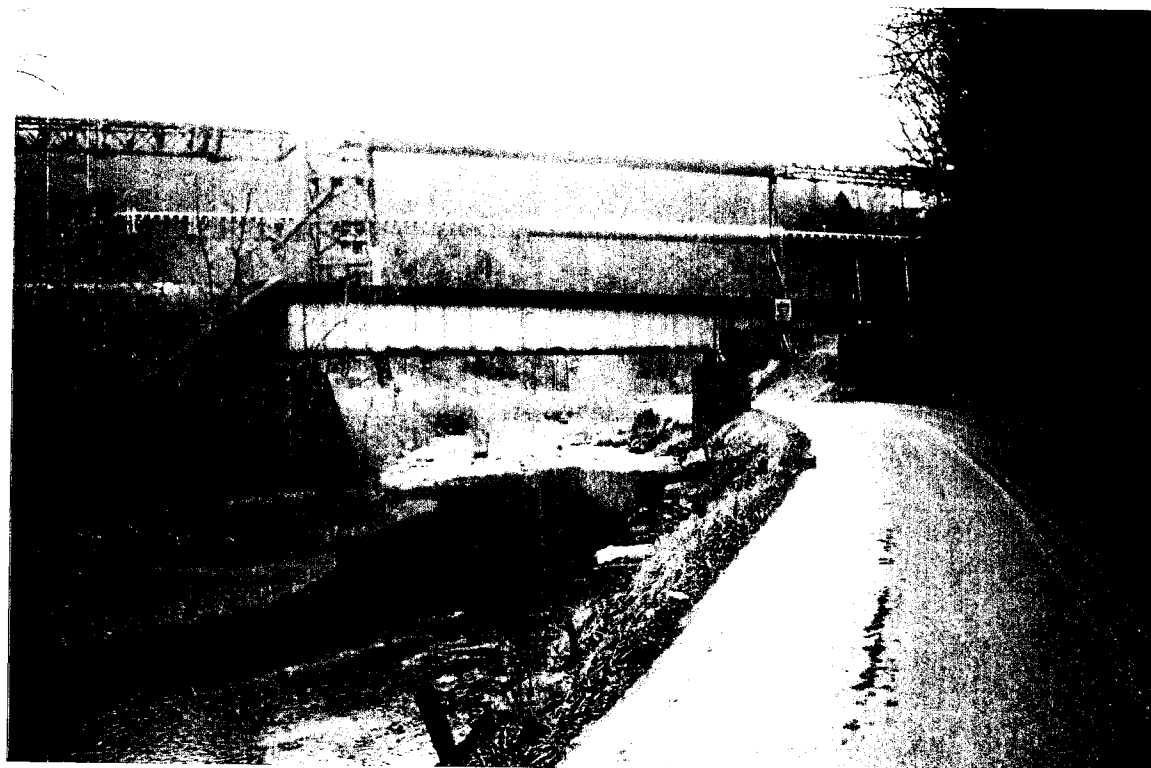
CSXT Bridge No. 14 (view 4)
