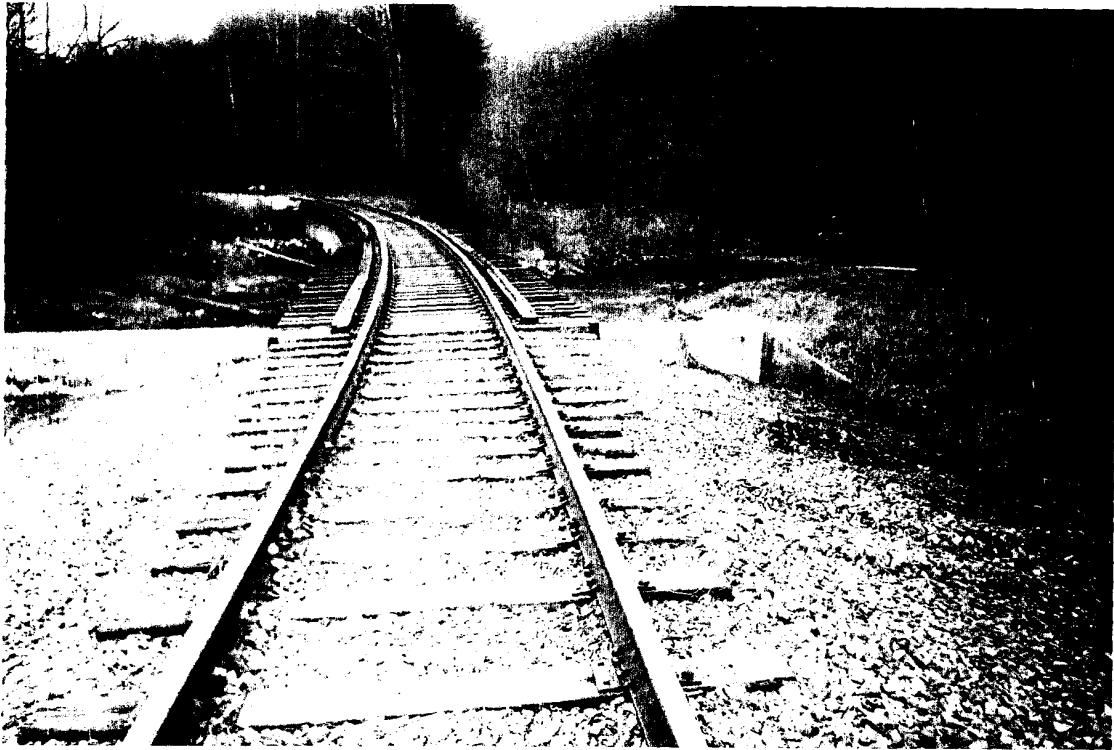
CSXT Bridge No. 10 (view 1)
