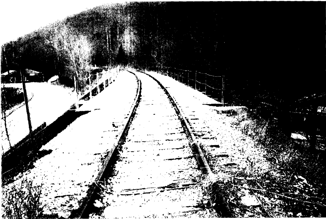
CSXT Bridge No. 13 (view 1)
