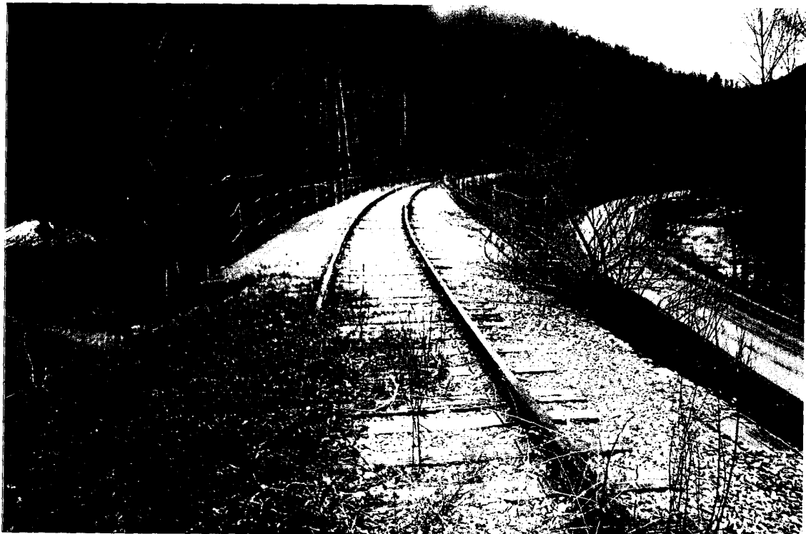
CSXT Bridge No. 13 (view 2)
