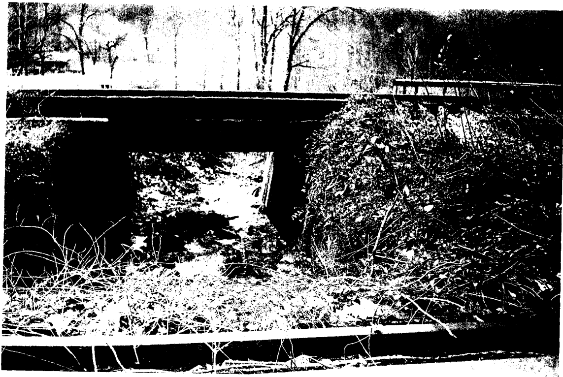
CSXT Bridge No. 12 (view 4)
