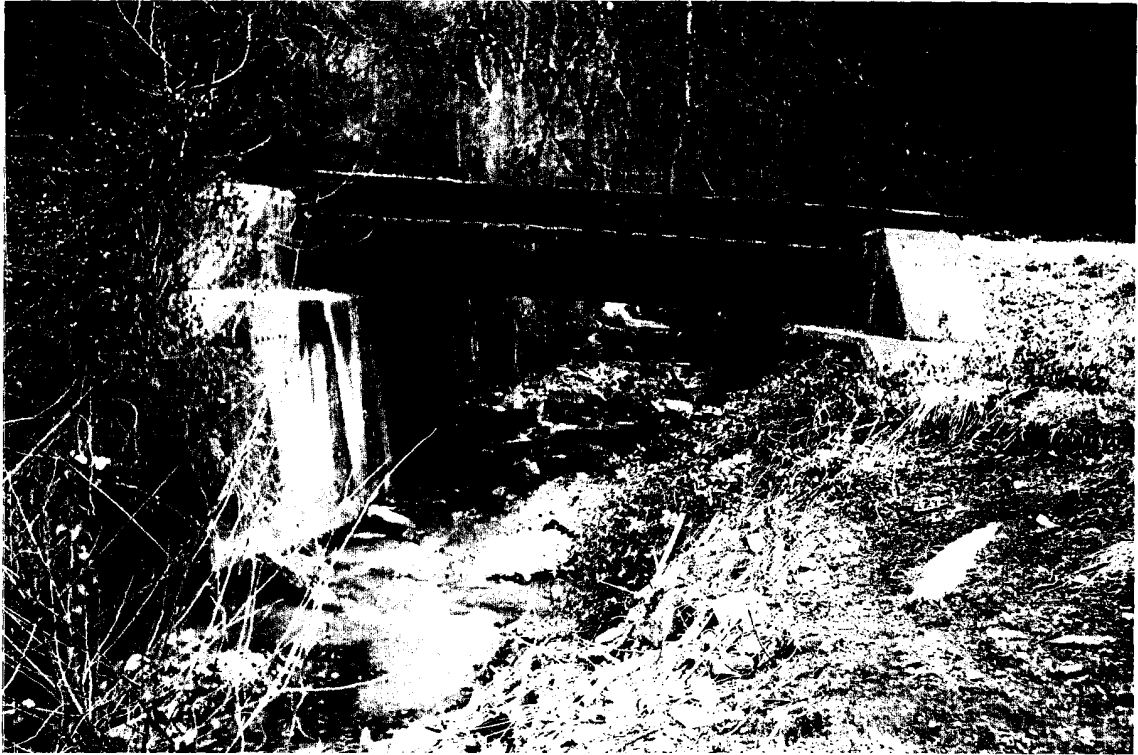
CSXT Bridge No. 12 (view 3)
