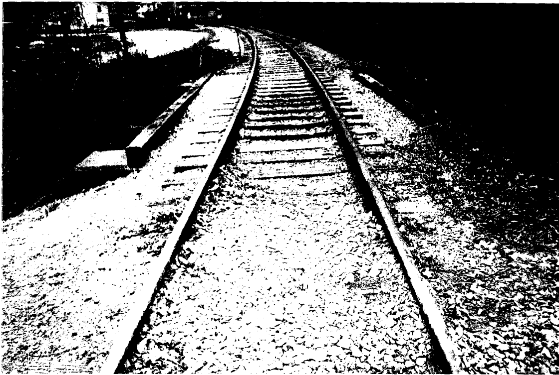
CSXT Bridge No. 12 (view 1)
