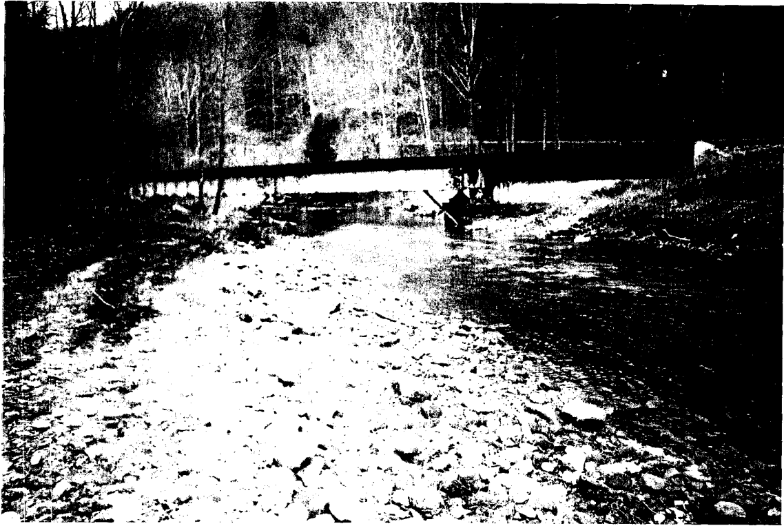
CSXT Bridge No. 10 (view 3)
