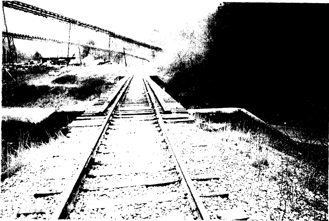
CSXT Bridge No. 14 (view 1)
