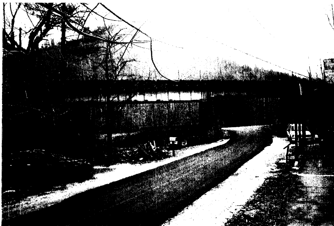
CSXT Bridge No. 13 (view 3)
