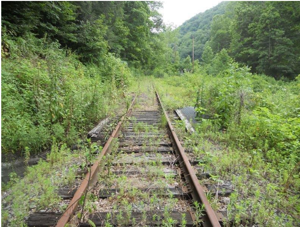
Bridge milepost CLN 9.30
