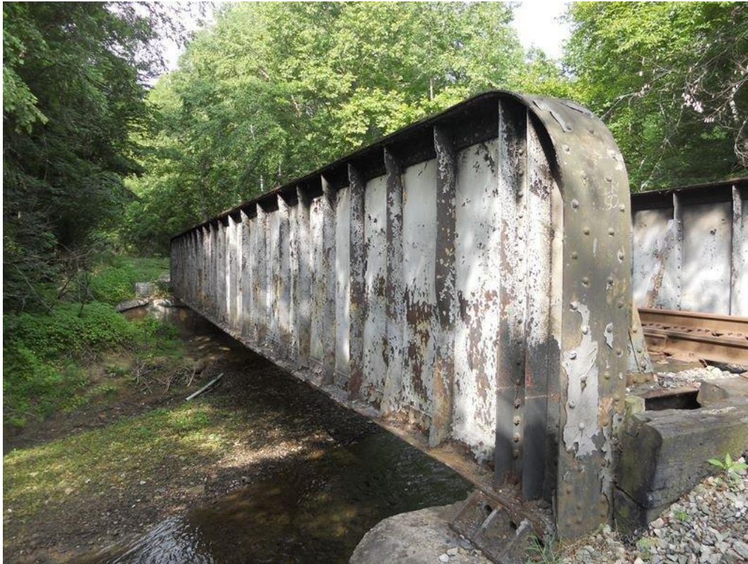
Bridge milepost CLN 0.50
