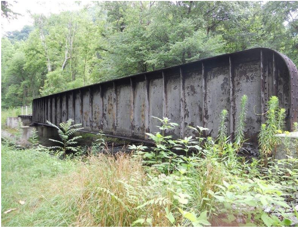
Bridge milepost CLN 3.80
