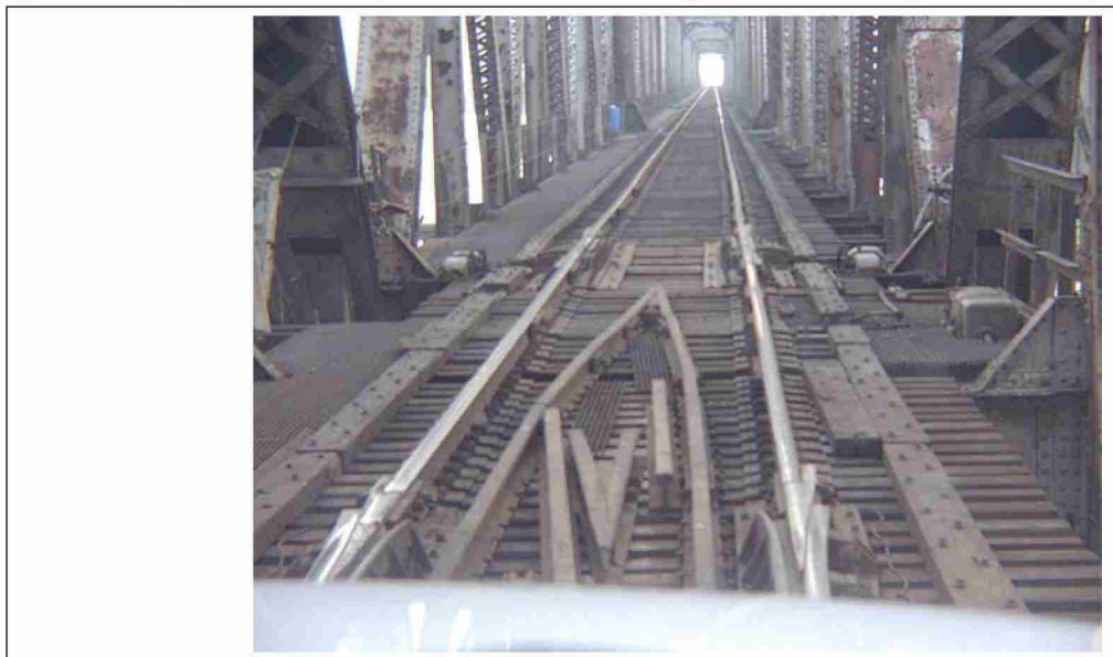
Figure 7-2 Rigolets Bridge MP 775.4 (miter rails and bridge truss looking southward)
