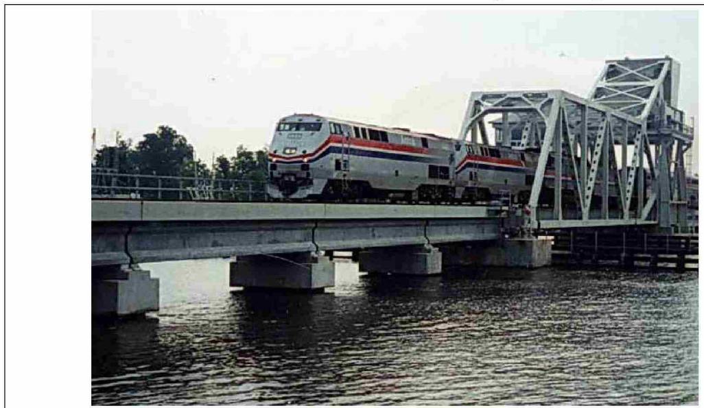
Figure 7-1 Pascagoula Bridge MP 706.8
