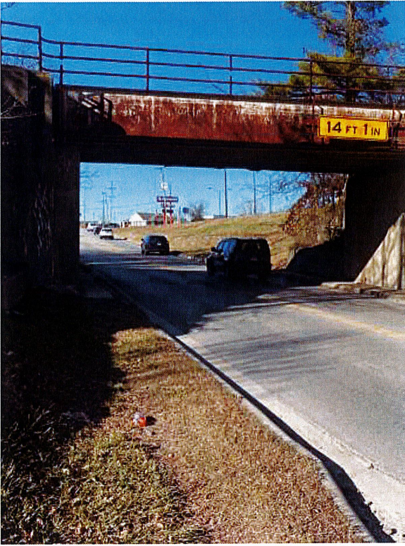
Kearney Road/10 Highway Westbound
