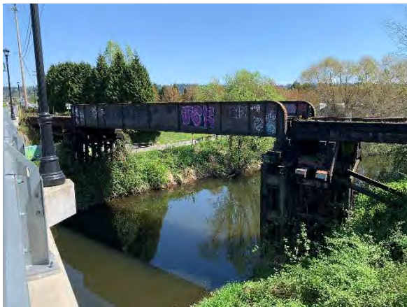
Figure 3 South Sammamish River Bridge, viewing southeast from NE 175th Street Bridge
