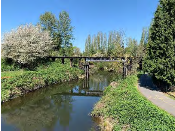
Figure 2 North Sammamish River Bridge, viewing north from NE 175th Street.
