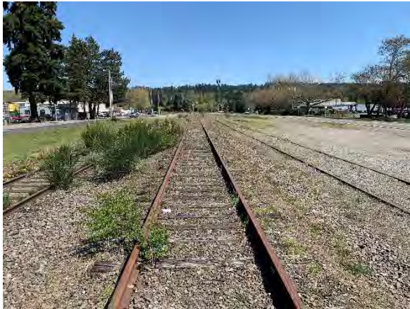
Figure 1 SLS&E segment northeast of 131st Avenue Bridge with transfer tracks to left and right, viewing northeast. [Note: Somerailroad ties have been removed from the southern transfer track (right)]
