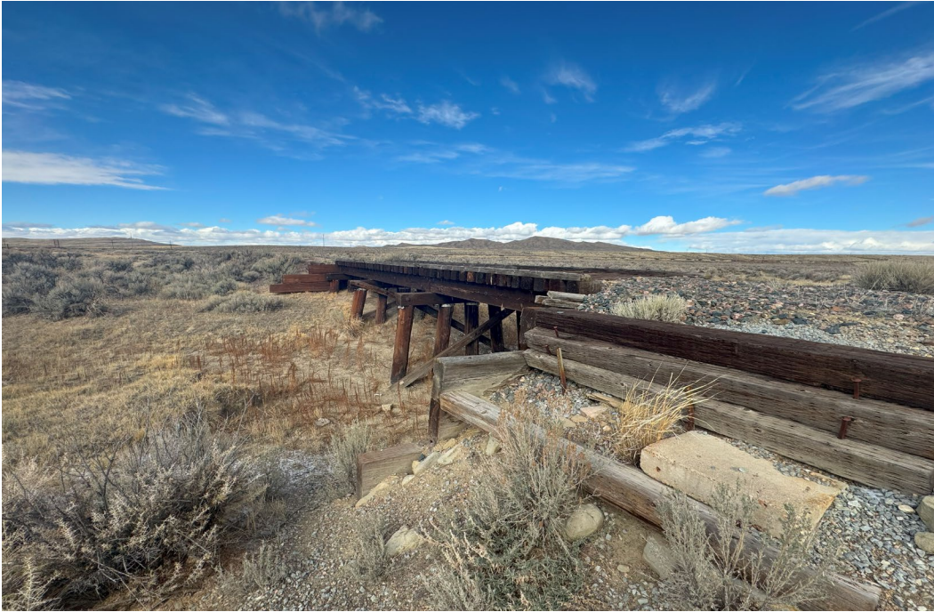
Bridge at M.P. 0.84
