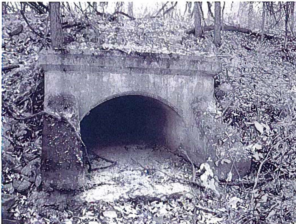
Arch Culvert (#1036) MP 219.8 (4.4 feet)
