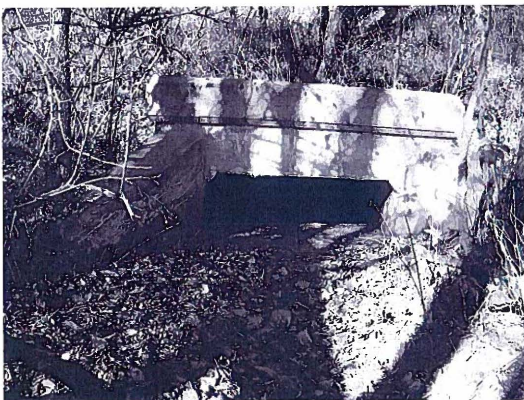
Box Culvert (#1134) MP 231.3 (3 feet)
