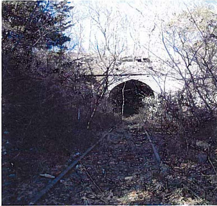
Tunnel No. 2 East Portal (MP 128.67 to 128.93)
