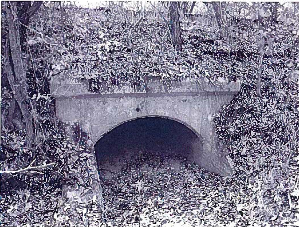
Arch Culvert (#1049) MP 221.7 (6.4 feet)
