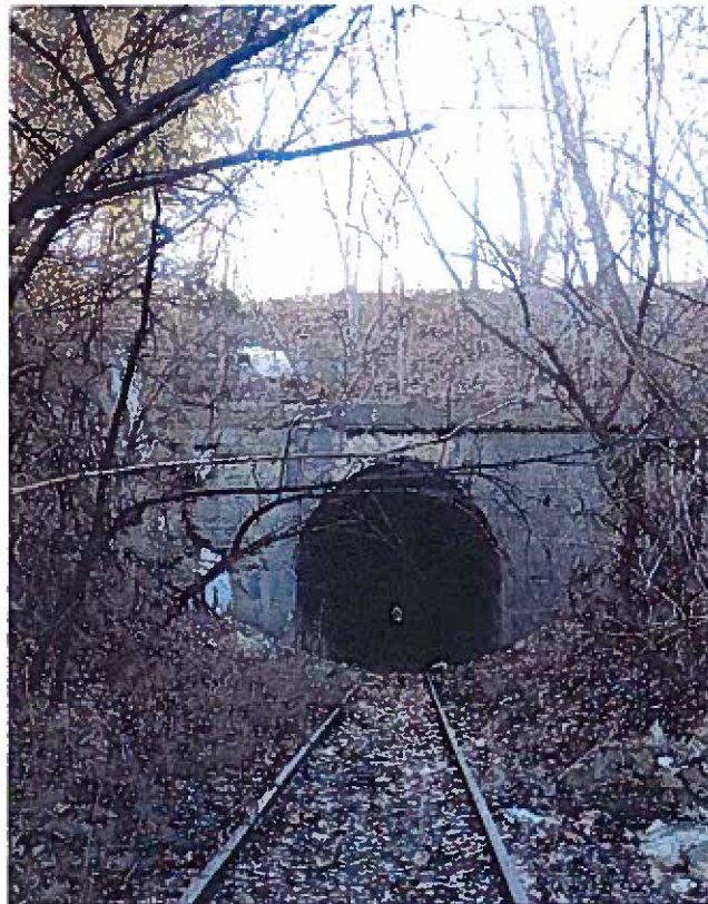
Tunnel No. 3 West Portal (MP 148.78 to 149.09)
