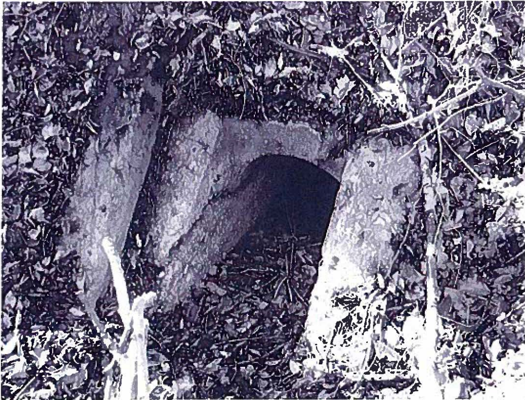
Arch Culvert (#1047) MP 221.5 (2 feet)
