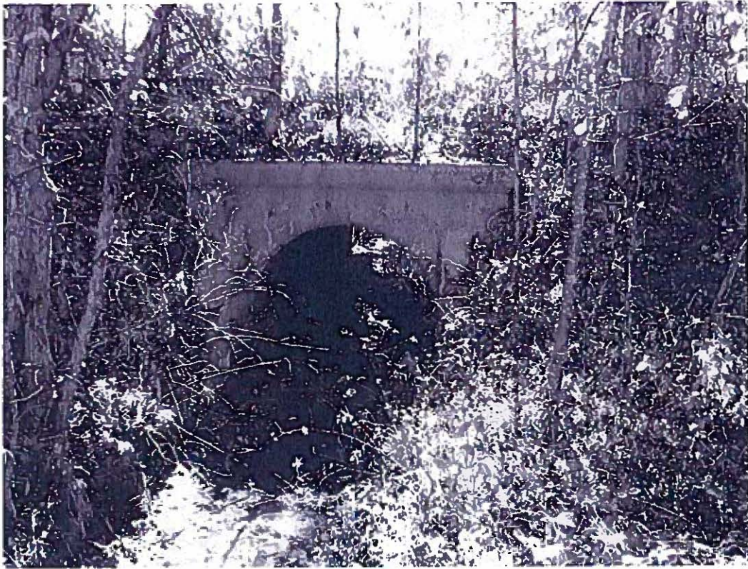
Arch Culvert (#1013) MP 217.1 (5.2 feet)
