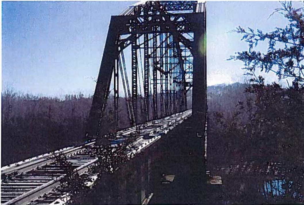
Osage River Bridge Photo 1 (approx. MP 143.3)
