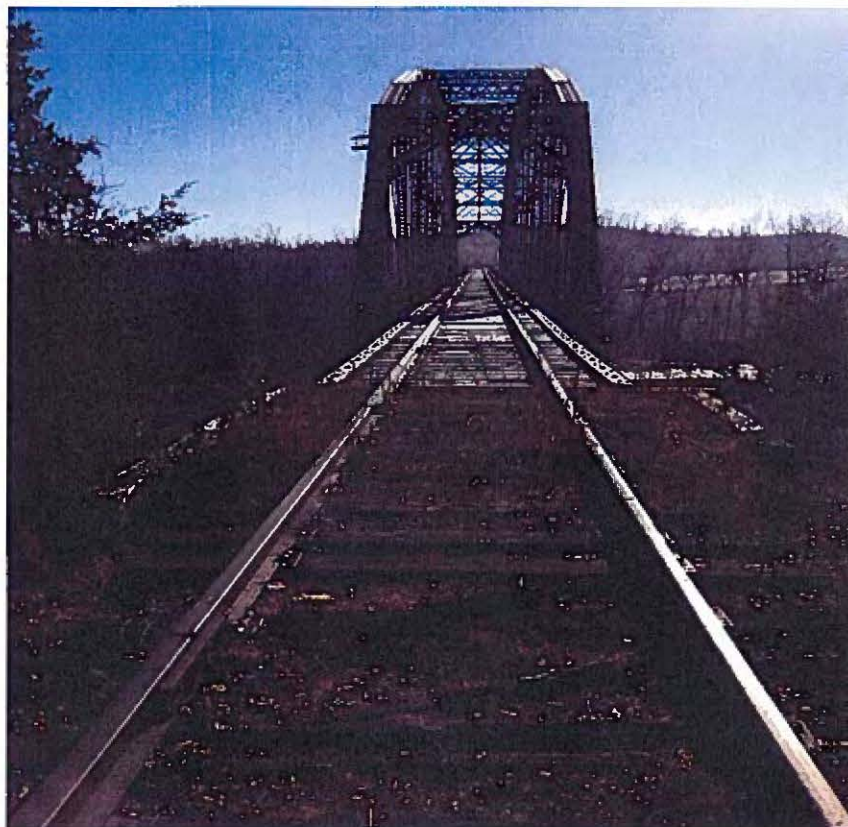
Osage River Bridge Photo 2 (approx. MP 143.3)
