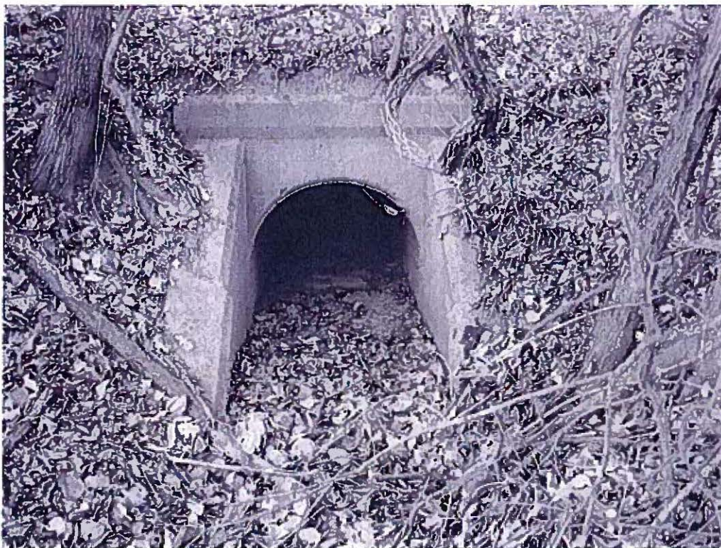
Arch Culvert (#1104) MP 228.6 (3 feet)
