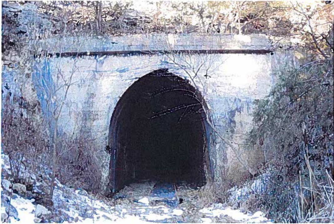
Tunnel No. 3 East Portal (MP 148.78 to 149.09)
