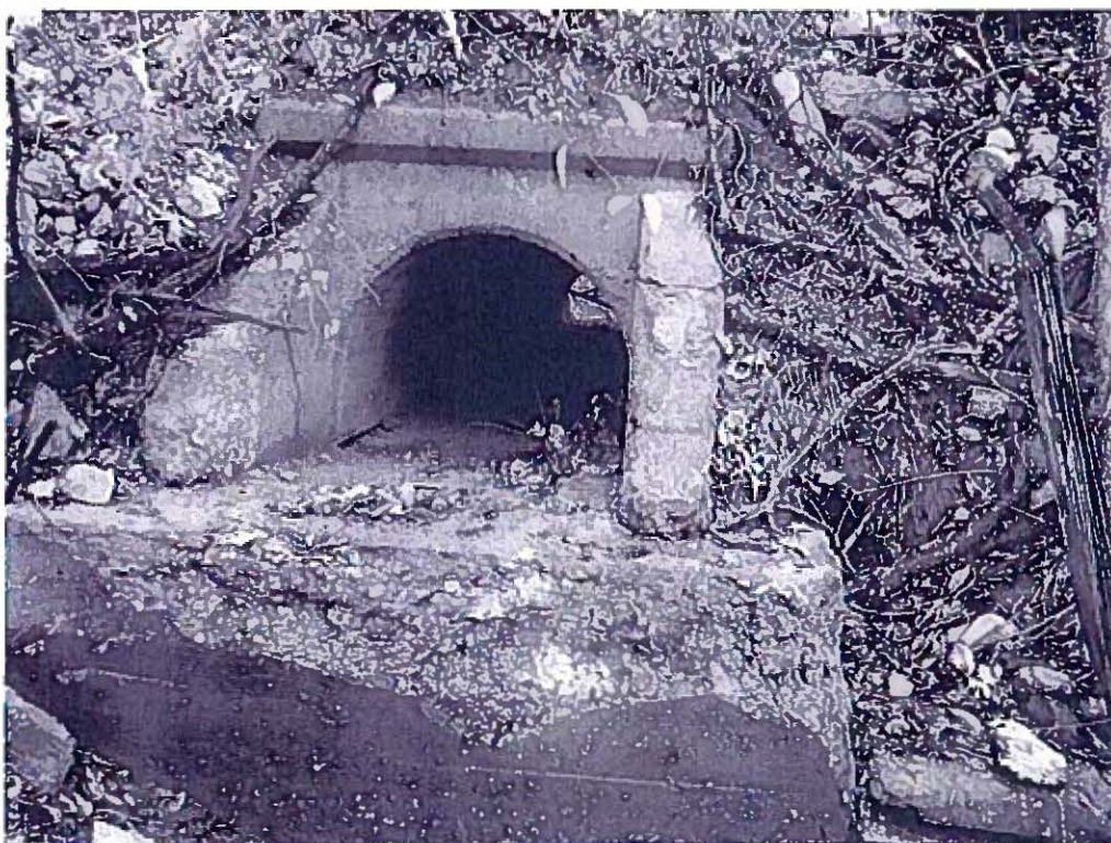
Arch Culvert (#1076) MP 225 (3.7 feet)
