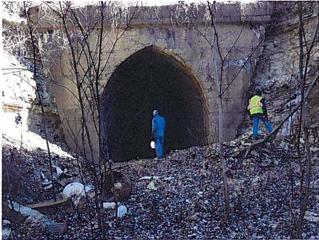
Tunnel No. 1 East Portal (MP 118.44 to 118.58)
