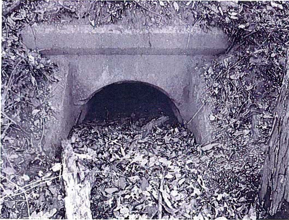
Arch Culvert (#1072) MP 224.2 (3 feet)
