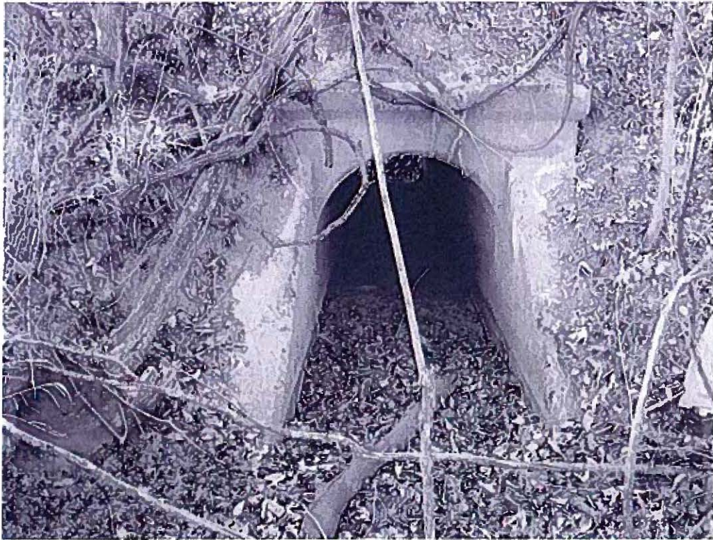
Arch Culvert (#1107) MP 228.9 (4 feet)
