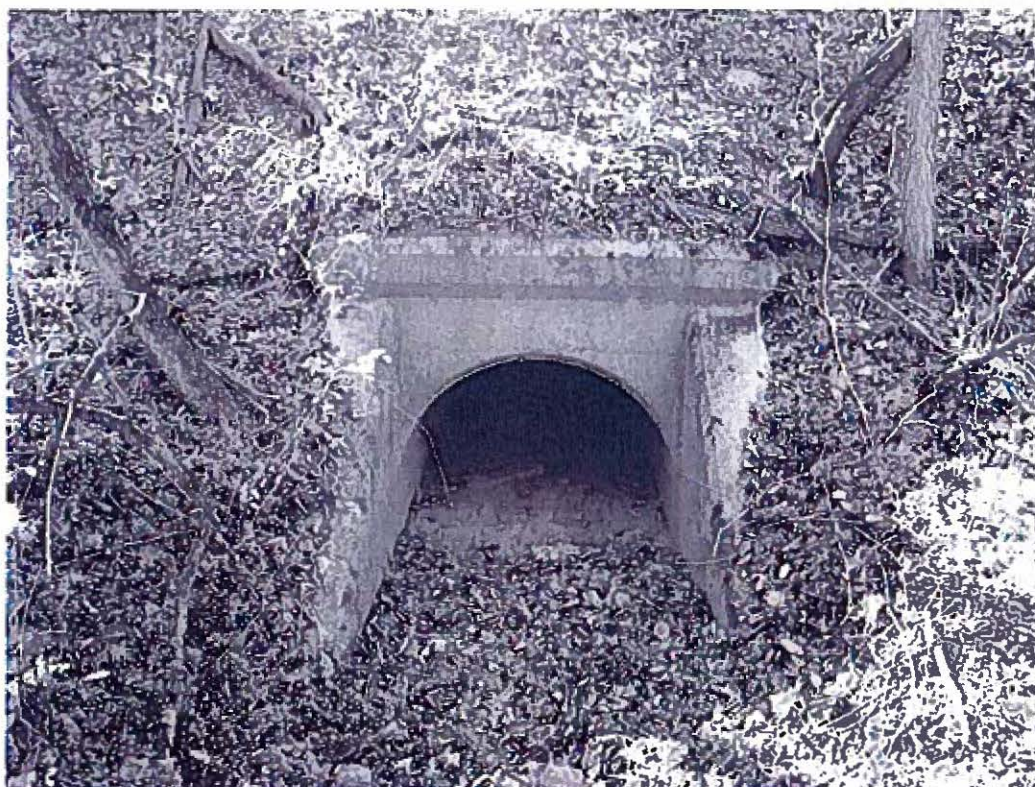
Arch Culvert (#1144) MP 232.7 (4 feet)
