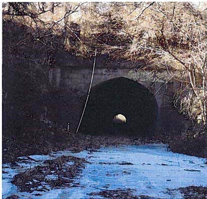
Tunnel No. 1 West Portal (MP 118.44 to 118.58)
