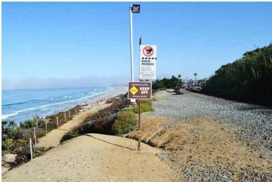
Figure 14 A path delineated by guardrails leads directly to the railroad corridor from Powerhouse Park in Del Mar, encouraging trespassers. Looking north from the vicinity of 15th Street near MP 244.2. (Source: WSP)
