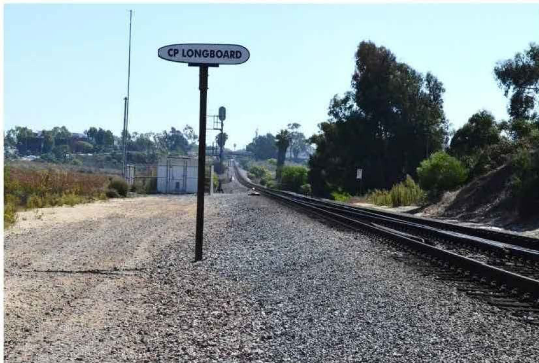
Figure 7 The rail corridor leading to the Buena Vista Lagoon bridge is commonly used by trespassers and is adjacent to several transient encampments. Looking south from CP Longboard/Eaton Street in Oceanside near MP 228.4. (Source: WSP)
