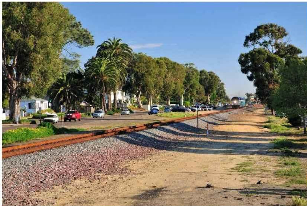
Figure 10 The railroad corridor in Encinitas is commonly used for informal parking and has no physical barriers to discourage trespassers. Looking south from Jupiter Street near MP 236.0. (Source: Caltrans District 11)
