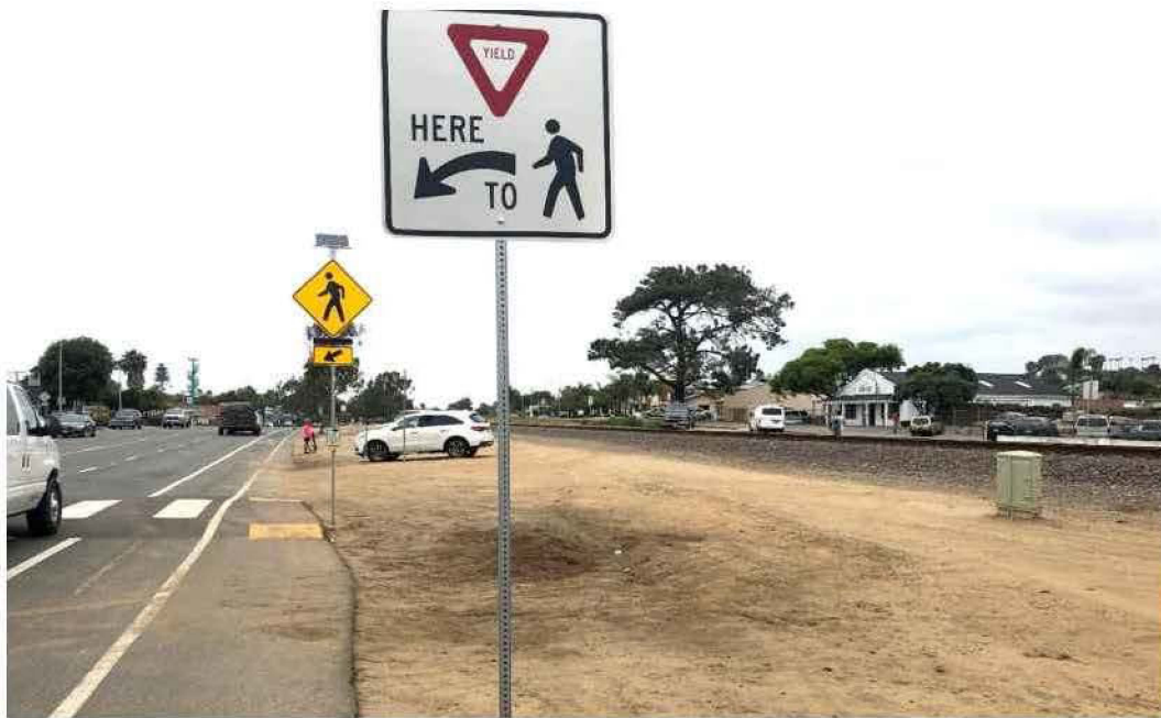
Figure 9 Newly installed pedestrian crossings of Coast Highway 101 in Encinitas may encourage trespassing in the railroad corridor. Looking north from Basil Street near MP 236.9. (Source: WSP)
