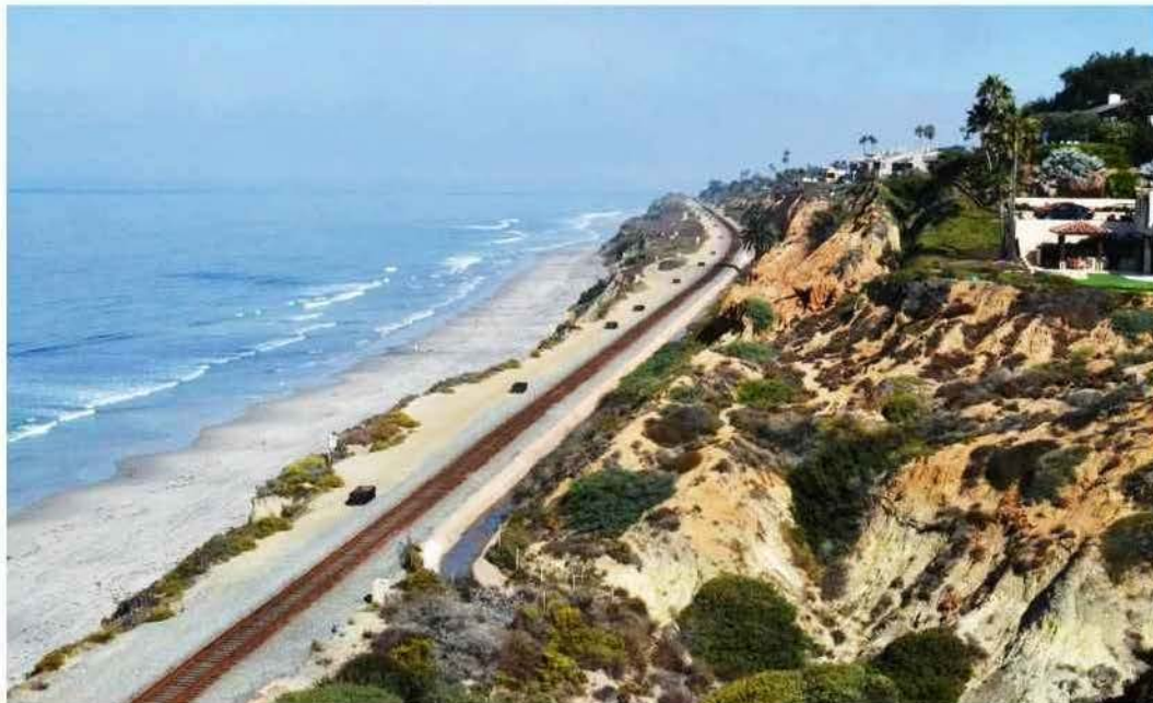
Figure 12 Steep bluffs on both sides of the railroad corridor in Del Mar encourage its use as a north-south pathway. Looking north from the vicinity of Carmel Valley Road near MP 245.5. (Source: WSP)
