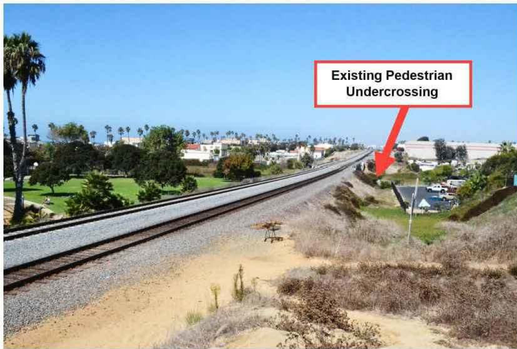
Figure 6 This common trespassing site in Oceanside is only 400 feet south of a legal pedestrian undercrossing that provides access to Buccaneer Beach Park and other coastal resources and connects to Coast Highway. Looking north from Morse Street near MP 227.7. (Source: WSP)
