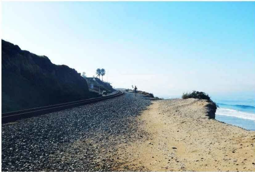
Figure 13 Joggers frequently use the railroad corridor in Del Mar as a north-south pathway. Looking south from the vicinity of 15th Street near MP 244.2. (Source: WSP)
