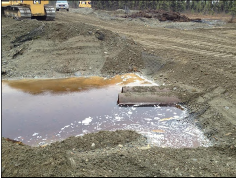
Figure 17: Newly located 12" pipes inlet on project left after water flow is reestablished. May 6, 2014.
