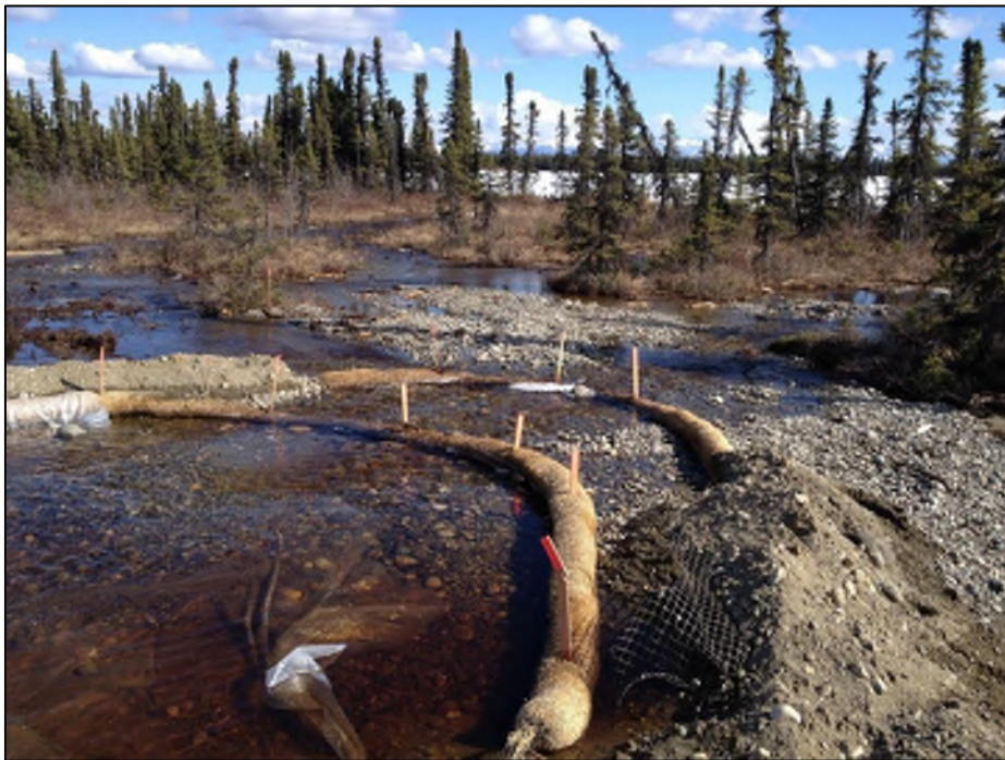
Figure 8: Outlet of the two 12" pipe with sediment mitigation measures in place. April 24, 2014.
