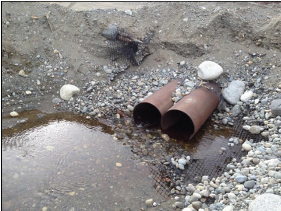
Figure 14: Inlet on project left to move impounded water with two 16" pipes. May 5, 2014. Notice the level of the impounded water has dropped significantly since April 22, 2014.
