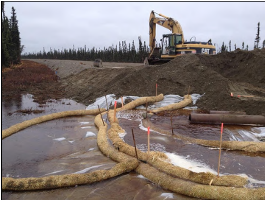
Figure 18: Newly located 12" pipes outlet on project right after water flow is reestablished. May 6, 2014.
