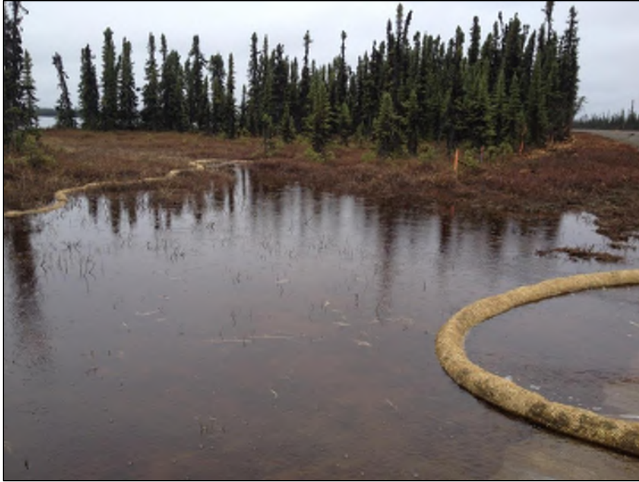
Figure 19: Southern most section of filled wetlands cleaned of fill on project right. Location of outlet for new 12" pipe water diversion. May 6, 2014.
