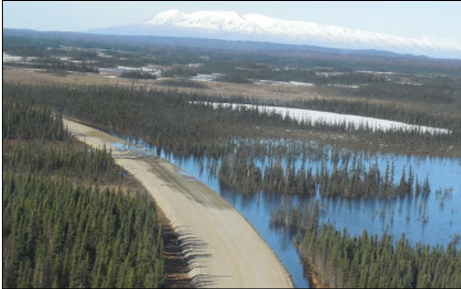
Figure 1: Aerial photograph of impounded water on project left between STA4600 and STA4615. April 21, 2014.
