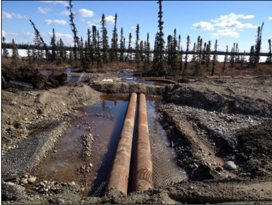
Figure 7: Long pipe moving impounded water toward the outlet and Muleshoe Lake. April 24, 2014.
