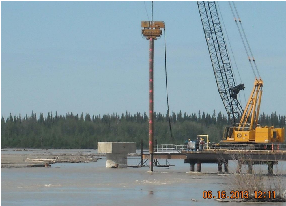
Figure 3. Pile driving for Trestle Build. Photographed June 16, 2013.
