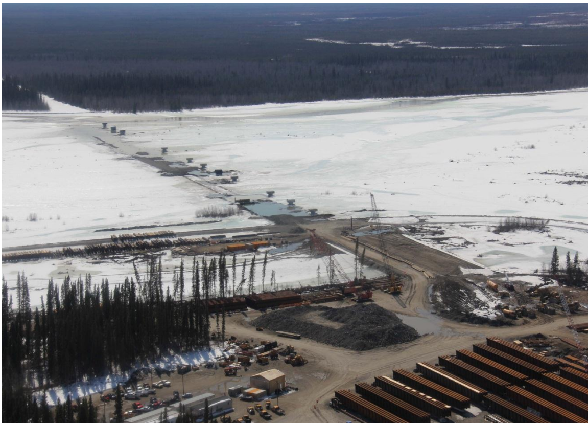
Figure 1. Overview of alignment and yard. Photographed May 10, 2013
