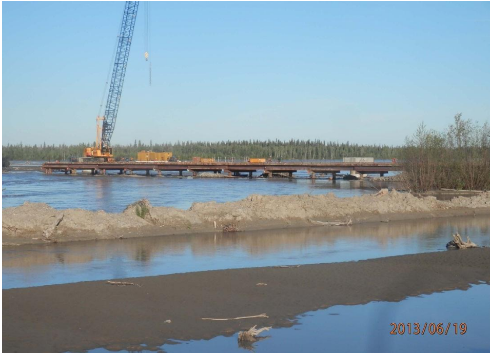
Figure 4. Trestle Progress, Photographed June 19, 2013
