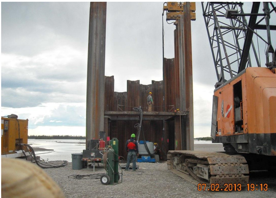
Figure 5. Cofferdam at Pier 10, Photographed July 2, 2013
