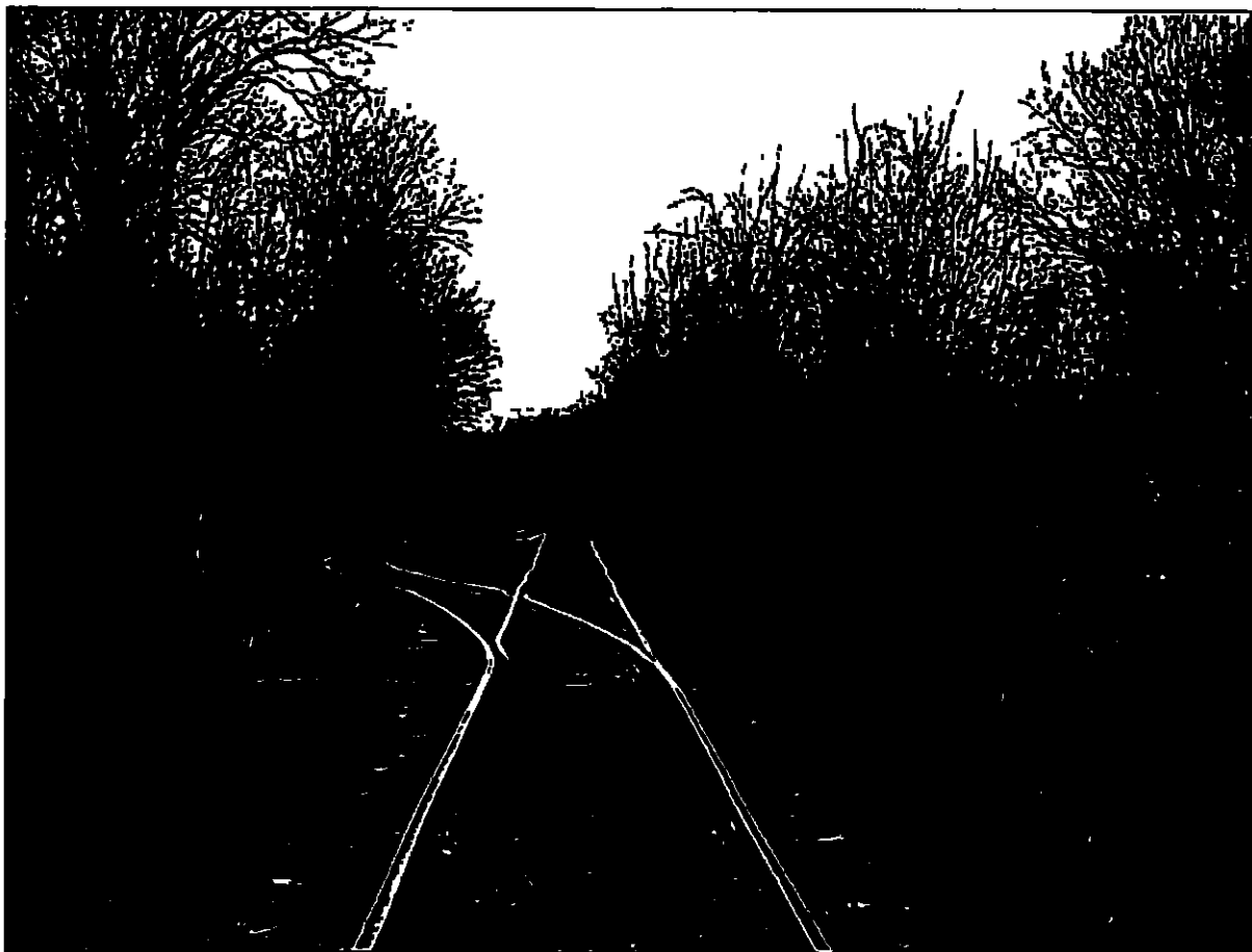
Cooper Lighting Switch (Foam Packaging Transload Area) (looking South)
