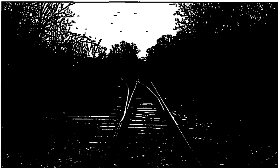
Entergy Baxter Wilson Plant Switch (looking North)
